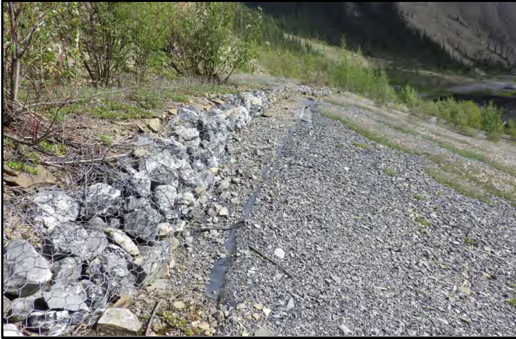
Photo B5: Water Storage Pond, Side 1A Crest of slope looking east. Gabions shown along crest of slope. (photo taken August 21, 2024)
