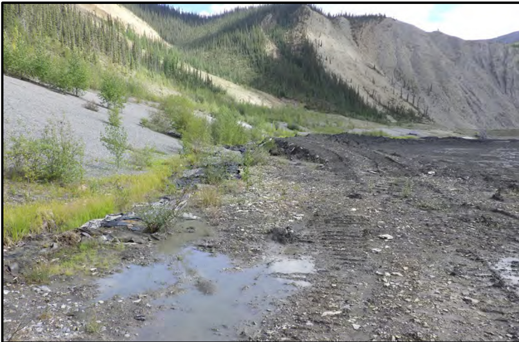
Photo B6: Water Storage Pond, Side 1A Toe of slope looking northeast. Exposed liner and stockpiled pond sediments shown. (photo taken August 21, 2024)
