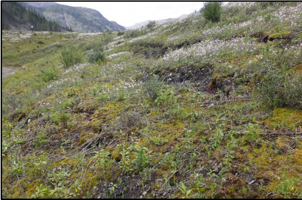
Photo B37: Water Storage Pond, Side 3B Middle of pond side slope looking southeast. Slumping and scarps shown on slope. (photo taken August 21, 2024)
