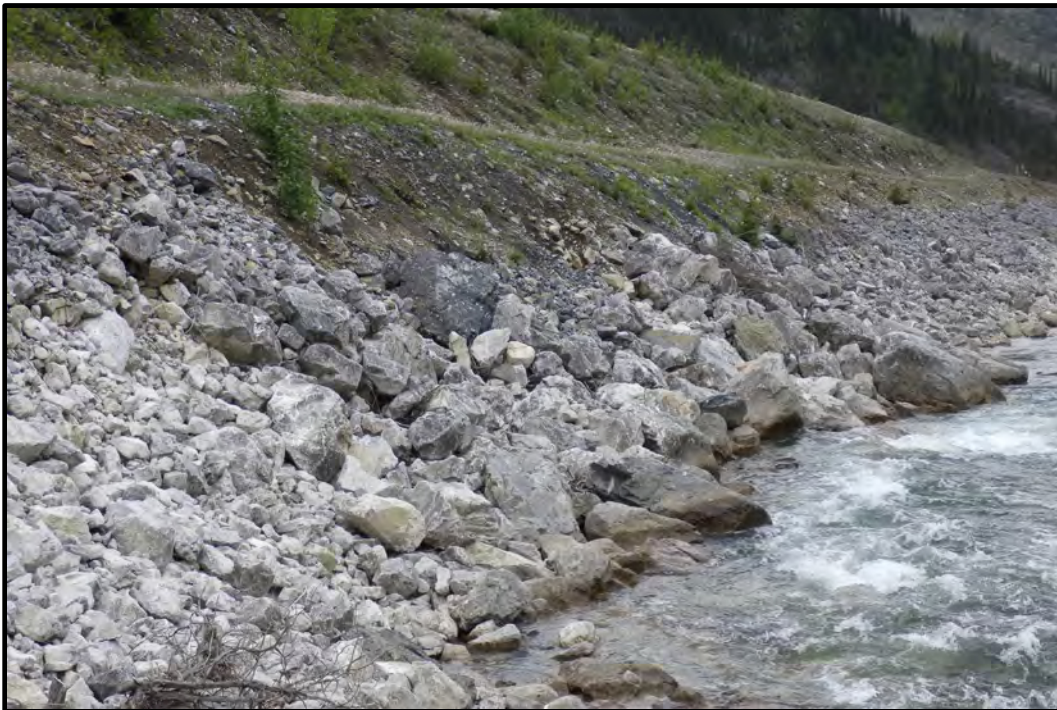
Photo B32: Water Storage Pond, Side 3B Toe of creek side slope looking northeast. Riprap erosion and settlement shown. (photo taken August 21, 2024)
