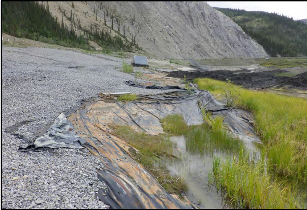
Photo B11: Water Storage Pond, Side 1B Edge of pond looking east. Exposed liner shown along toe of slope. (photo taken August 21, 2024)
