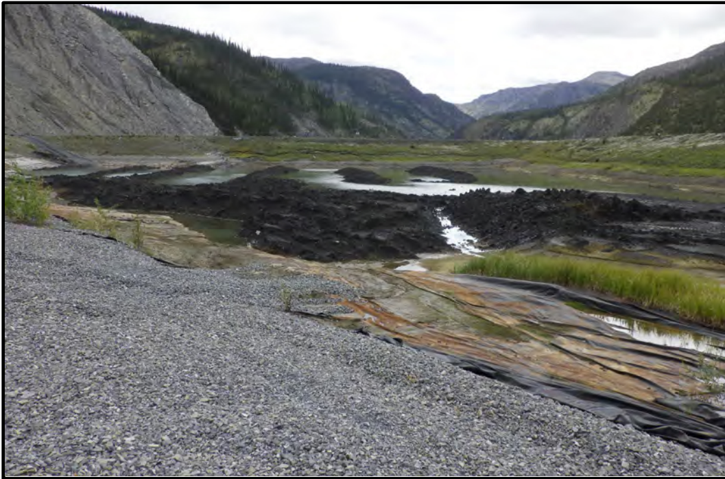
Photo B13: Water Storage Pond, Side 1B Toe of slope looking southeast. Exposed liner and stockpiled pond sediment shown. (photo taken August 21, 2024)
