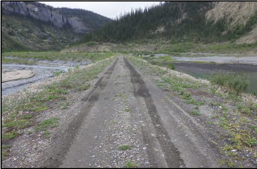
Photo B35: Water Storage Pond, Side 3B Top of embankment looking northwest. Minor rutting shown along top. (photo taken August 21, 2024)
