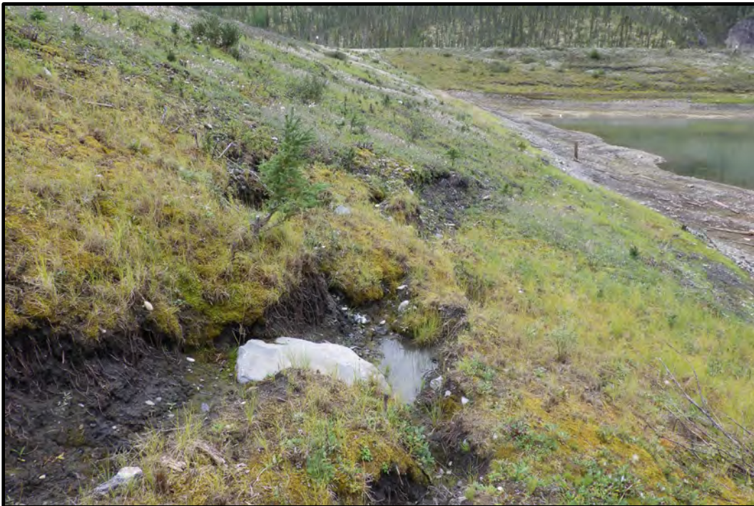
Photo B42: Water Storage Pond, Side 4 Middle of pond side slope looking southwest. Slumping and scarps shown on slope. (photo taken August 21, 2024)
