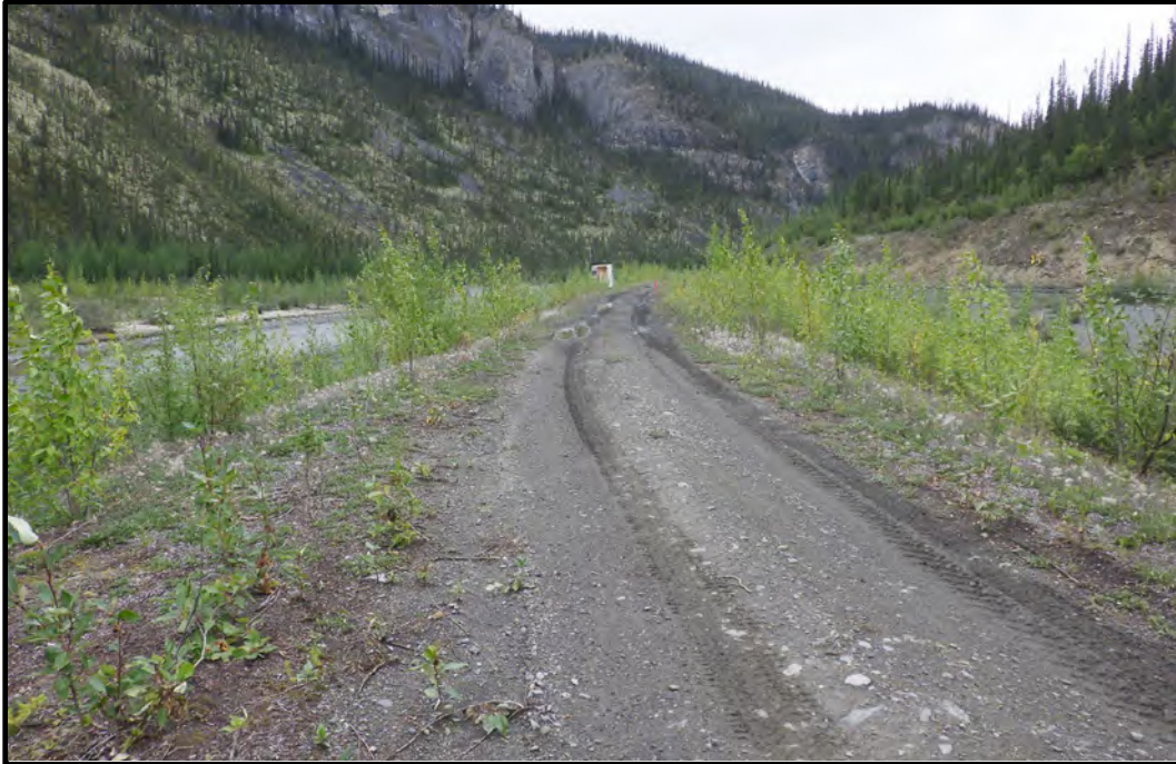
Photo B23: Water Storage Pond, Side 2 Top of embankment looking northwest. Moderate vegetation shown on side slopes. (photo taken August 21, 2024)
