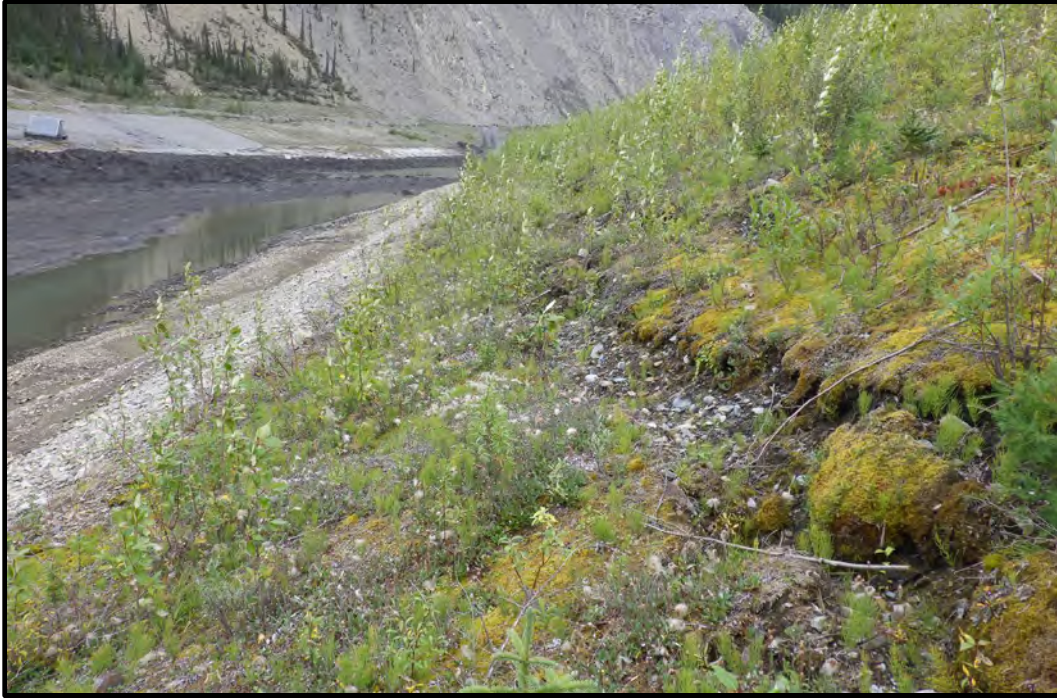
Photo B27: Water Storage Pond, Side 3A Middle of pond side slope looking east. Old slumping and scarps shown along slope. (photo taken August 21, 2024)
