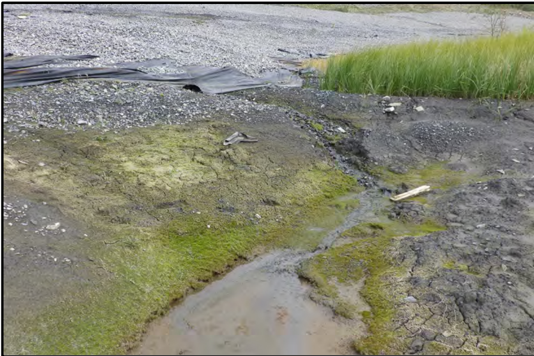
Photo B12: Water Storage Pond, Side 1B Toe of slope looking northeast. Water seepage shown from behind old liner. (photo taken August 21, 2024)
