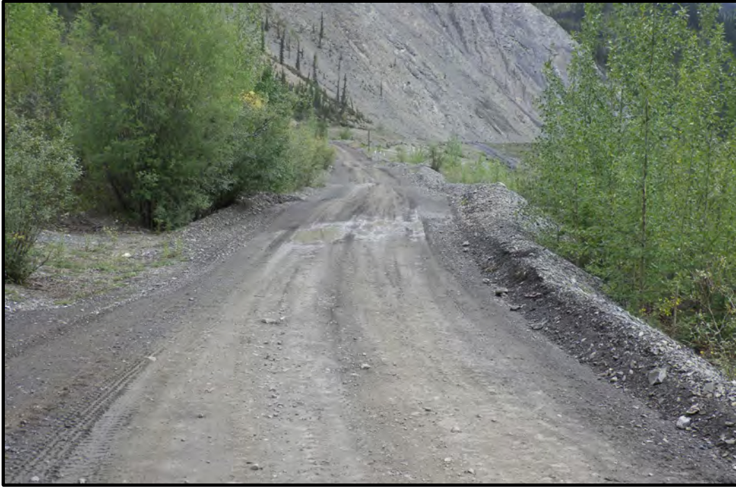
Photo B9: Water Storage Pond, Side 1B Access road on top of embankment looking east. Ponding and subsidence shown. (photo taken August 21, 2024)
