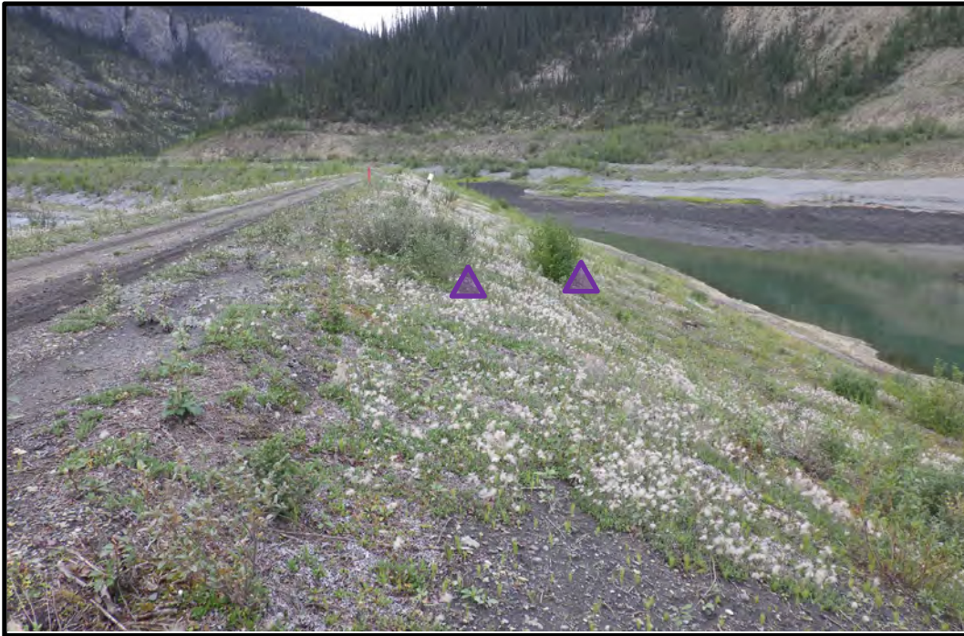
Photo B39: Water Storage Pond, Side 3B Crest of pond side slope looking northwest. Animal burrows shown on slope. (photo taken August 21, 2024)
