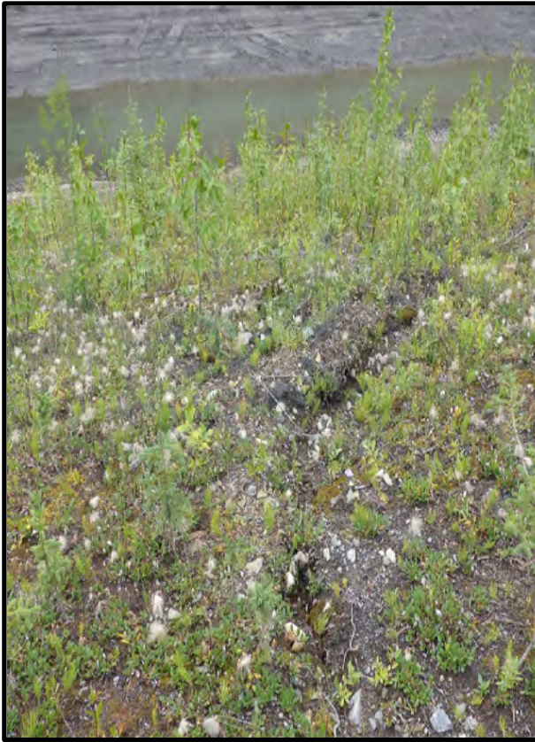
Photo B29: Water Storage Pond, Side 3A Crest of slope near corner with Side 3B looking north. Erosion gully shown from crest of embankment on pond side slope. (photo taken August 21, 2024)
