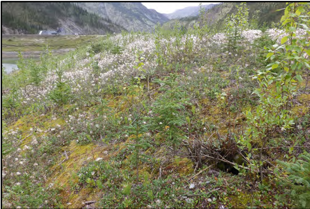
Photo B36: Water Storage Pond, Side 3B Crest of pond side slope looking southeast. Animal burrow shown in slope. (photo taken August 21, 2024)
