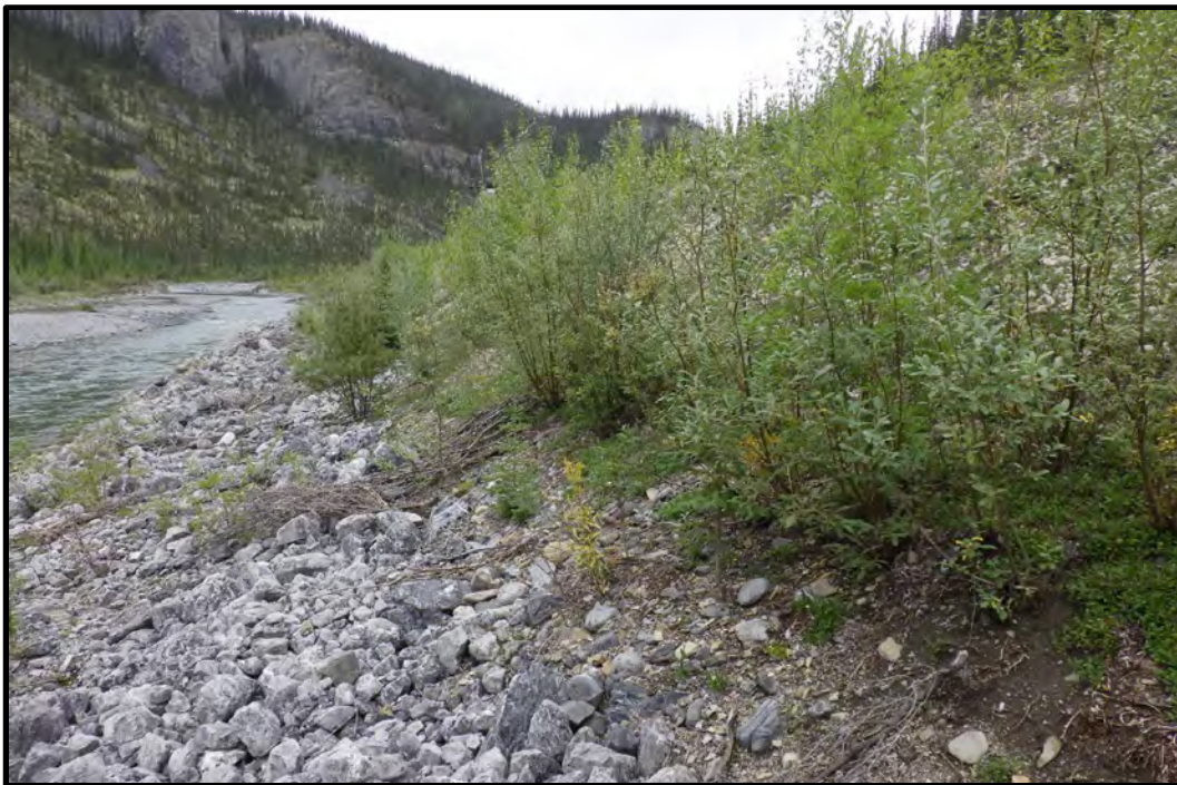
Photo B20: Water Storage Pond, Side 2 Toe of creek side slope looking northwest. Old creek debris shown on top of riprap. (photo taken August 21, 2024)
