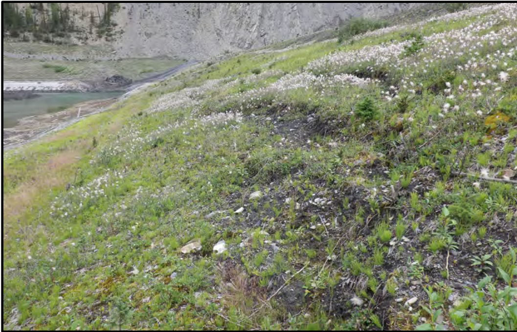
Photo B41: Water Storage Pond, Side 4 Middle of pond side slope looking northeast. Slumping and scarps shown on slope. (photo taken August 21, 2024)
