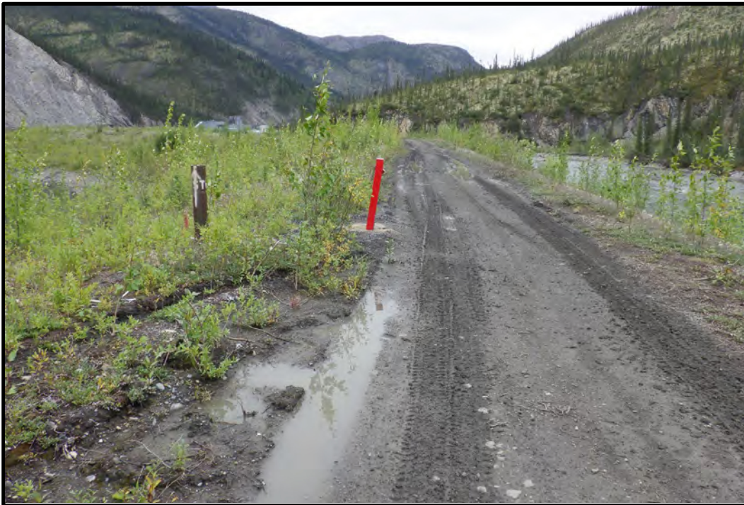
Photo B22: Water Storage Pond, Side 2 Top of embankment looking southeast. Rutting and ponded water shown along top. (photo taken August 21, 2024)
