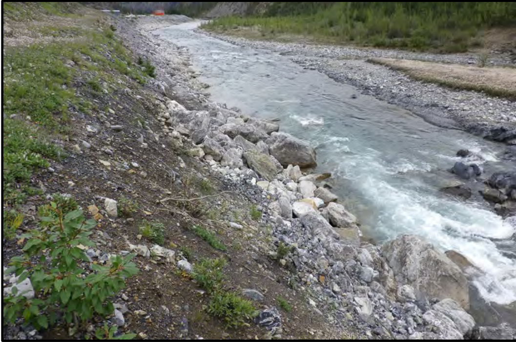
Photo B33: Water Storage Pond, Side 3B Middle of creek side slope looking southeast. Riprap erosion and settlement shown. (photo taken August 21, 2024)
