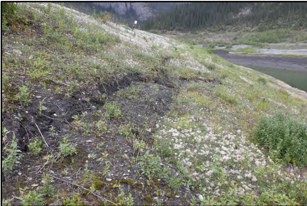
Photo B38: Water Storage Pond, Side 3B Middle of pond side slope looking northwest. Slumping and scarps shown on slope. (photo taken August 21, 2024)
