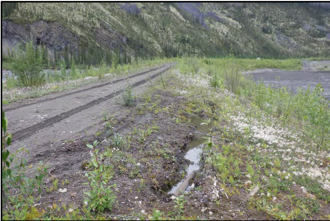
Photo B26: Water Storage Pond, Side 3A Top of embankment looking west. Rutting and ponding water shown. (photo taken August 21, 2024)
