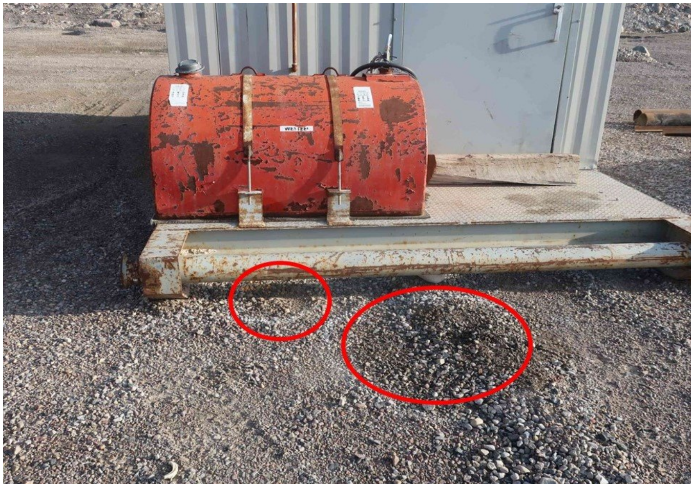
Figure 8 Spills (circled in red) on the east side of the pit previously noted that require cleanup.
