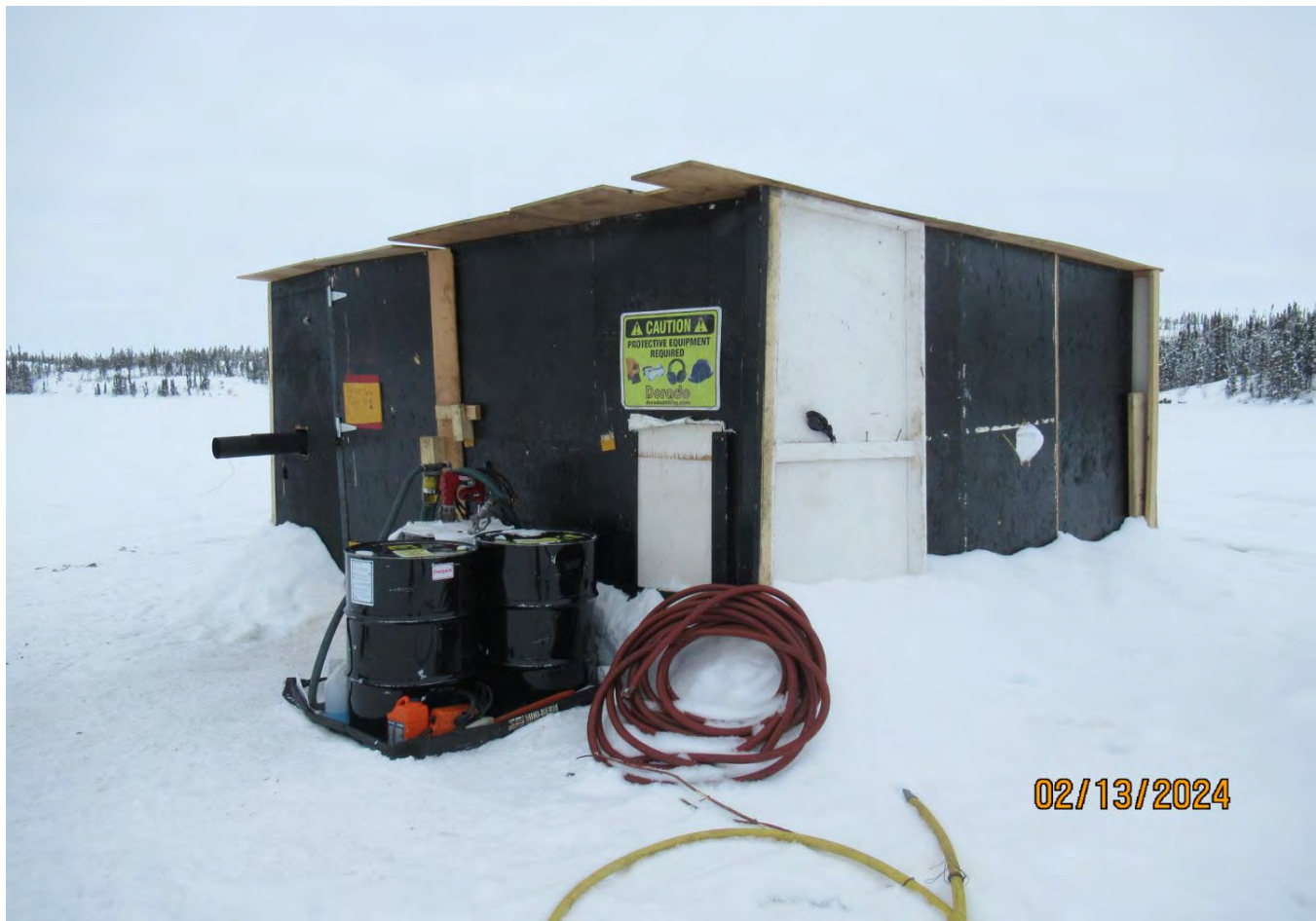
Figure 44 Ancillary equipment in the pump shack has secondary containment and fuel containers tertiary containment.
