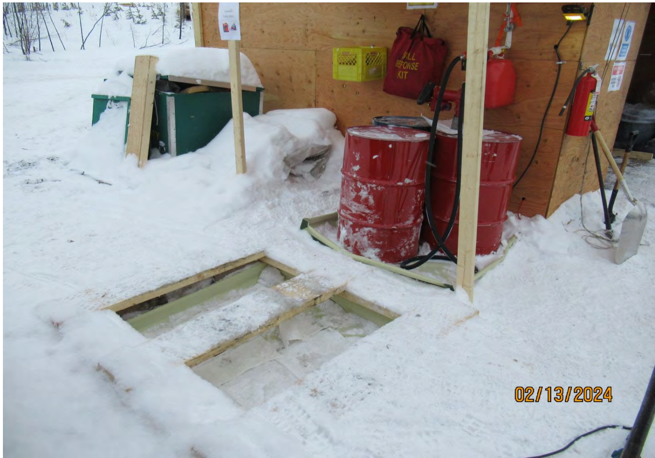
Figure 26 Gasoline drums have been placed in secondary containment and snowmobiles are being fueled overtop of this secondary containment structure.
