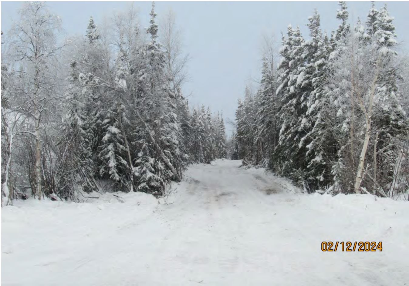
Figure 4 Initial icing of the portages is underway. As a reminder the portages must be iced in from shoulder to shoulder to comply with Condition #18 of the land use permit.
