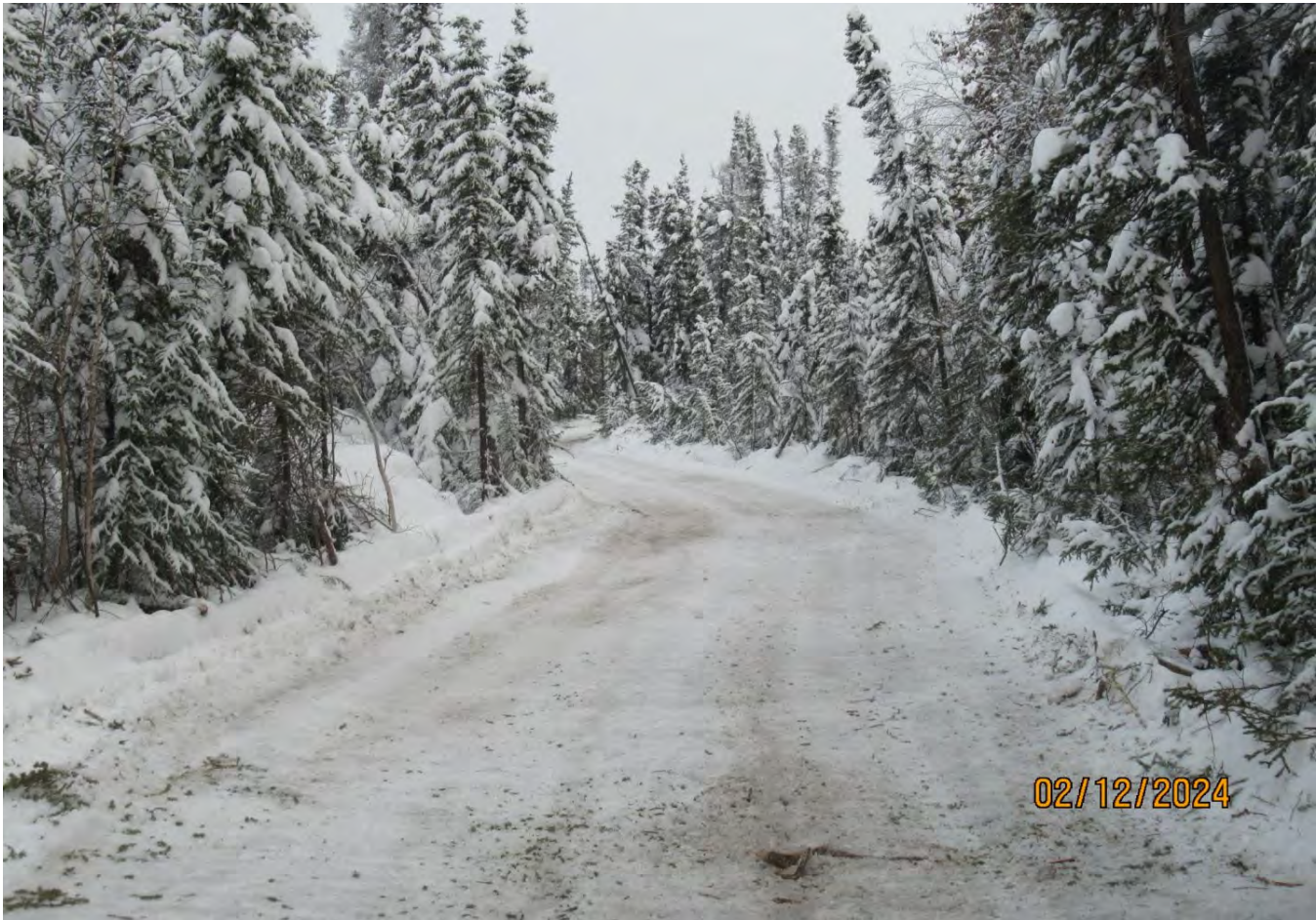
Figure 4 Initial icing of the portages is underway. As a reminder the portages must be iced in from shoulder to shoulder to comply with Condition #18 of the land use permit.
