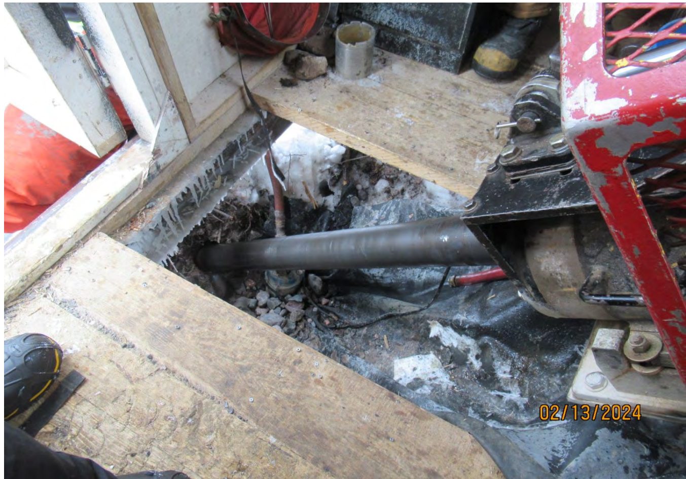
Figure 46 A pond liner and submersible pump are being used to collect drill waste for pumping to a natural depression when setting casing.
