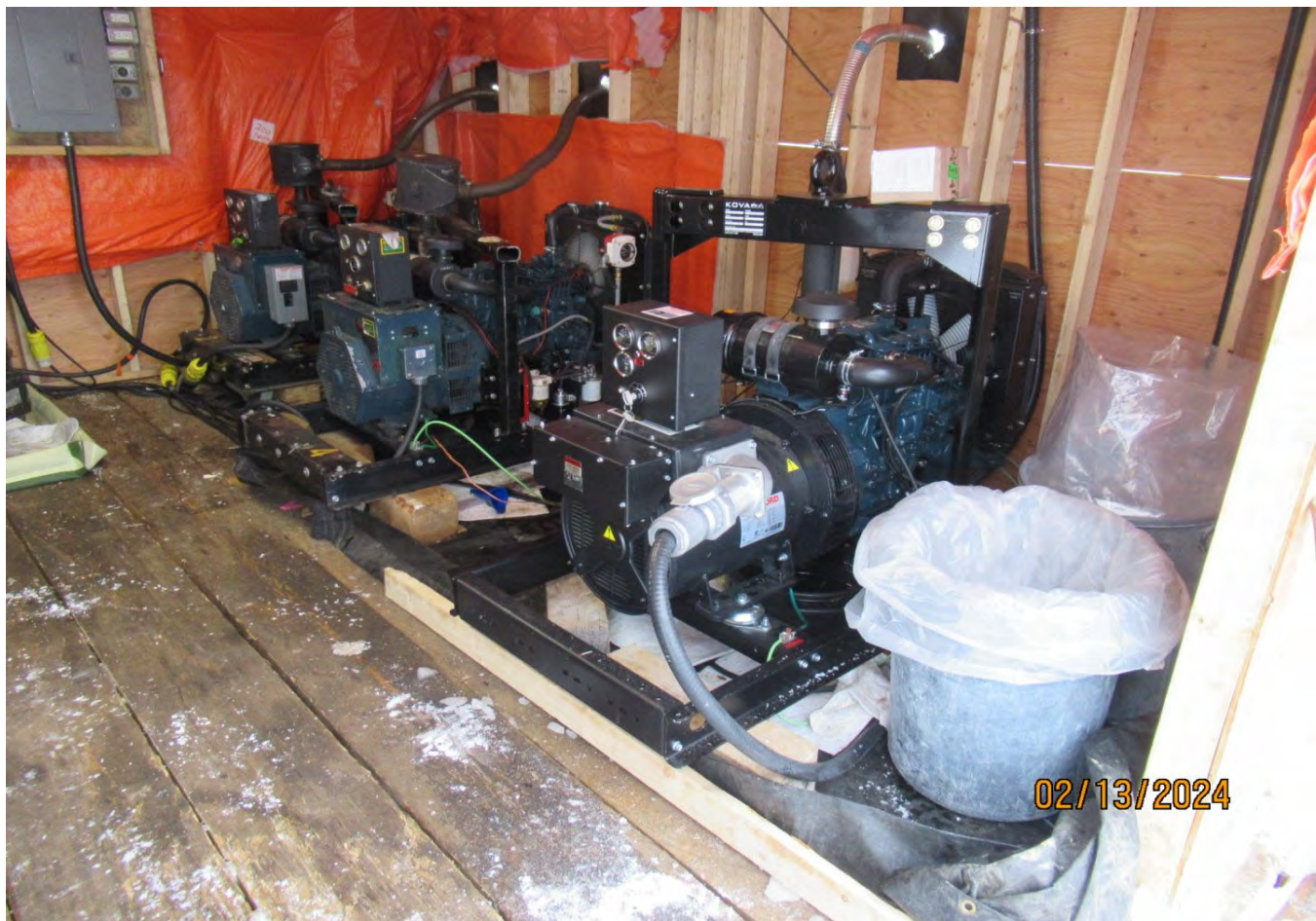
Figure 28 Camp generators have secondary containment present.
