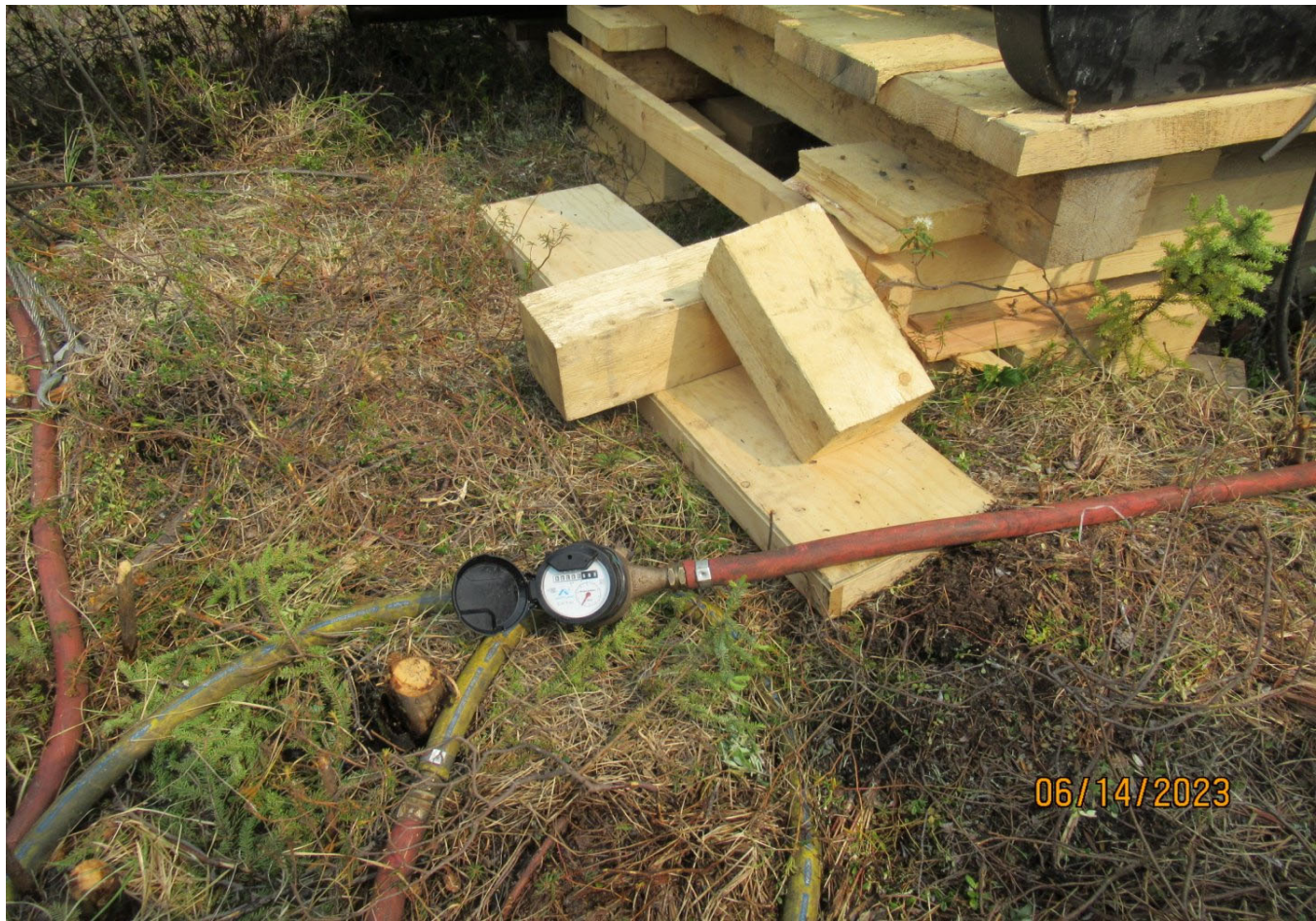
Figure 6 Water use is being metered at the Dorado drill. Volumes are being recorded daily.
