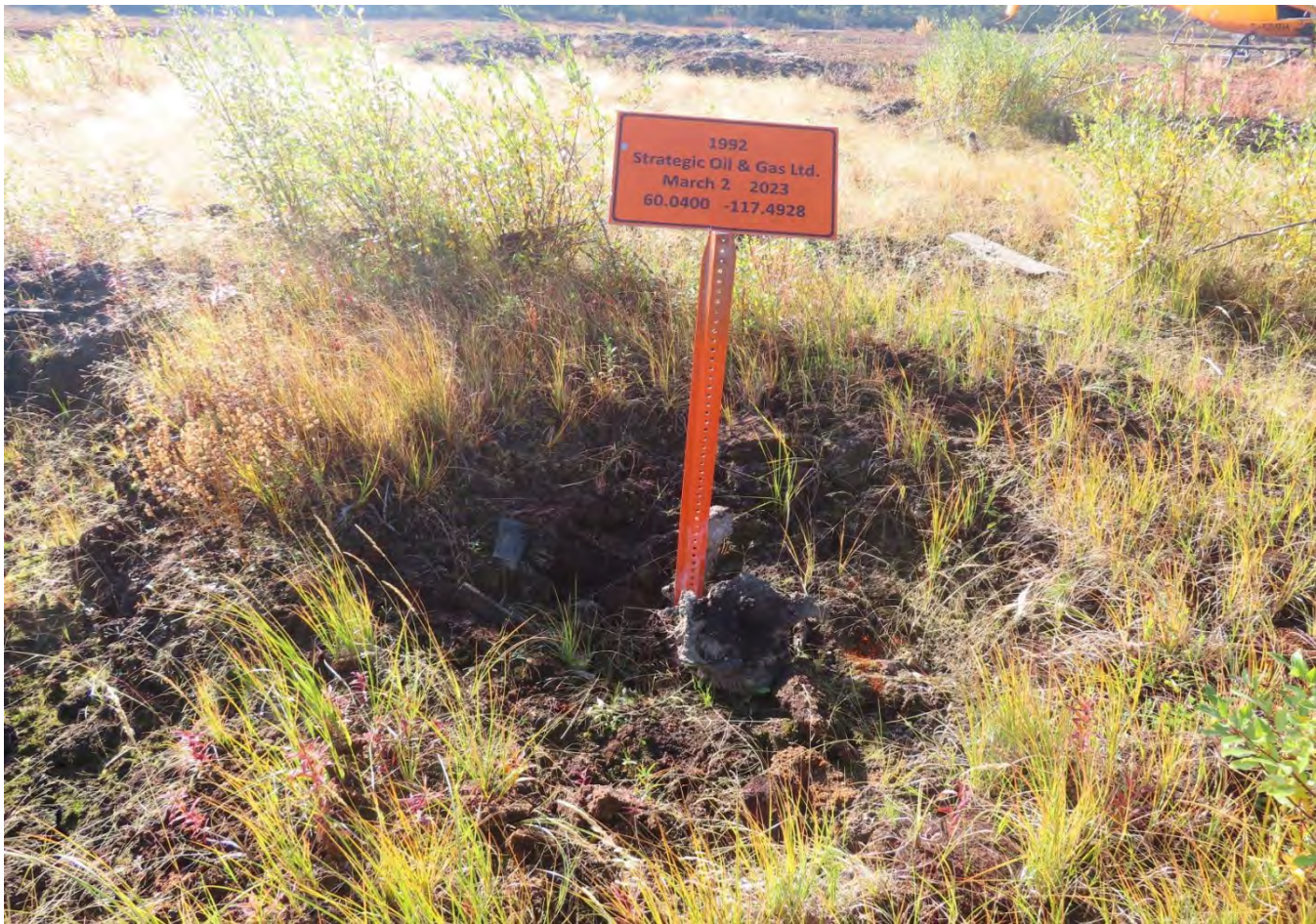
Figure 44 F-73: Backfill of F-73 well center appears satisfactory.
