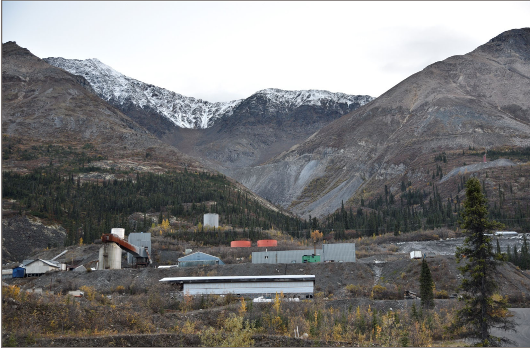
Photo 9: Waste Rock Stockpile #3 facing southwest. Waste rock pushed over existing slope during operations to form pile
