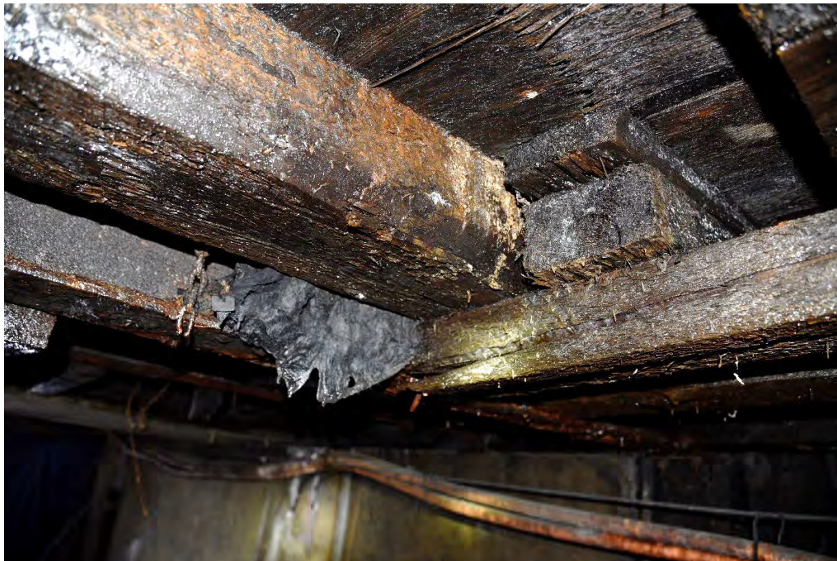
Photo 28: Cracked timber support in the crown of the Conveyor Adit.
