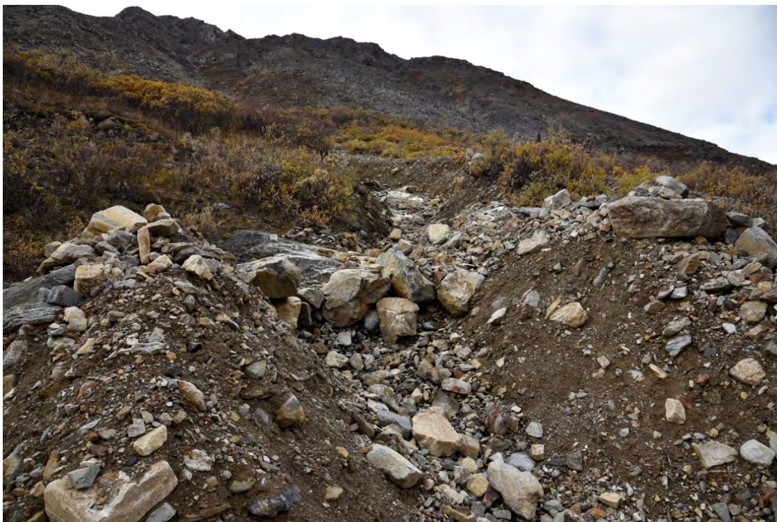
Photo 8: Drainage Channel 1 that crosses the Open Pit Access Road. Note levees potentially formed by debris flows
