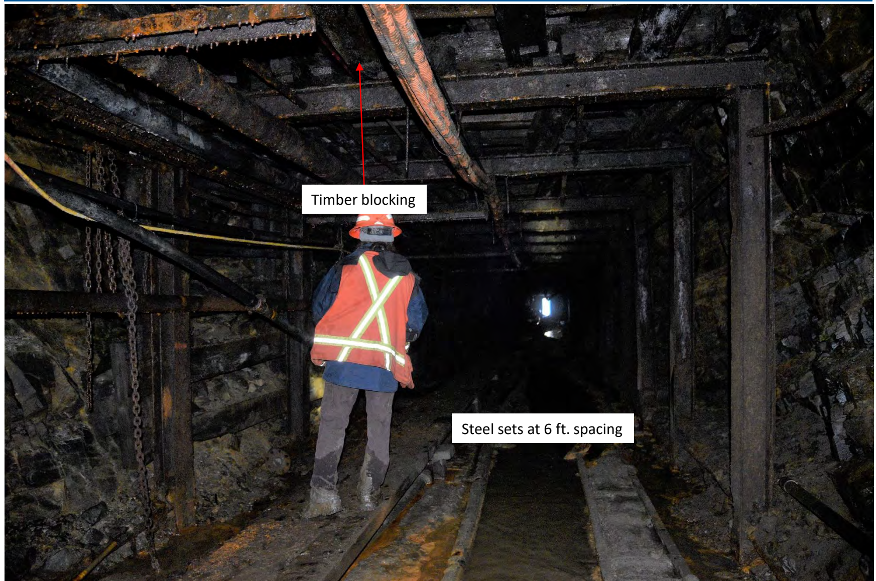
Photo 26: Steel sets with timber blocking at 70 m
