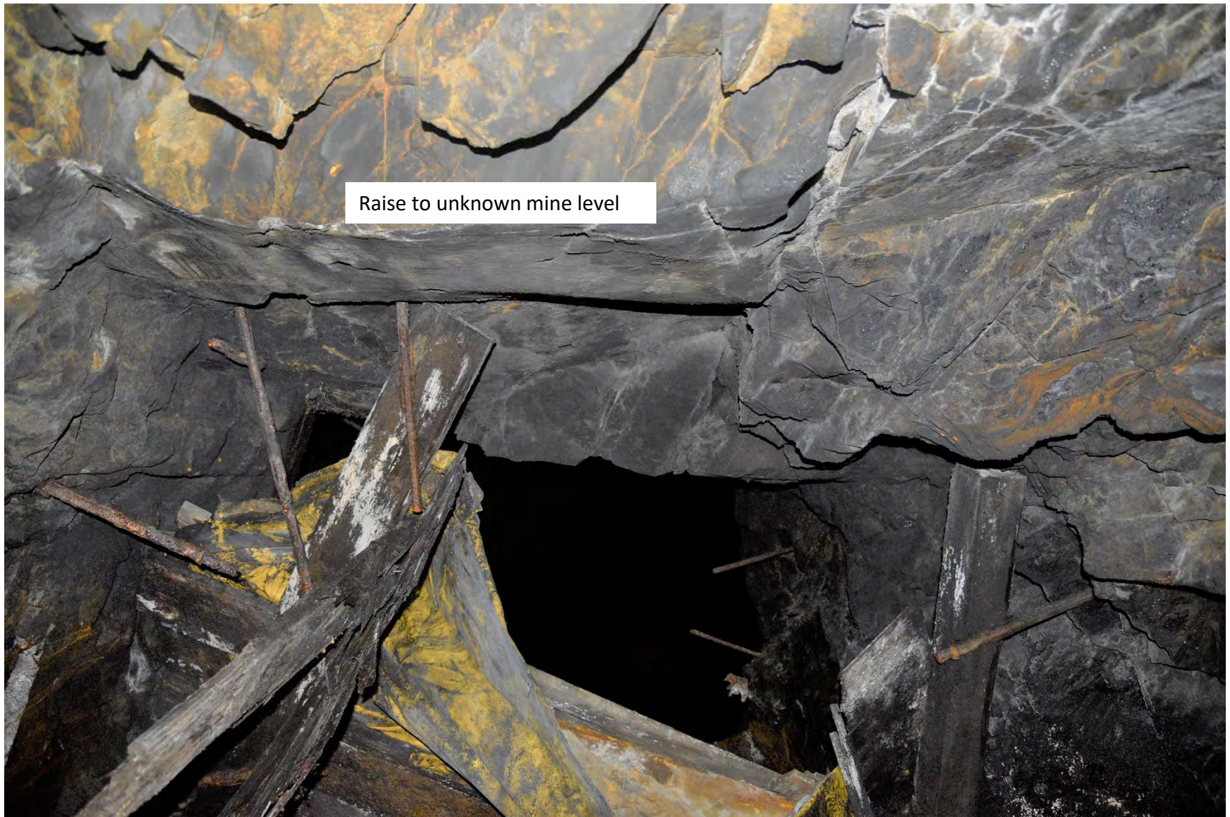
Photo 11: Raise to unknown mine level at 495 m
