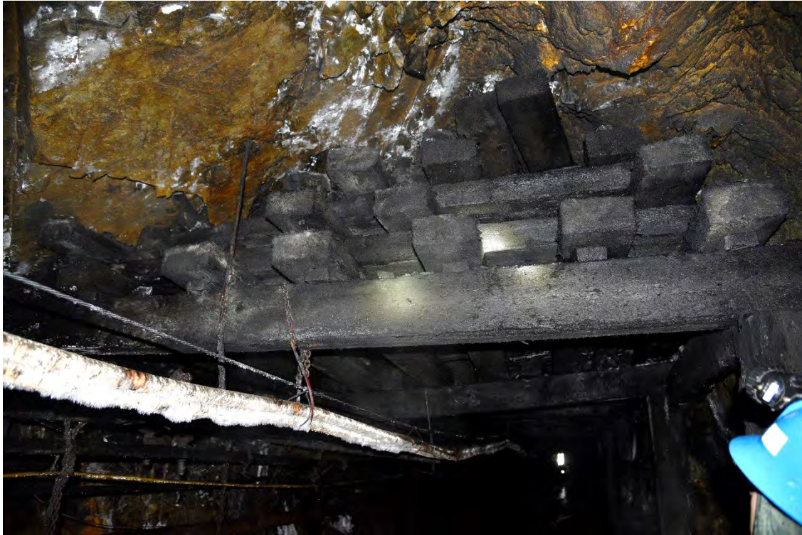
Photo 26: Conveyor Adit crown support.
