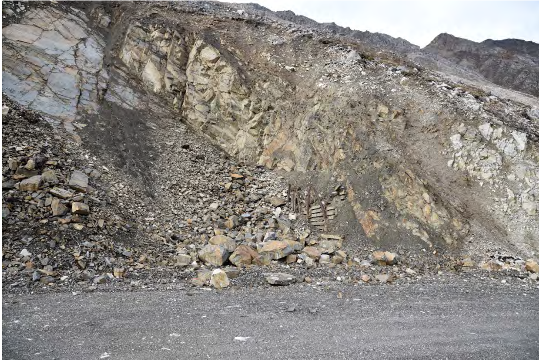
Photo 14: Remnants of the Alimak Adit visible along the Open Pit Access Road; this area should be backfilled with inert aggregate material.
