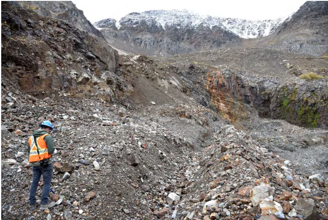
Photo 7: Rock fall berm below the upper bench-face of the Southeast Wall of the Open Pit, iron staining and seepage on the SW Wall is visible in the background.
