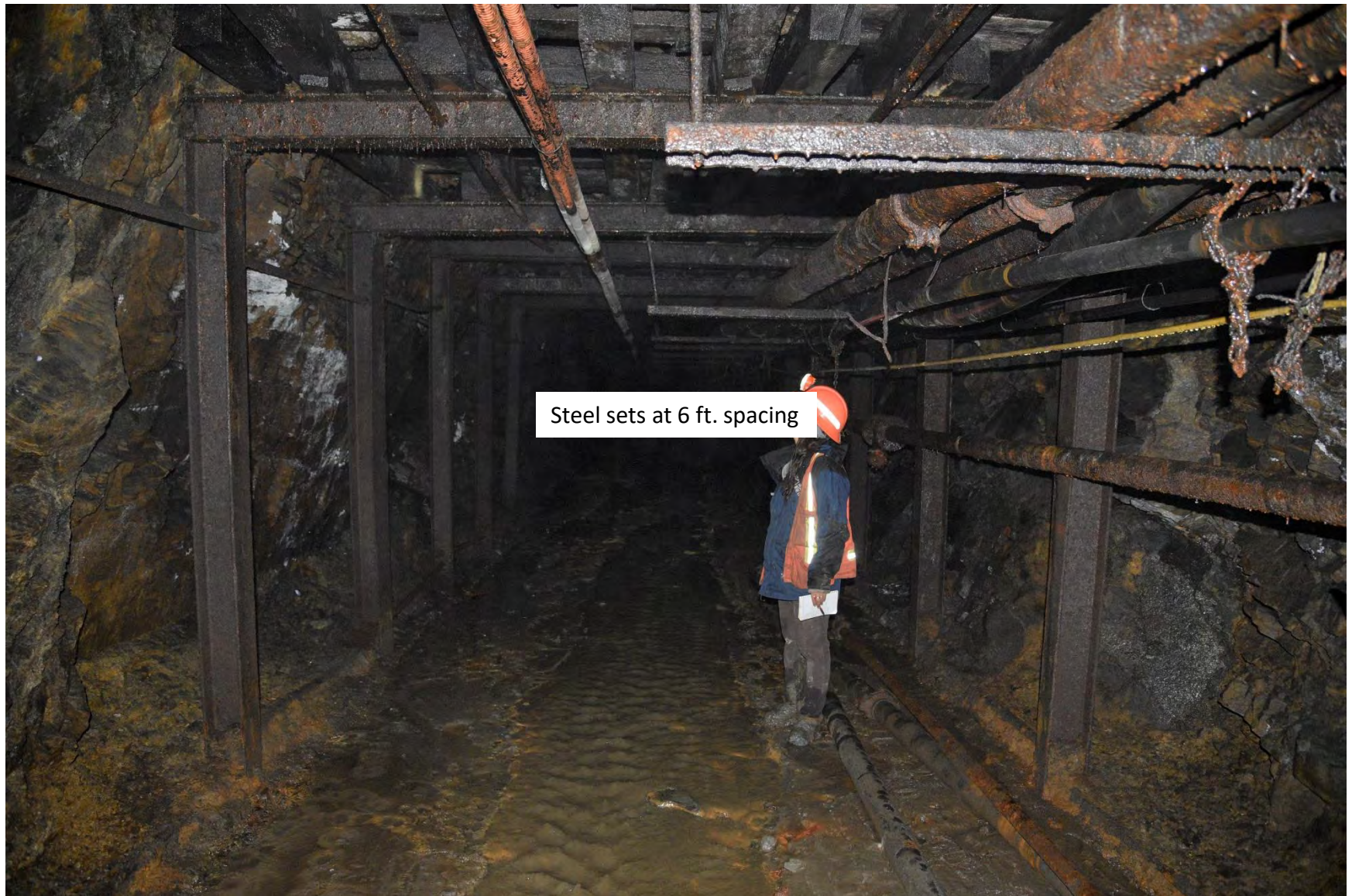
Photo 19: Steel sets from 223 to 235 m.
