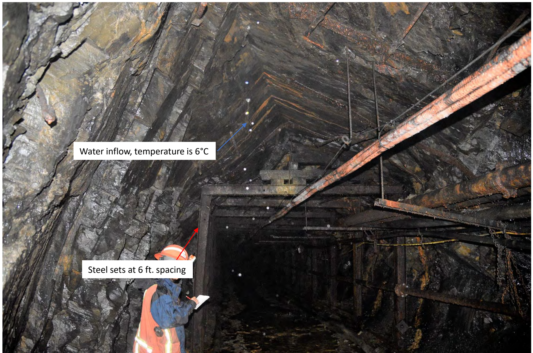
Photo 22: Water inflow temperature measurement at 154 m
