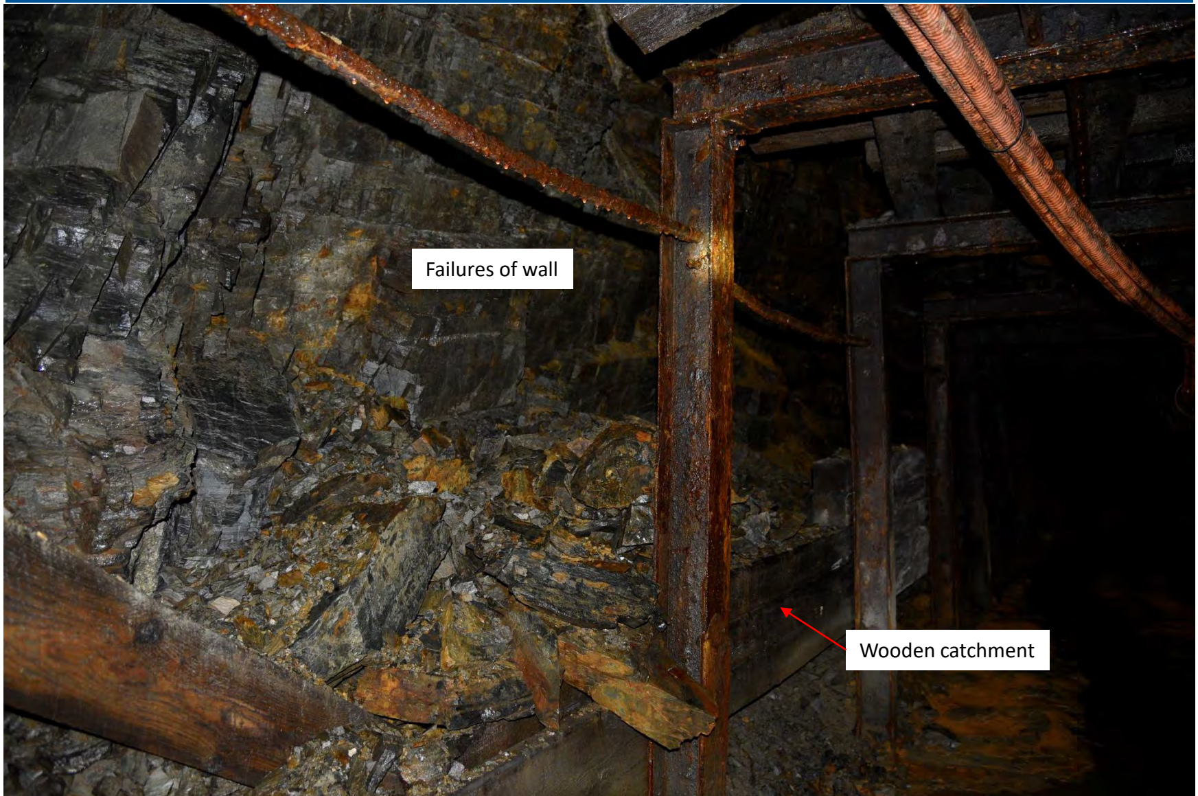
Photo 29: Failure from adit wall in wooden catchment from 20 to 30 m
