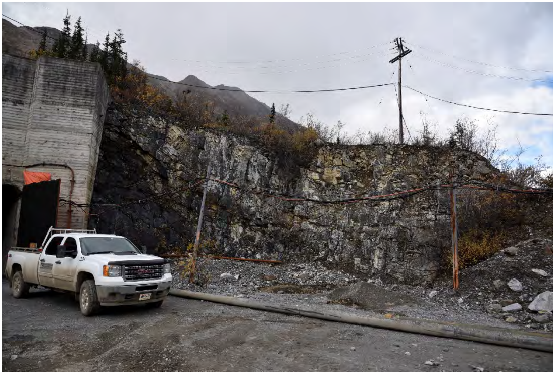
Photo 22: Northwest Slope of the Main Haulage portal. It is recommended that a 4 m setback distance be maintained for workers and equipment during closure and remediation work.
