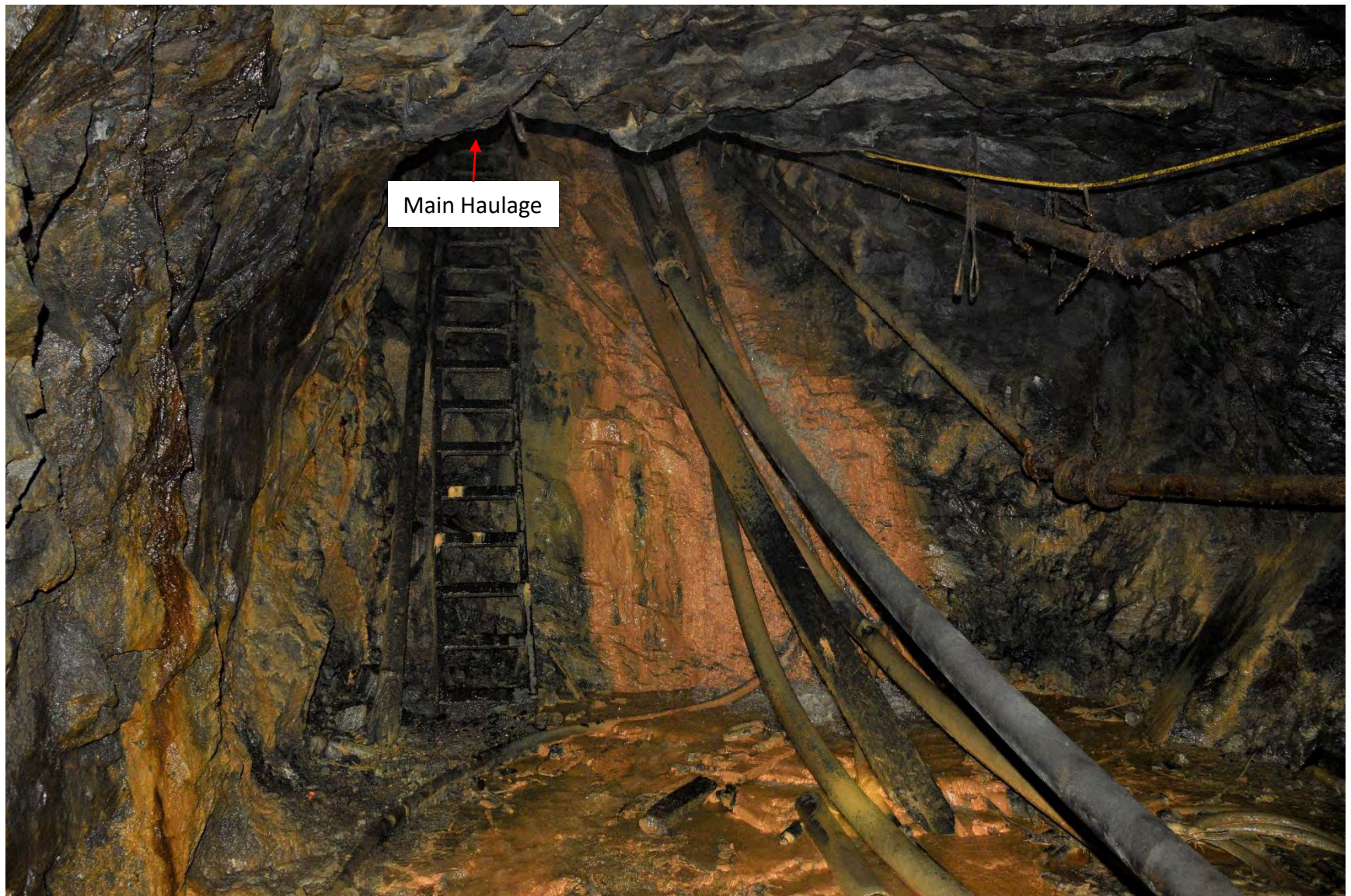
Photo 8: Inclined raise from Conveyor Adit to Main Haulage
