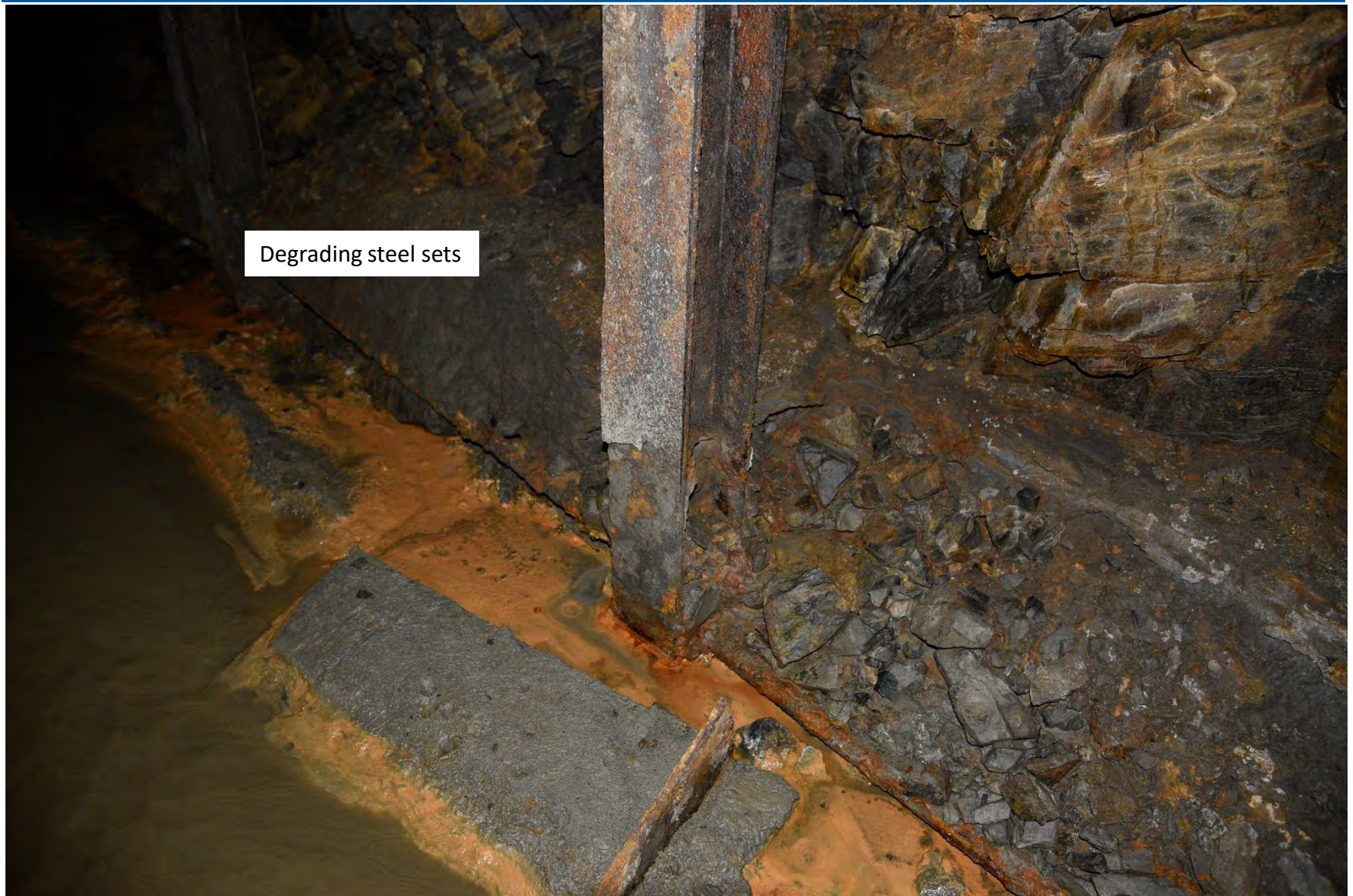
Photo 27: Highly corroded and deteriorated steel sets.
