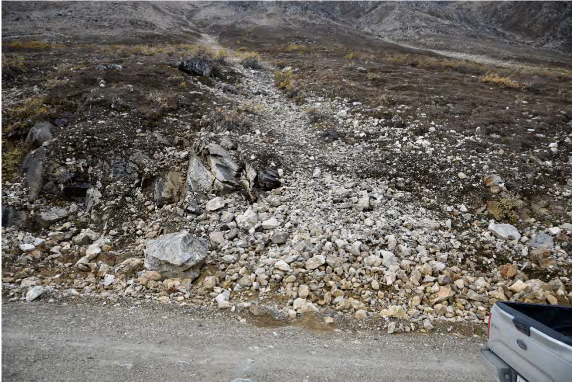
Photo 11: Drainage Channel 4 crossing the Open Pit Access Road.
