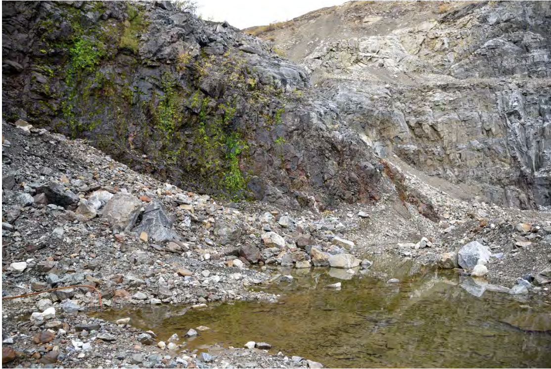
Photo 5: Southwest wall of the Open Pit showing seepage through the upper bench-face, ponding water on the upper-middle bench, and the rock fall berm to the right of the photo.
