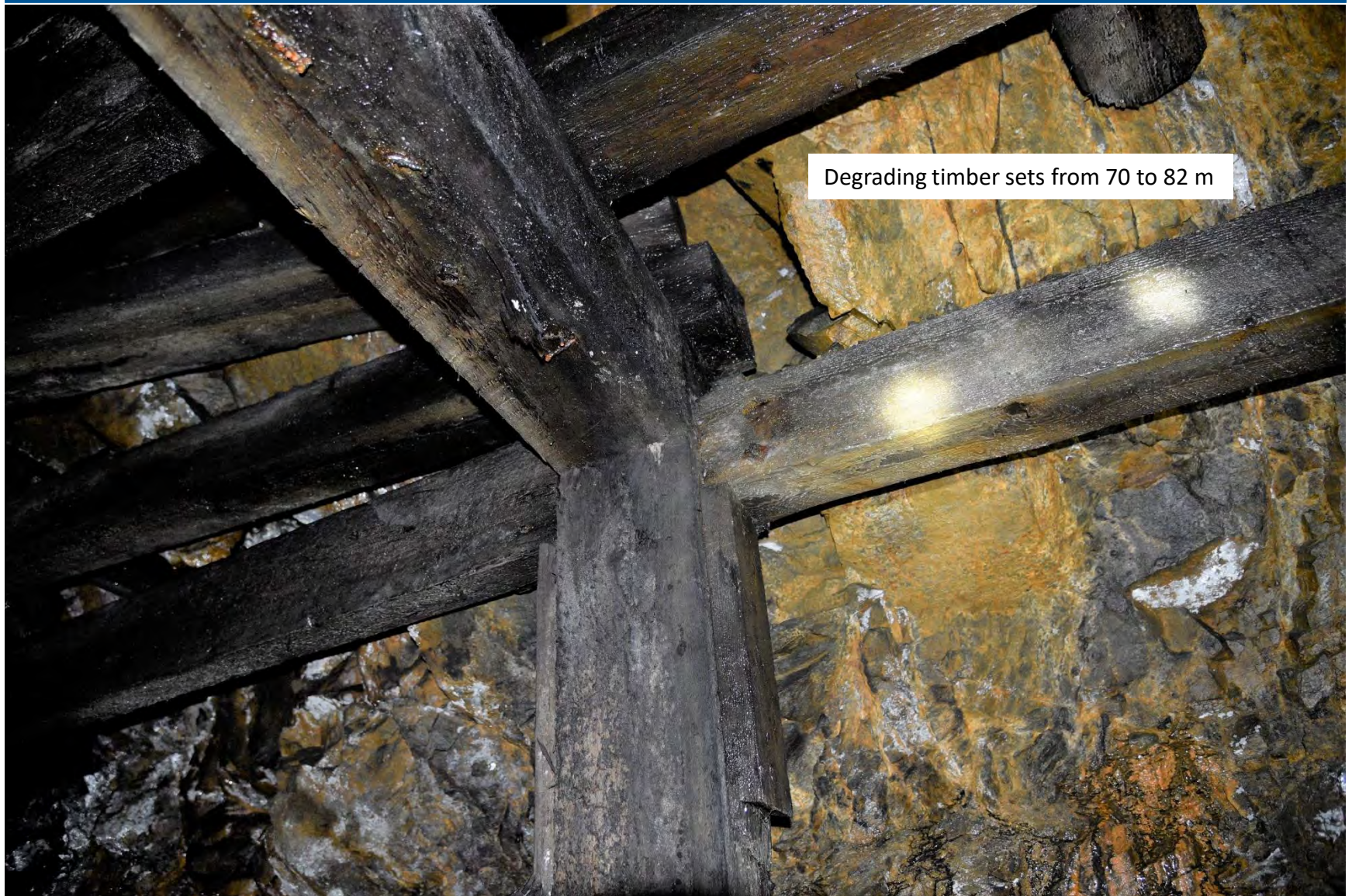
Photo 24: Degrading timber set connection
