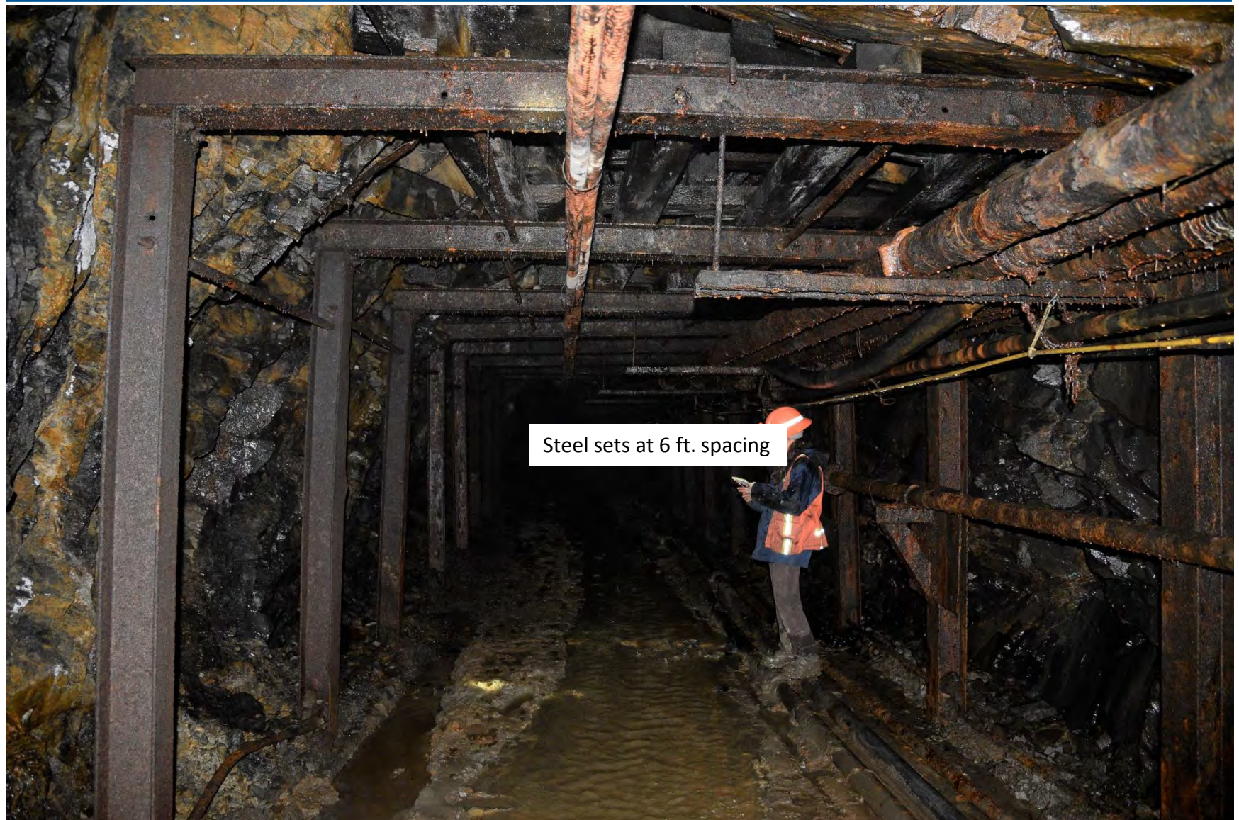
Photo 20: Steel sets from 196 to 207 m.
