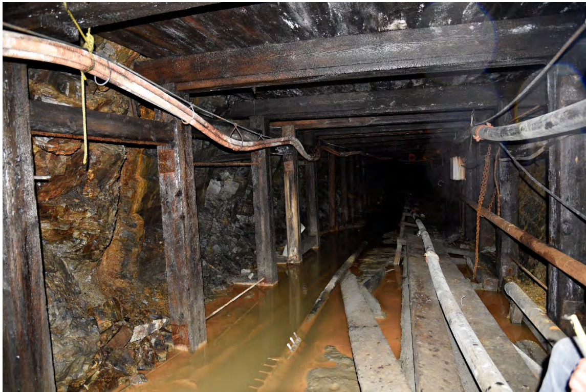
Photo 27: Conveyor Adit timber sets support, poor rock mass conditions (left), and iron staining of the rock mass and water.
