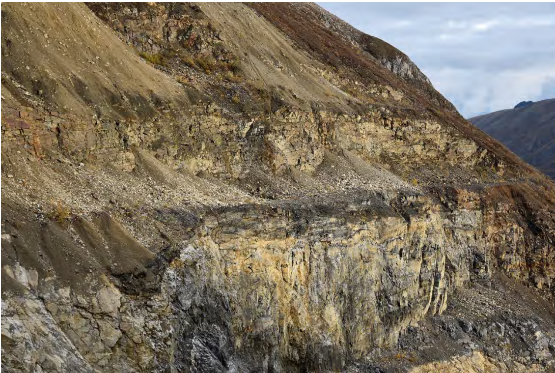
Photo 2: Upper benches of the NW wall of the Open Pit completely filled in with talus material
