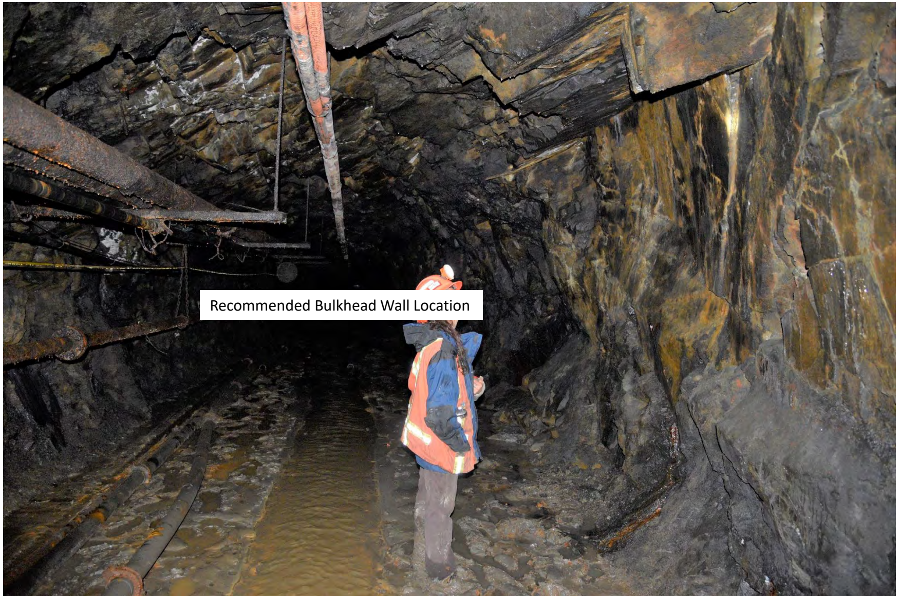
Photo 12: Recommended Bulkhead Location in Conveyor Adit (470 to 480 m)
