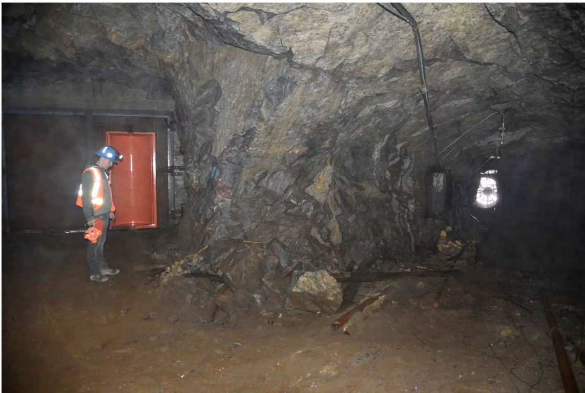
Photo 20: Stress release of the pillar at the intersection of the manway and vent portal of the Vent Adit.
