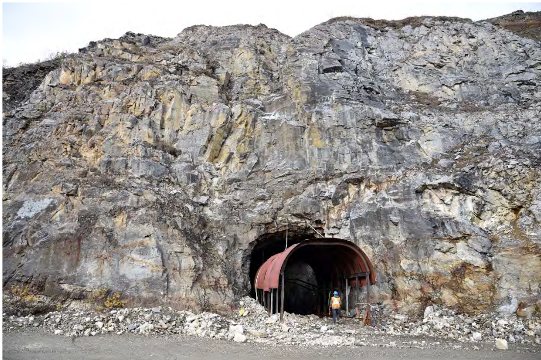
Photo 15: The PUG Portal and slope. The metal canopy structure should be removed, and slope stabilization should include an allowance for scaling and rock bolting.
