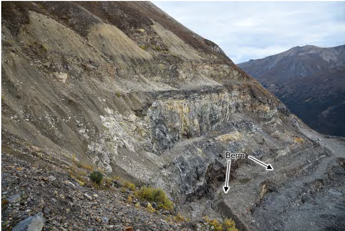
Photo 1: Northwest wall of the Open Pit showing benches filled with talus material, and rock fall berm on the second-lowest bench
