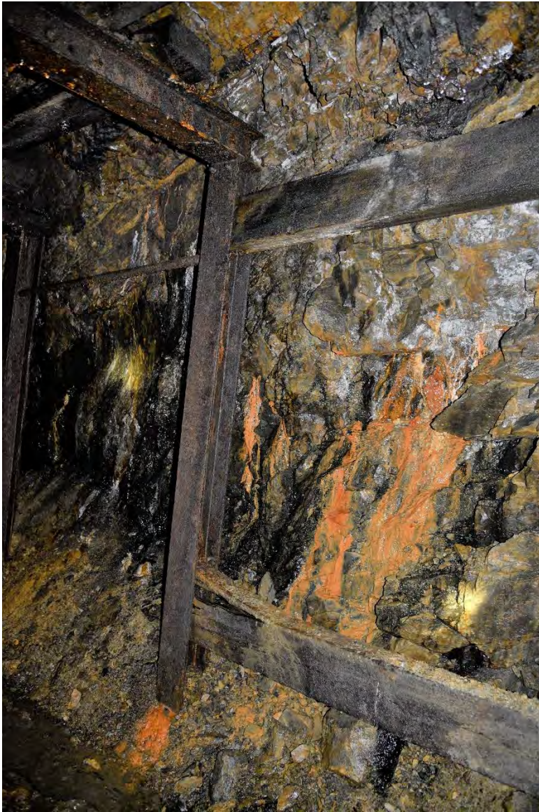
Photo 25: Current condition of timber and steel sets
