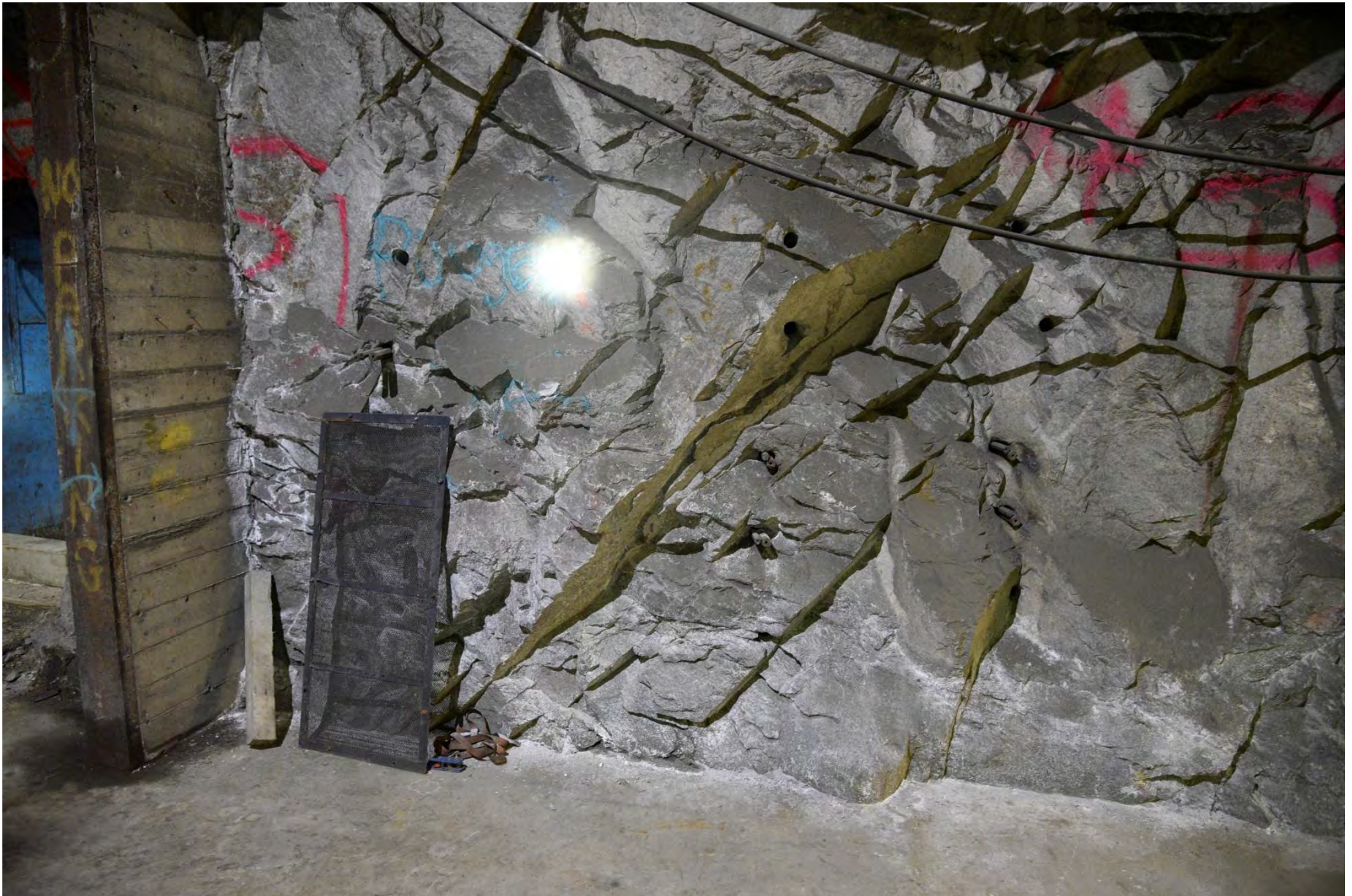
Photo 4: Jointing visible on workshop wall
