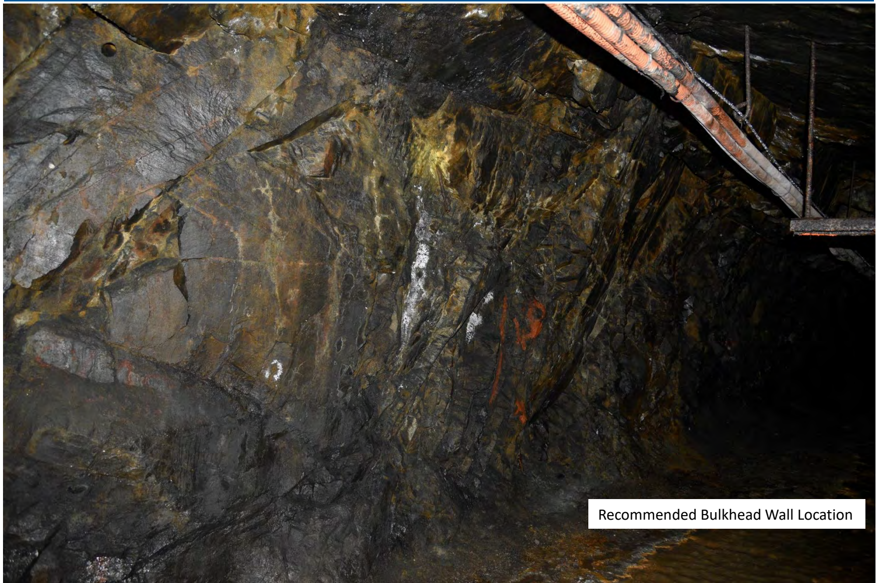
Photo 13: Rock mass at Recommended Bulkhead Location in Conveyor Adit (470 to 480 m)
