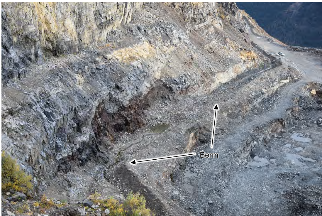
Photo 4: Lower benches of the NW wall of the Open Pit showing rock fall berm, providing effective catchment to benches below.
