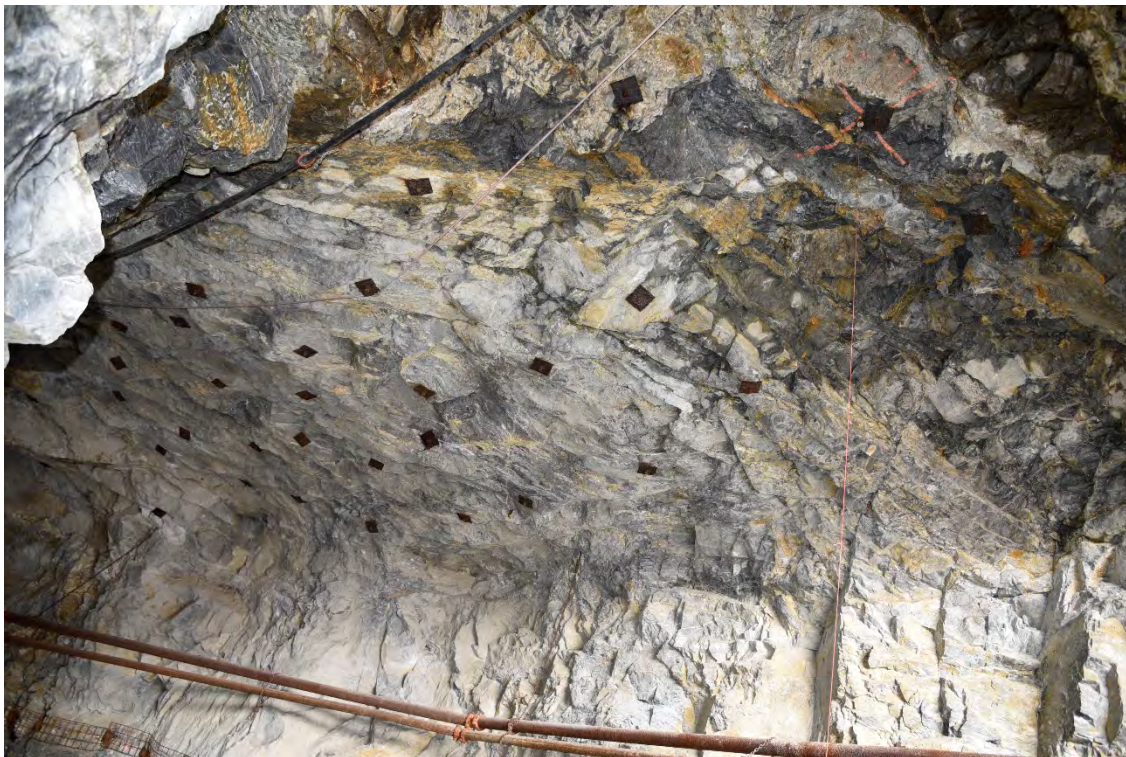
Photo 16: Pattern bolting in the crown of the PUG Adit.
