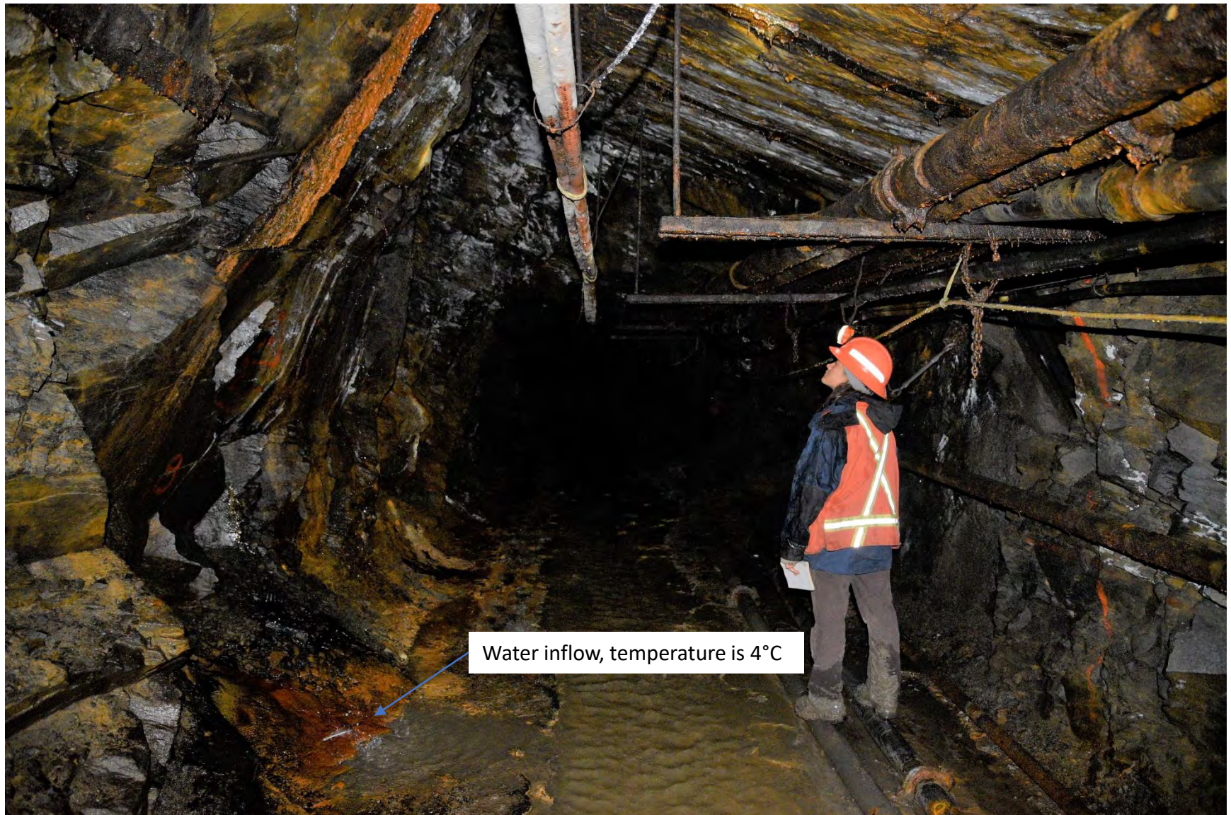
Photo 21: Water inflow temperature measurement at 157 m
