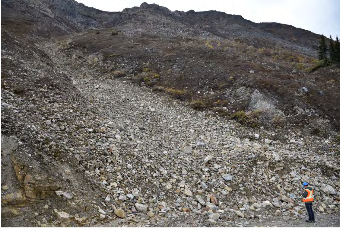
Photo 9: Drainage Channel 2, which is the most significant channel that crosses the Open Pit Access Road; the person in the photo is 1.8 m tall, for scale.
