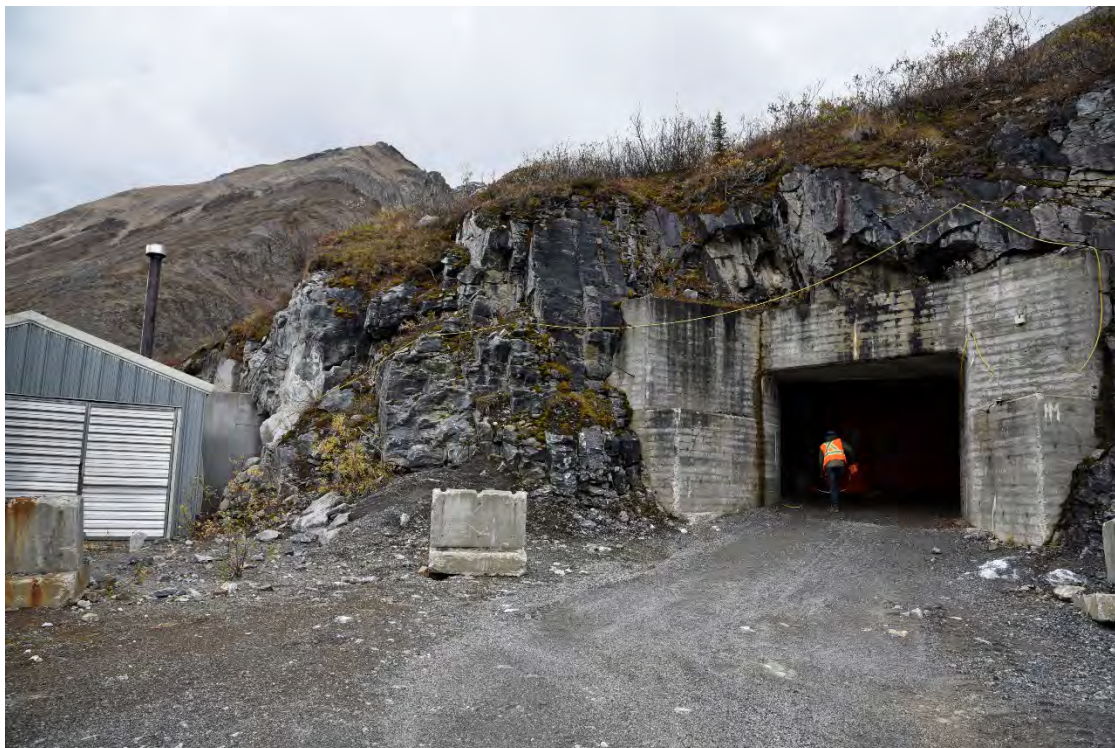
Photo 17: The Vent Adit, showing the vent portal (left) and manway (right, where the person is pictured). The vent buildings to the left should be removed.
