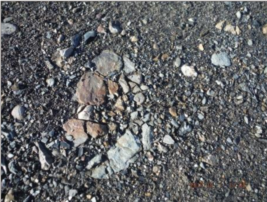
Photo 2: Typical mixed material in airstrip including crushed waste rock and fill. Minor oxidation alteration and weathering of select fragments is noted. (October 1, 2017)
