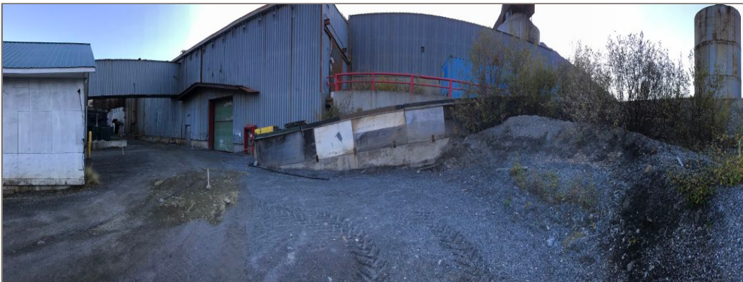
Photo 2: Panorama of Mill Building. Concentrate building (white) visible on left. (September 5, 2017)
