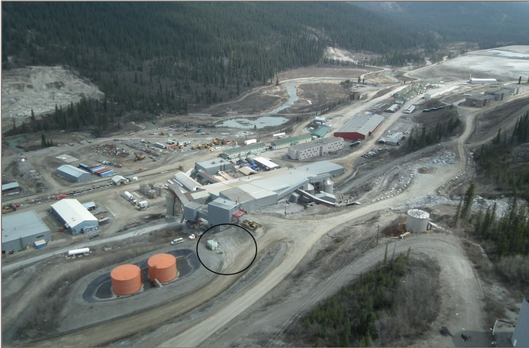
Photo 3: Facing east at current tank farm and fuel transfer area (circled). Photo provided by NATC. (May 29, 2014)
