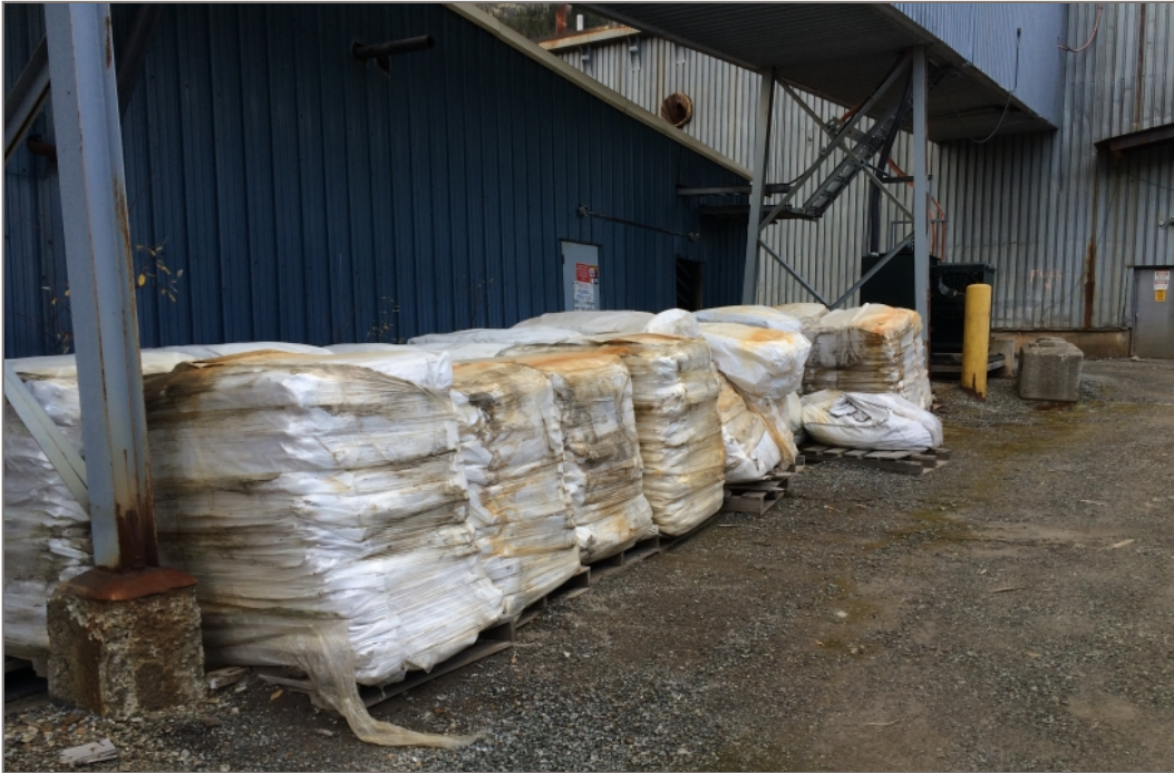
Photo 1: Facing south between Power House Building and Tungsten Concentrate Storage Building. Mill Building is visible on the right. (September 20, 2017)
