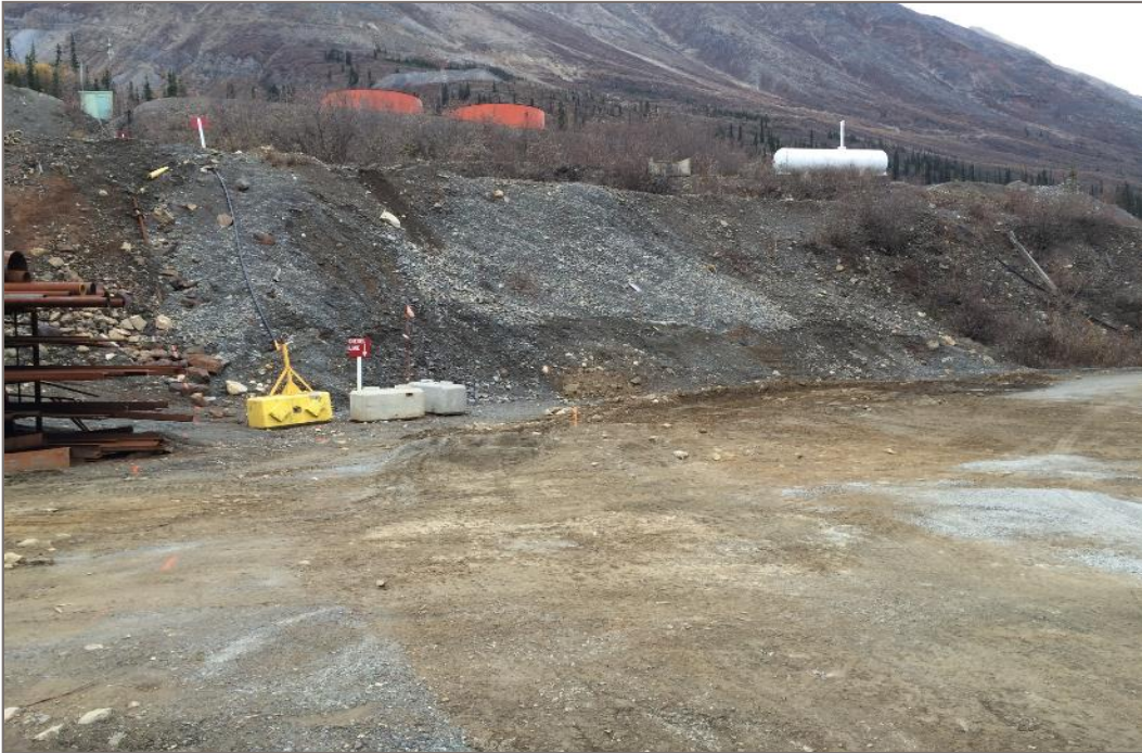
Photo 1: Facing west at diesel line from elevation of old tank farm and fueling area. Tank farm visible in background. (September 21, 2017)
