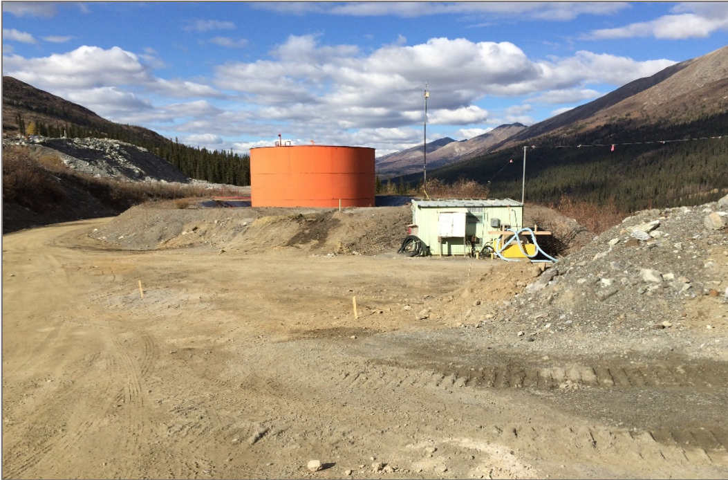
Photo 1: Facing northwest at fuel transfer area. Current tank farm visible in background. (September 17, 2017)
