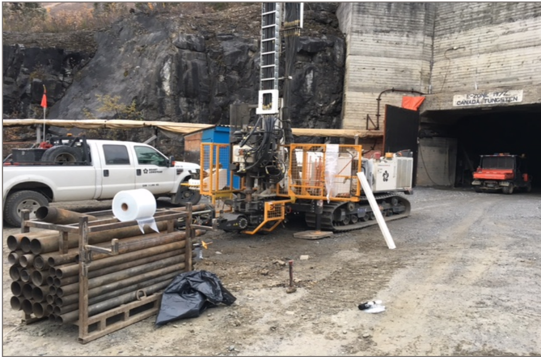
Photo 1: Drilling in front of main portal. (September 17, 2017)
