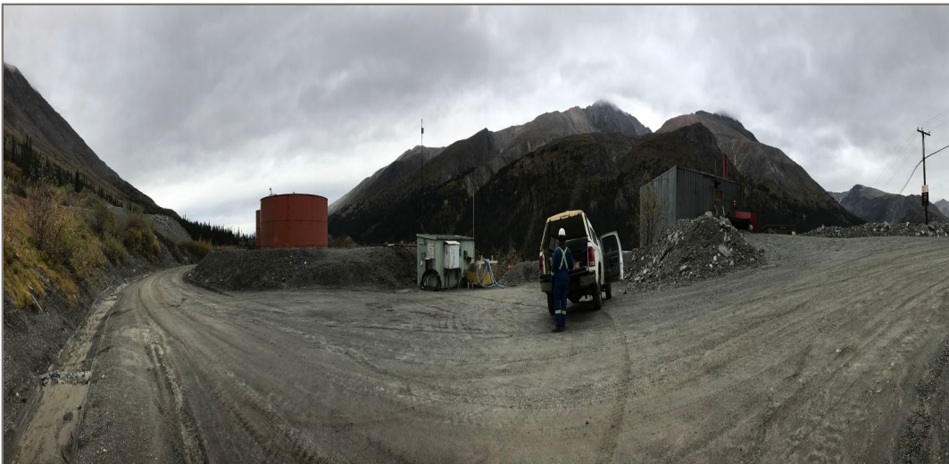
Photo 2: Panorama of fuel transfer area (on other side of truck, between truck and tank farm). Tank farm visible on the left. (September 4, 2017)
