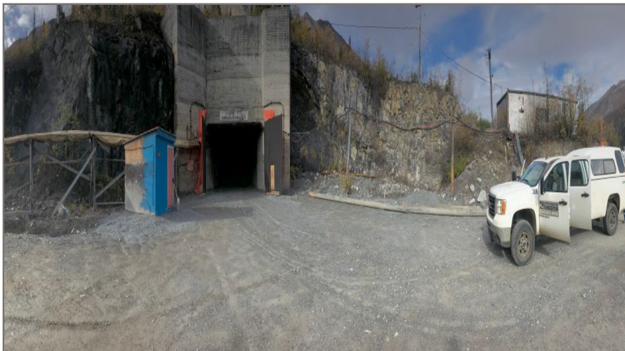
Photo 2: Panorama of main portal and former fuel area. (September 17, 2017)
