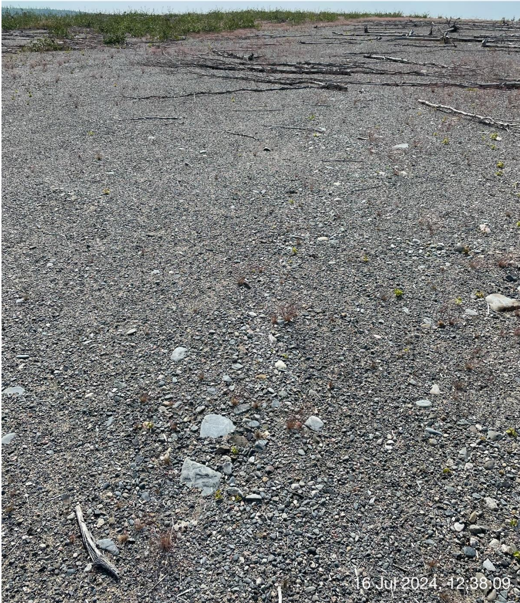
Photo 9: Willow branches cover the top of the TSCA to mitigate potential erosion – partially healed erosion channel visible.
