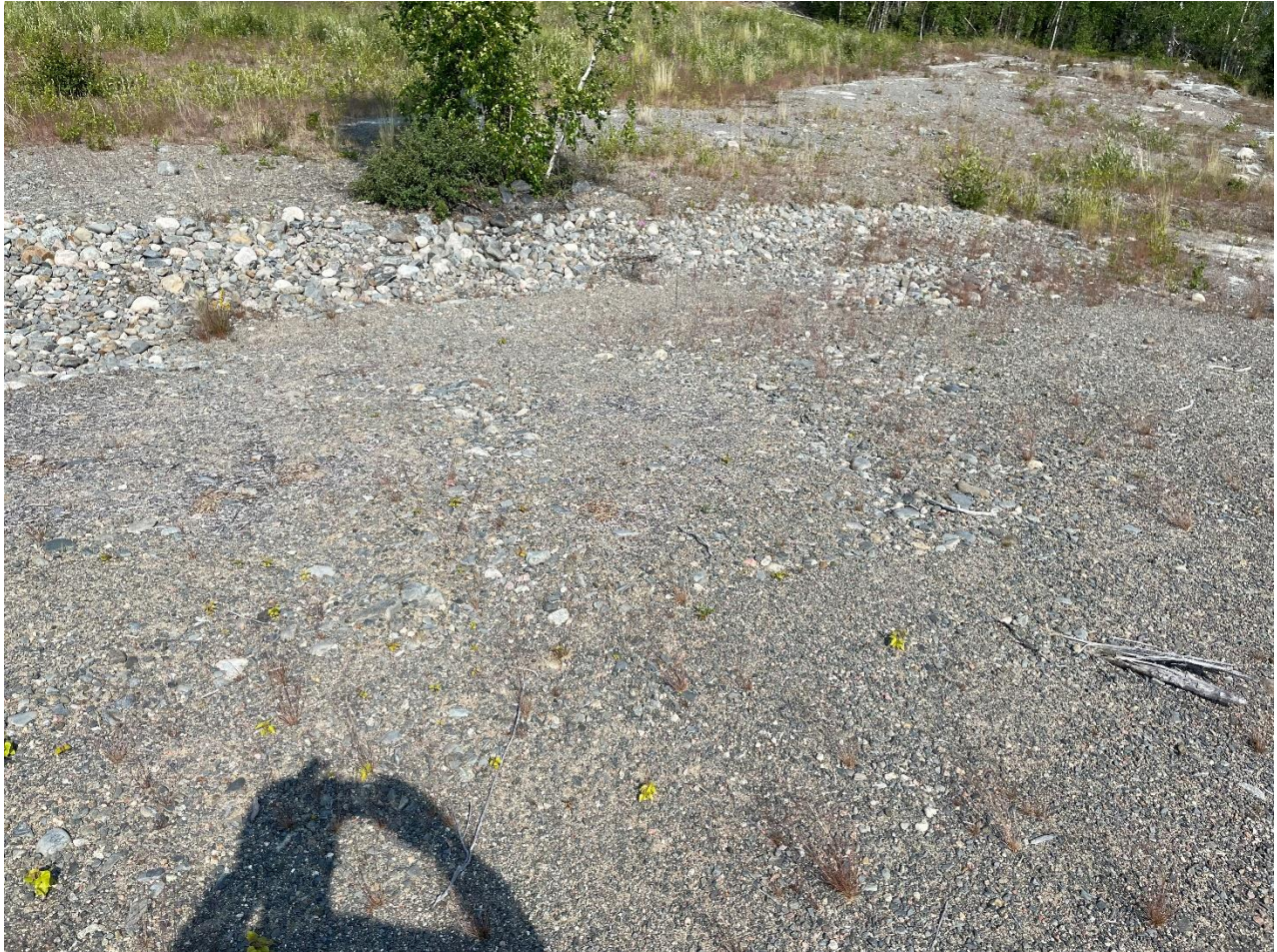
Photo 8: TSCA north slope with partially healed erosion channels – looking toward perimeter ditch.
