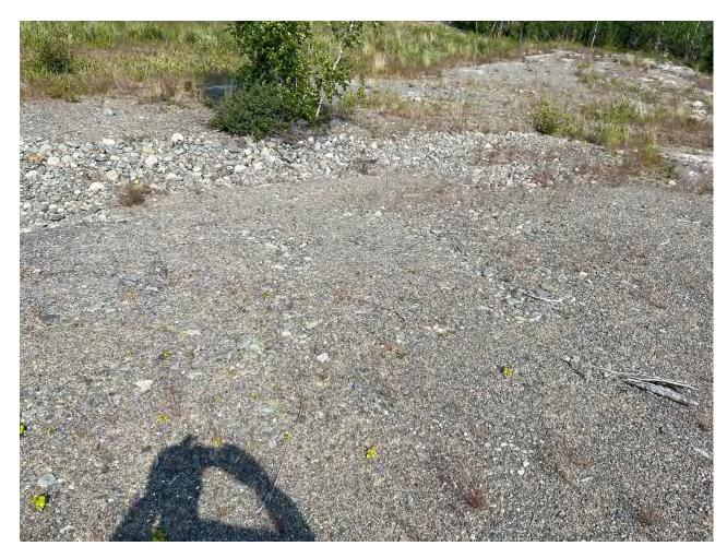
Photo 8: TSCA north slope with partially healed erosion channels – looking toward perimeter ditch.
