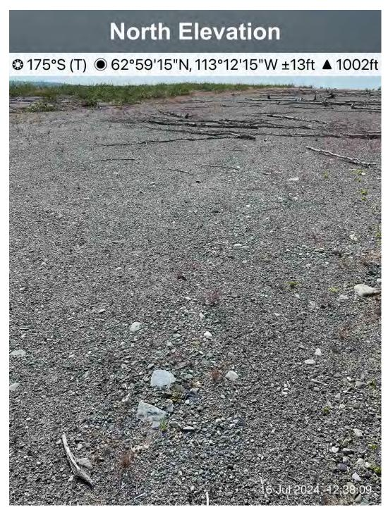
Photo 9: Willow branches cover the top of the TSCA to mitigate potential erosion – partially healed erosion channel visible.
