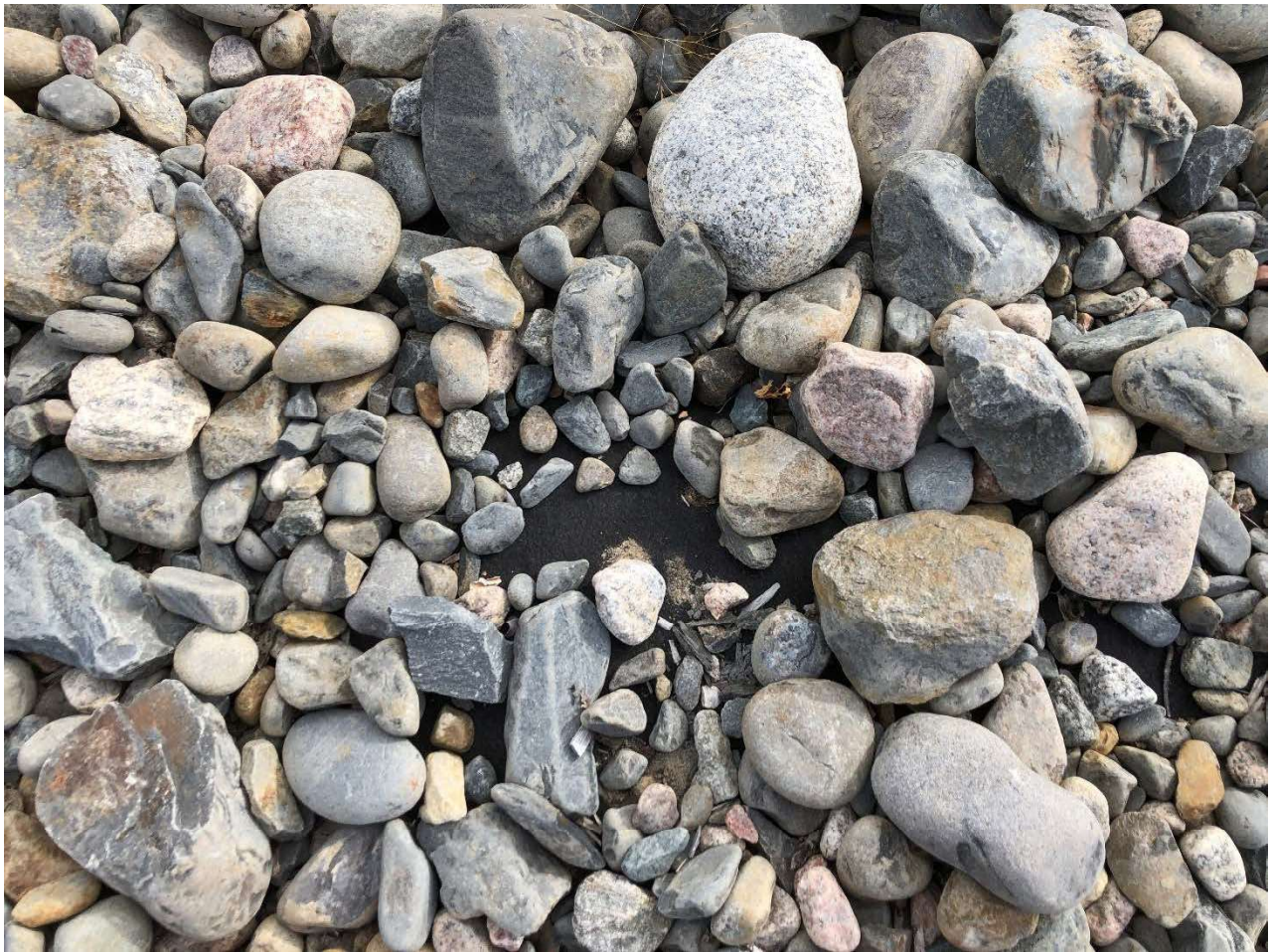
Photo 8: TSCA exposed liner at West Ditch.
