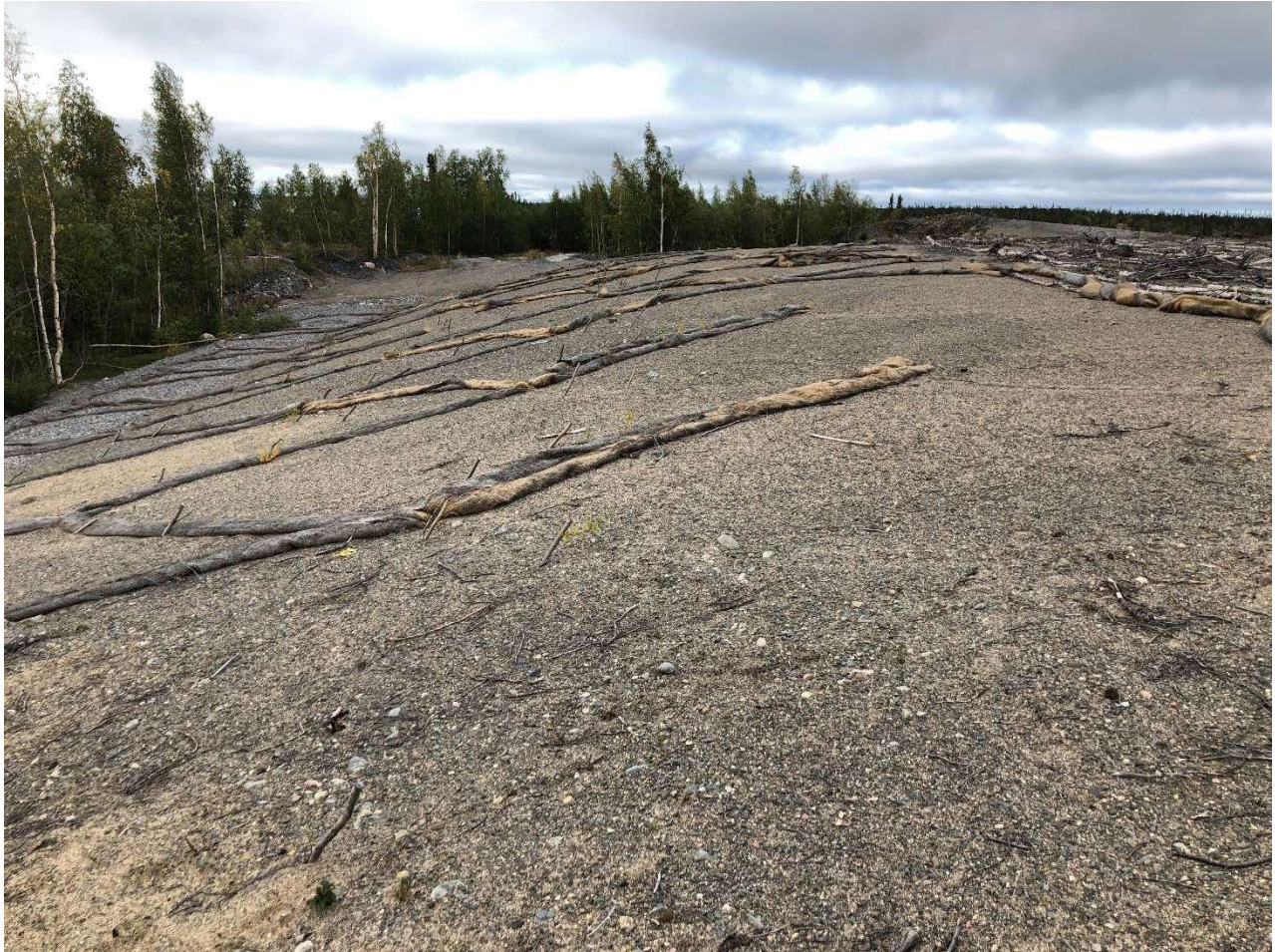
Photo 3: Eastern slope of the TSCA, looking south, protected with coco-mats and willow branches in segments to mitigate potential erosion.
