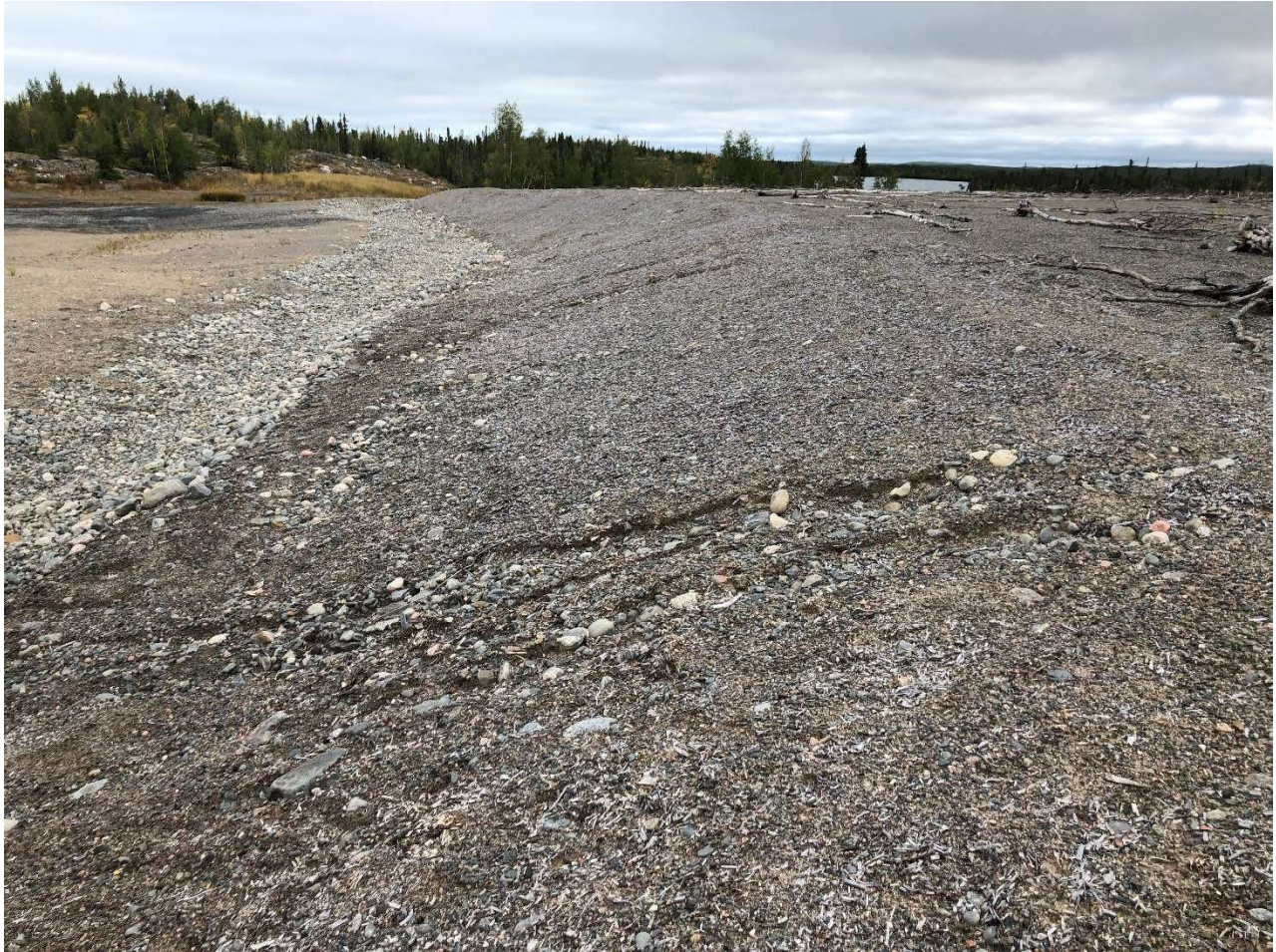
Photo 5: Ditch 1 – West Perimeter. Rip Rap stone lining ditch. Slope erosion.
