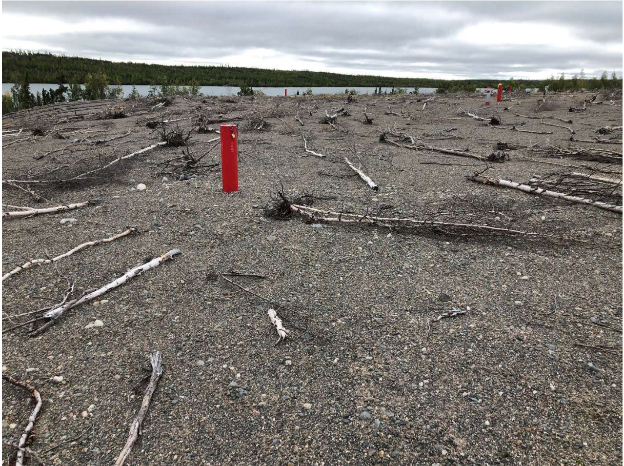
Photo 9: Willow branches cover the top of the TSCA to mitigate potential erosion.
