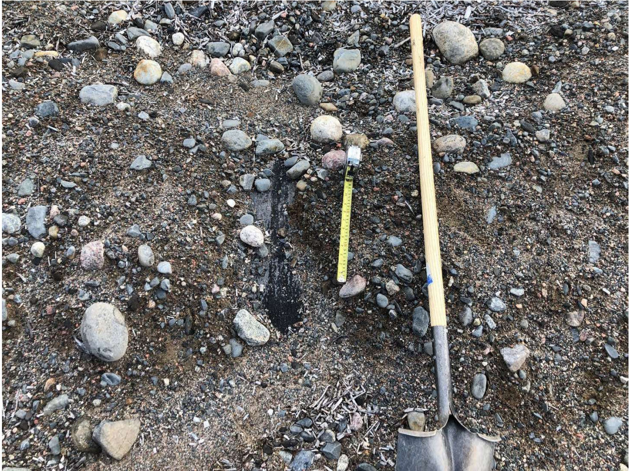
Photo 15: TSCA West Slope exposed liner.
