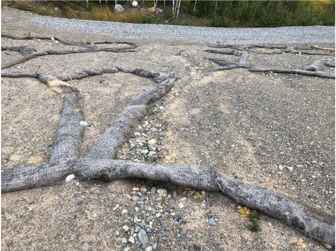
Photo 11: North TSCA Perimeter Slope. Surface Erosion.
