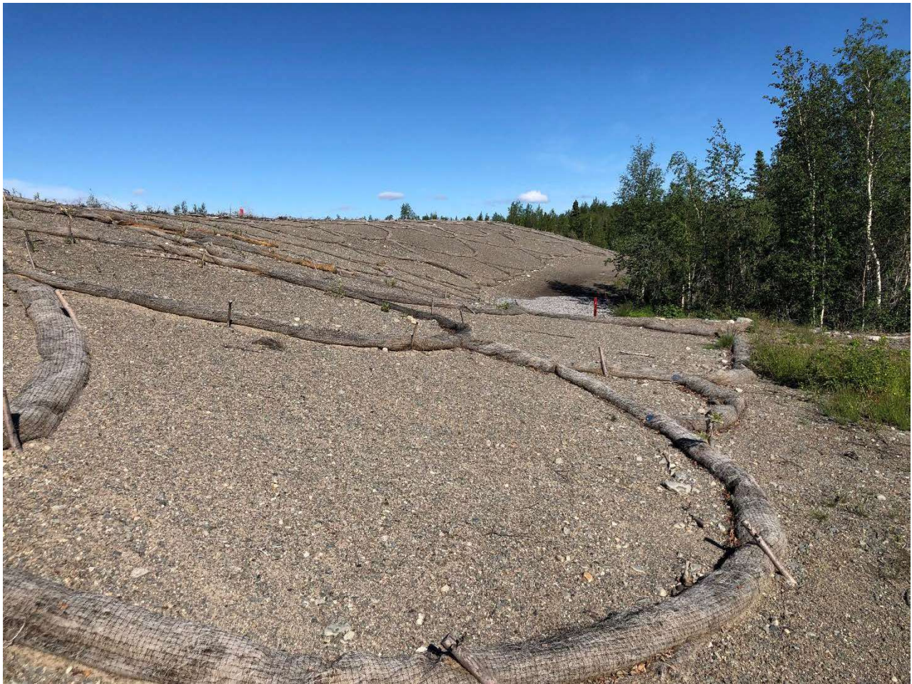
Photo 2: Northern slope of the TSCA, looking West, protected with coco-mats and willow branches in segments to mitigate potential erosion. MW3 in the far right. Photo taken in July 2020.
