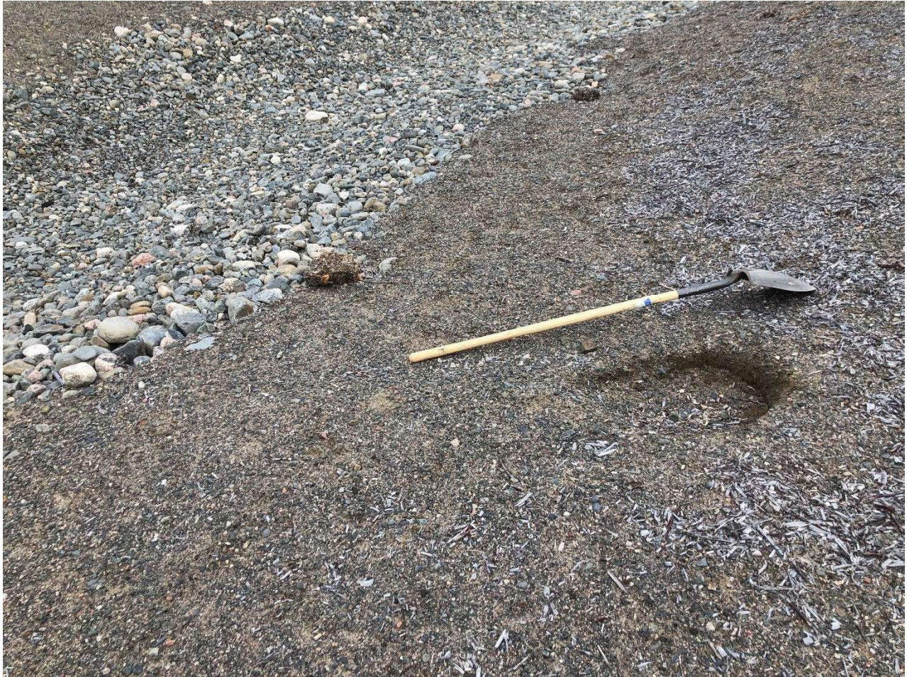
Photo 6: South Perimeter and south ditch. Animal burrow.
