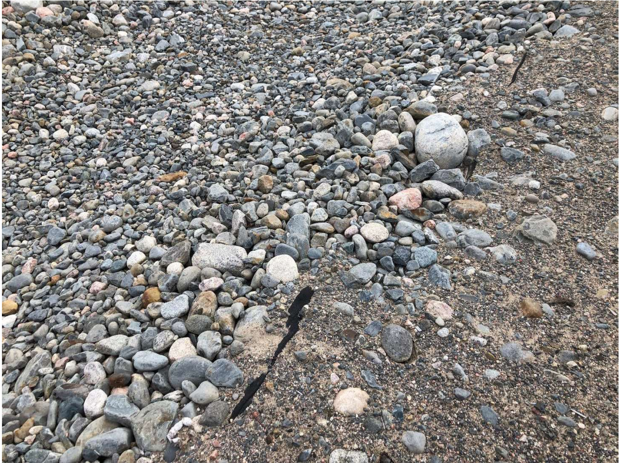
Photo 4: Exposed geofabric at TSCA toe.
