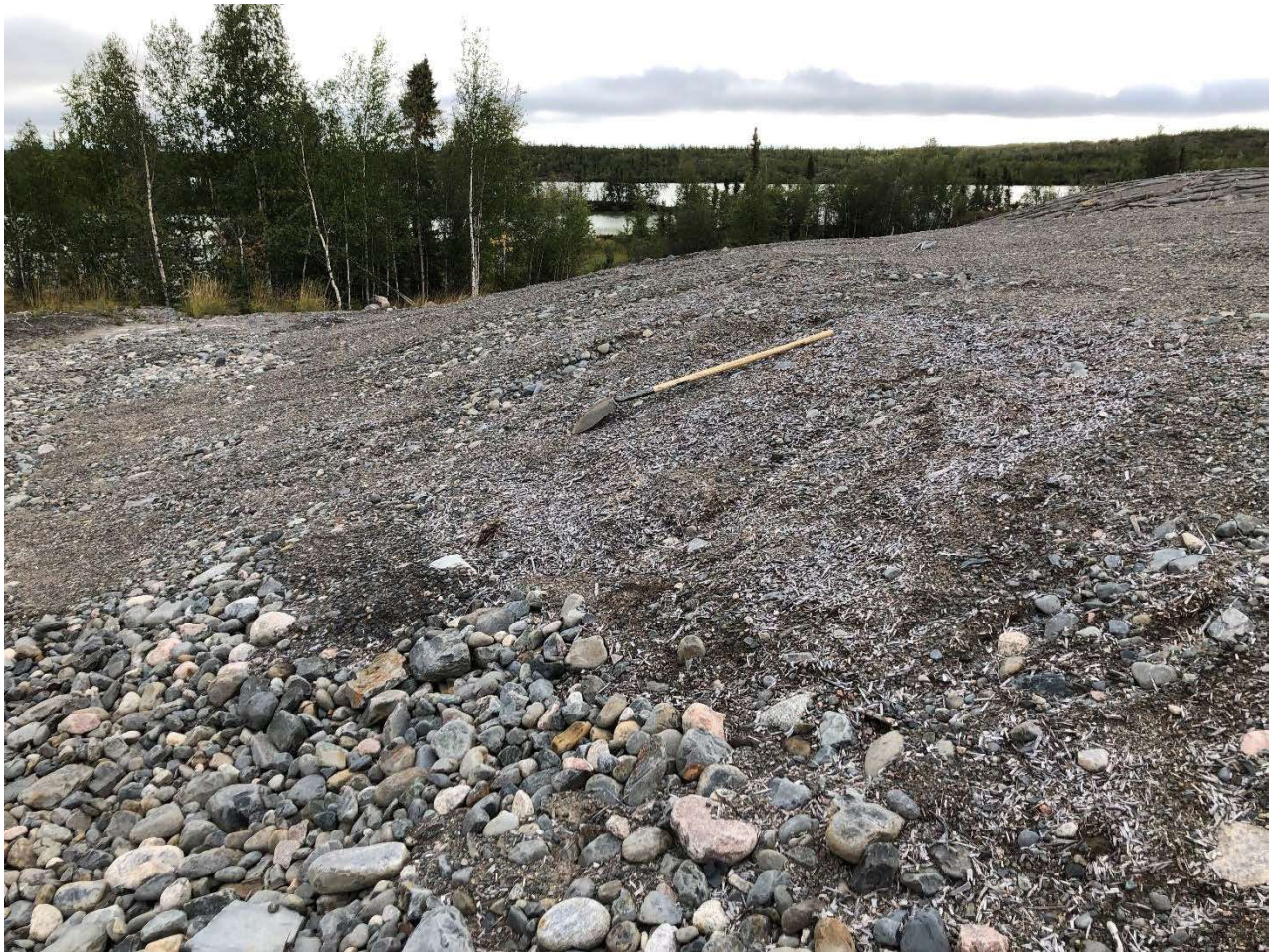
Photo 10: Northwest TSCA Perimeter Slope. Surface Erosion.
