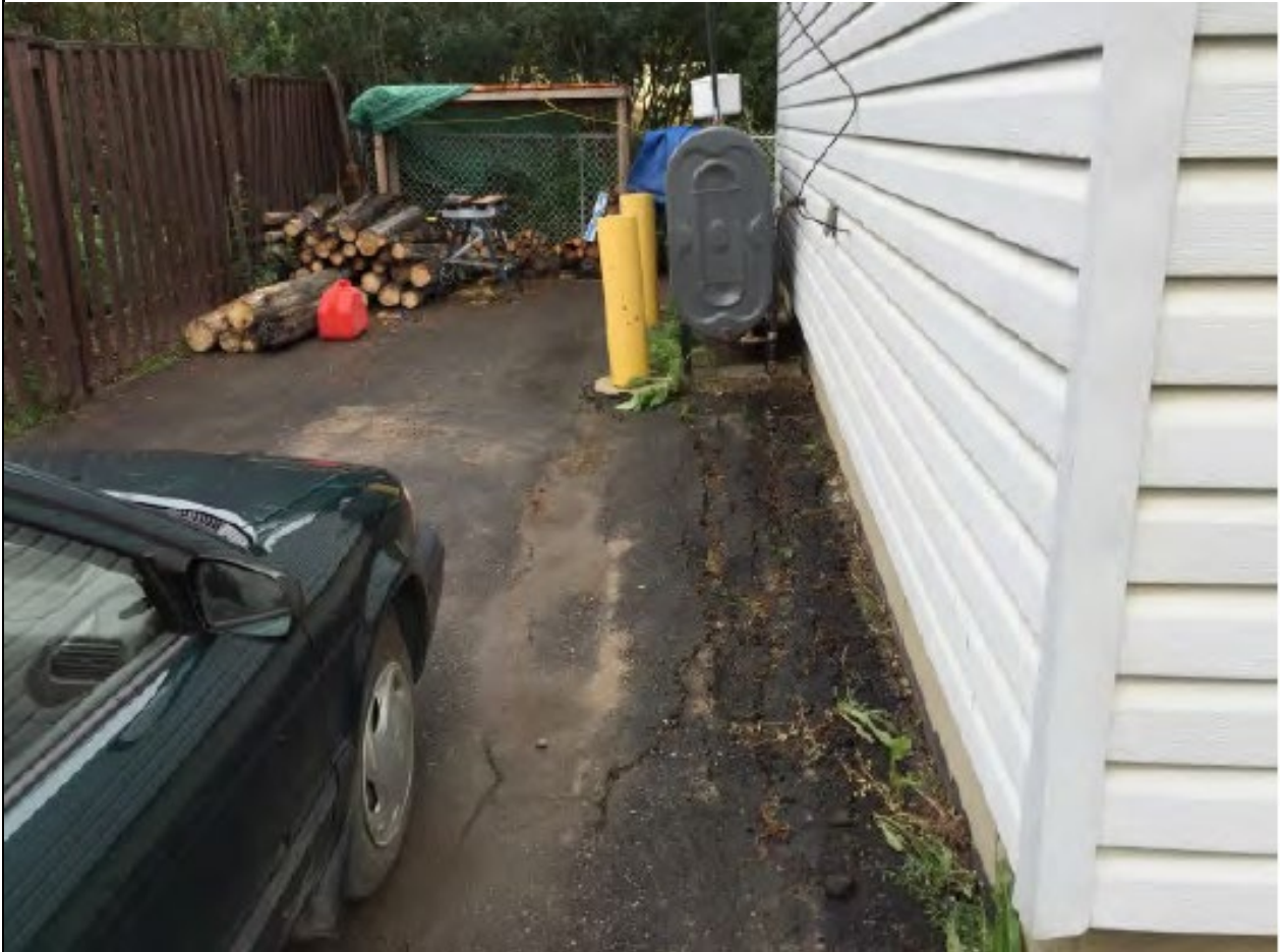
Photo 4: 9818 101st Residence – Historical Fuel Oil Tank Not In Service Minor Leak From Adapter
