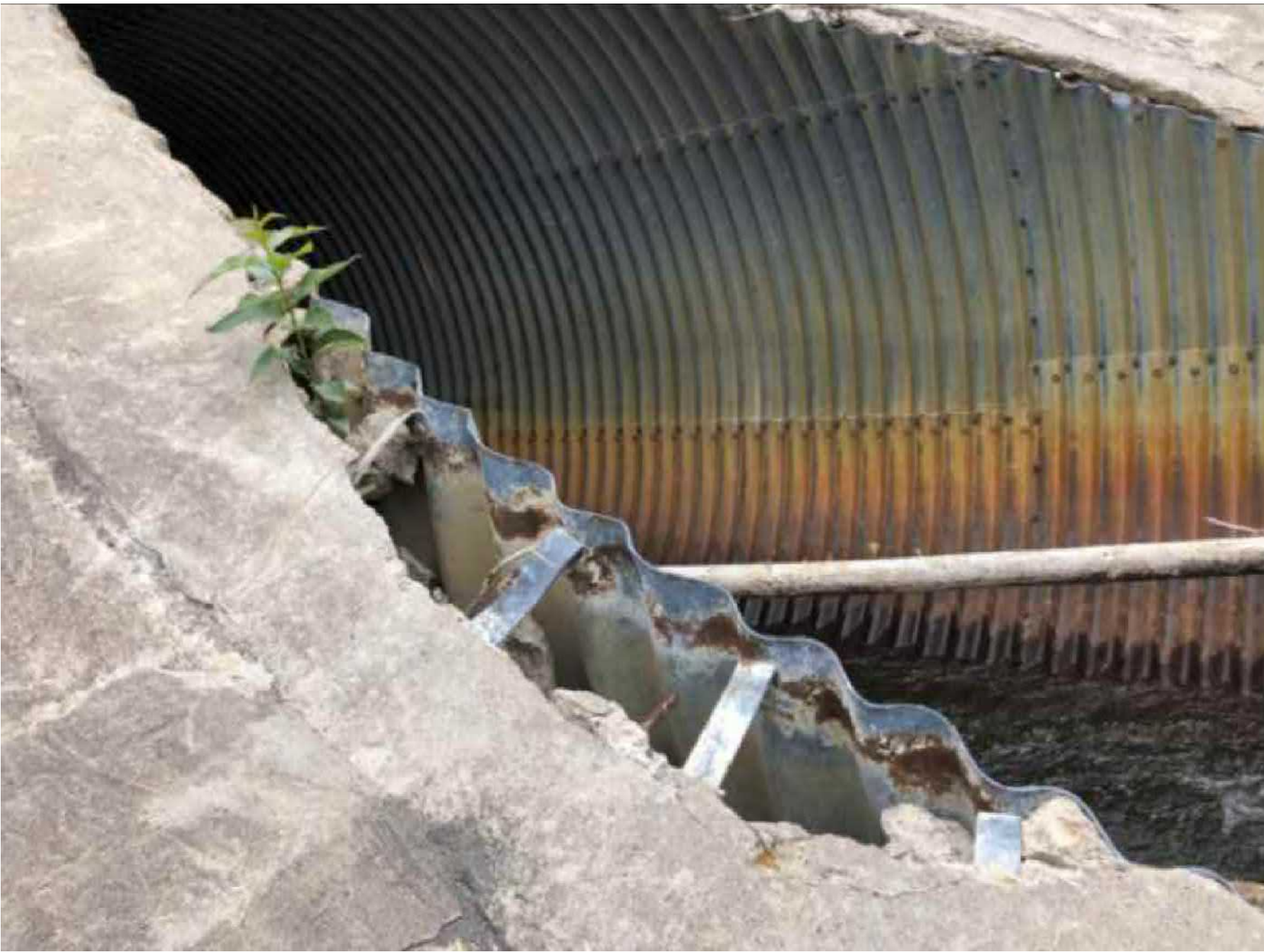
TYPICAL INLET PROTECTION CONCRETE SPALL N.T.S
