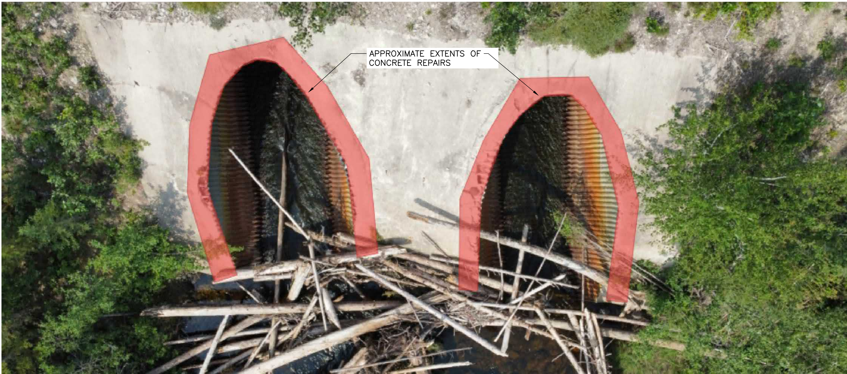
CULVERT INLET HEADWALL CURRENT CONDITION N.T.S
