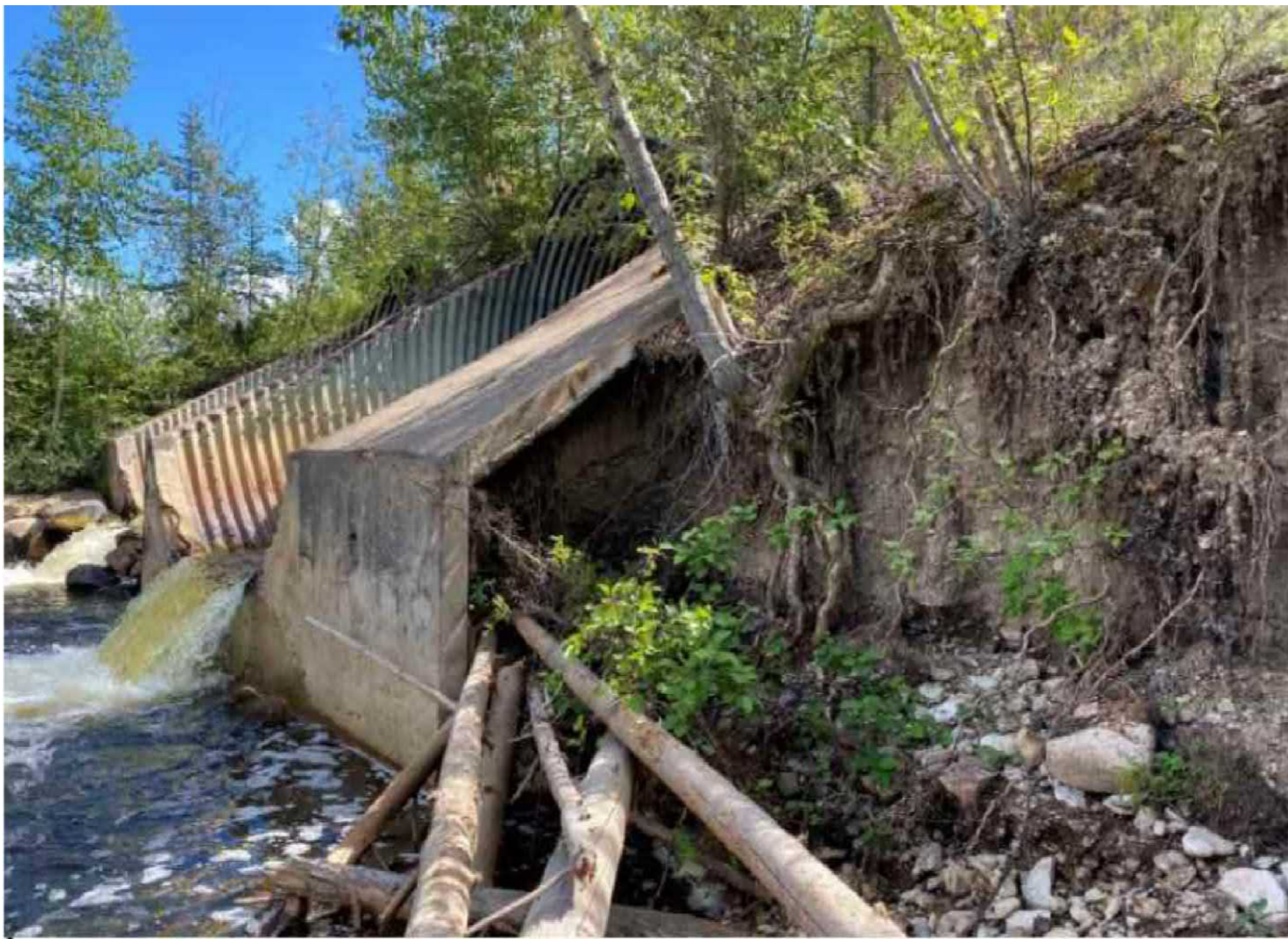
SCOUR BEHIND WEST BARREL OUTLET PROTECTION N.T.S
