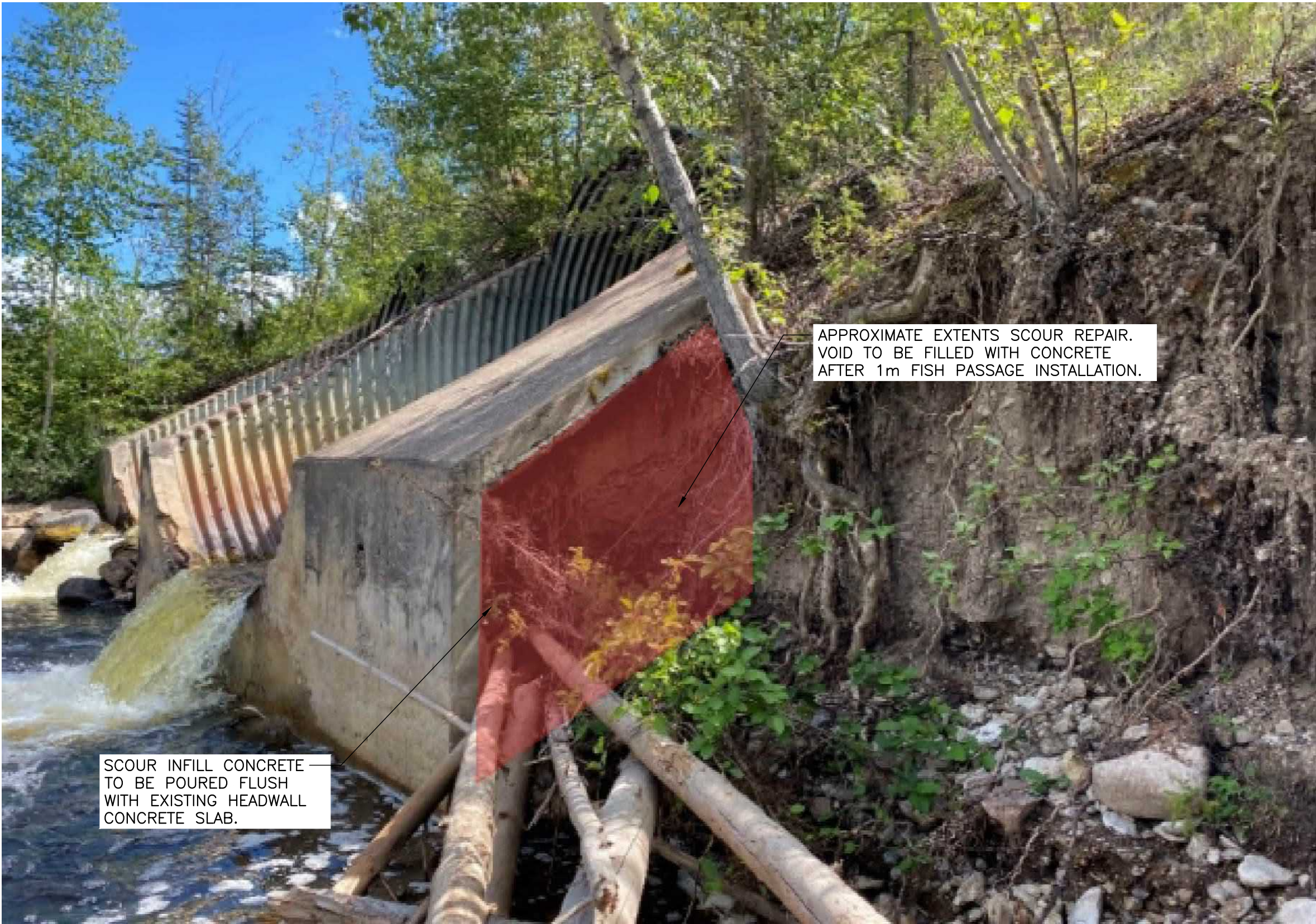
WEST CULVERT OUTLET SCOUR CURRENT CONDITION N.T.S
