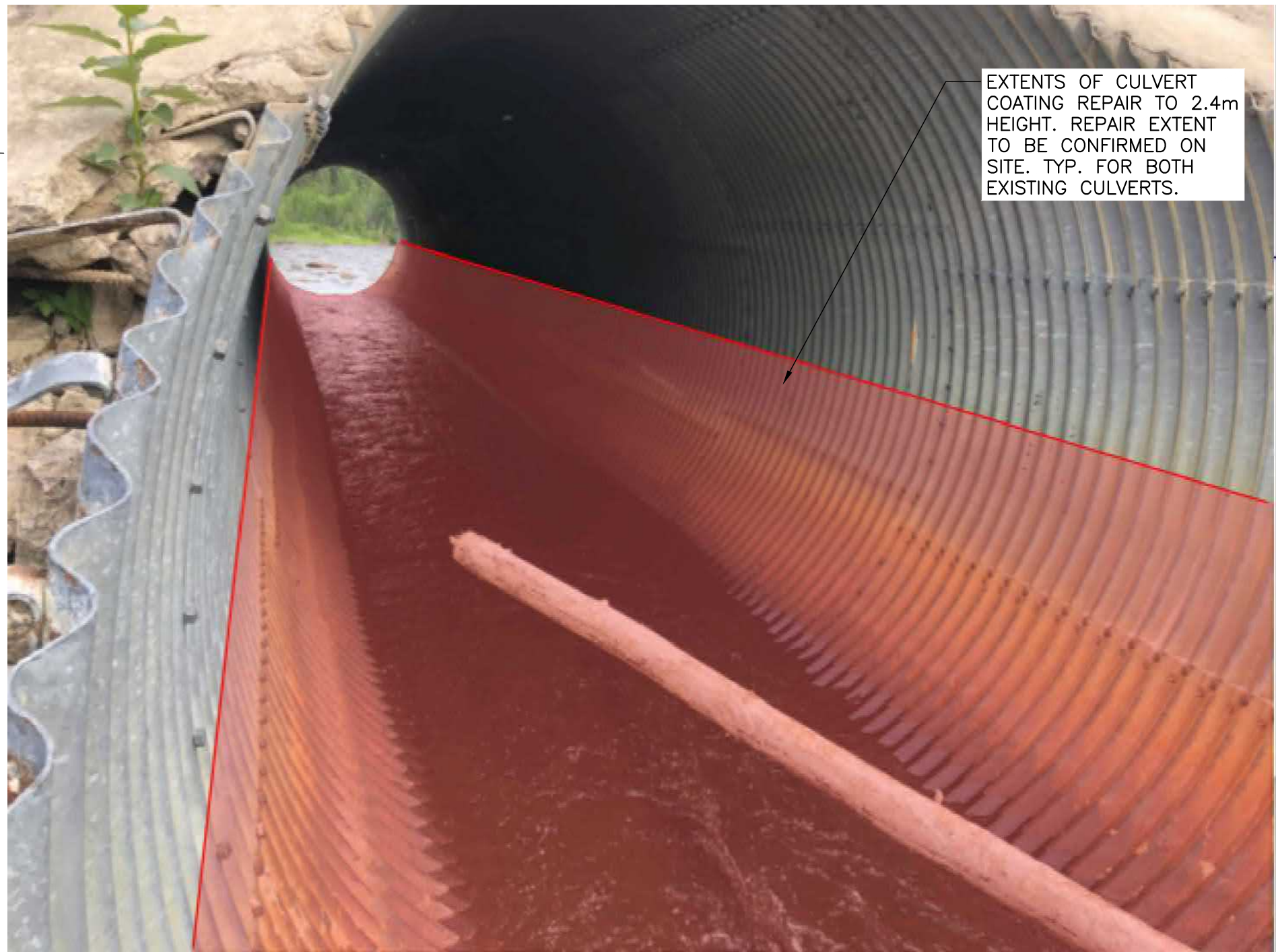
EXTENTS OF CULVERT COATING REPAIRS N.T.S
