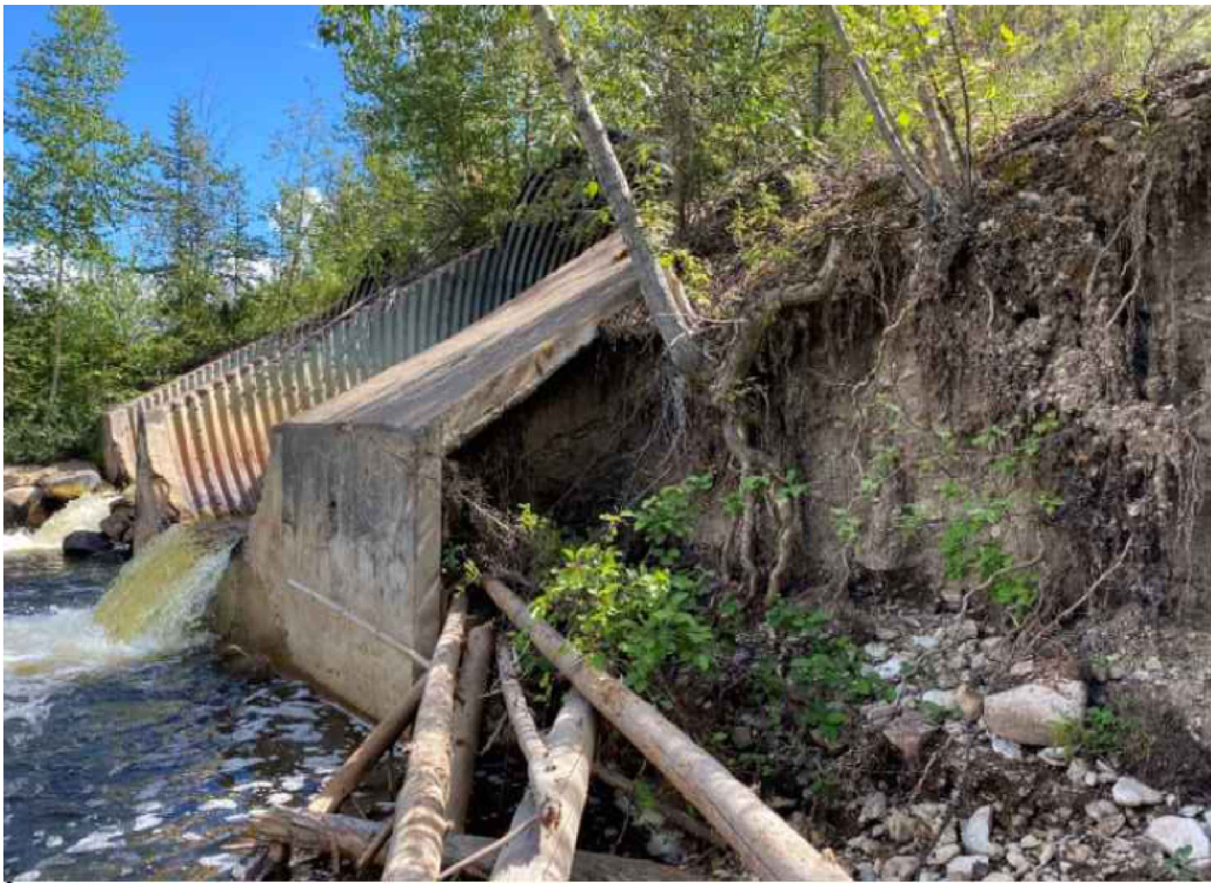
SCOUR BEHIND WEST BARREL OUTLET PROTECTION N.T.S
