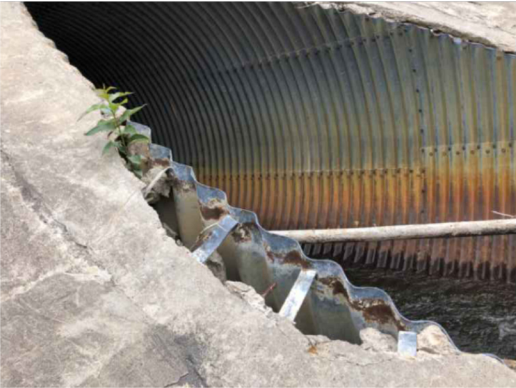
TYPICAL INLET PROTECTION CONCRETE SPALL N.T.S
