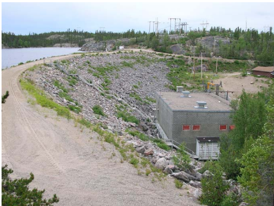
Photo 4 Snare Rapids Main Dam – downstream face in good condition, brushing recommended as part of regular maintenance.
