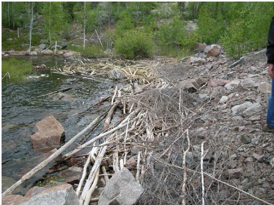
Photo 24 Side Dam 4 – accumulations of woody debris near left abutment.
