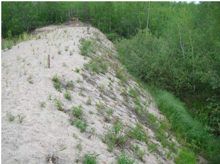
Photo 30 Side Dam 9B - downstream slope is in a satisfactory condition
