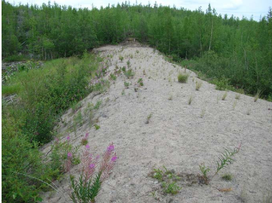
Photo 27 Side dam 9B – crest profile shows possible signs of minor settlement near centre – survey recommended to determine if topping-up is required to reinstate the crest design level.
