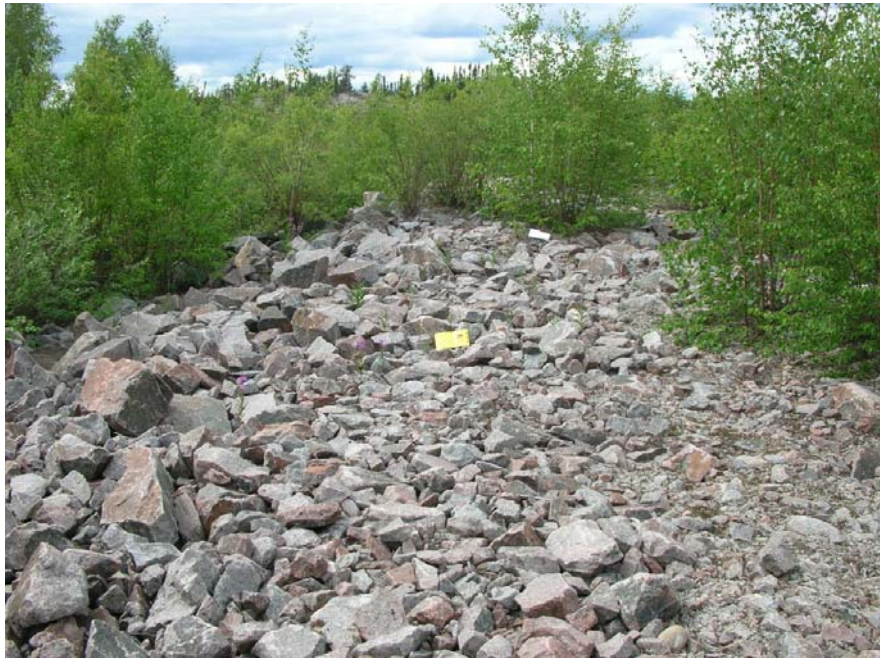
Photo 19 Side Dam 5B – apparent low point on crest near the right abutment.
