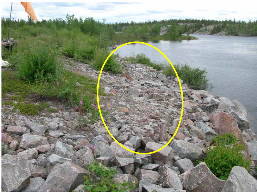
Photo 20 Side Dam 5B – finer riprap identified in some locations.
