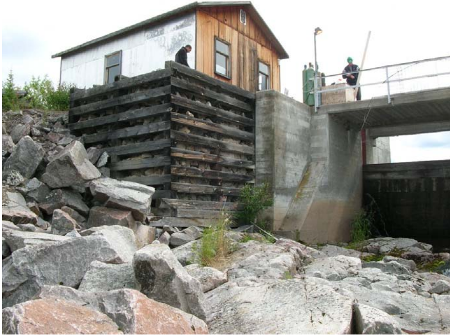
Photo 11 Spillway 5B - timber crib retaining wall at downstream right abutment retains Side Dam 5B fills.
