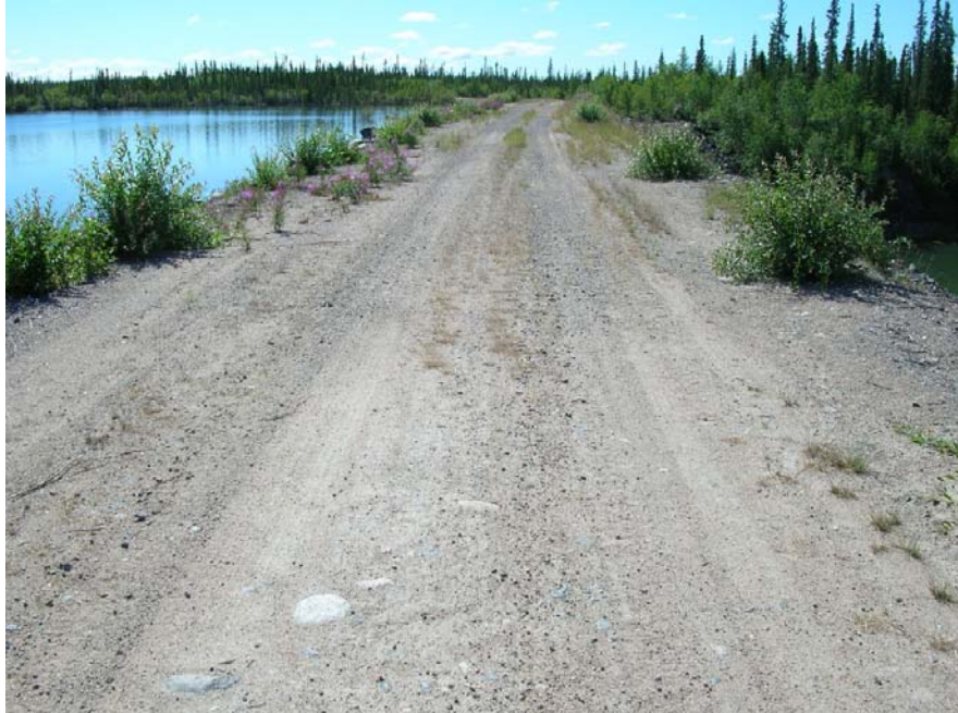
Photo 63 Snare Forks Dam – crest planar with no signs of settlement, cracks or erosion.
