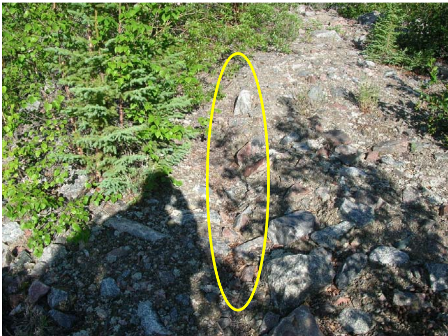
Photo 46 Saddle Dam No. 2 - discontinuous longitudinal depressions occurring near the upstream and downstream sides of the crest show no change from previous reports.
