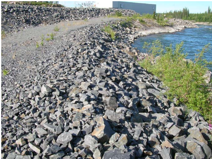
Photo 52 Snare Cascades Power Canal Dyke - crest of the lower bench is typically planar with no signs of instability or distress.
