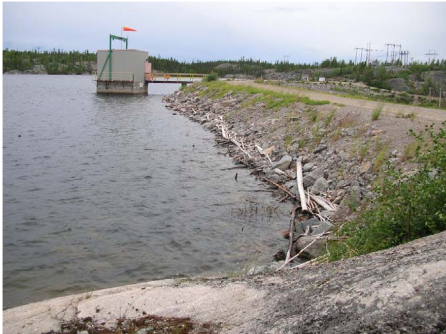
Photo 3 Snare Rapids Main Dam – woody debris accumulated along upstream face to be removed as part of regular maintenance.
