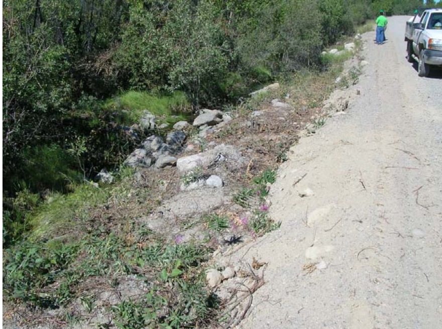
Photo 71 Freeboard Dyke 2 - ponded water along the downstream toe originates from foundation seepage at the left abutment.
