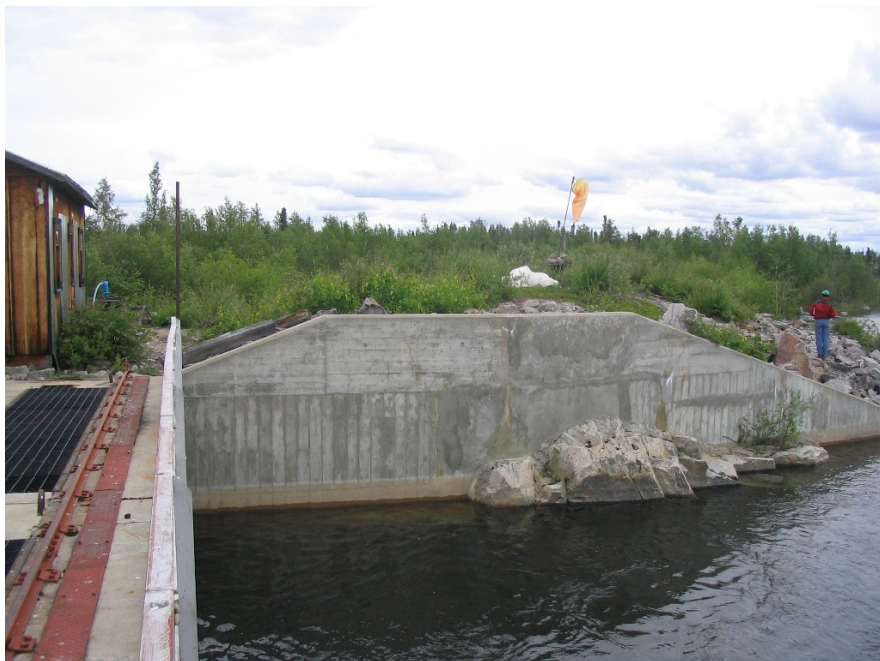
Photo 10 Spillway 5B – retaining wall along upstream right abutment retains fills from Side Dam 5B.
