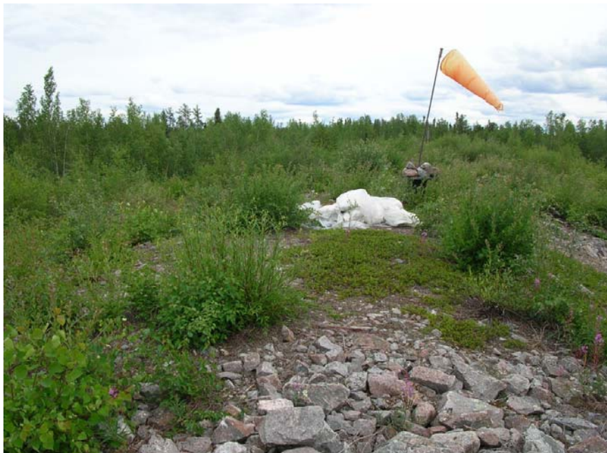
Photo 18 Side Dam 5B – typical crest condition. Brushing of crest and slopes required to permit proper inspection in the future.
