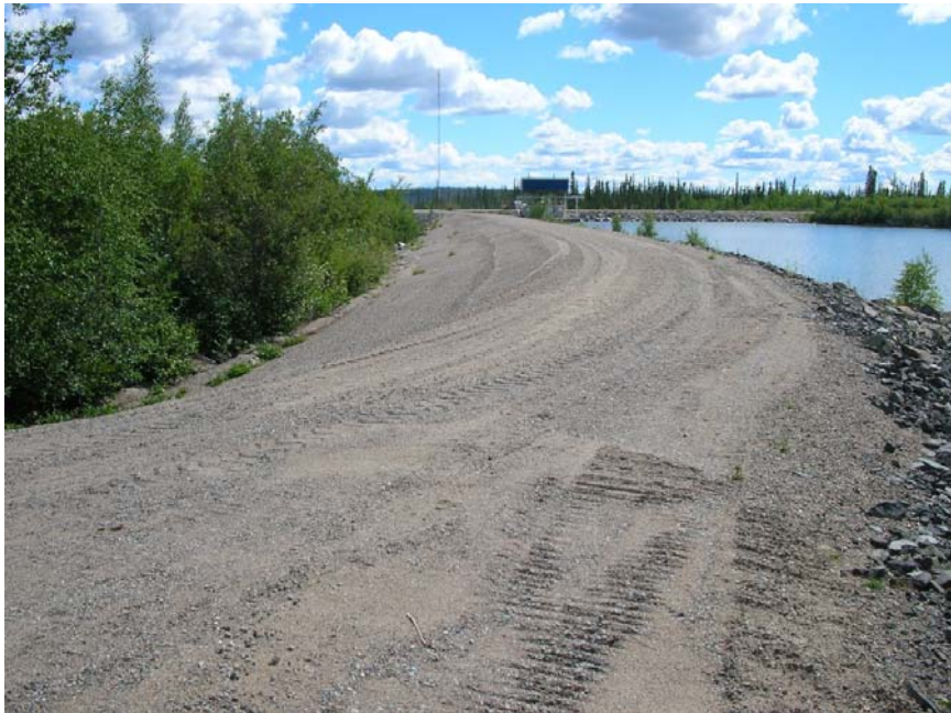
Photo 82 North Dyke – crest recently topped-up at the time of inspection and appeared to be in satisfactory condition. The crest is planar with no cracks, settled areas or erosion.
