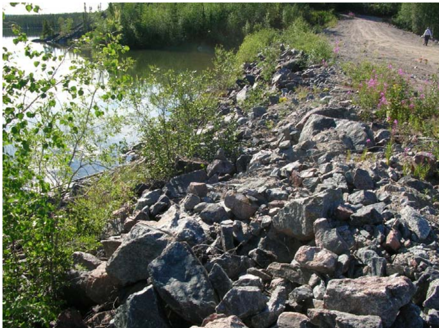
Photo 44 Saddle Dam No. 1 – upstream face satisfactory. Brushing required as part of on-going maintenance.
