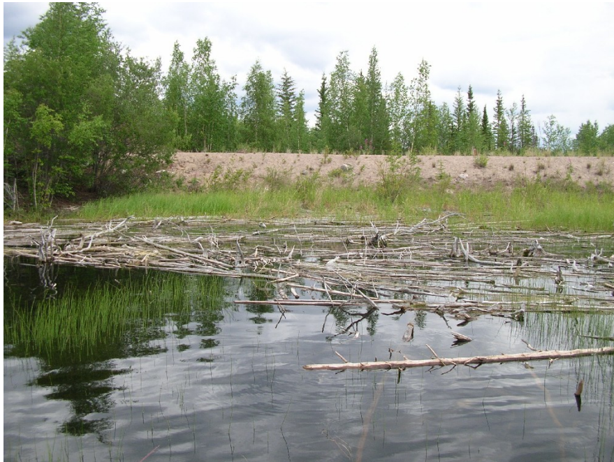
Photo 29 Side Dam 9B – woody debris mat accumulating near upstream face.
