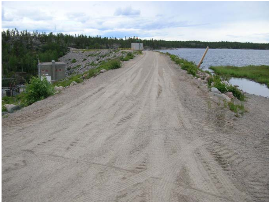
Photo 1 Snare Rapids Main Dam – typical crest condition.
