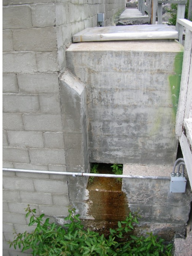
Photo 7 Snare Rapids Main Dam – seepage collection and measurement sump for seepage from the central portion of the dam.
