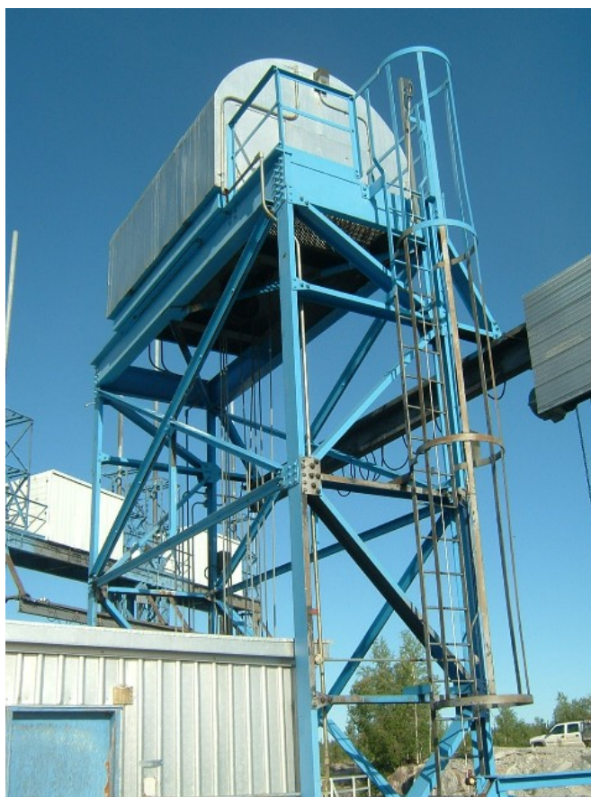
Photo 41 Snare Falls Intake – elevated hoist house and support structure general arrangement.
