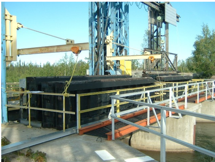
Photo 38 Snare Falls Spillway – stoplogs in satisfactory condition and in close proximity for quick installation.
