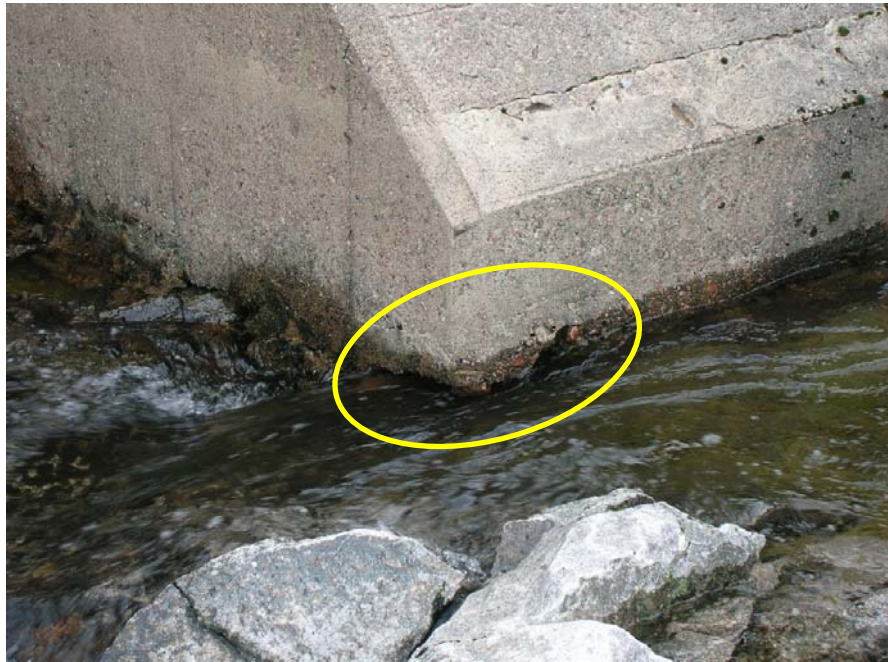
Photo 13 Spillway 5B – pier undercutting observed at other pier locations.
