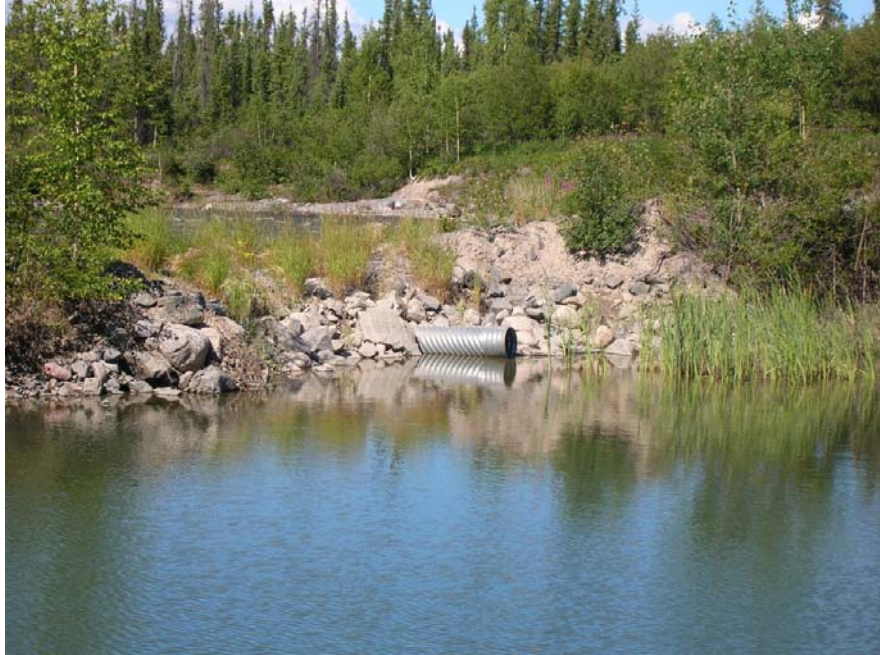
Photo 61 Snare Forks Dam - culvert installed through the cofferdam. Invert slightly below pond level.
