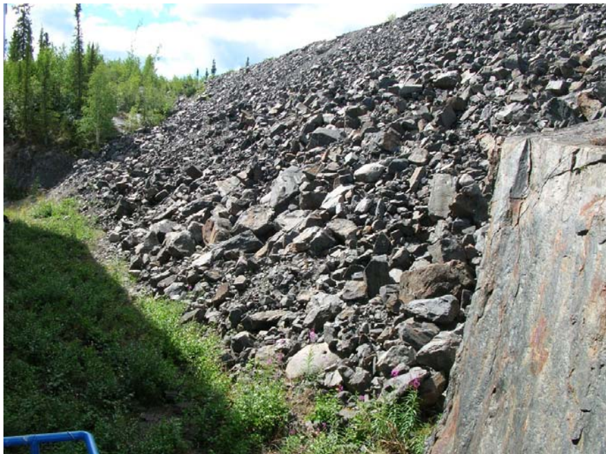
Photo 78 Strutt Lake Dam - downstream shell of the dam is planar with no settled areas, erosion gulleys or evidence of abutment seepage.
