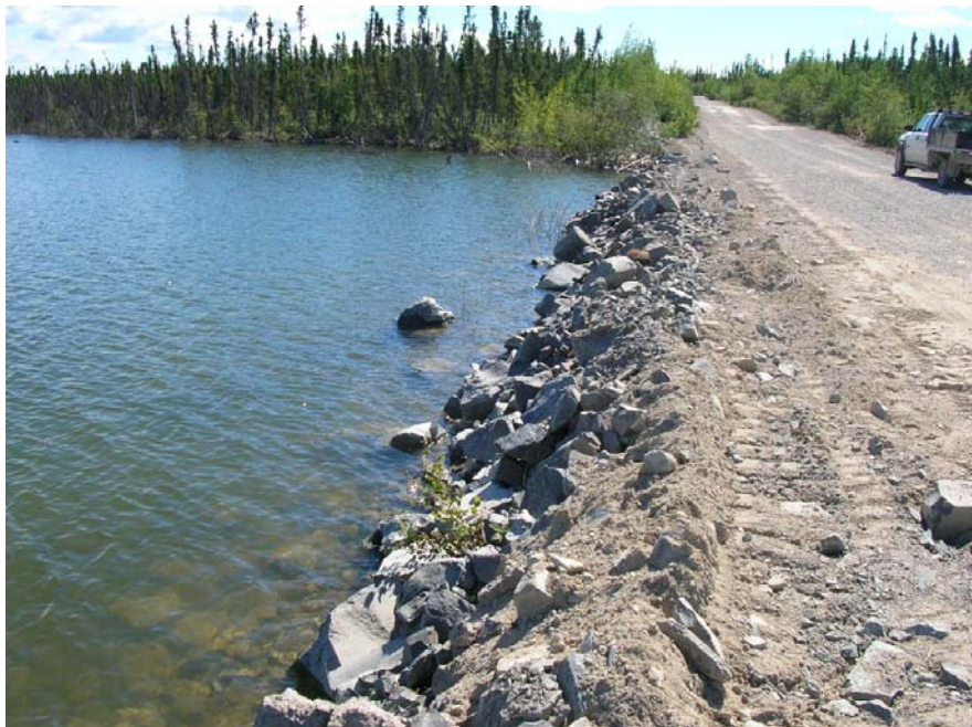
Photo 70 Freeboard Dyke 2 – riprap on upstream face is in acceptable condition.
