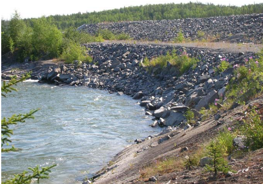
Photo 54 Snare Cascades Power Canal Dyke - downstream slope of the lower bench is planar, with no signs of instability or other distress. The rockfill protection appears sound and in good condition.
