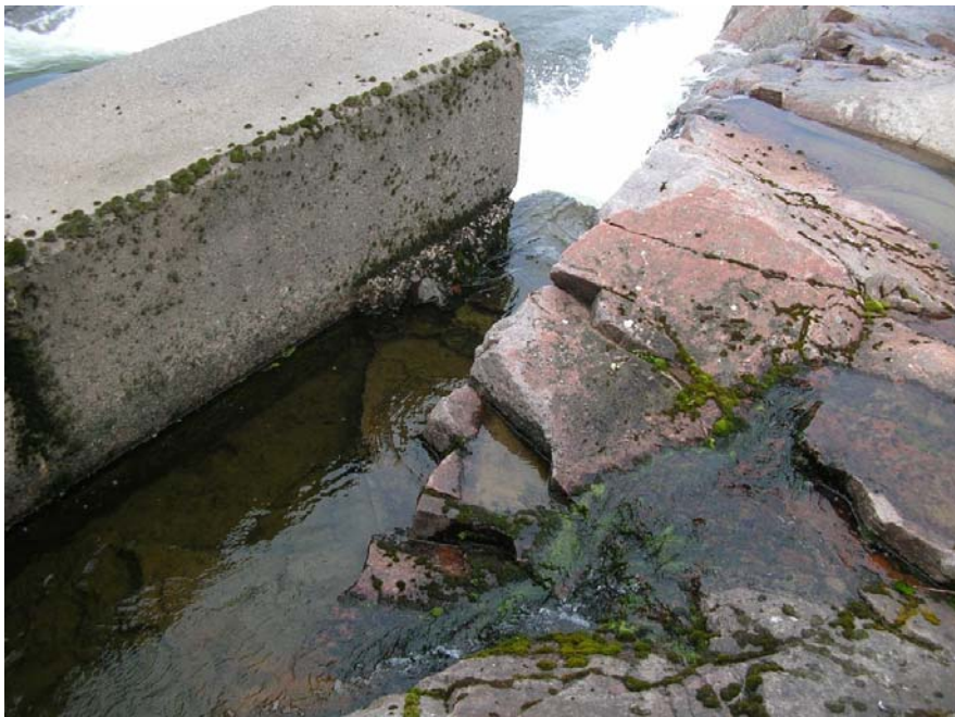
Photo 12 Side Dam 5B – undercutting of pier between spillway Bay 2 and 3
