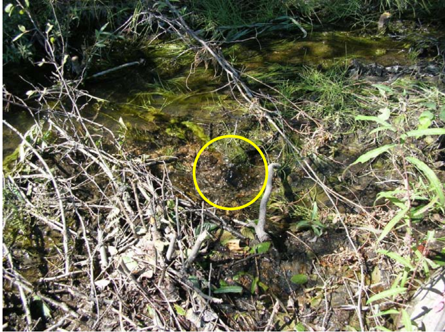
Photo 73 Freeboard Dyke 2 – small boil (5 cm max) discharging clear water beneath the ponded water within approximately 2 m of the toe of the dyke. .
