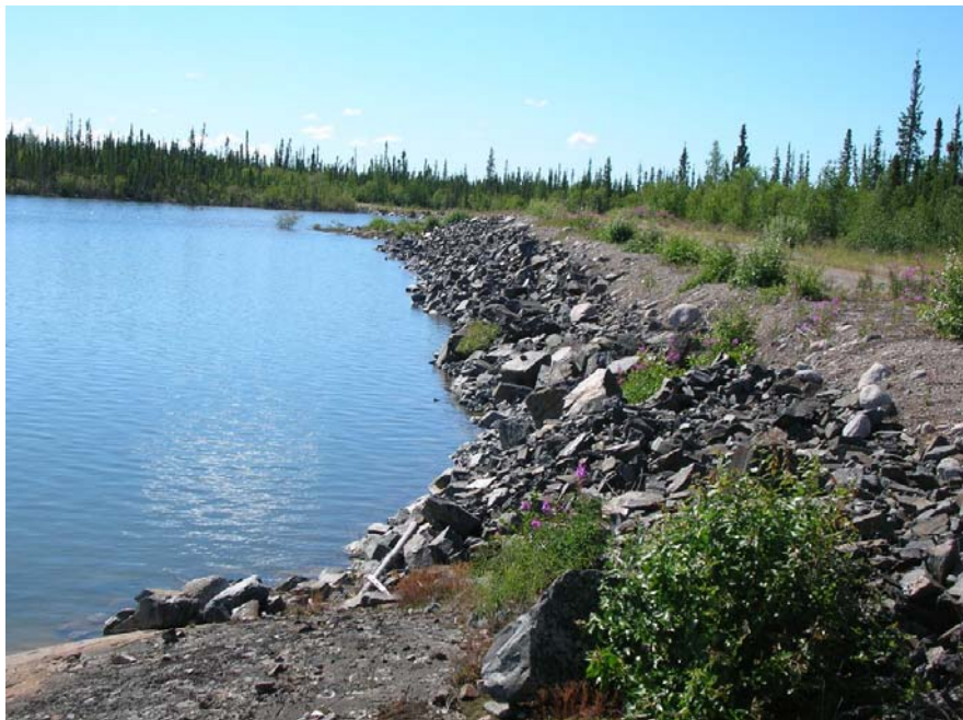
Photo 64 Snare Forks Dam - upstream slope typically shows no signs of settled areas or instability with no erosion or beaching of the riprap evident.
