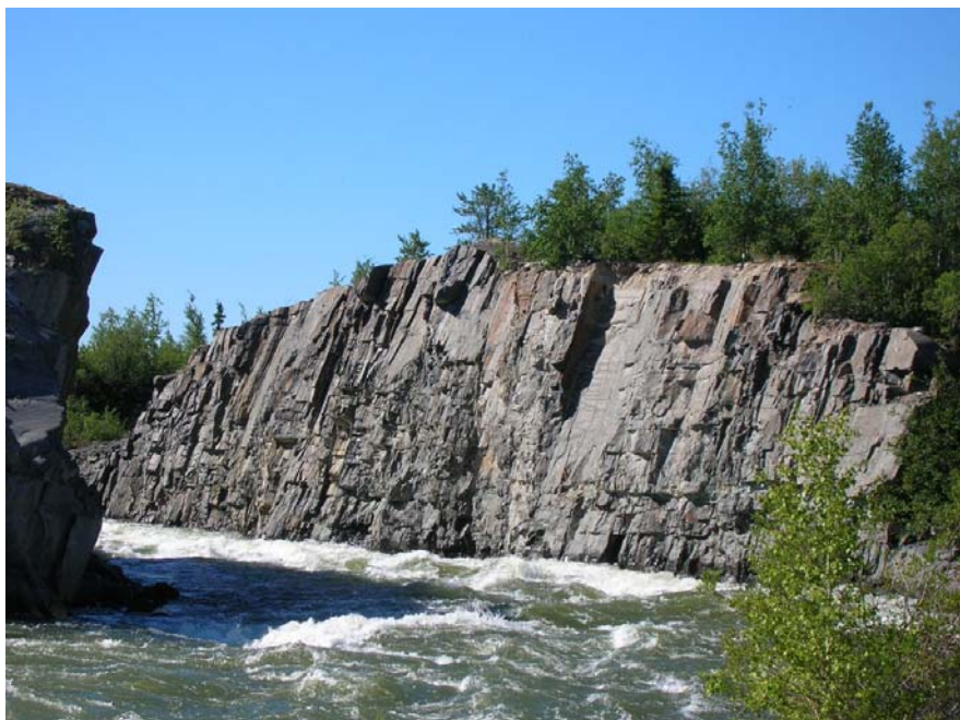
Photo 60 Snare Forks Spillway - excavated channel downstream of the spillway control structure is in good condition.
