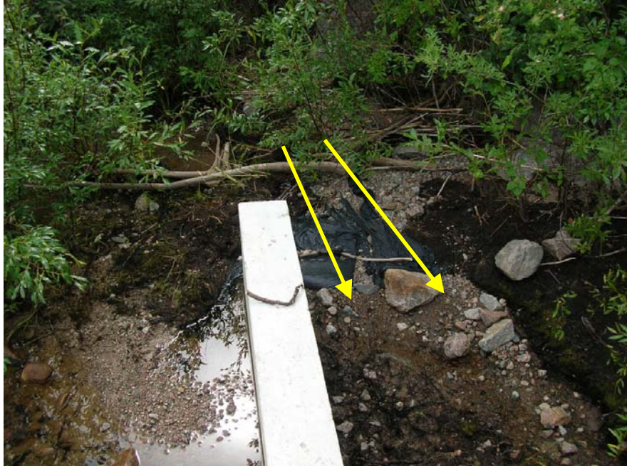
Photo 17 Side Dam 5B – area along left side of measuring weir structure where flow by-pass is observed to occur. Lateral extension of the wall is recommended to contain all future seepage flows.
