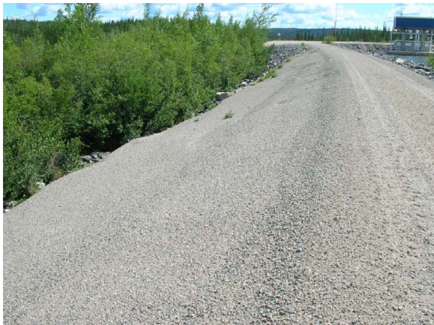
Photo 84 North Dyke - downstream shell is planar, with no erosion gulleys or evidence of seepage.
