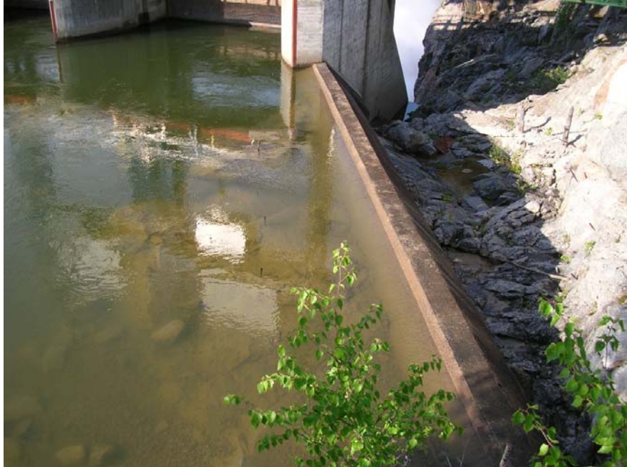
Photo 35 Snare Falls Spillway – side channel auxiliary spillway concrete control structure.
