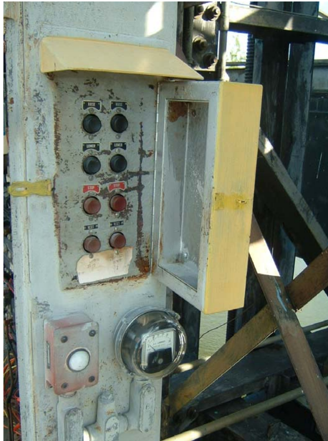
Photo 39 Snare Falls Spillway - gate operation is by manual pushbutton from the control panel at road level.
