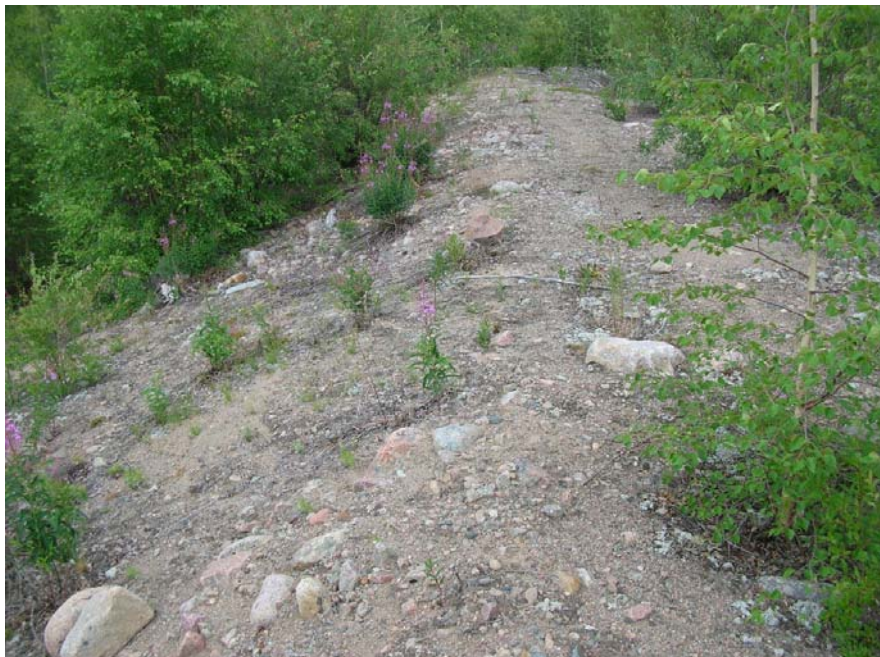
Photo 22 Side Dam 4 – some gullying on downstream face evident due to surface runoff.
