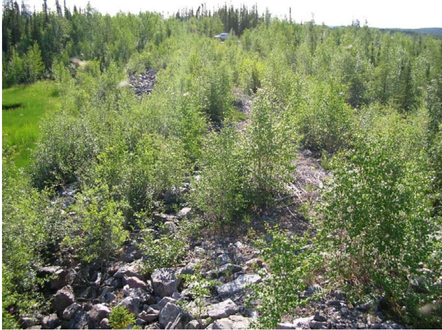
Photo 45 Saddle Dam No. 2 – Crest and slopes overgrown with saplings and dense brush. Brushing required to permit proper inspection.
