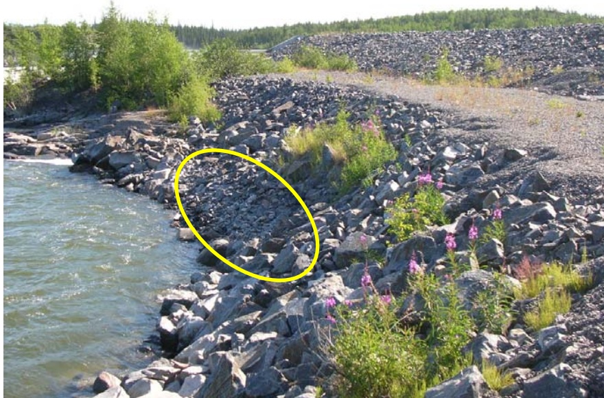
Photo 55 Snare Cascades Power Canal Dyke - localized area on the lower slope where the rockfill appears finer than the surrounding material, but there is currently no associated beaching or erosion. Brushing recommended..
