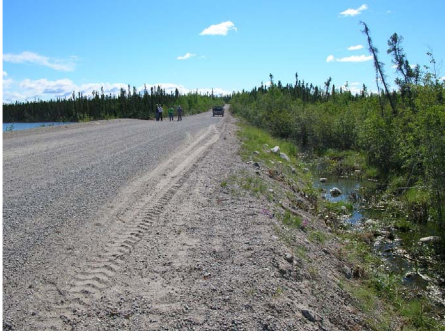
Photo 69 Freeboard Dyke 2 - downstream shoulder of the dyke cross section appears lower than at the centerline.
