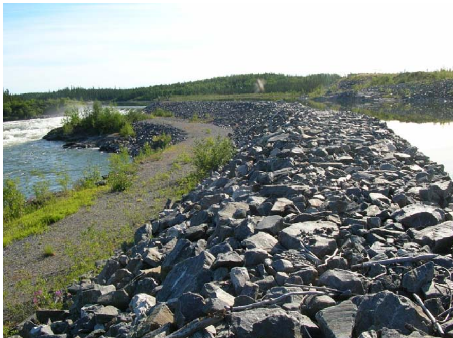
Photo 48 Snare Cascades Power Canal Dyke – crest typically planar with no obvious settled areas, erosion or abnormalities.
