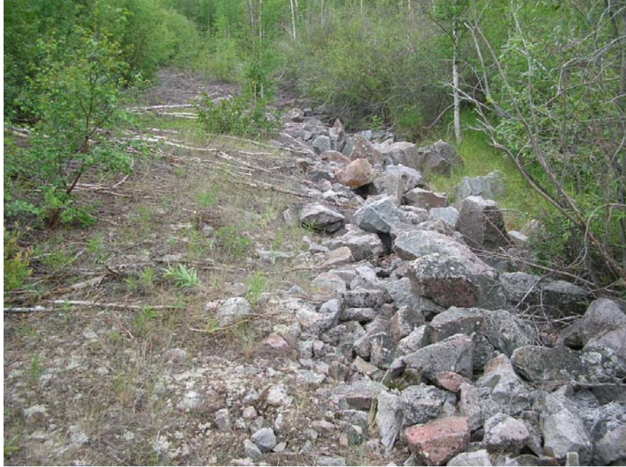
Photo 25 Side Dam 4 – rockfill toe berm shows no signs of cracking identified in earlier reports. Brushing of toe and slope required to permit proper inspection in the future.
