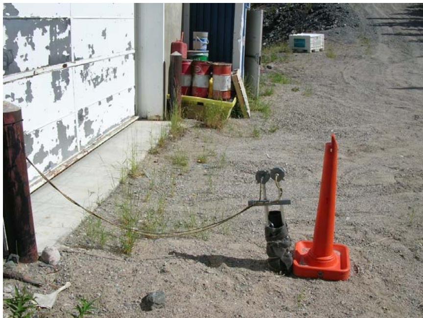
Photo 80 Snare Forks Powerhouse - heat traced perforated PVC pipe installed along the SW side of the powerhouse to address the minor seepage observed from the rockfill downstream.
