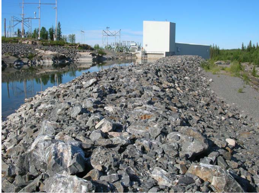
Photo 49 Snare Cascades Power Canal Dyke – slight narrowing of the crest at about mid-dyke in an area where additional rockfill has been added to cover the previously observed exposures of concrete cut-off wall.
