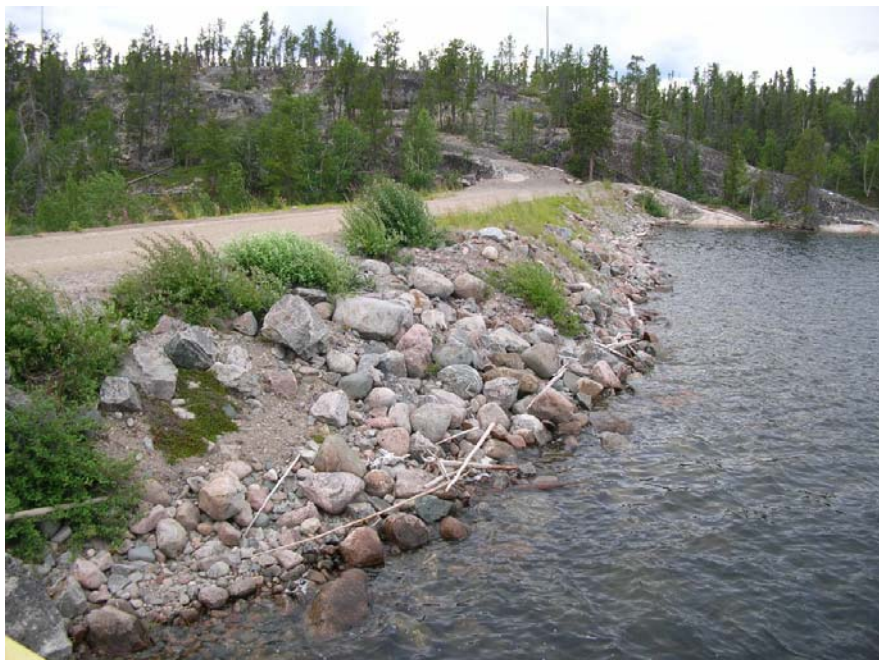
Photo 2 Snare Rapids Main Dam – vegetation along crest shoulder and upstream face to be removed
