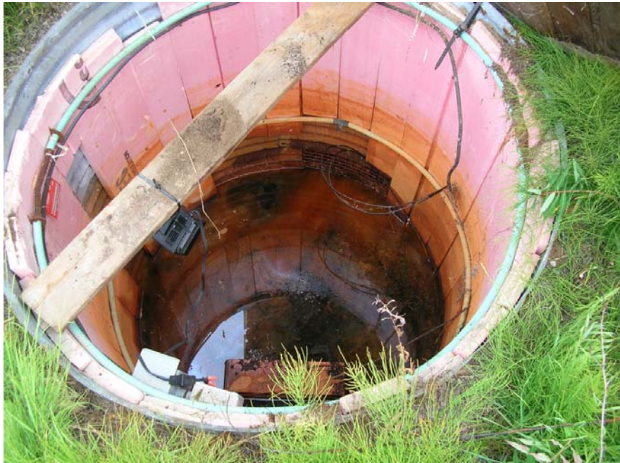
Photo 5 Snare Rapids Main Dam – heated sump collecting seepage from downstream left abutment. No inflows at time of inspection.
