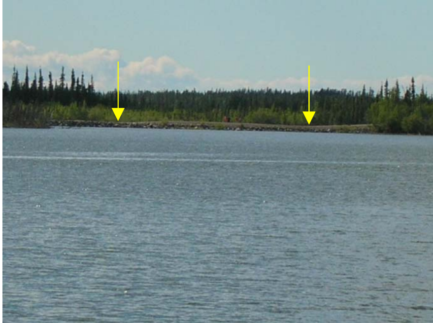
Photo 67 Freeboard Dyke 2 - crest exhibits an undulating profile with two visible depressions in the crest – one at each abutment.
