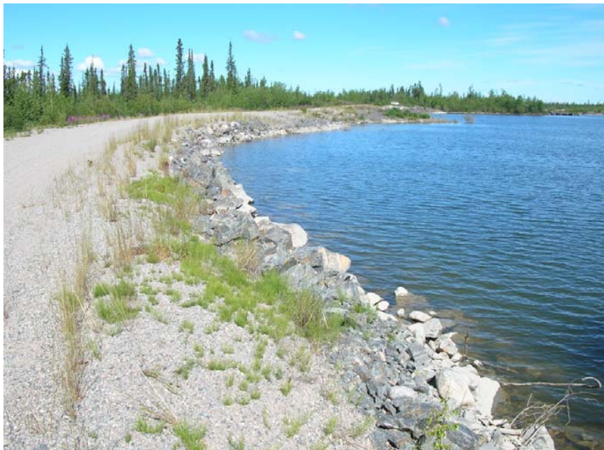
Photo 74 Freeboard Dyke 2 - upstream riprap generally satisfactory.
