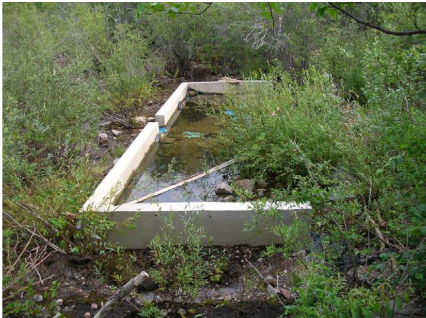
Photo 16 Side Dam 5B – general arrangement of measuring weir constructed in 1999 downstream of Side Dam 5B seepage area.
