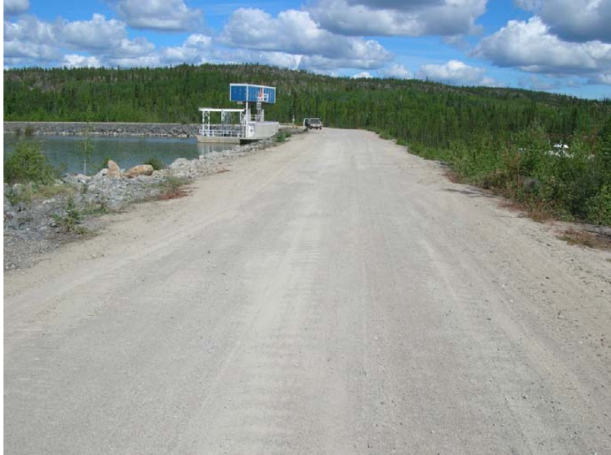
Photo 77 Strutt Lake Dam - crest is planar, with no visible settlement, cracks or erosion.
