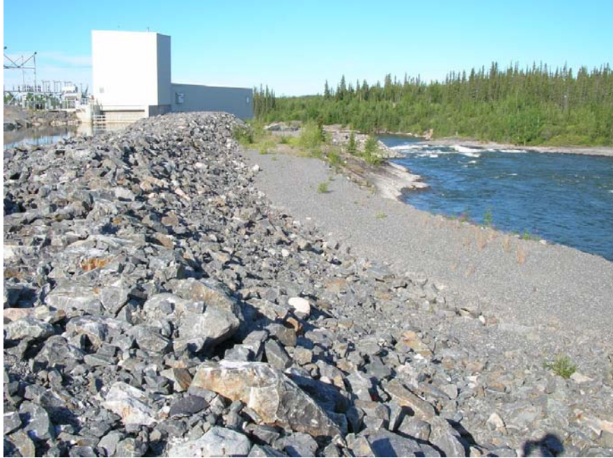
Photo 51 Snare Cascades Power Canal Dyke - downstream slope is planar with no signs of erosion, instability or seepage.
