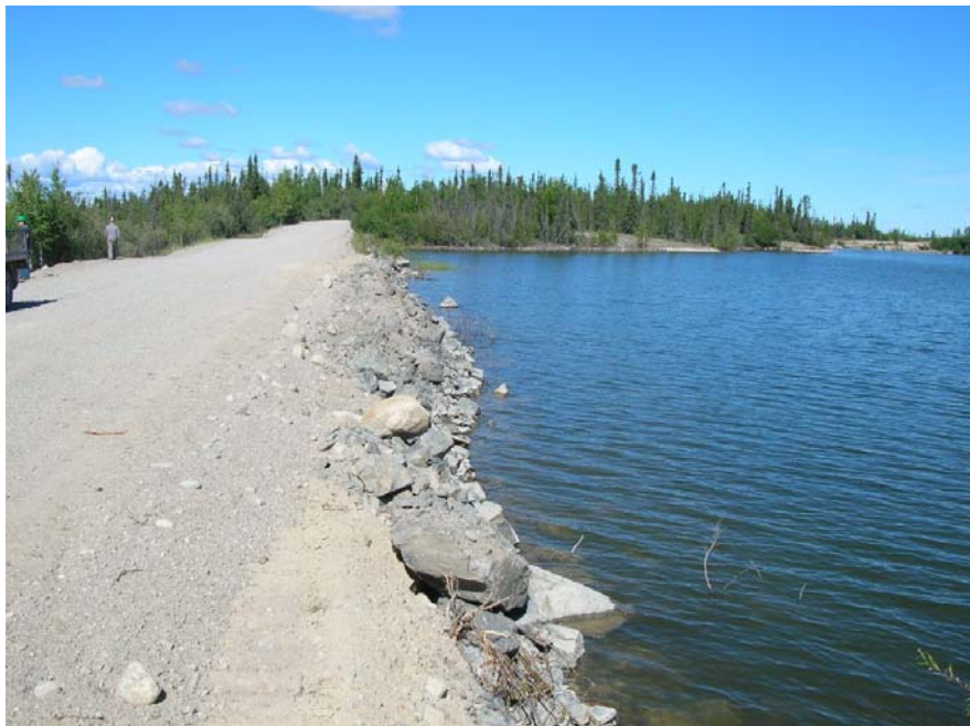
Photo 68 Freeboard Dyke 2 – crest exhibits no longitudinal cracking but recently placed sand fill may mask actual condition.
