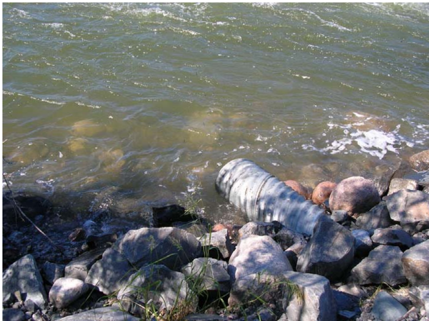
Photo 62 Snare Forks Dam – the outlet of the culvert through the cofferdam is partly submerged during spillway operation precluding seepage measurement.
