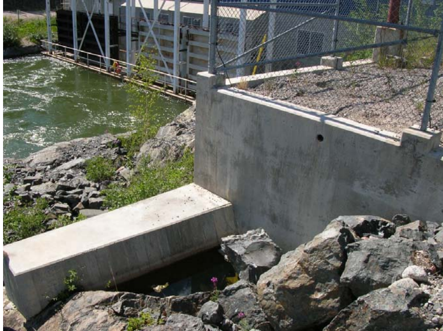
Photo 85 Snare Forks Powerhouse - minor seepage through the bedrock near the SE corner of the powerhouse and switchyard as evident by the ponded water at the switchyard retaining wall.
