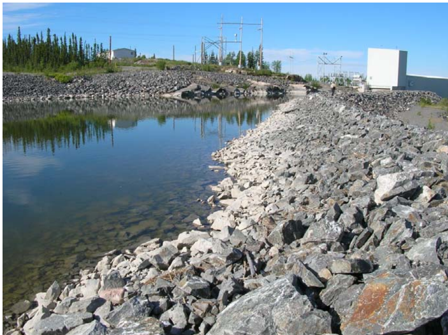
Photo 50 Snare Cascades Power Canal Dyke - upstream slope is typically planar with a slight distortion in the slope of the fill in the area where the new rockfill was added. The rockfill is in good condition.
