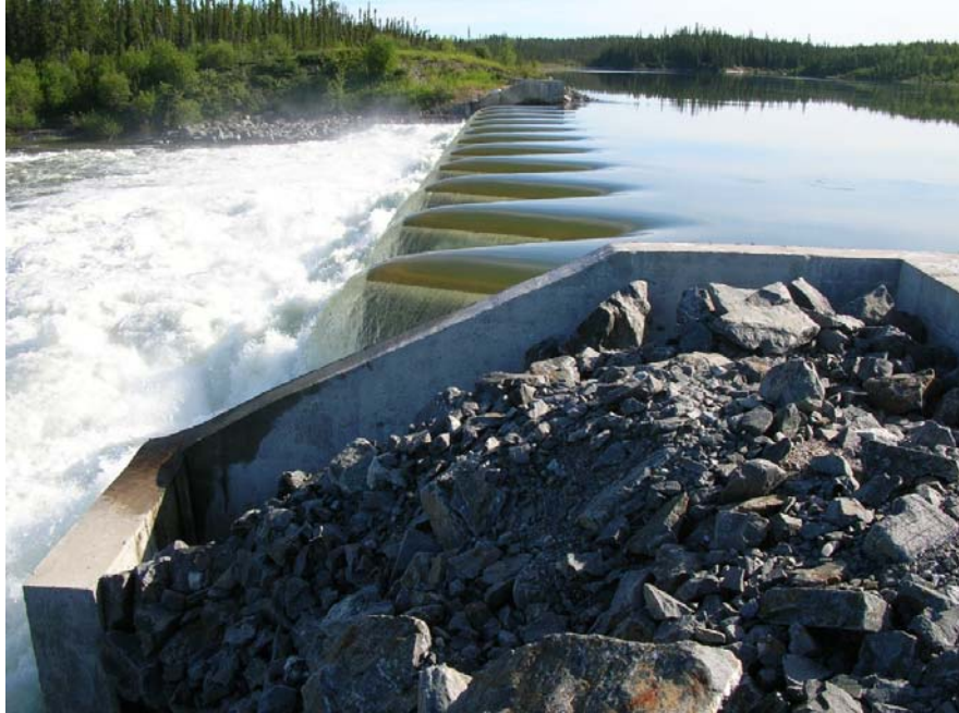
Photo 47 Snare Cascades Spillway – flow over the labyrinth spillway is smooth and uniform. Q = 126 \text{ m}^3/\text{s}
