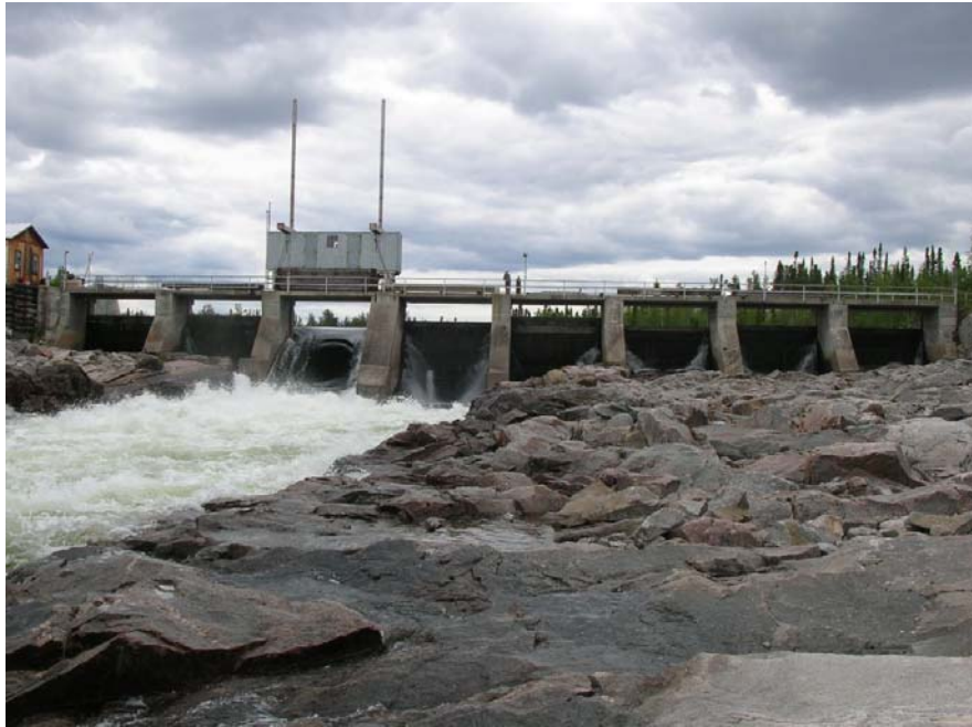
Photo 9 Spillway 5B – general view from downstream. Q = 142 \text{ m}^3/\text{s} .
