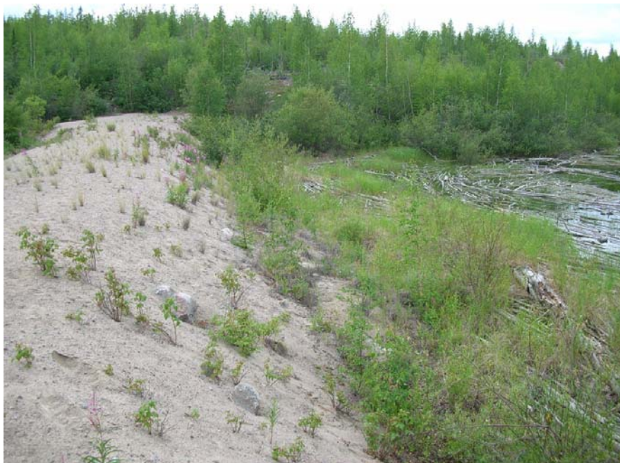
Photo 28 Side Dam 9B - upstream slope of the dam shows some signs of minor rutting in areas due to surface run-off. 30 cm layer of fine rockfill or crushed gravel recommended. Brushing required as part of on-going maintenance.
