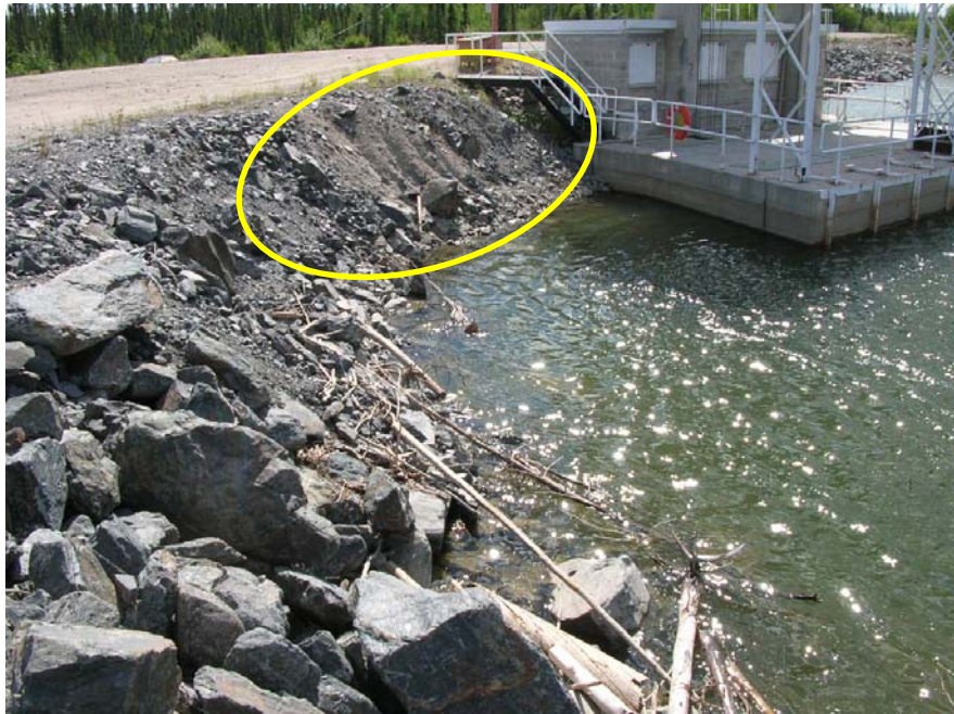
Photo 79 Strutt Lake Dam - riprap on the upstream slope is generally satisfactory. Localized area immediately left of the intake lacks some larger size particles. Monitoring required.
