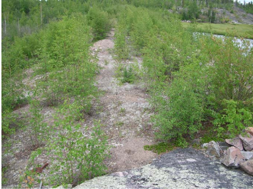
Photo 21 Side Dam 4 – typical crest condition. Some minor erosion and undulations in profile. Brushing of crest and slopes required to permit proper inspection in the future.
