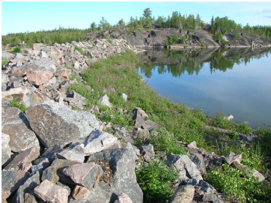
Photo 32 Snare Falls Dam – upstream riprap satisfactory. Brushing recommended as part of on-going maintenance.
