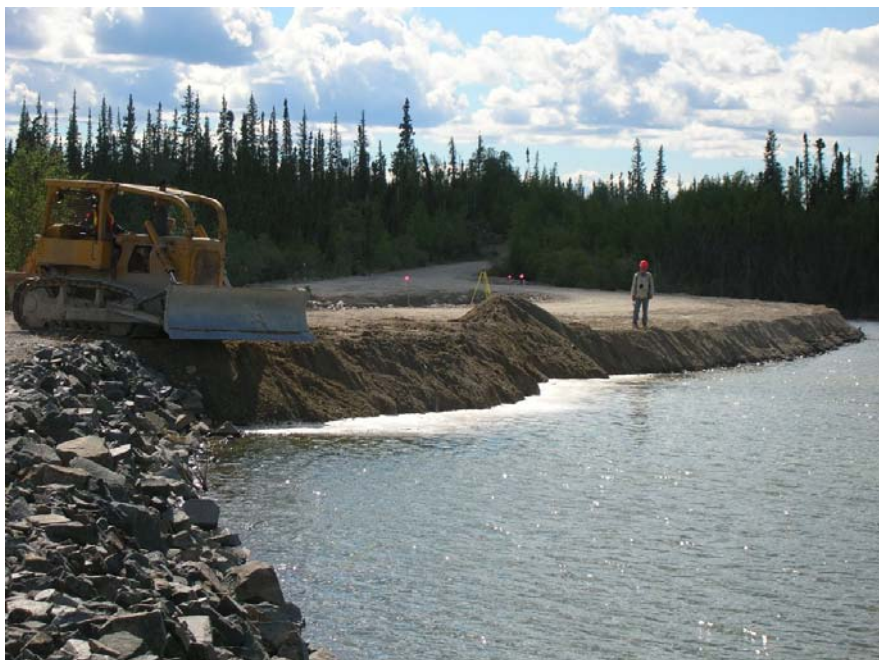
Photo 66 Freeboard Dyke 1 – reconstruction in progress following breach in June 2006.
