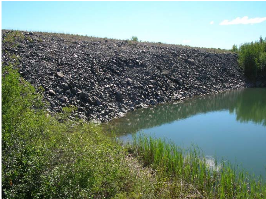
Photo 65 Snare Forks Dam - downstream shell is planar with no settled areas or evidence of instability.
