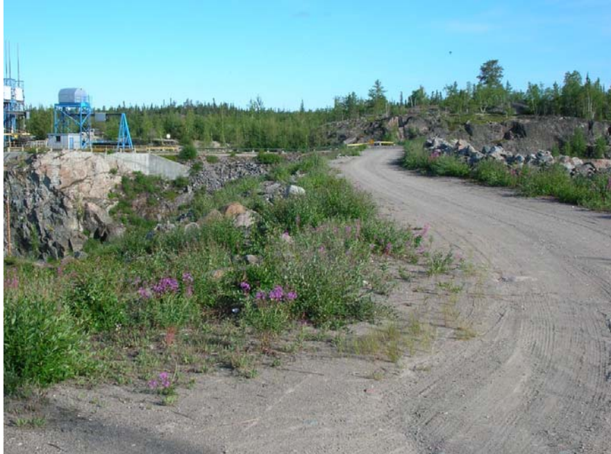
Photo 31 Snare Falls Main Dam – crest condition satisfactory. Brushing recommended as part of on-going maintenance.
