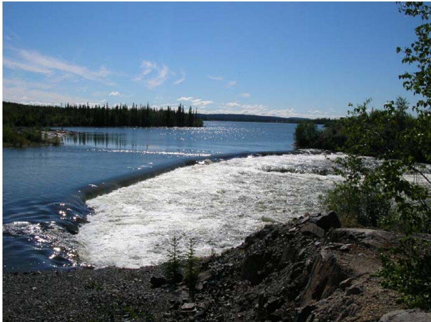
Photo 59 Snare Forks Spillway - flow over the concrete spillway is smooth with no irregularity in the flow pattern, Q = 85 \text{ m}^3/\text{s} .
