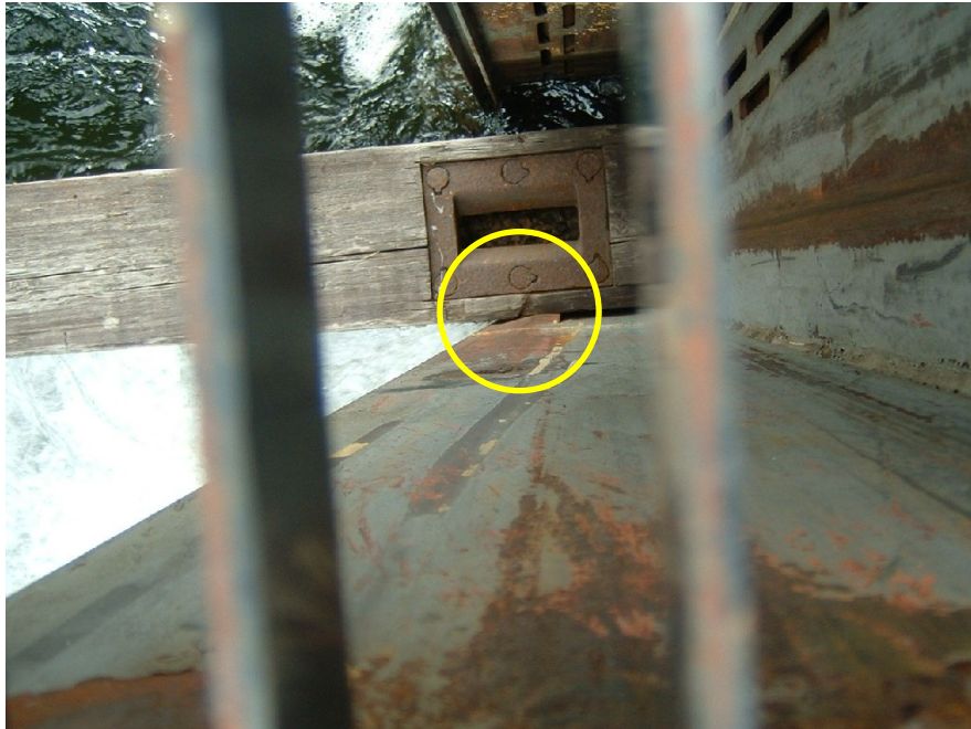
Photo 15 Spillway 5B - 1 cm bulge and corresponding tear in the left side steel embed of spillway Bay 4, approximately 2 m below deck level.
