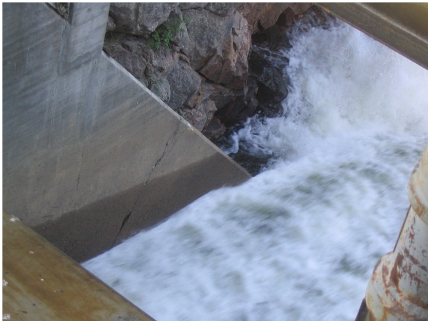
Photo 36 Snare Falls Spillway - diagonal cracks on the downstream end of both abutment piers unchanged from previous inspections.
