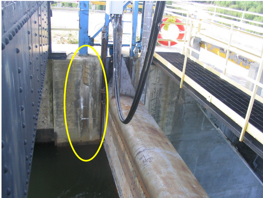
Photo 37 Snare Falls Spillway - vertical cracks in concrete adjacent to left gate guide (heated).
