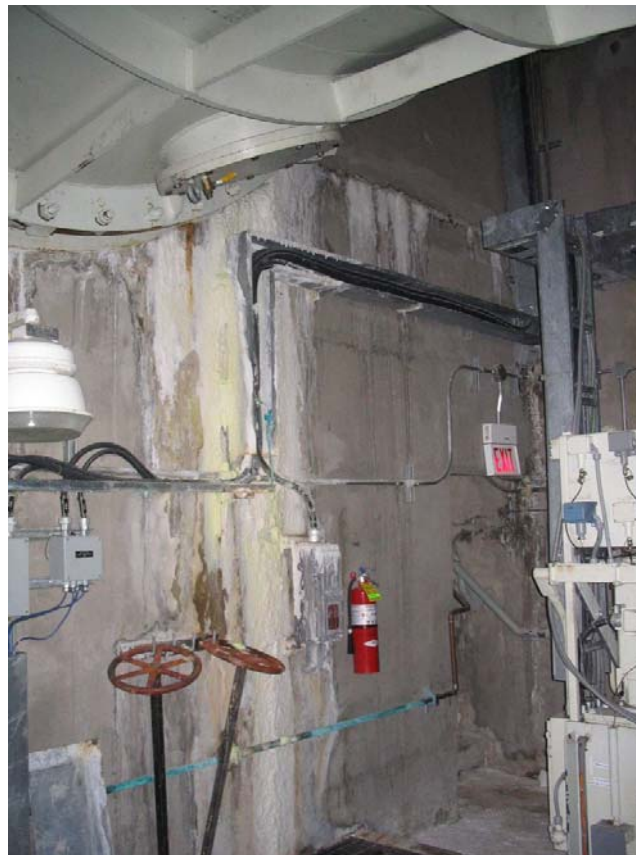
Photo 58 Snare Cascades Intake and Powerhouse - multiple zones of cracks, seepage and efflorescence.
