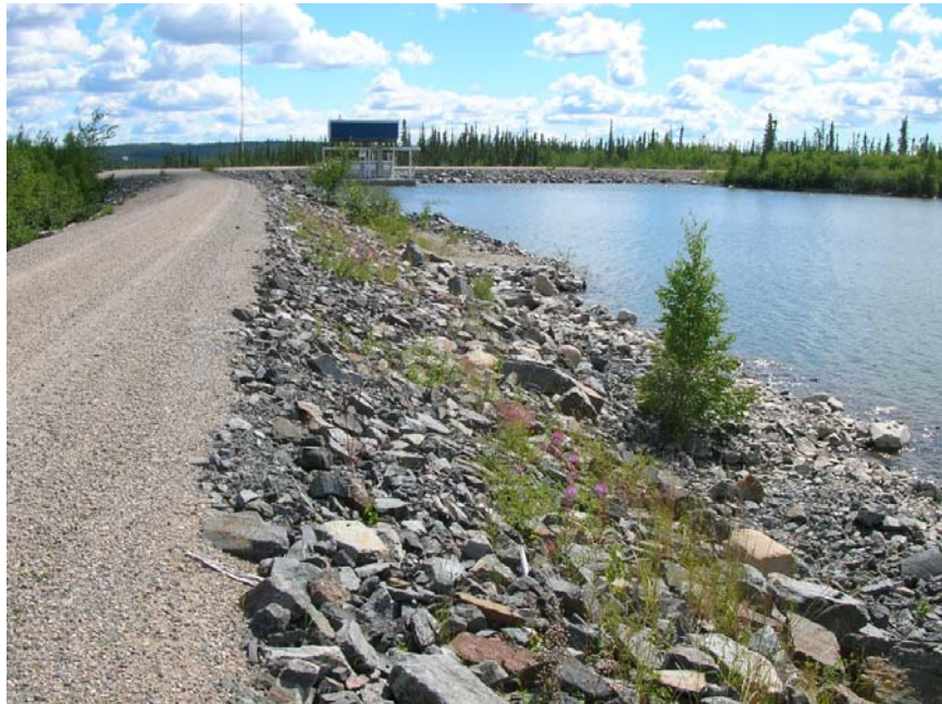
Photo 83 North Dyke - riprap on the upstream face is satisfactory. .
