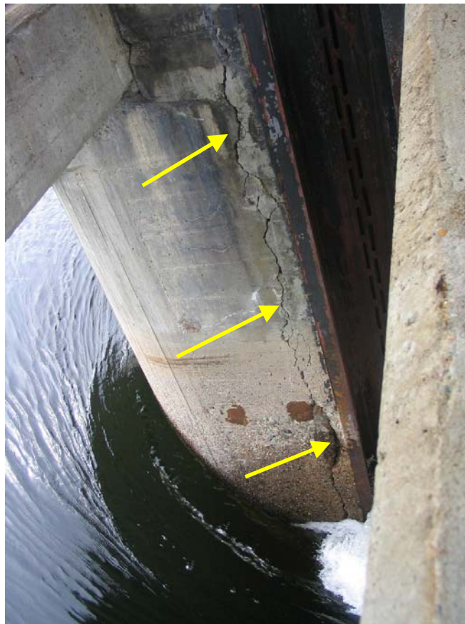
Photo 14 Spillway 5B - cracks in the second stage concrete around the heated gains in spillway Bay 3 and 4.
