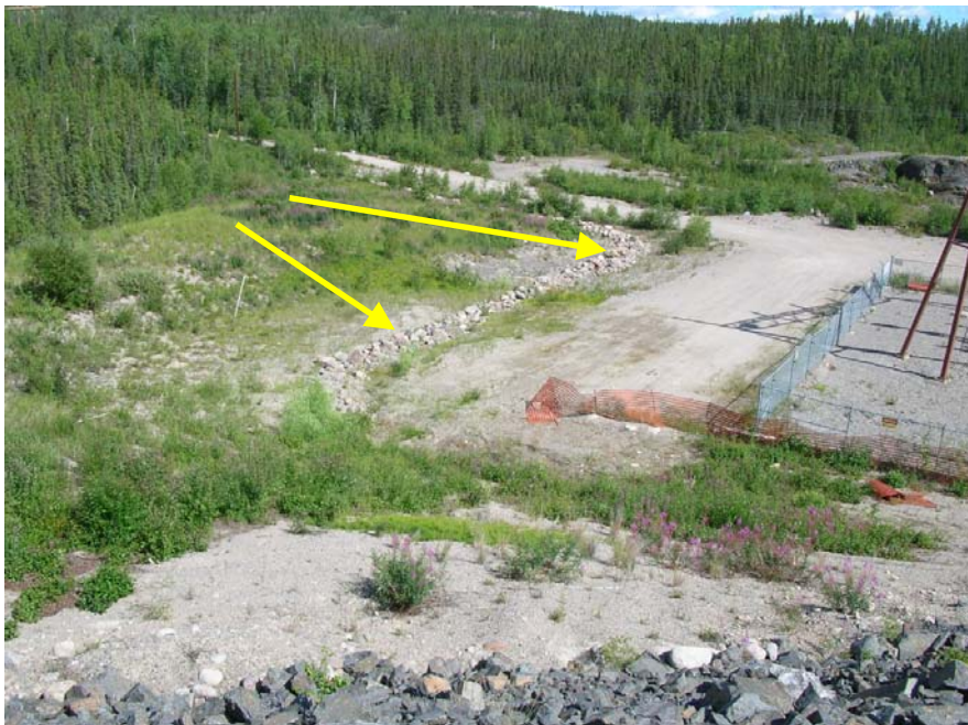
Photo 76 Strutt Lake Dam - rock fill French drain between downstream toe and switchyard. Drain outflows not monitored. Dry at the time of inspection.
