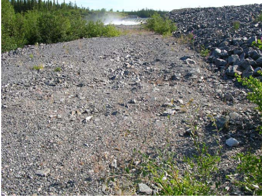
Photo 53 Snare Cascades Power Canal Dyke - some localized depressions in the surface of the lower bench crest near the upstream end.
