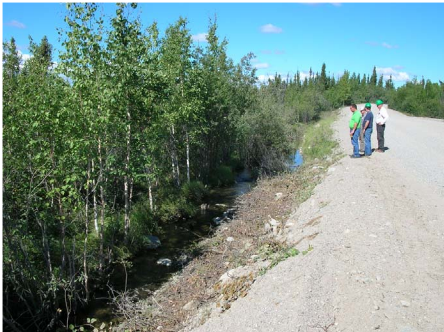
Photo 72 Freeboard Dyke 2 –seepage from foundation flows down the toe of the downstream slope, collecting in the low point.
