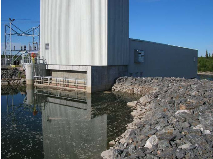
Photo 57 Snare Cascades Intake and Powerhouse - steel frame superstructure including the cladding appears in sound condition.
