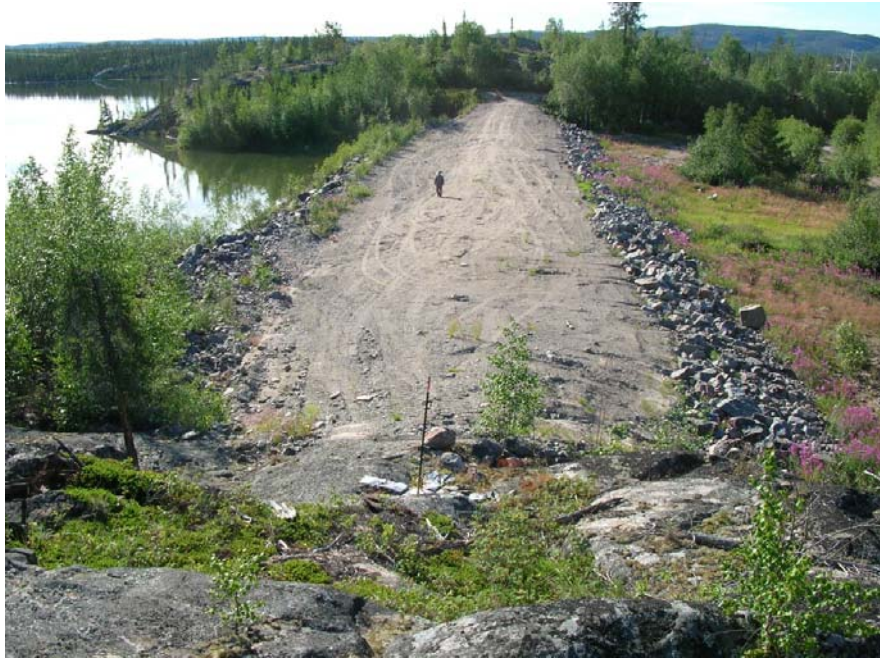
Photo 43 Saddle Dam No. 1 – crest lowered by 2.7 m in 2003 as an emergency flood handling improvement.
