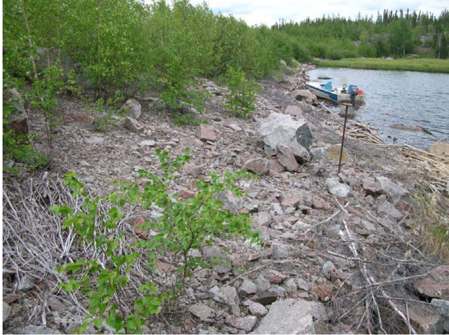
Photo 23 Side Dam 4 – upstream face riprap showing signs of deterioration towards the left abutment.
