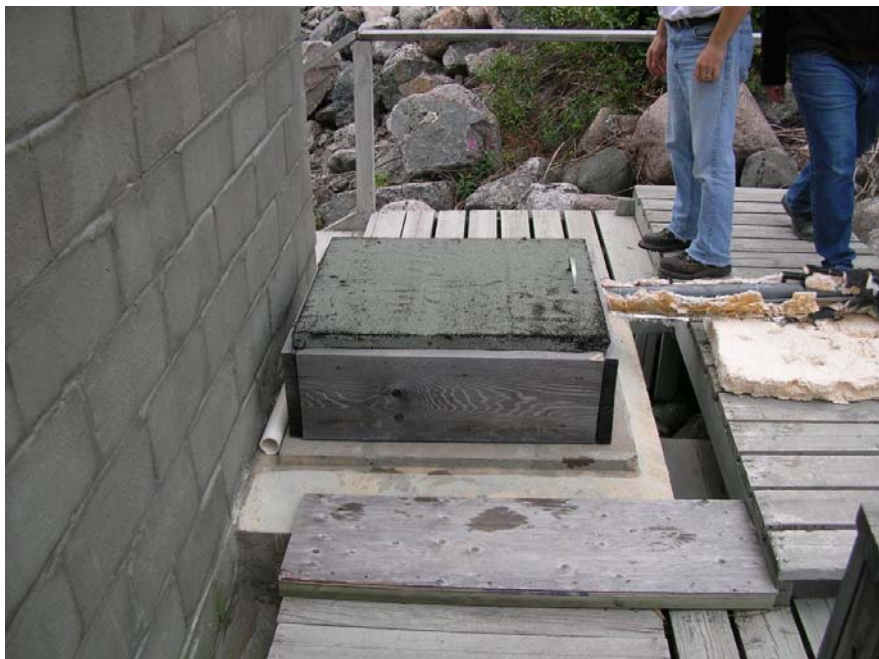
Photo 8 Snare Rapids Power Tunnel – seepage collection and measurement sump for seepage from the power tunnel.
