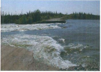
Figure 1: Breach in side weir (Dyke #1)
