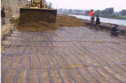
Geogrids are typically installed horizontally between layers of fill material to reduce the likelihood of sloughing. Advantages
