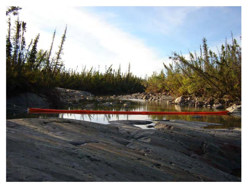
Photograph 3: View of Upper Reach from Rock Cascade (Silt Curtain #2)
