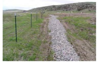
Exhibit 9: Example of a Filter Berm (geotextile fabric not visible)
