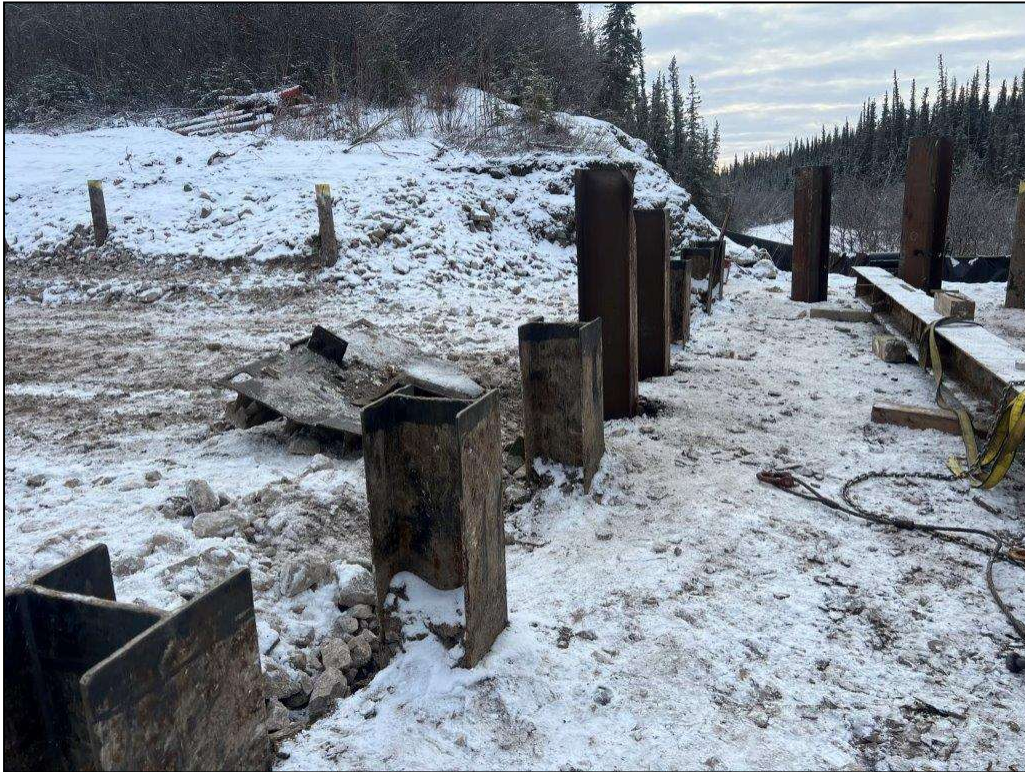
Photo 5 – Existing Dead Man Wall Piles
