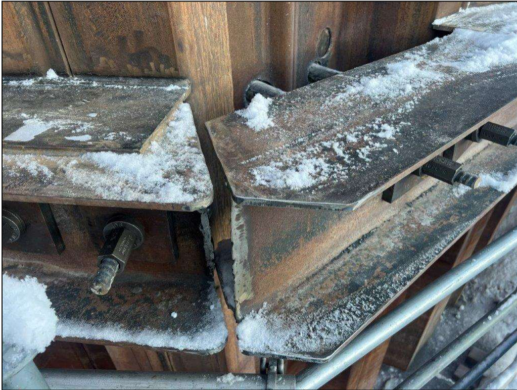
Photo 9 – Existing Sheet Pile Wall Waler Cut at Corner
