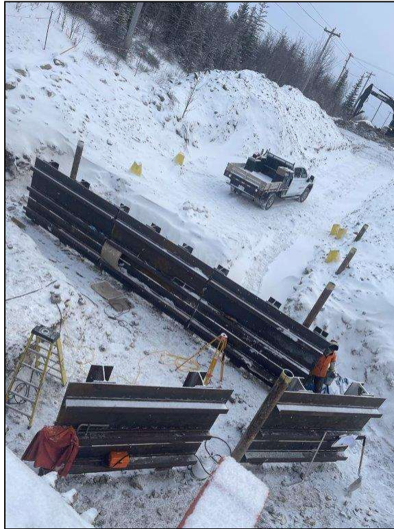
Photo 3 – New and Existing Dead Man Wall Reinforced Plates
