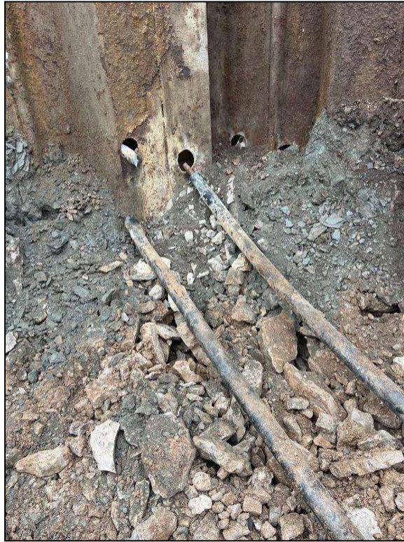
Photo 7 – Existing Tieback Structure Broken Threadbar
