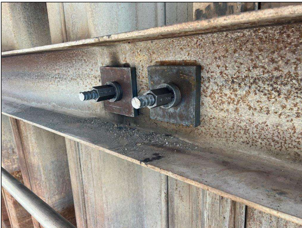
Photo 10 – Threadbar Washers and Nut (Typical)
