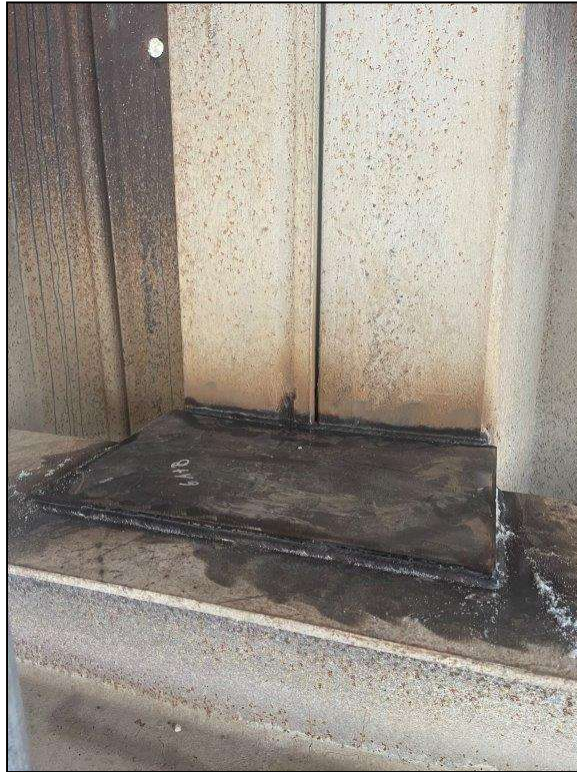
Photo 1 – Existing Sheet Pile Wall Waler Top Flange Connection (Typical)
