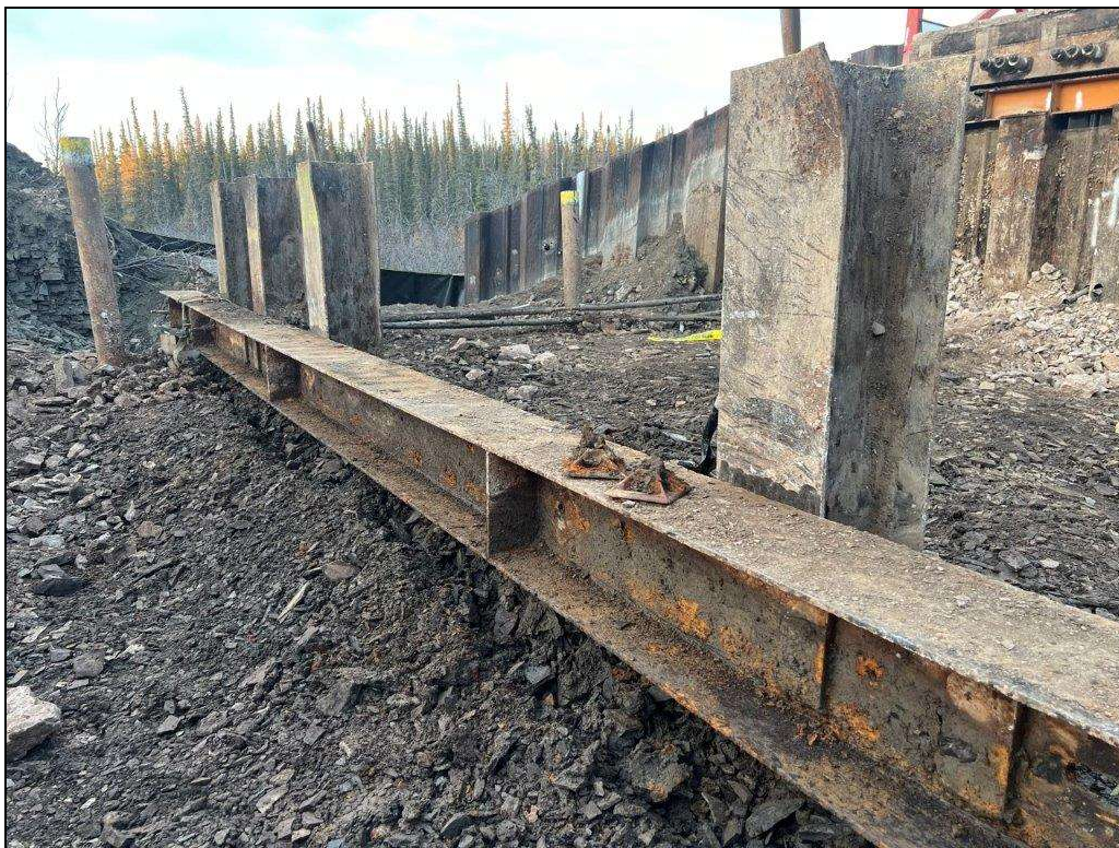
Photo 6 – Existing Tieback Structure
