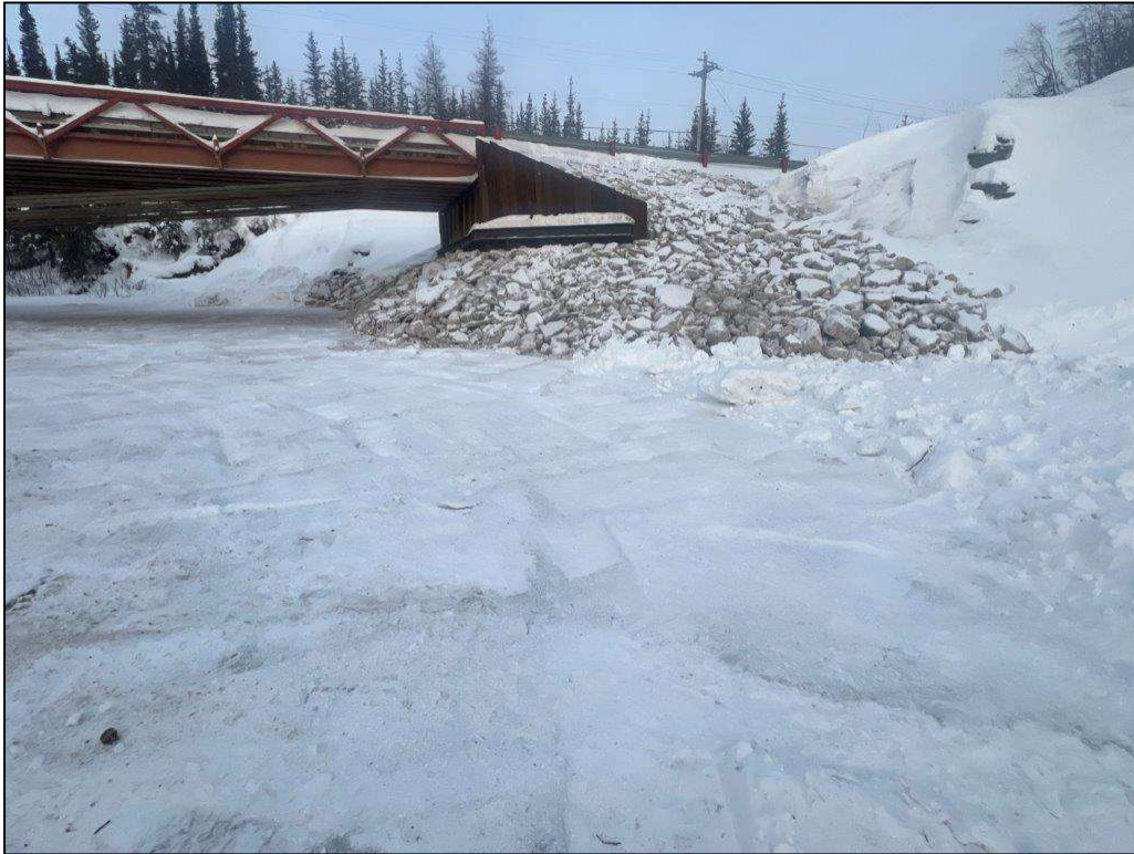
Photo 15 – Sheet Pile Wall With Rip Rap
