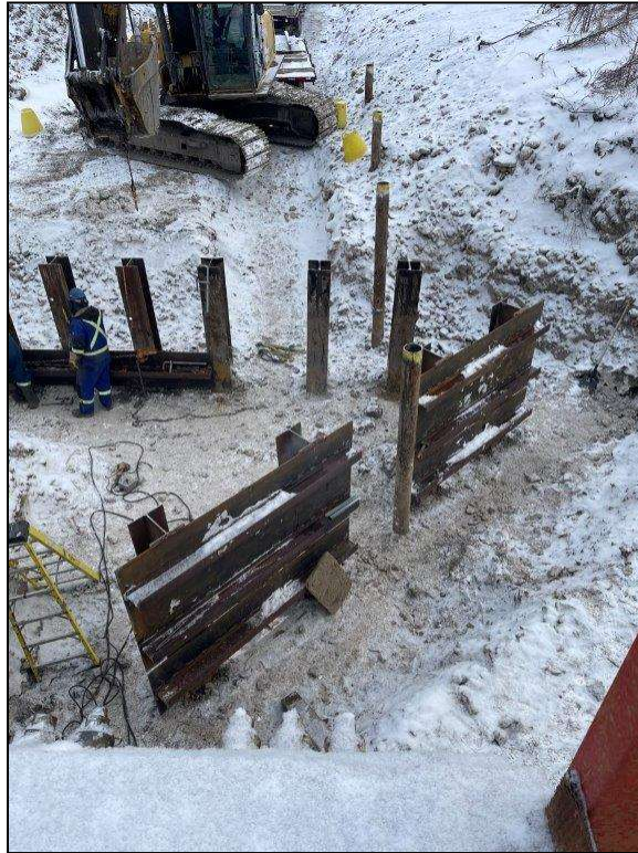
Photo 3 – New Dead Man Wall Reinforced Plates
