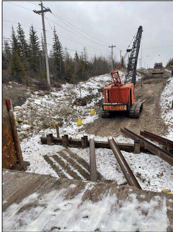
Photo 5 – Link Belt Pile Driver
