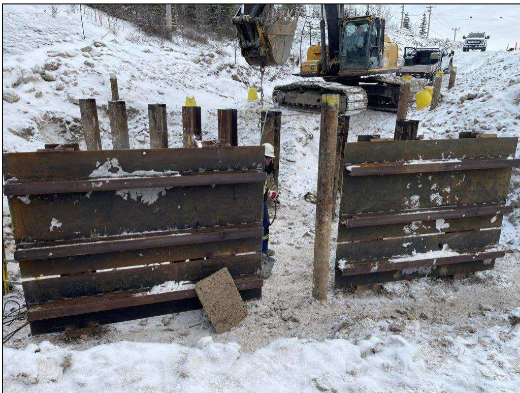
Photo 2 – New Dead Man Wall Reinforced Plates
