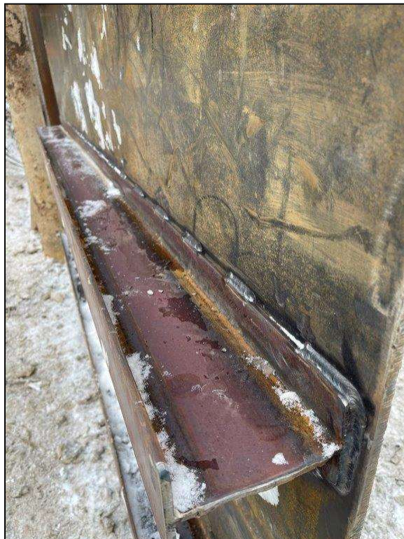
Photo 4 – New Dead Man Wall Reinforced Plate Top Stitch Welds (Typical)
