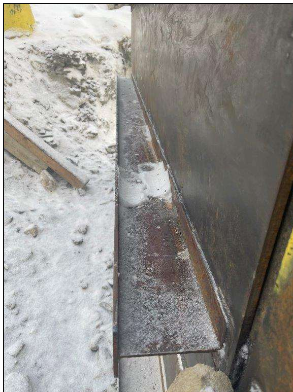
Photo 6 – Existing Dead Man Wall Reinforced Plate Top Stitch Welds (Typical)
