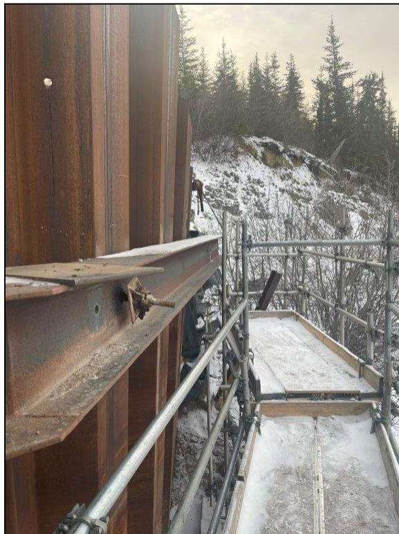
Photo 4 – Existing Sheet Pile Wall Waler
