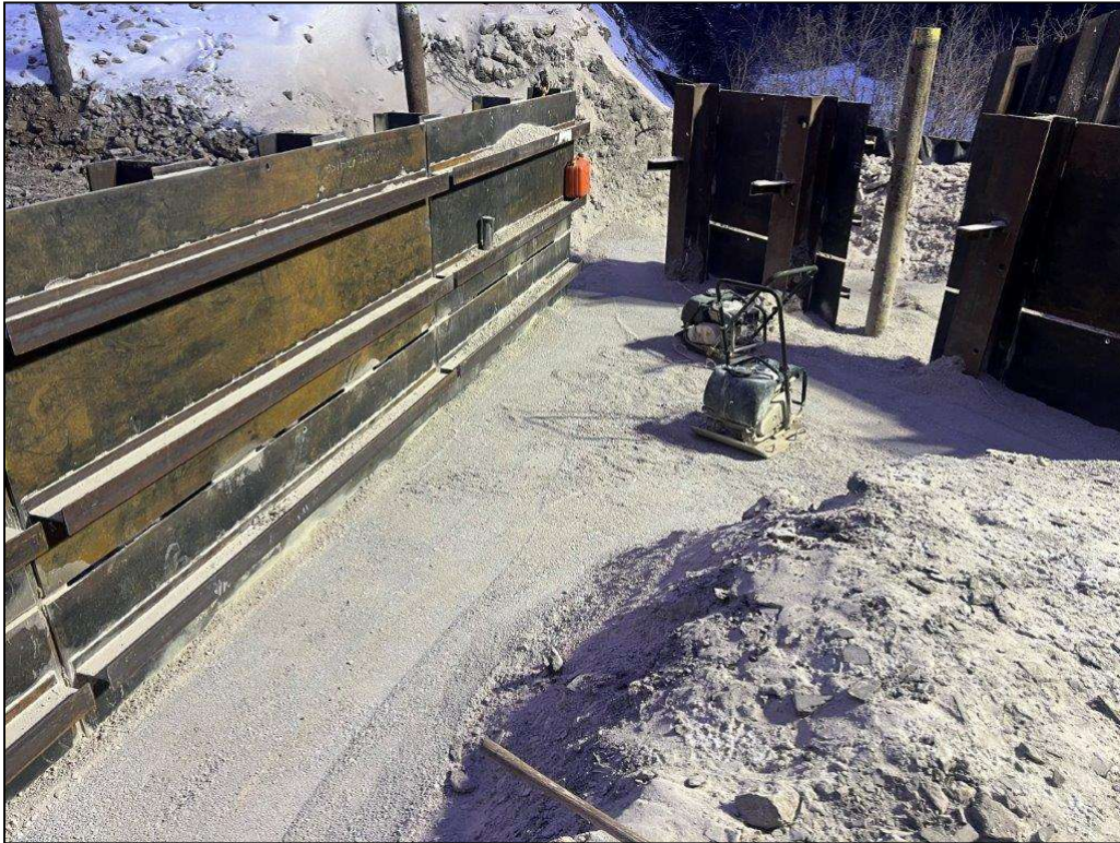
Photo 3 – Compacted Fill
