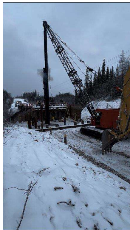
Photo 2 – Driving Piles for New Dead Man Wall
