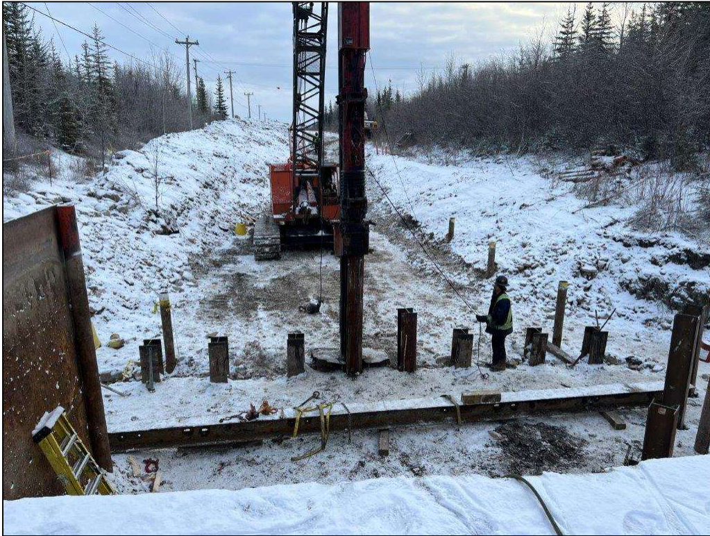
Photo 1 – Driving New Piles for Existing Dead Man Wall
