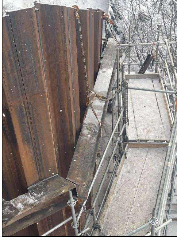
Photo 7 – Adjusting Existing Sheet Pile Wall Waler
