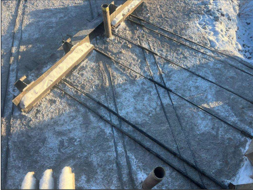
Photo 11 – New Tieback Structure Threadbars
