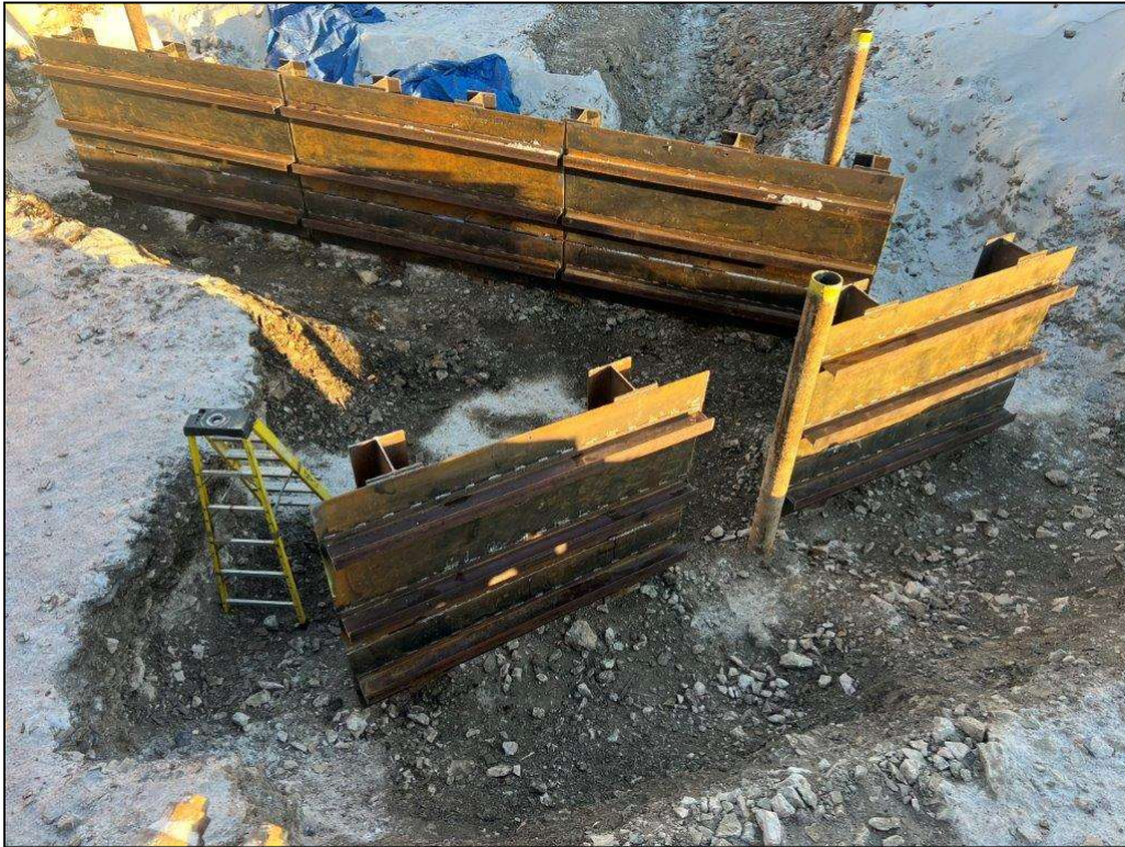
Photo 1 – Dead Man Walls Prior to Backfilling
