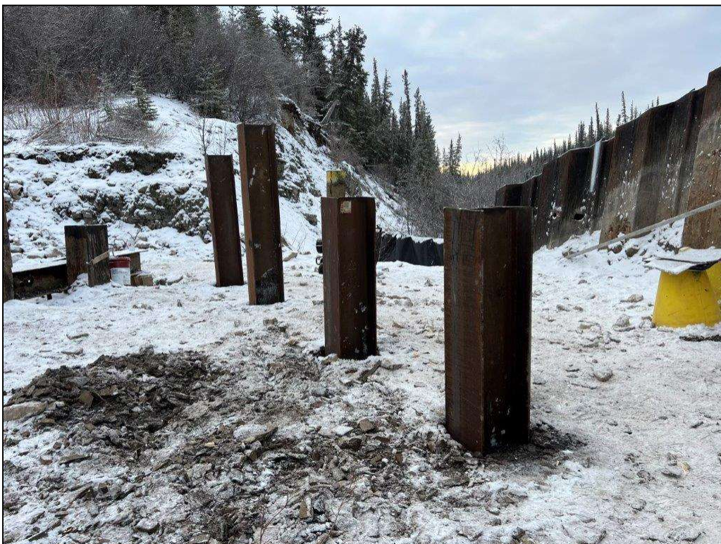
Photo 4 – New Dead Man Wall Piles
