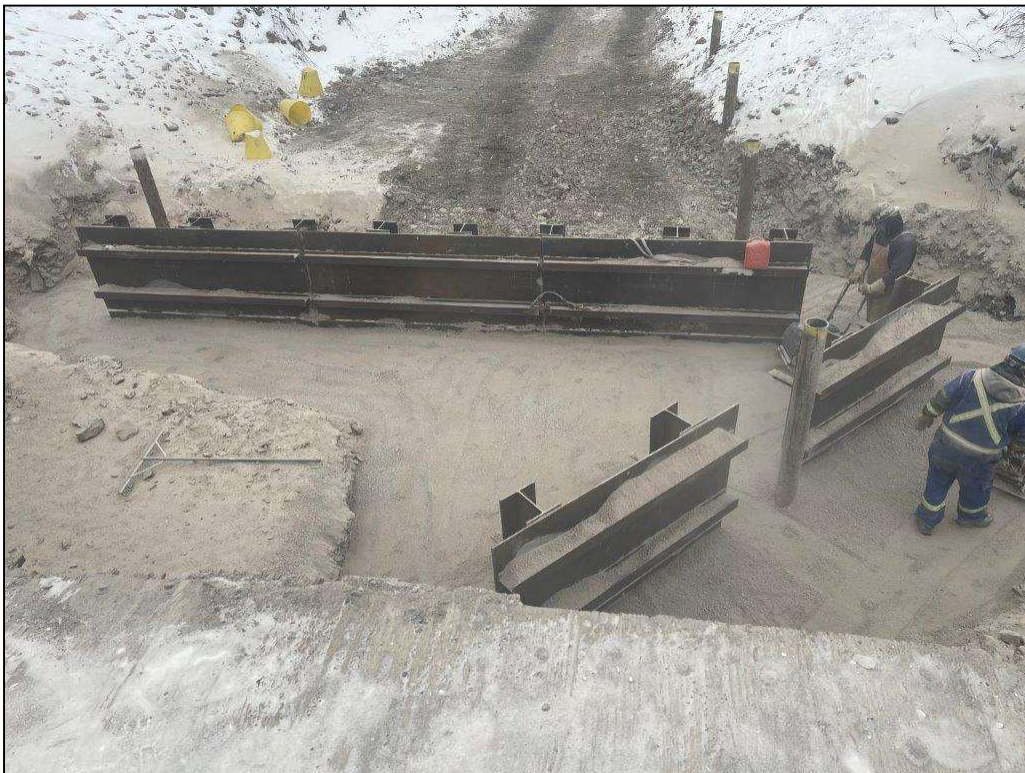
Photo 2 – Compacting Fill
