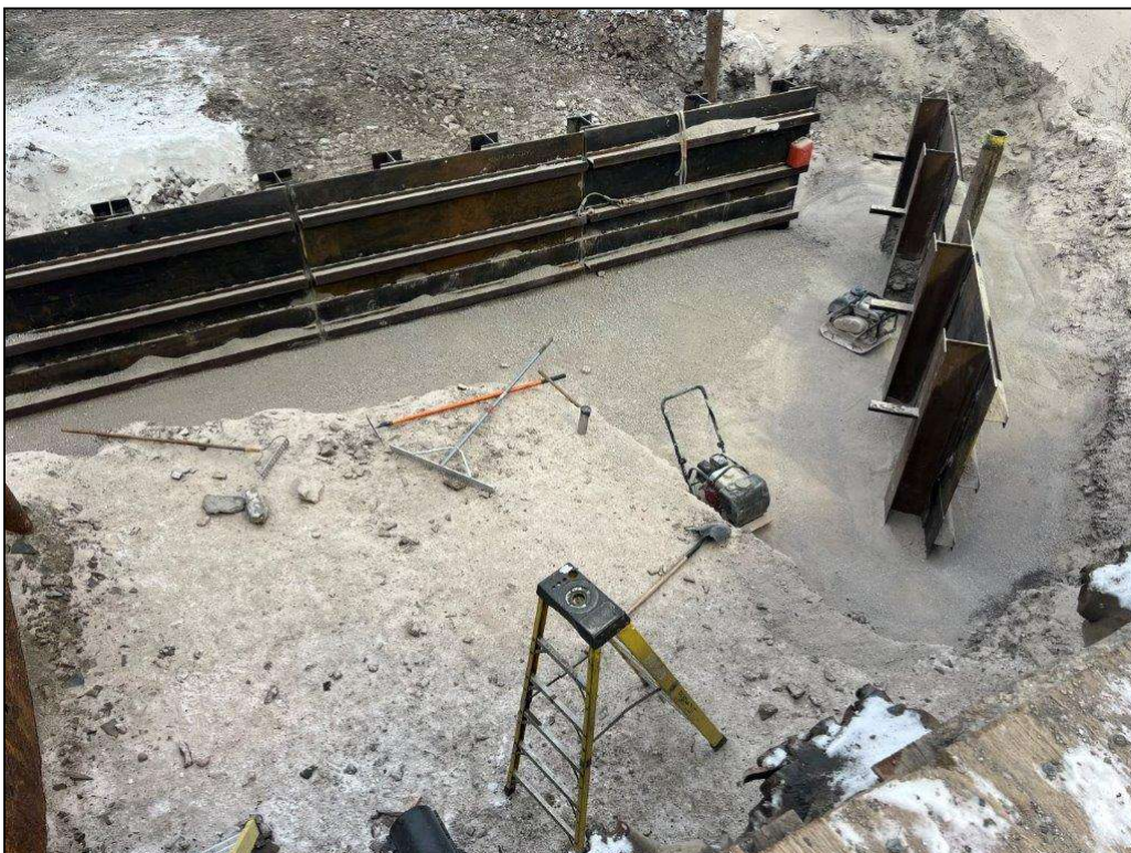
Photo 4 – Compacted Fill
