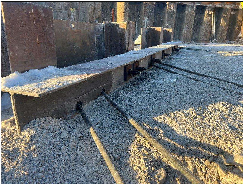
Photo 8 – New Dead Man Wall Waler and Threadbars
