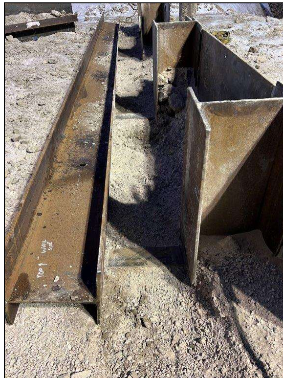
Photo 2 – Installing New Dead Man Wall Waler
