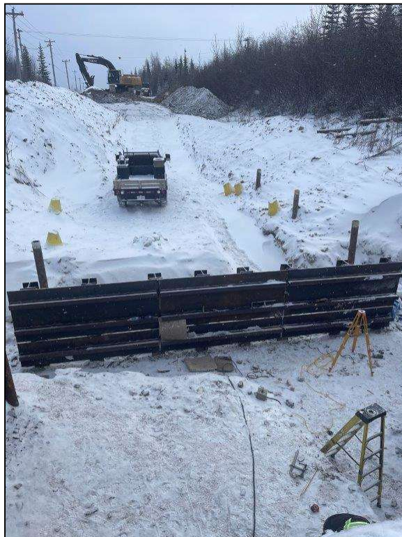
Photo 2 – Existing Dead Man Wall Reinforced Plates
