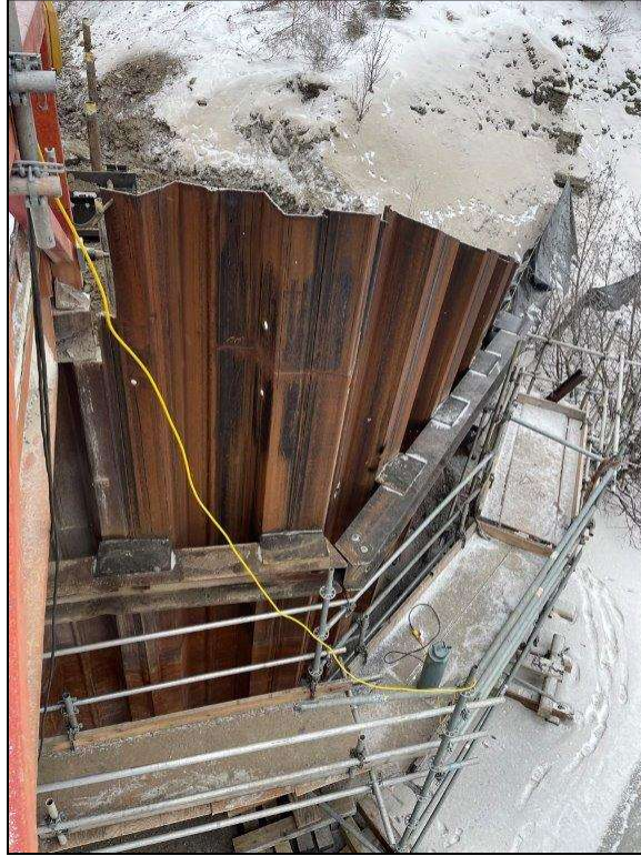
Photo 5 – Adjusted Existing Sheet Pile Wall Waler
