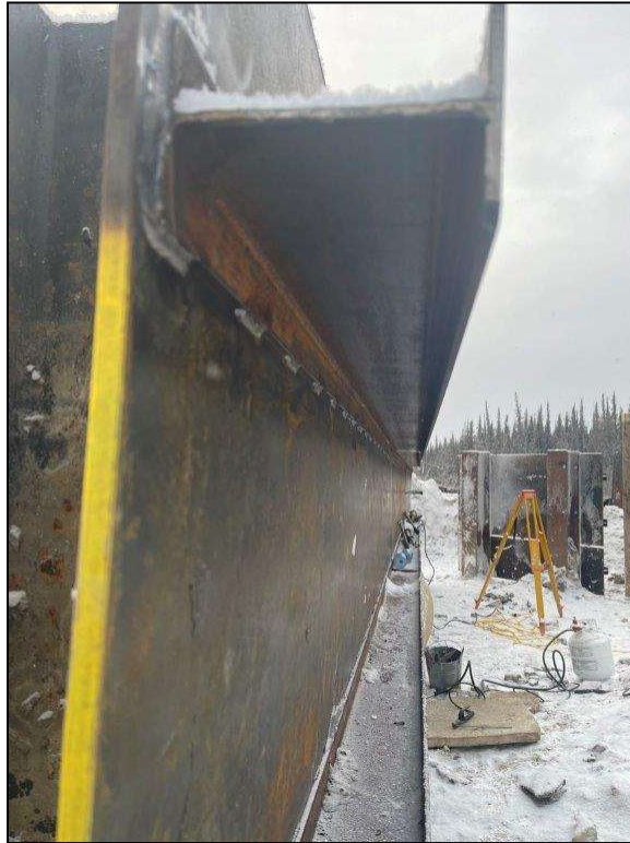
Photo 5 – Existing Dead Man Wall Reinforced Plate Bottom Stitch Welds (Typical)
