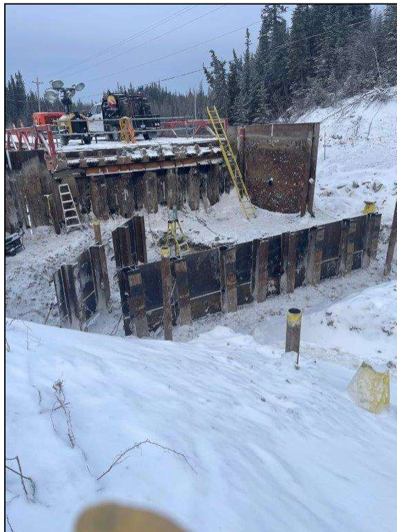
Photo 4 – New and Existing Dead Man Wall Reinforced Plates
