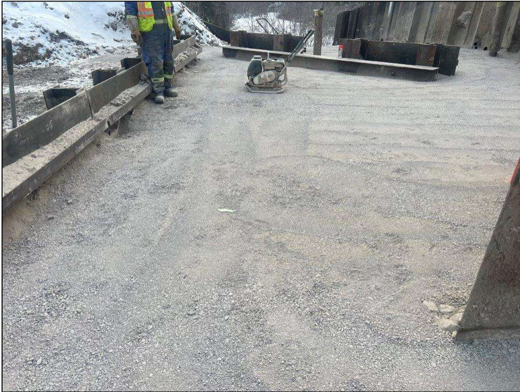
Photo 3 – Compacted Fill
