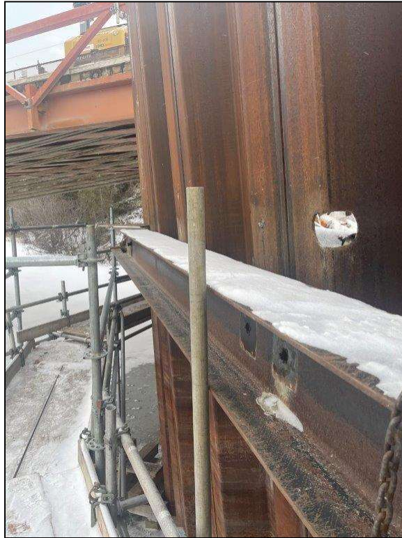
Photo 3 – Existing Sheet Pile Wall Waler
