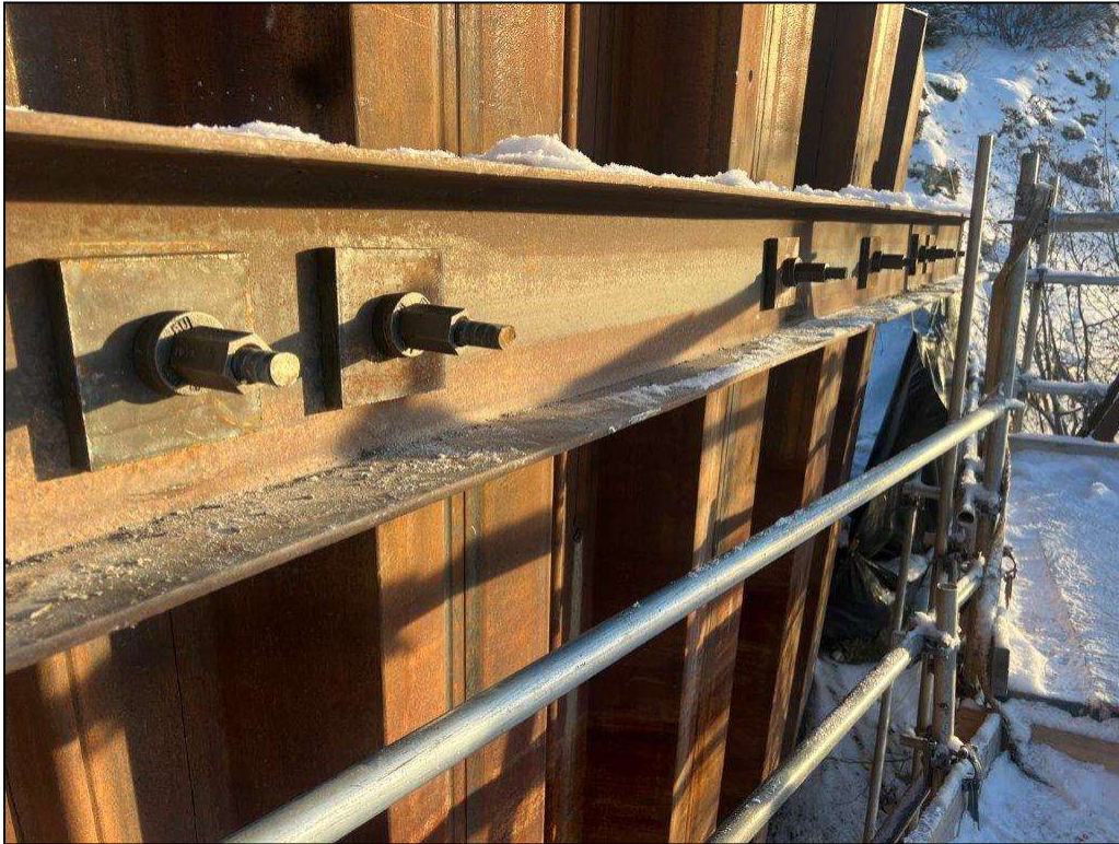
Photo 7 – Existing Sheet Pile Wall Waler
