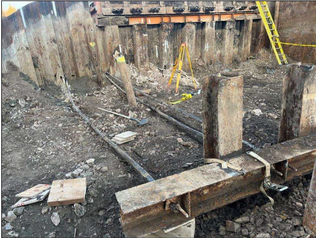
Photo 3 – Existing Tieback Structure
