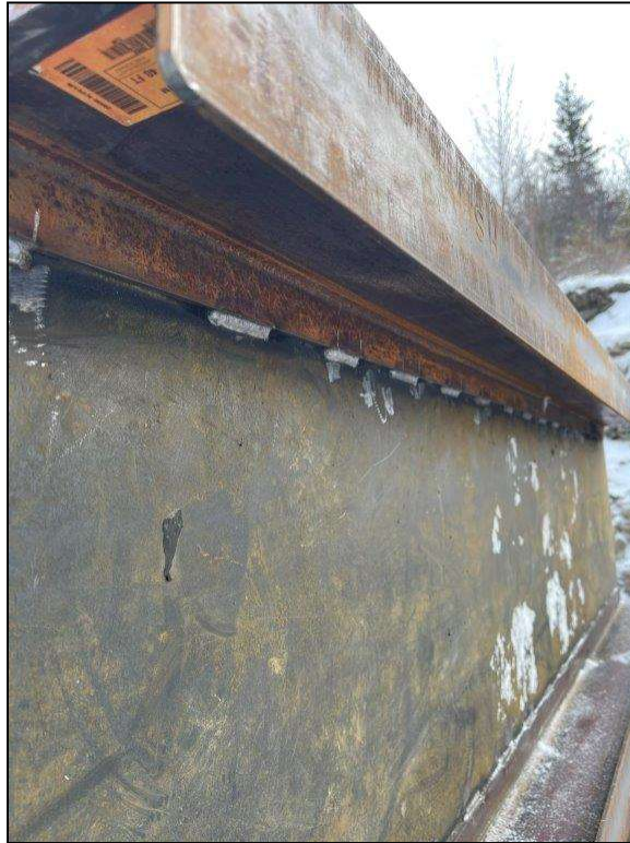
Photo 5 – New Dead Man Wall Reinforced Plate Bottom Stitch Welds (Typical)
