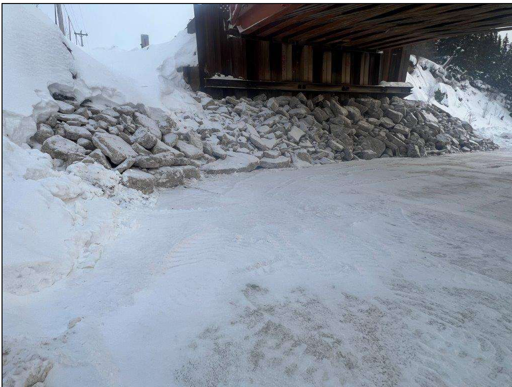
Photo 16 – Sheet Pile Wall With Rip Rap
