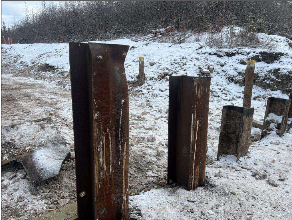
Photo 3 – New Piles for Existing Dead Man Wall
