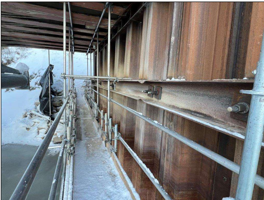
Photo 6 – Existing Sheet Pile Wall Waler
