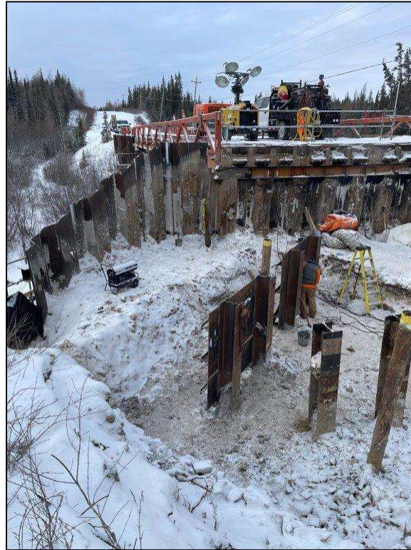
Photo 1 – Installing New Dead Man Wall Reinforced Plates
