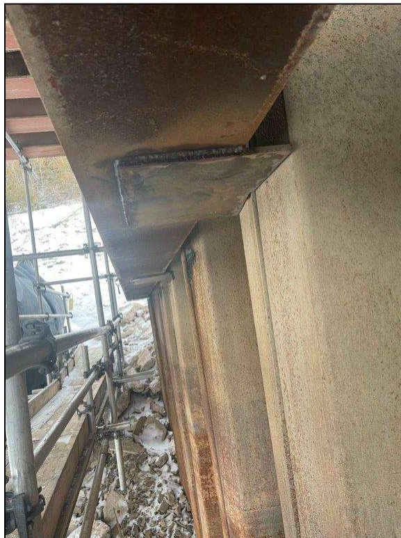
Photo 2 – Existing Sheet Pile Wall Waler Bottom Flange Connection (Typical)
