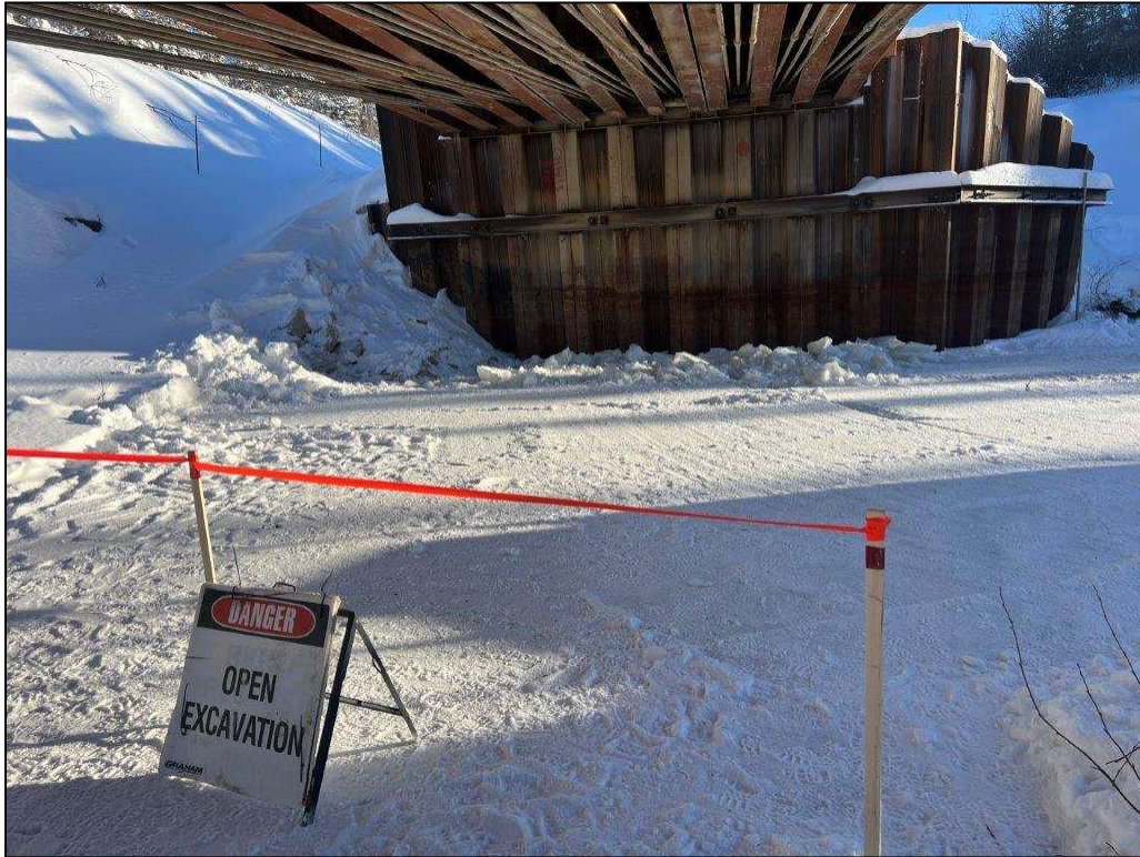
Photo 1 – Sheet Pile Wall Without Rip Rap
