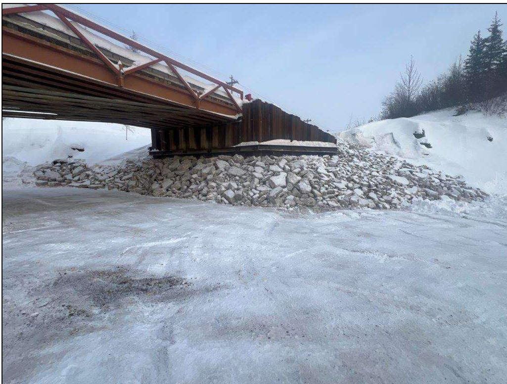
Photo 14 – Sheet Pile Wall With Rip Rap
