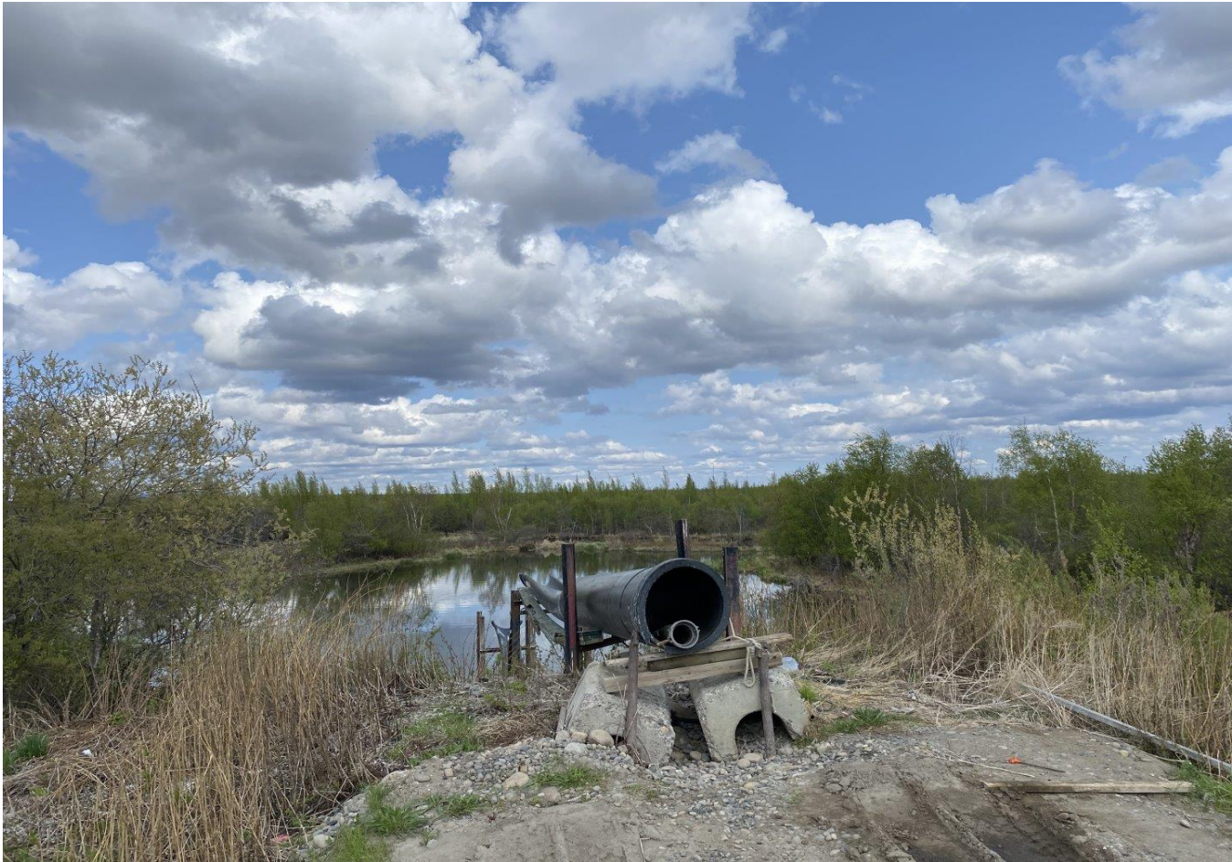
Figure 4 Water Intake Pipe to the Water Intake Facility from Great Bear River
