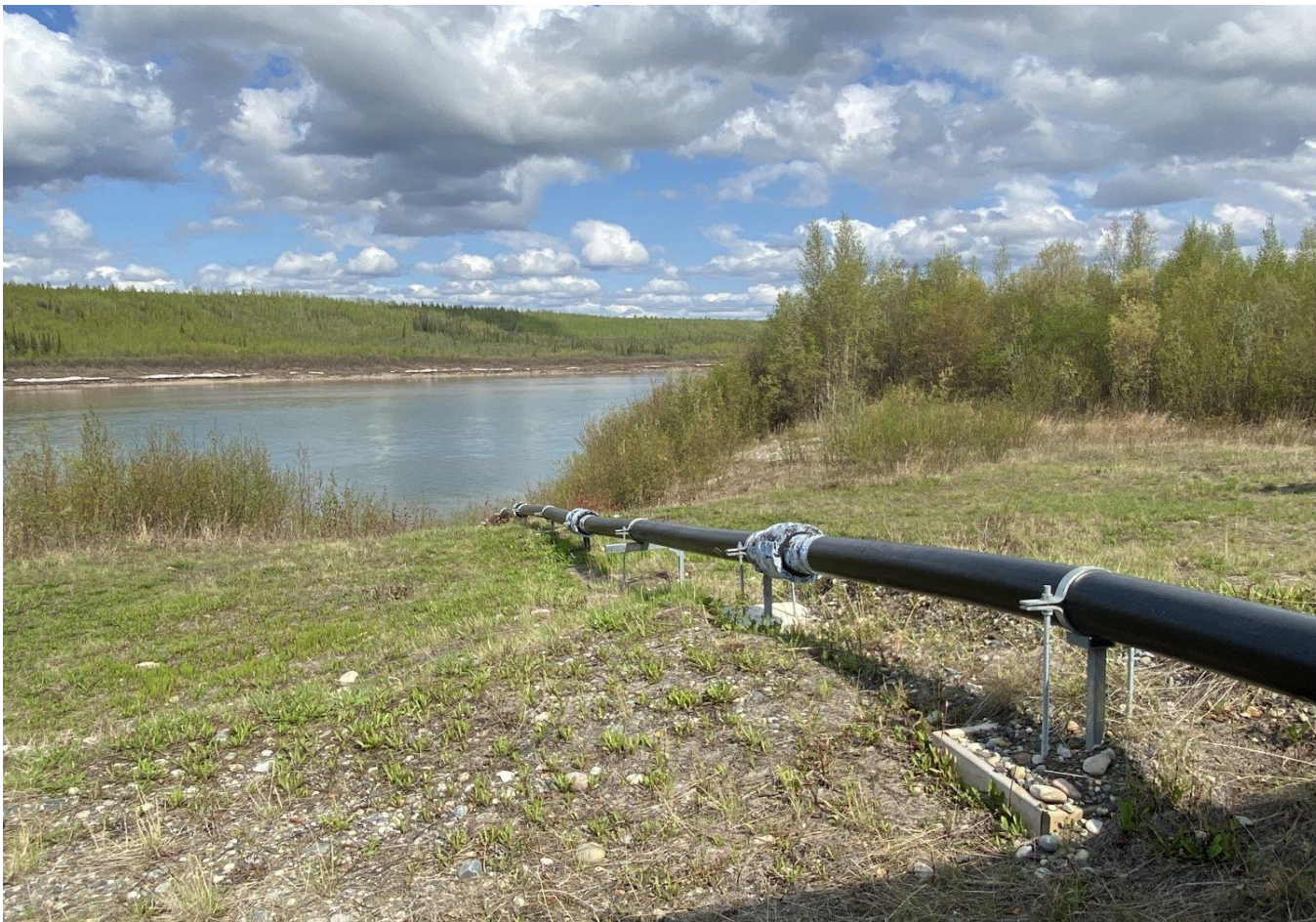
Figure 4 Water Intake Pipe to the Water Intake Facility from Great Bear River
