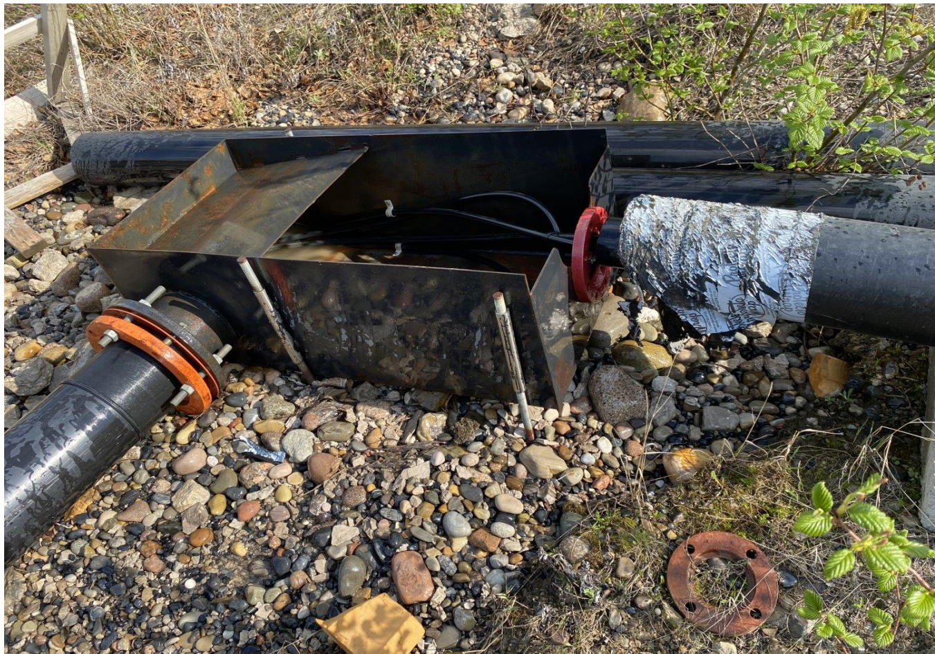
Water Intake Pipe towards the Great Bear River below water treatment plant
