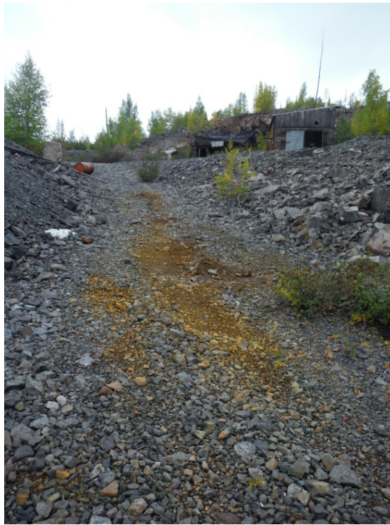
Photo 69: Iron staining at Smallwood on waste rock road leading to lake.
