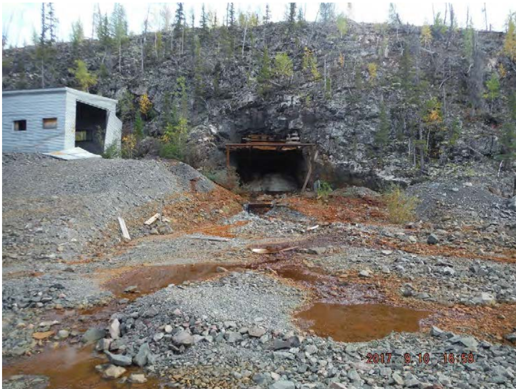
Photo 31 Norex Mine- Station NX-1: Sampled flowing water pooled in front of adit
