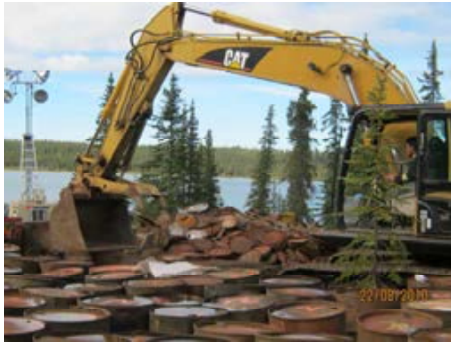
South side of the Bay cache. Crushing of barrels using excavator and platform
