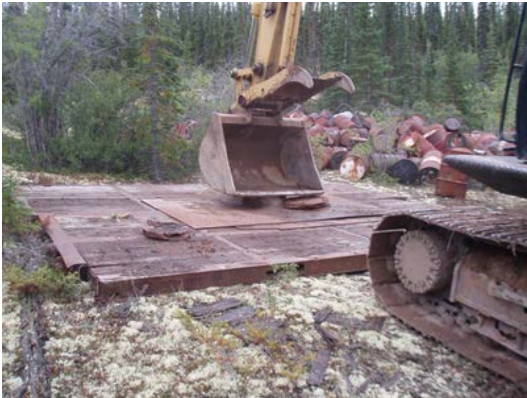
Photo 5: Crushing a drum at Sawmill Bay on August 14, 2010 ↑
