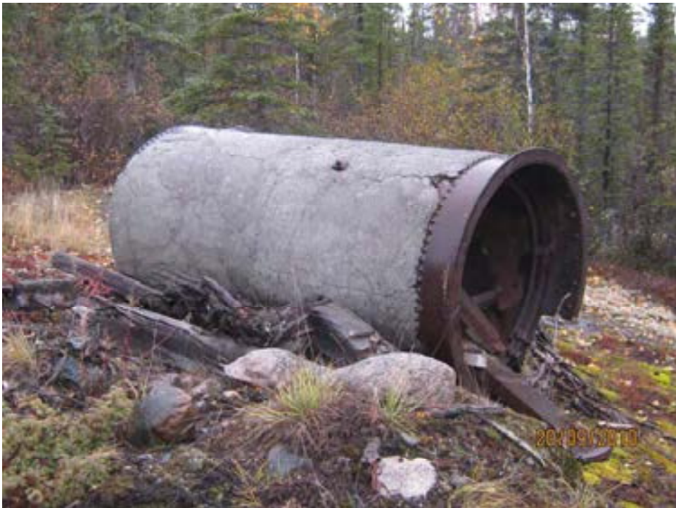
Boiler at Contact Lake East Arm coated in ACM, labelled as 'Not in Contract'
