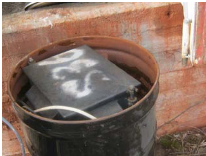
Transformer from inside Powerhouse loaded into steel overpack
