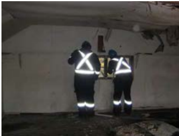
Cabin 1 DDT removal around windows and doors.
