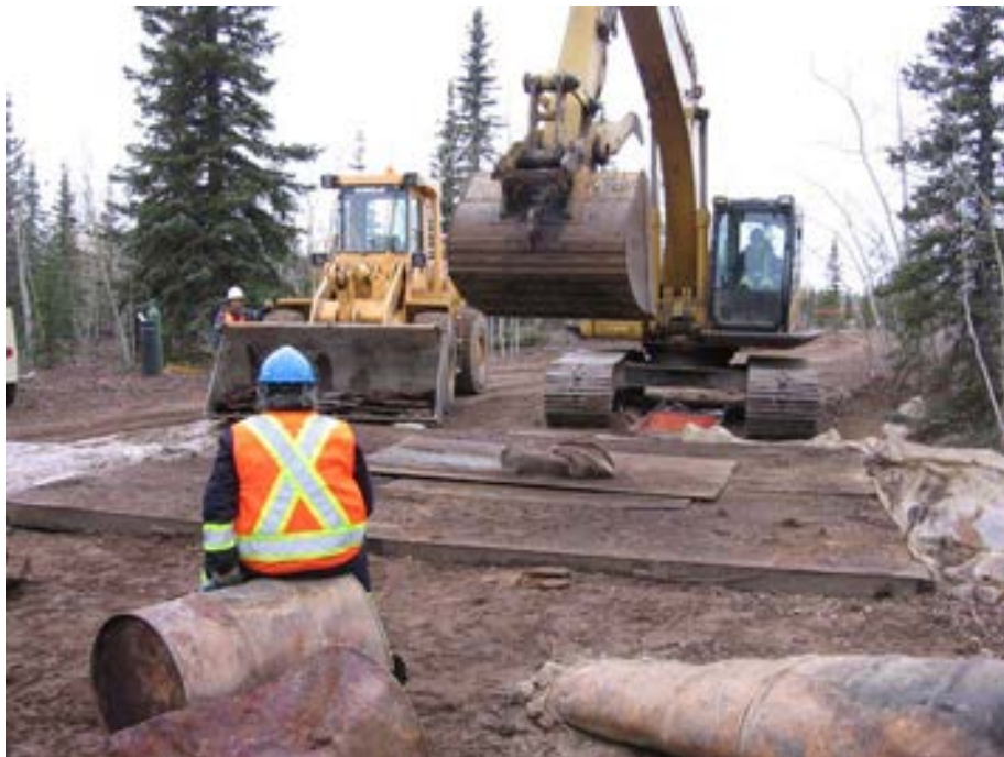
Drum crushing
