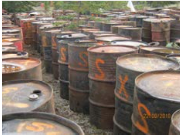
Categorizing Barrels. Note barrels placed in rows of 2 wide to allow for inspection and sampling if nec.
