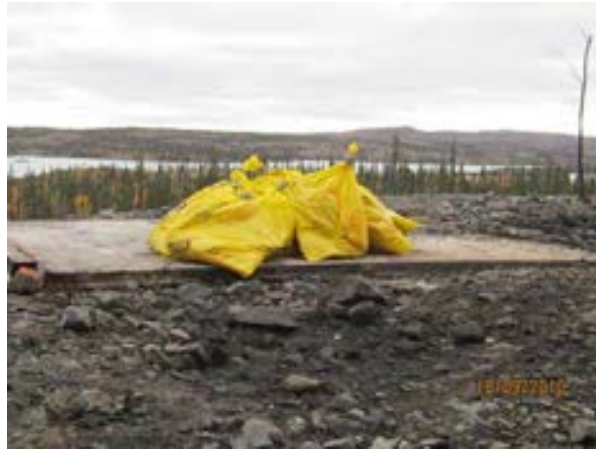
Double-bagged Asbestos containing material
