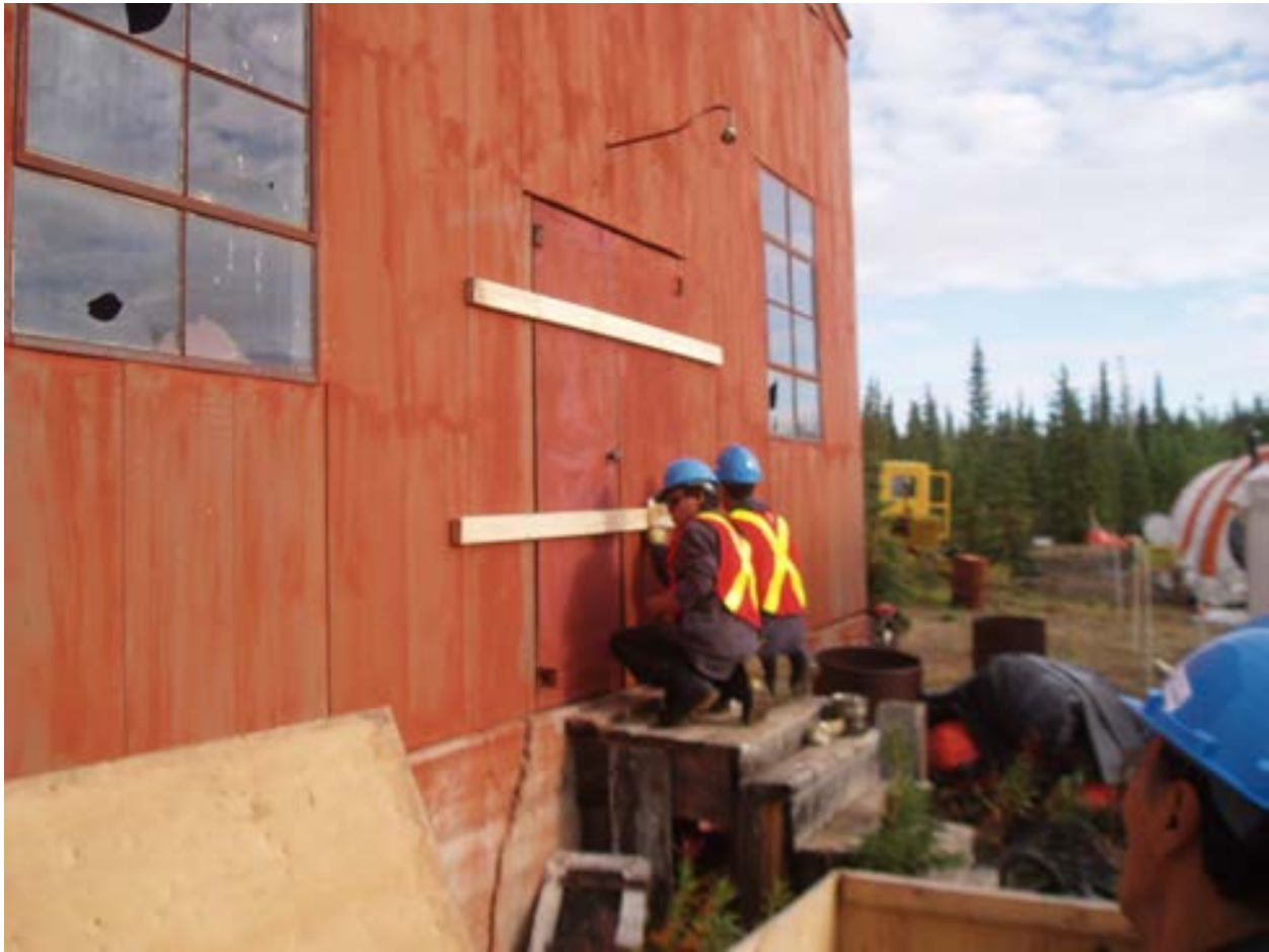
Closure of the main door of the Power House, the door is also latched on the inside. The two doors at the north side are sealed in the same fashion.
