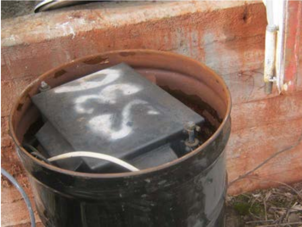
Photo 55: Transformer with PCB containing oil, from inside Power House, Sawmill Bay. Transformer removed and packed in steel drum for transportation to Yellowknife ↑
