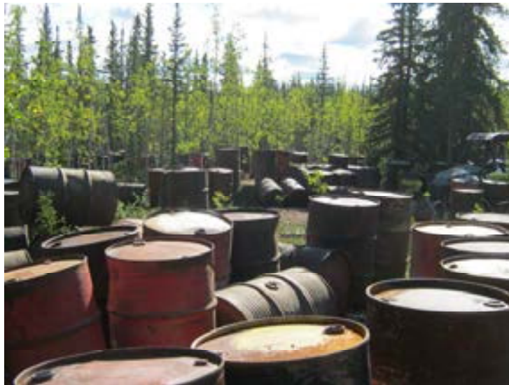
Hauled barrels in rows to allow for inspection
