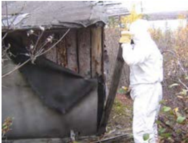
Cabin 5 asbestos abatement prior to demolition.
