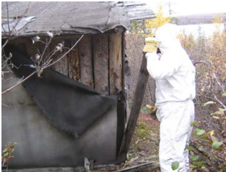
Photo 4: Cabin 5 asbestos abatement prior to demolition, Contact Lake ↑
