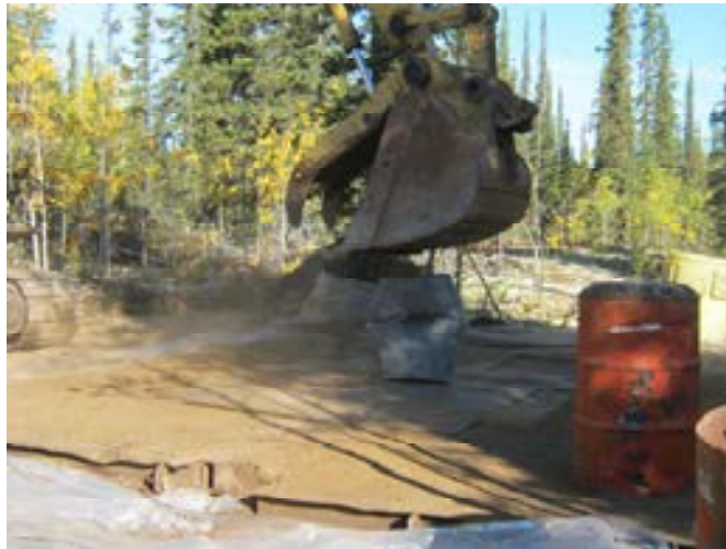
Crushing barrel
