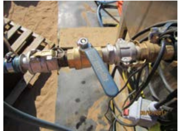
Photograph No. 38: Flow from oil-water separator to polishing unit restricted by valve.
