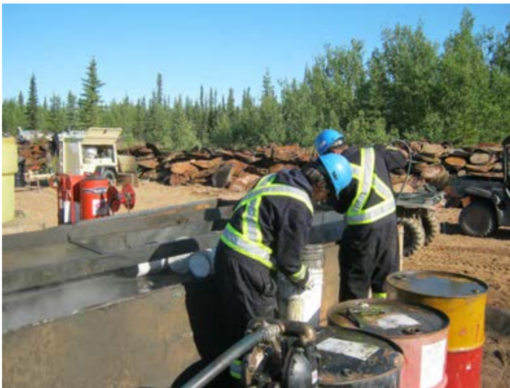
Cleaning and disassembling the barrel wash station.
