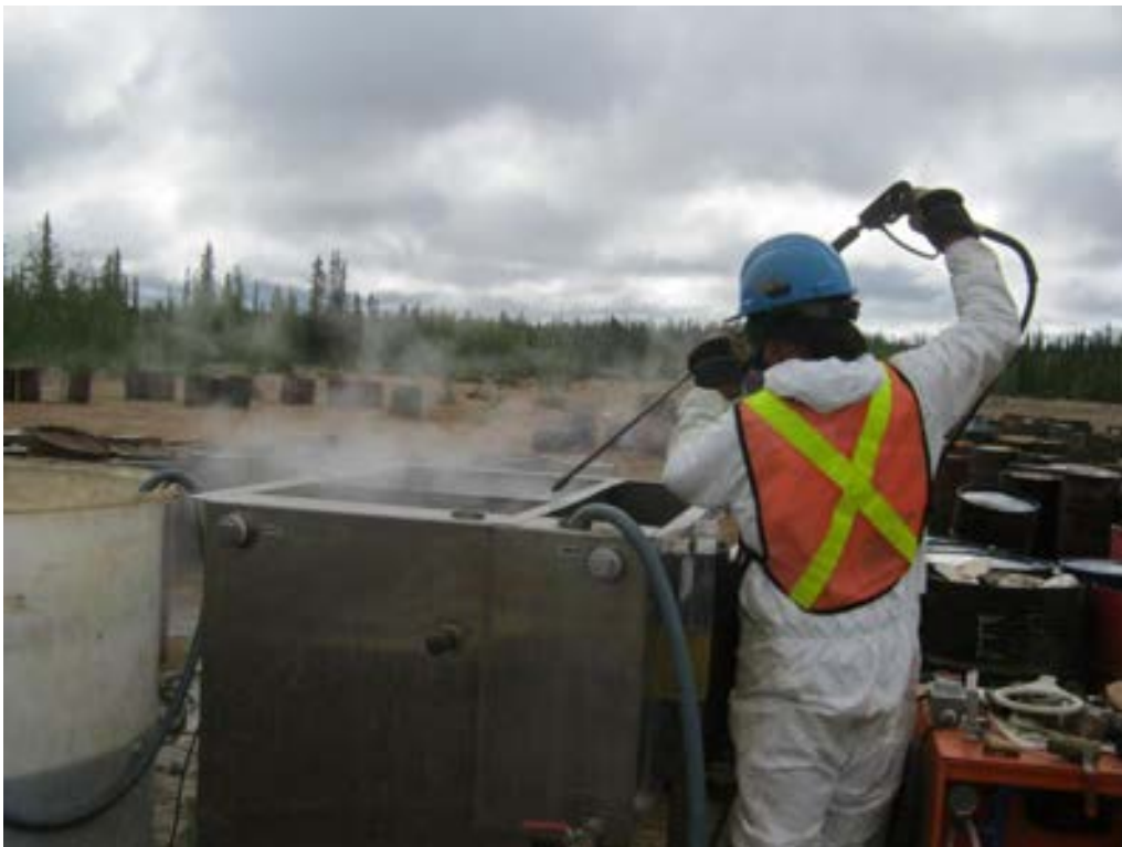
Cleaning out the oil/water separator.
