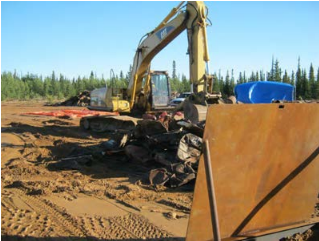
Crushing drums.
