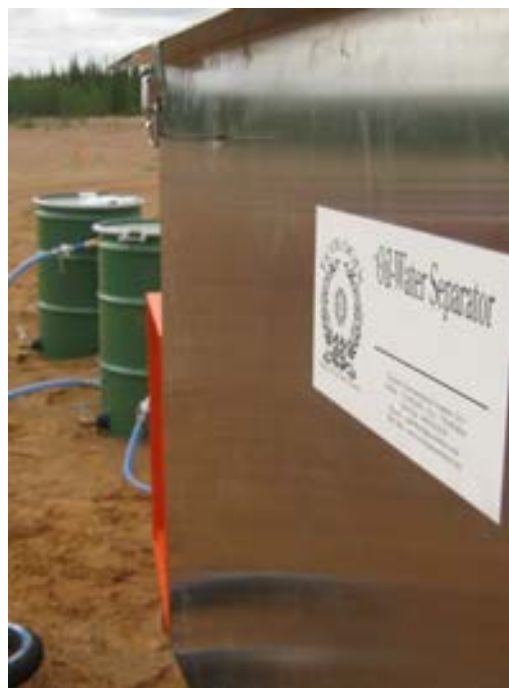
Putting the pieces together of the water treatment system. Note the oil water separator in the foreground. Also note that these will be assembled on the liner inside the bermed area when in operation.
