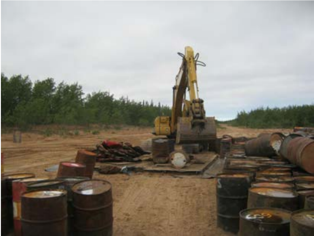
Crushing drums with the excavator. The 6'x6' safety shield is to the left of the frame. There are no labourers aiding the excavator.
