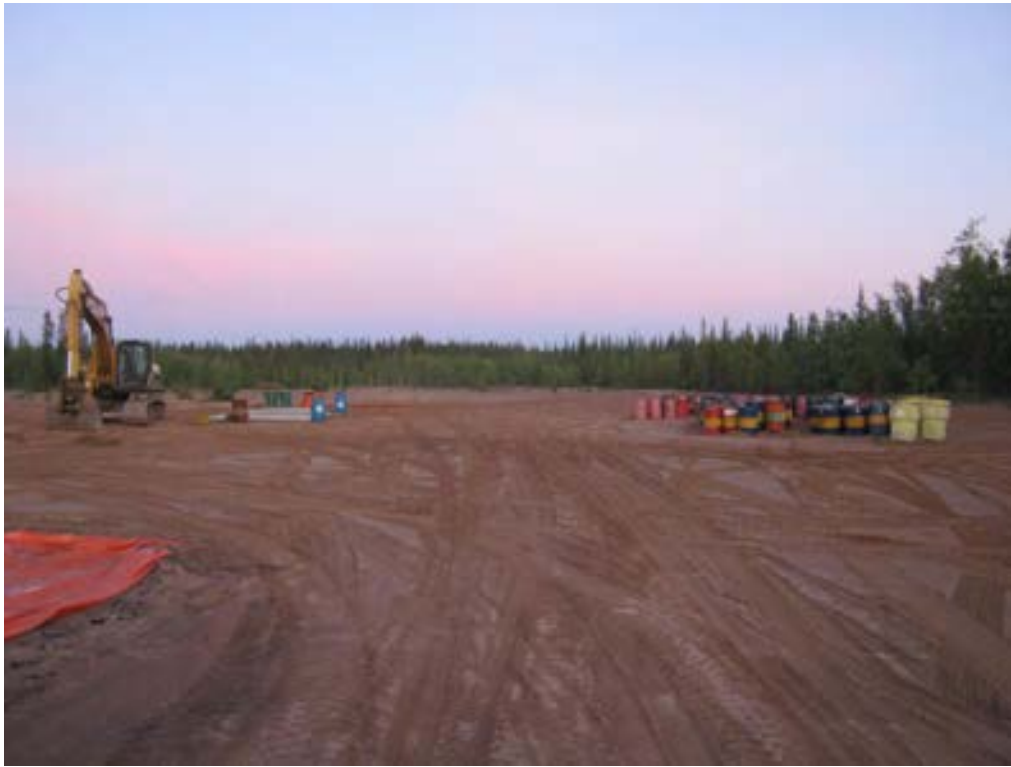
The site of the former airstrip drum cache. Barrels to the right of the frame are consolidated product and process waste. To the left of the frame, the bladders will be discharged and removed once results below applicable standards and approval have been received.
