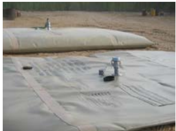
Photograph No. 24: Grey holding bladders which store treated water prior to discharge.
