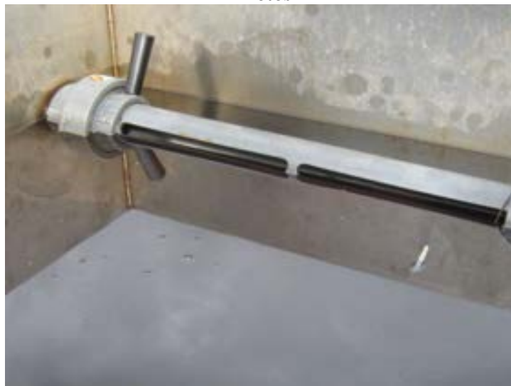
Oil being skimmed off the top in the oil-water separator.
