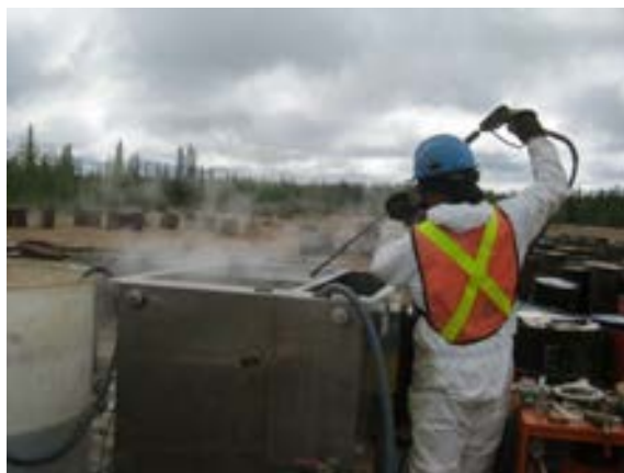
Photograph No. 54: Cleaning the o-w separator
