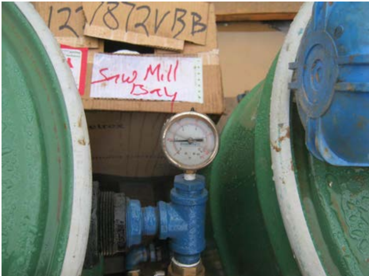
Treatment system in use. System pressure is roughly 3 psi.
