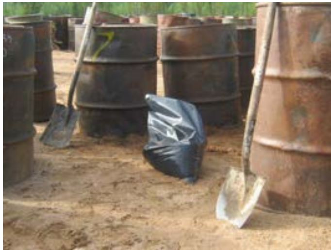
Sand shovelled into poly bag from a 0.15 L spill of watery oil
