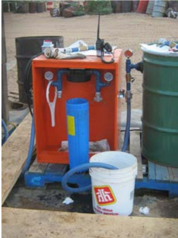
Changing out the sediment filter housed in the blue cylinder.
