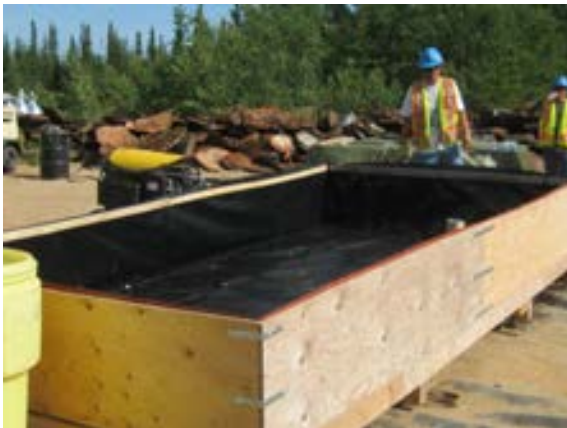
Photograph No. 17: Drum wash station construction.
