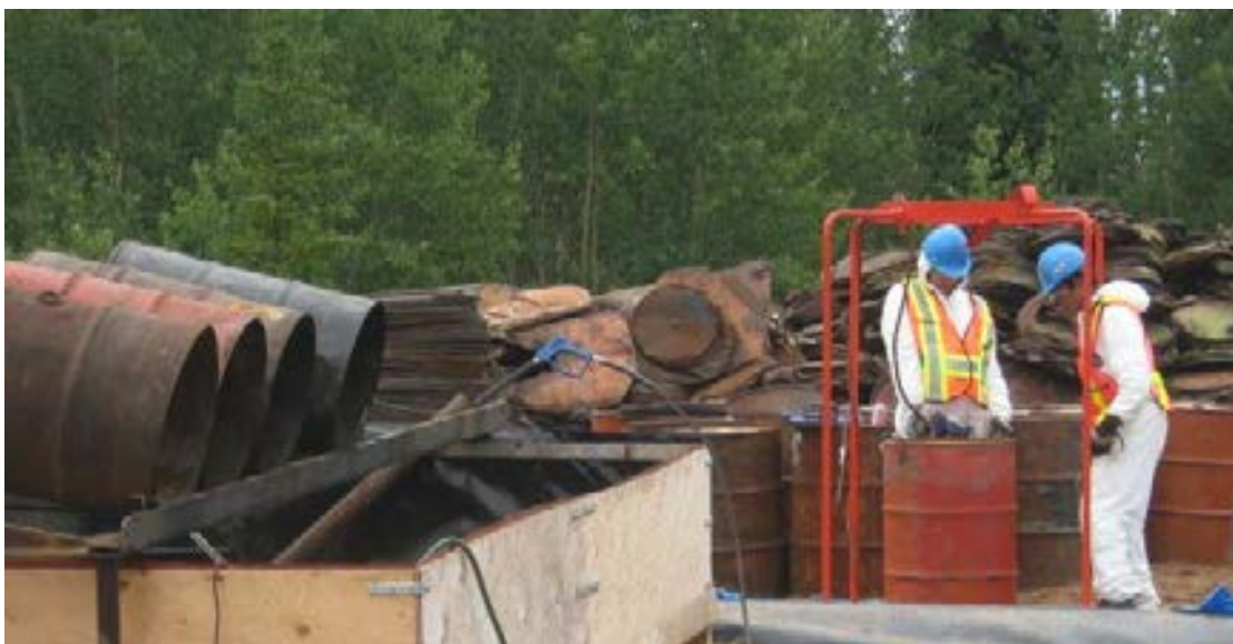
Drum deheading adjacent to the drum wash.
