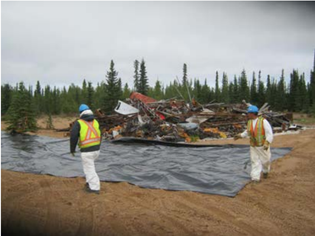
Spreading out plastic under the location of the new crushed drum stockpile.
