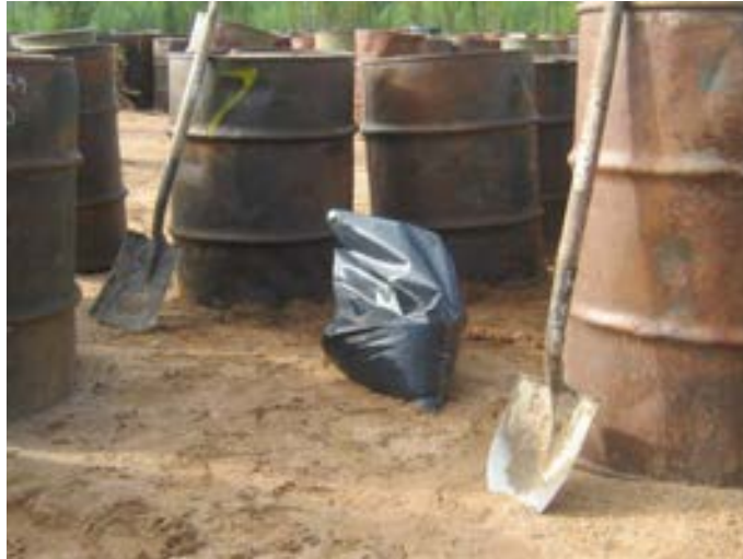
Minor spill of old diesel, the impacted sand was shovelled into poly bags
