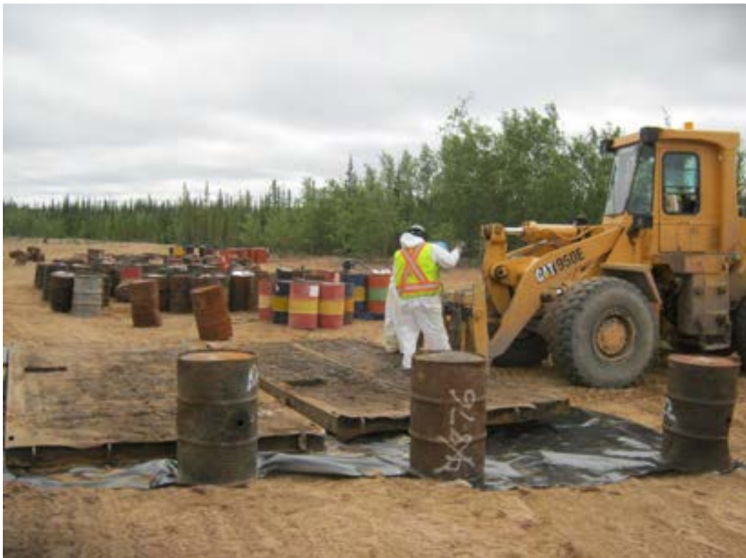
Moving the crushing pad to the airstrip. Note the plastic liner under the pad.
