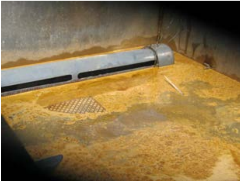
Liquid inside the oil water separator. The grey tube collects surficial oil.
