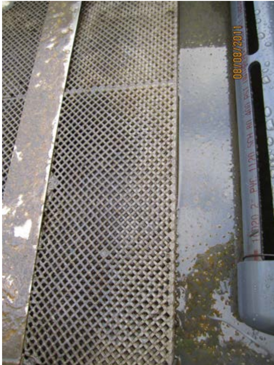
The honey comb structure of the oil-water separator. Note the beads of oil.
