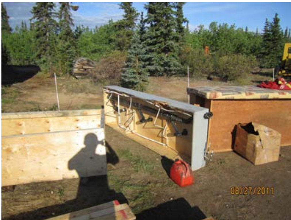
Disassembled plumbing from the shower stalls.
