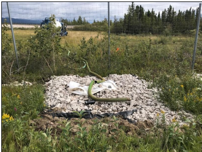
Photo 12: Discharge of sump water on pad. August 8, 2019
