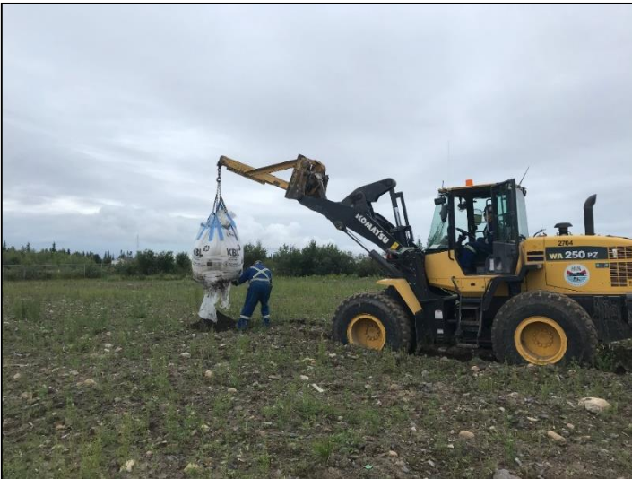
Photo 10: Emptying of compliant soil bags. August 8, 2019
