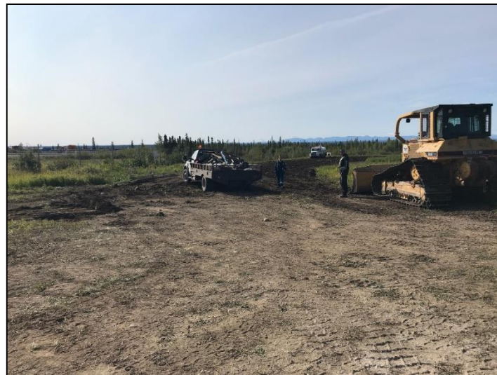
Photo 13: Spreading of bagged soil along east side of LTU. August 8, 2019
