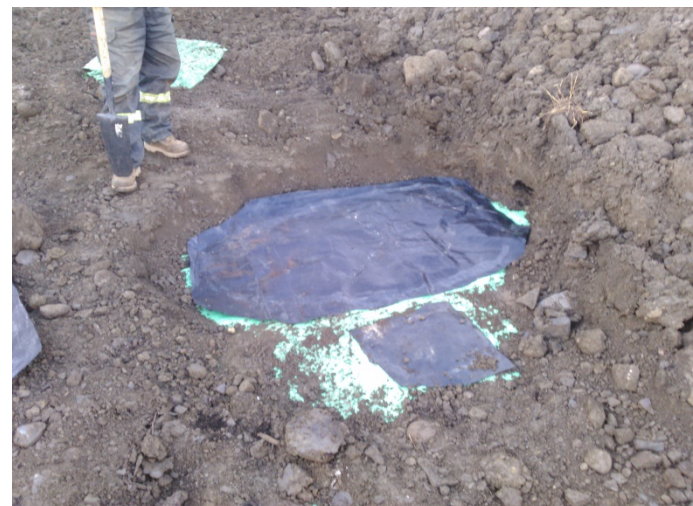
Photo 12: Completed liner repair, October 2017
