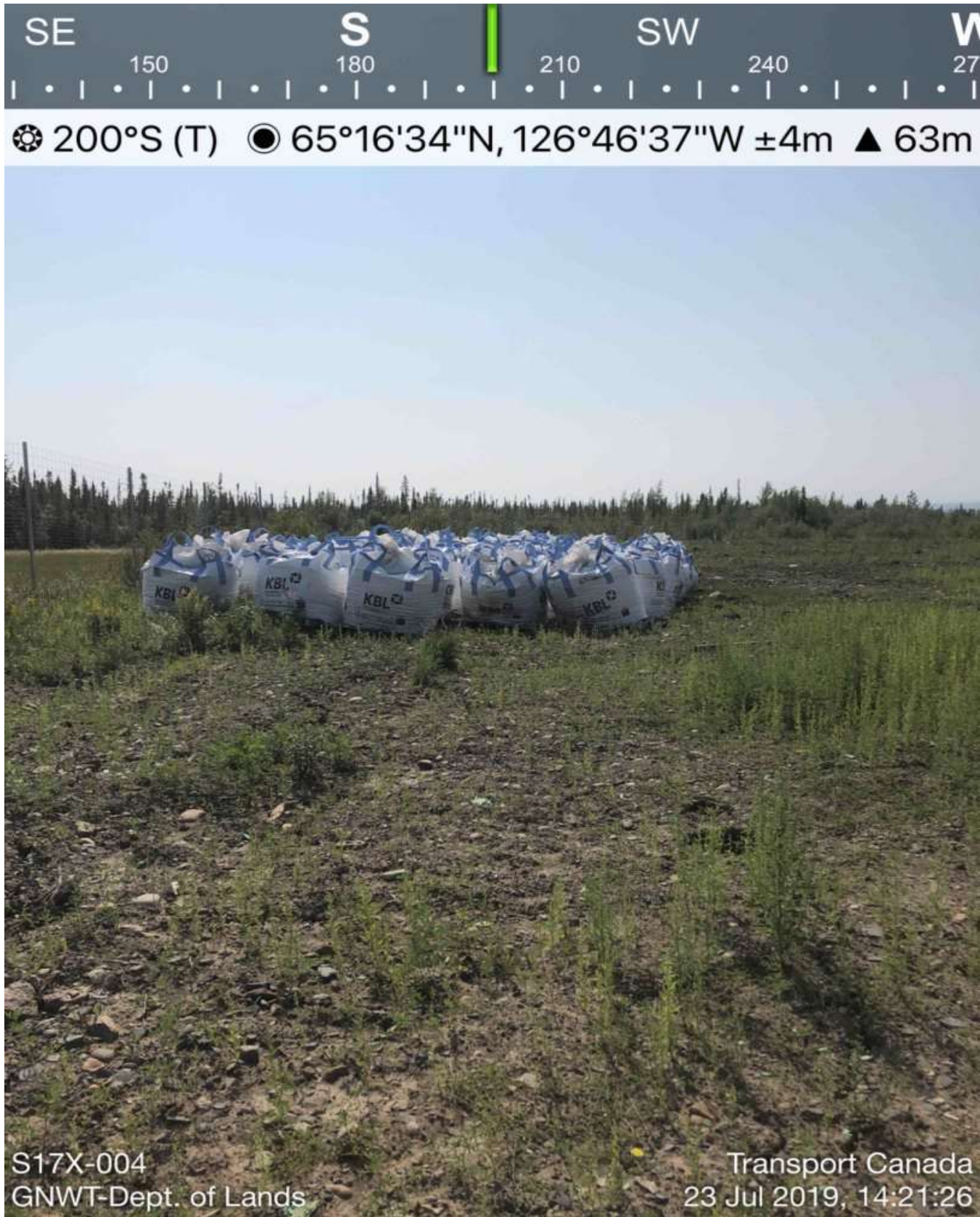
Figure 2 Contaminated soil in lined heli-sacks (48).
