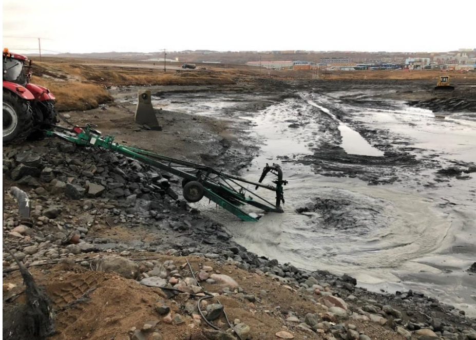
Figure 2.3: City of Iqaluit Lagoon Sludge Management: Sludge Pumping
