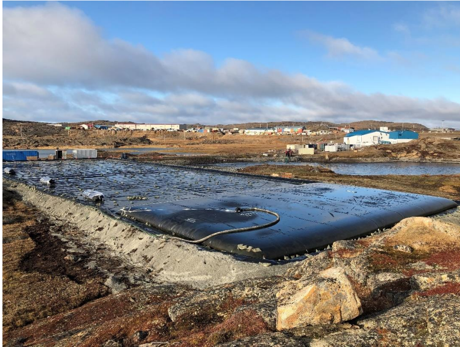
Figure 2.2: City of Iqaluit Lagoon Sludge Management: Geotubes Being Filled
