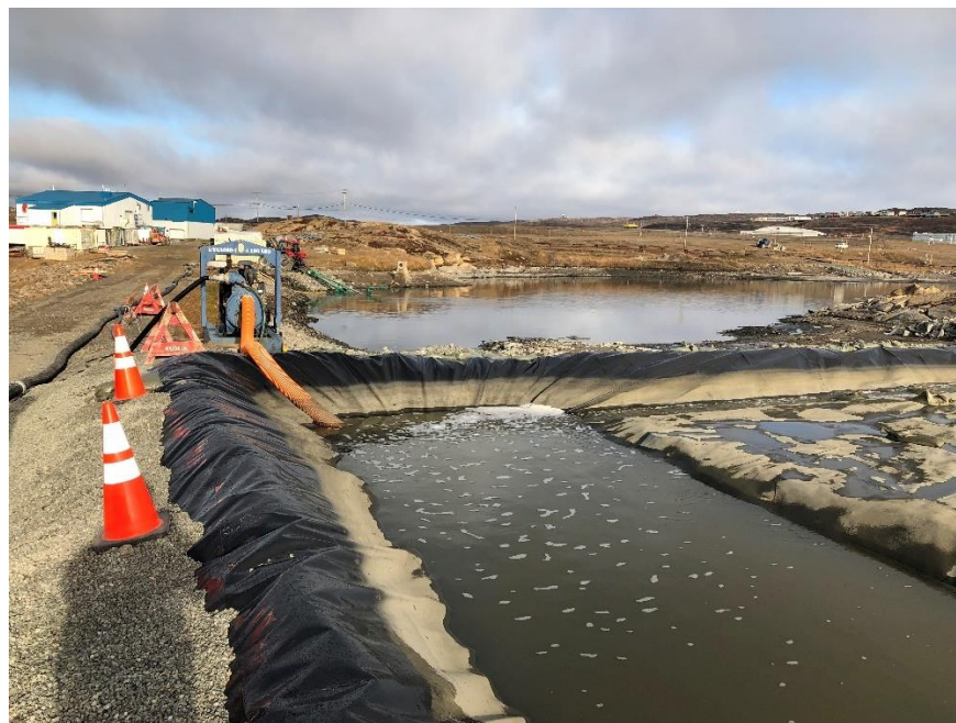
Figure 2.4: City of Iqaluit Lagoon Sludge Management: Filtrate Collection
