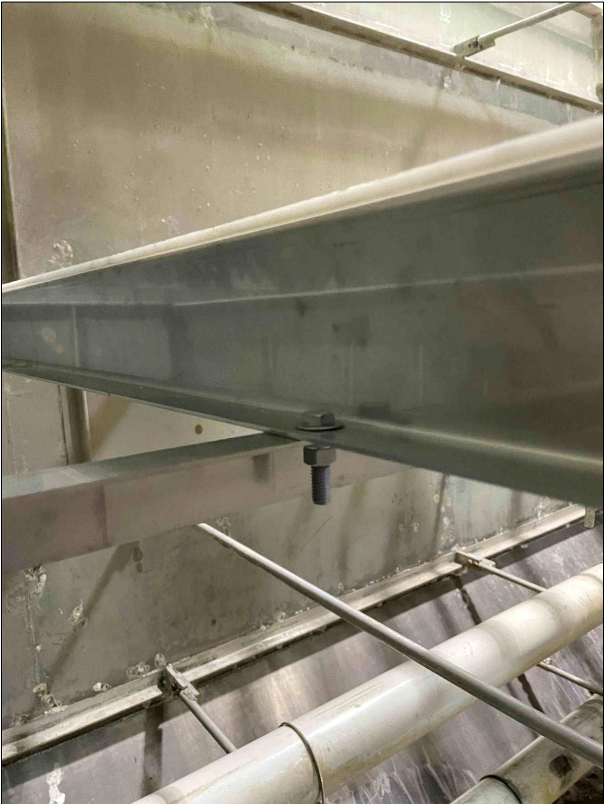
New Support Beam Installation
