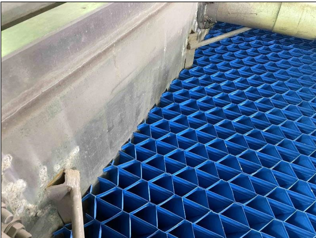
Front Angled Lamella Module Section Installed
