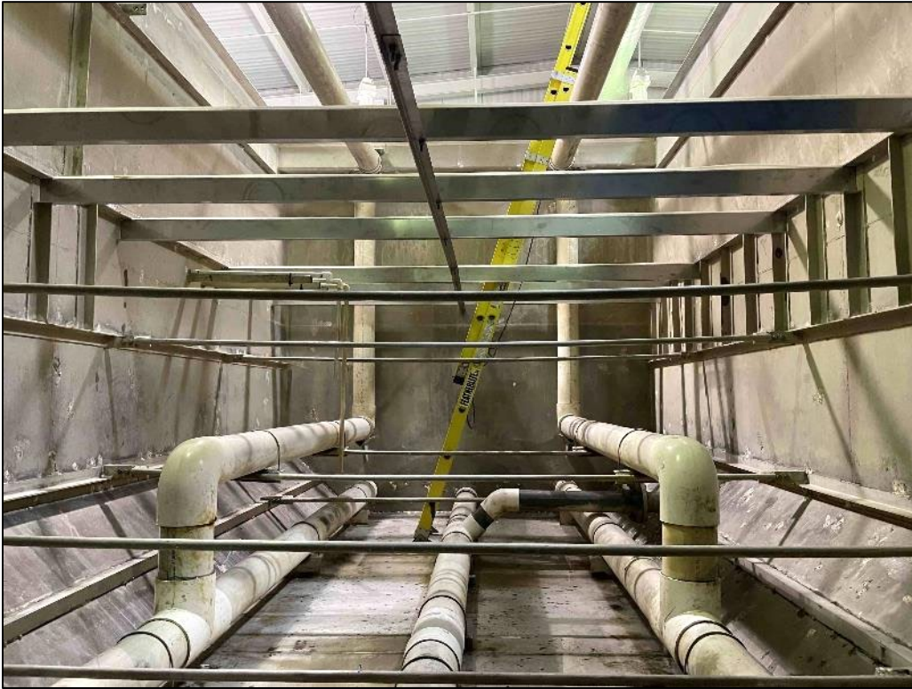
Support Beam Installation Completed
