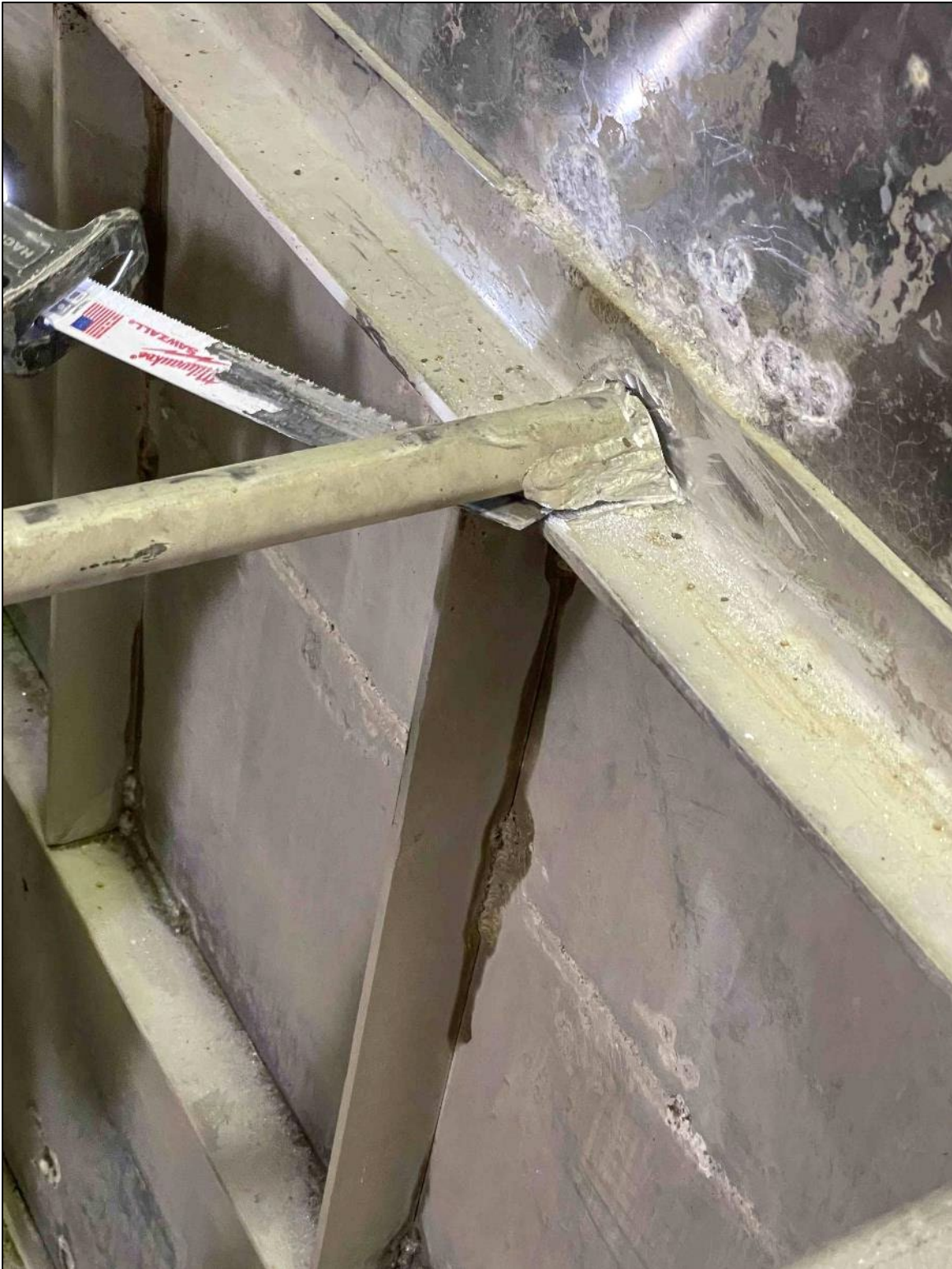
Existing Support Beam Removal
