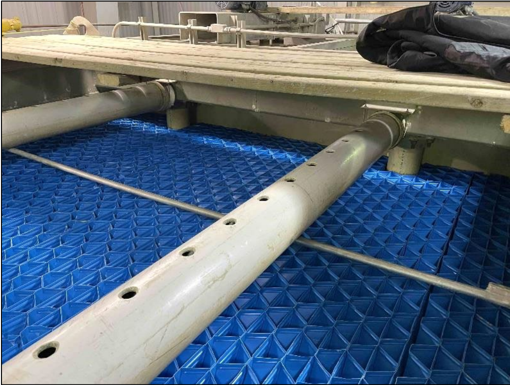
Back End of Lamella Modules Installed
