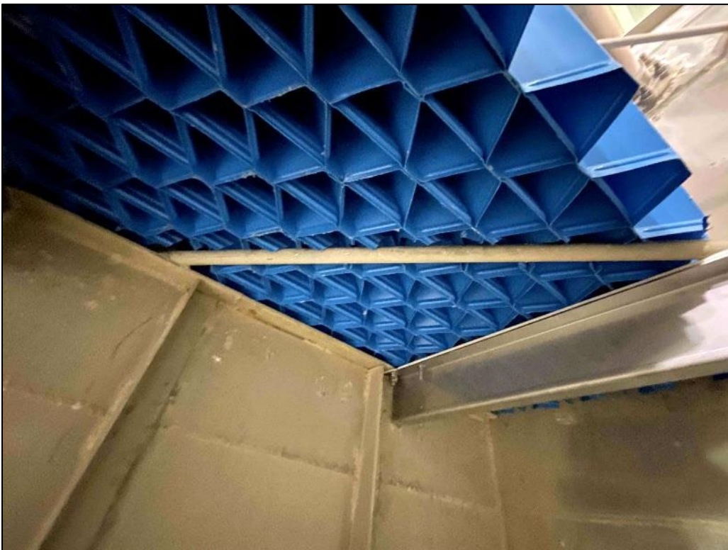
Front Side Lamella Module Installation
