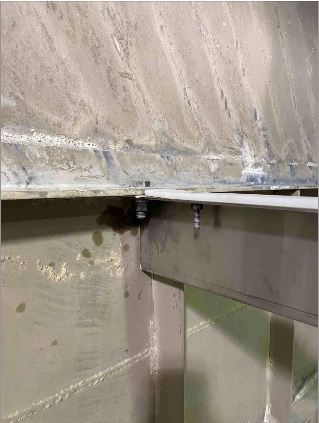
New Support Beam Installation
