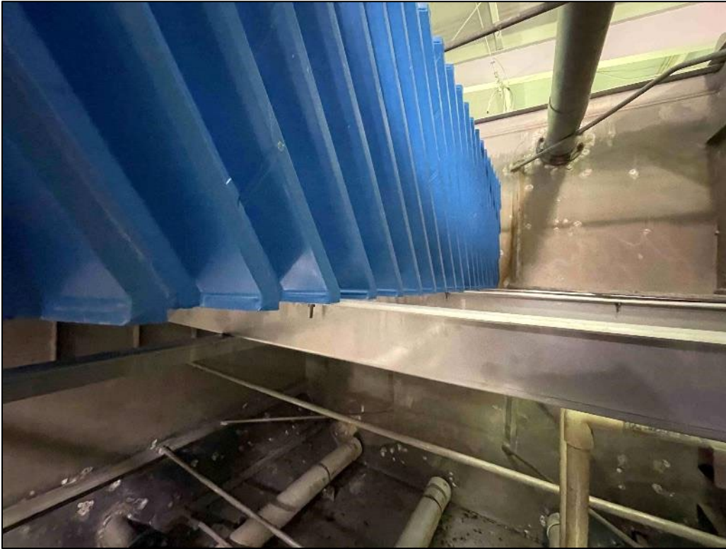
Lamella Module Installation
