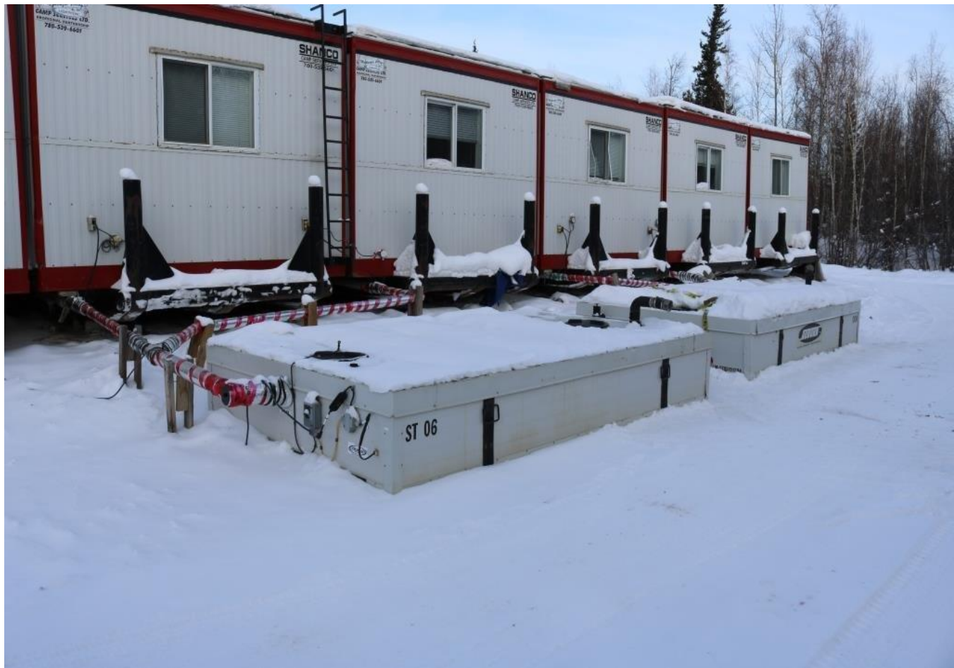
Figure 14 Fuel tank with drip trays, no spill kit- Camp
