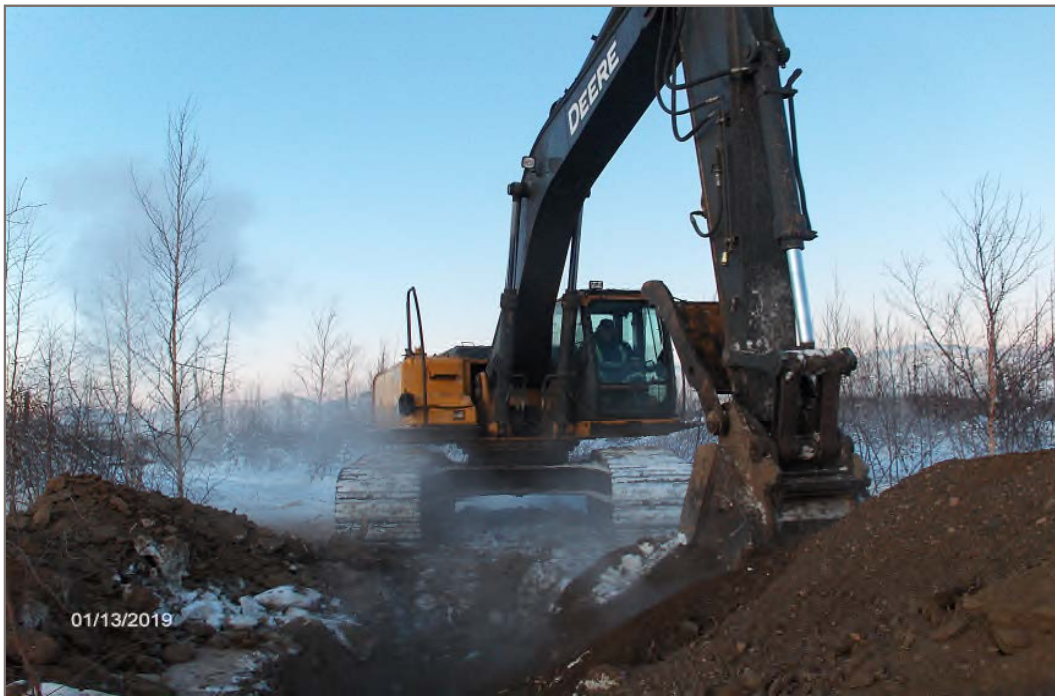
Photo 4: John Deere 270D LC excavator used for testpitting.
