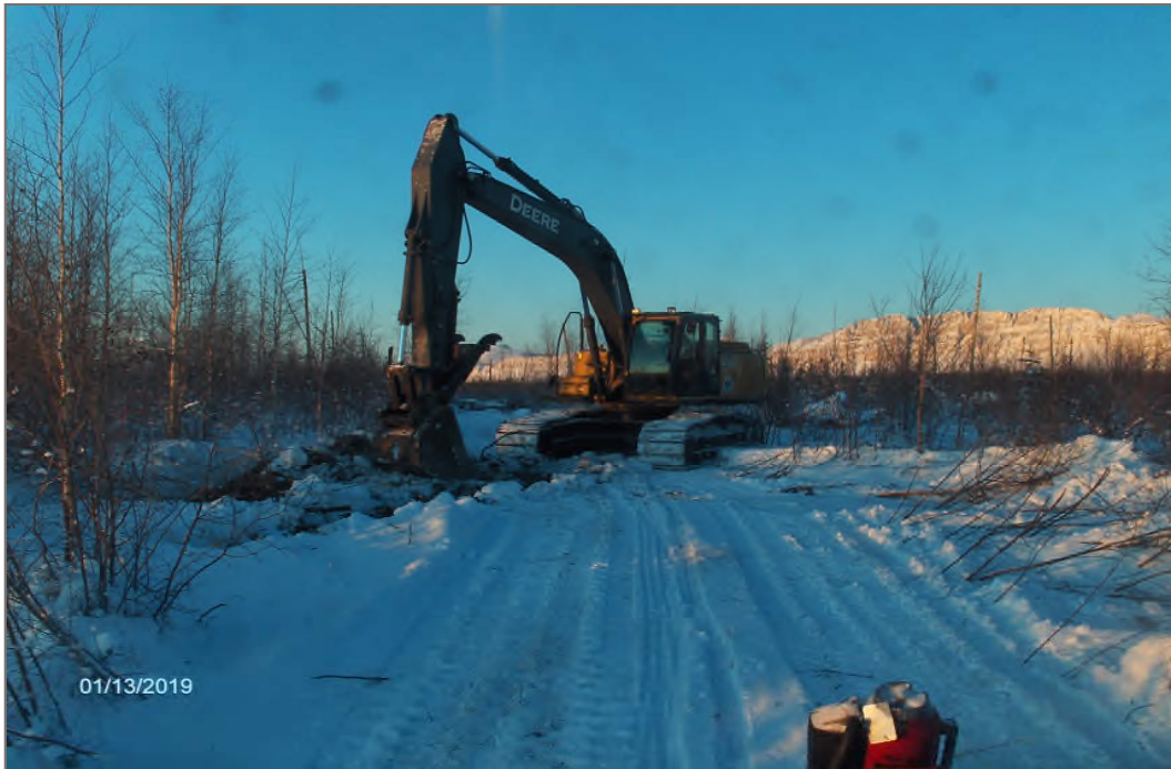
Photo 3: Excavating Testpit 6 at Prospect 1.
