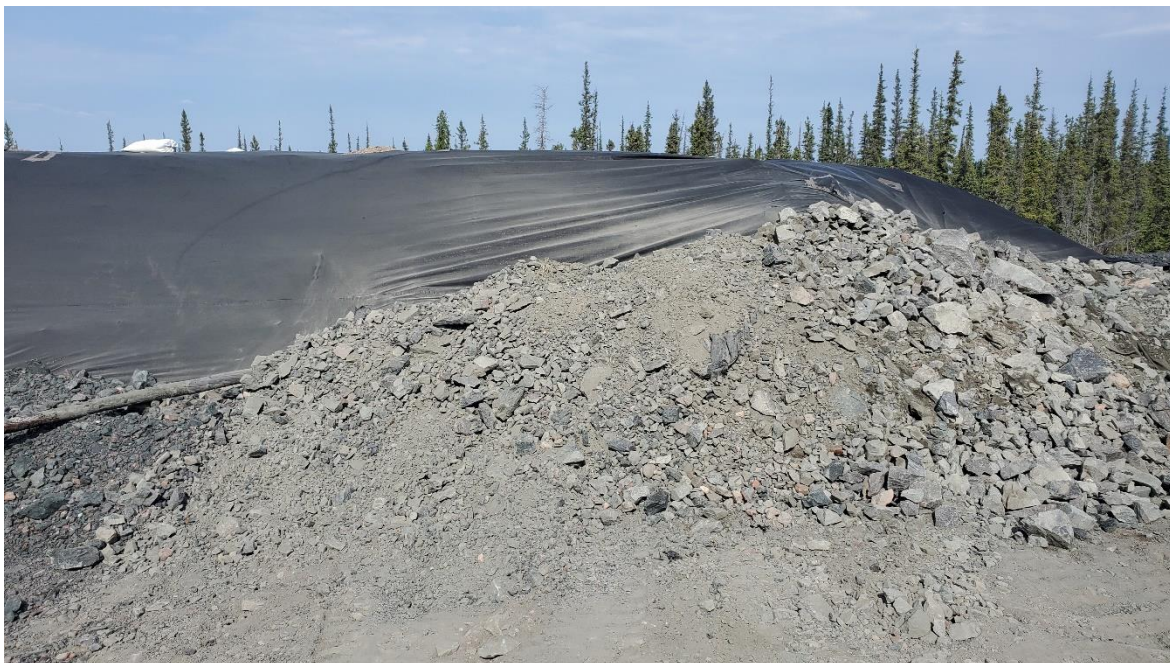
Photo 2 Repaired tear in the ore pile cover
