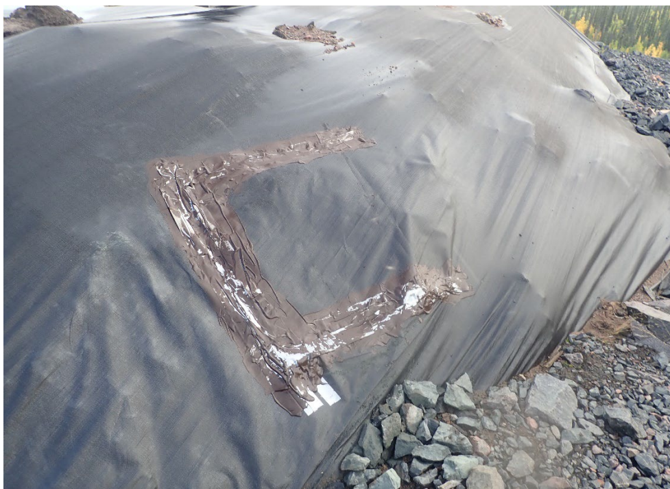
PHOTO 4 Ore sample collection hole repair
