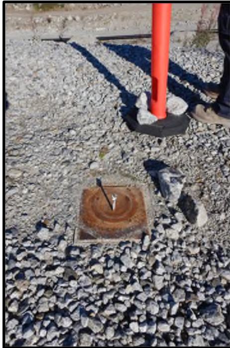
Photo D39: Blast vibration monitoring geophone mounting plate installed along the downstream crest.
