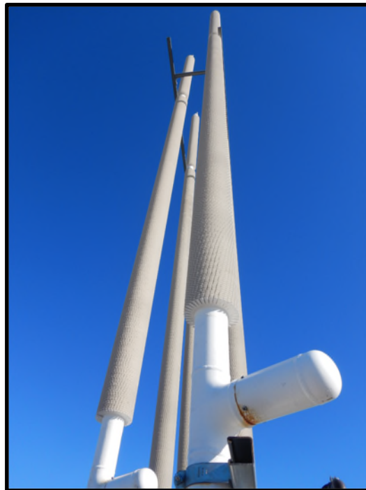
Photo D12: General view of thermosyphon radiators.
