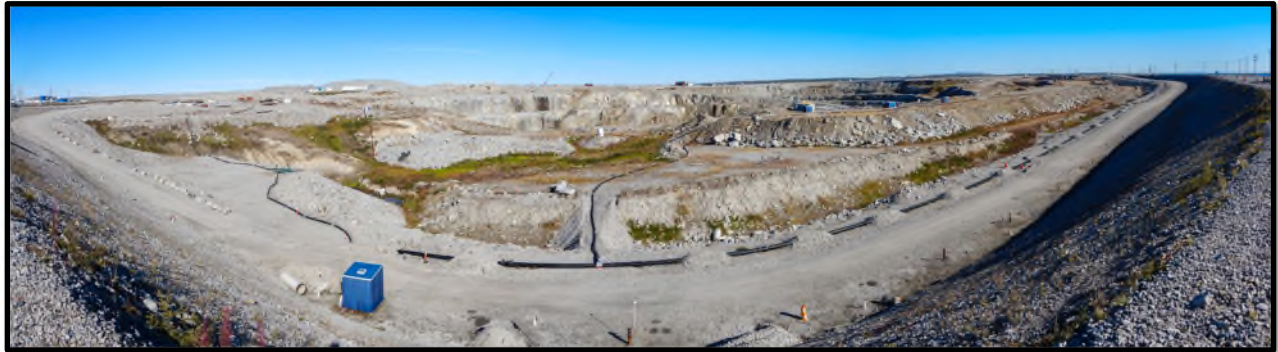
Photo D7: General view of the DPS-6 infield area from the downstream crest of the A418 Dike near Station 0+800.
