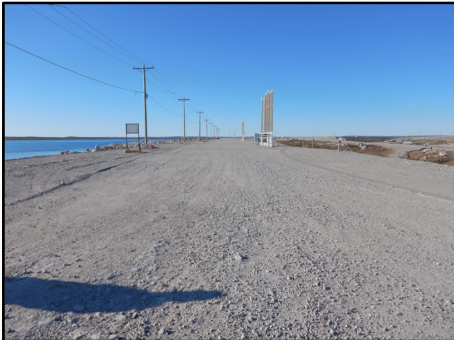
Photo D2: North Abutment top of dike near Station 0+000, looking south.
