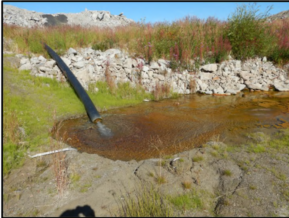
Photo D15: Redirected water from one depressurization well being discharged into DPS-6 intake pond.
