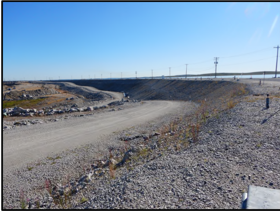
Photo D5: South Abutment downstream slope near Station 1+000, looking east.
