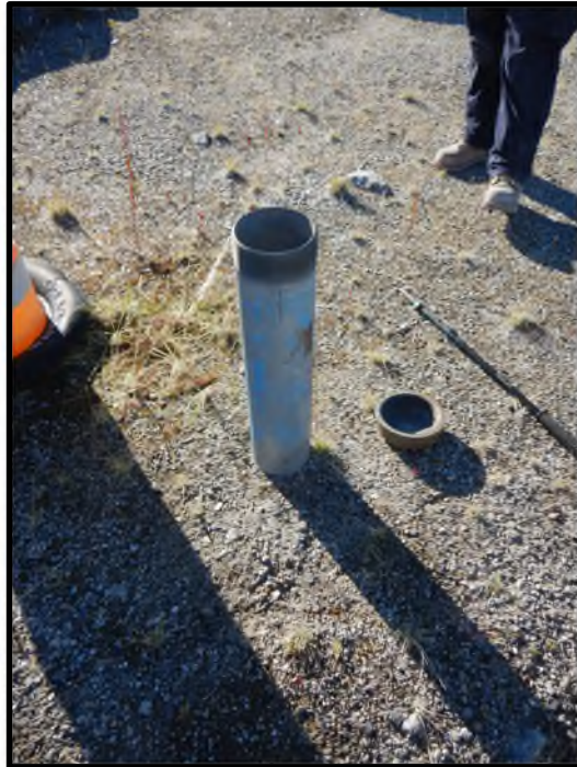
Photo D35: Protective casing for a survey monument.
