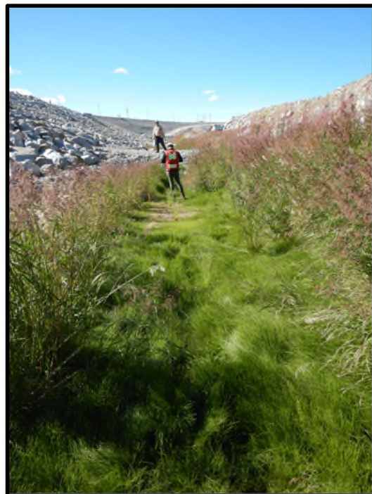
Photo D24: Downstream toe ditch near Station 0+550 showing abundant vegetation.
