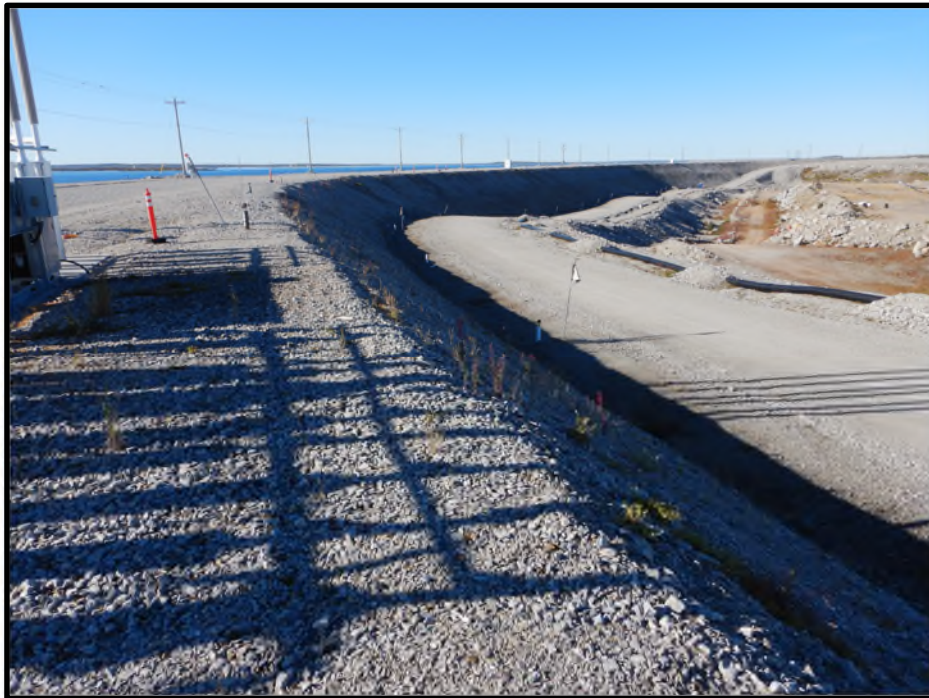
Photo D6: Downstream slope near Station 0+350, looking south.
