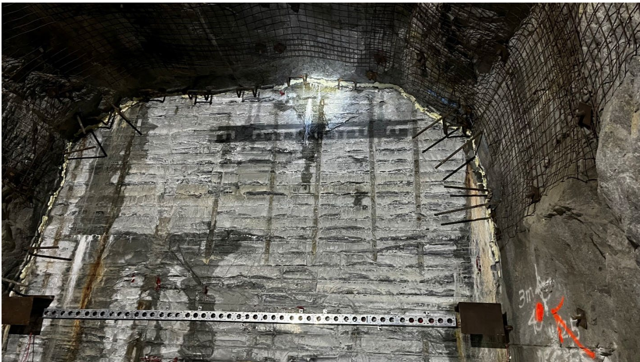
Photo 6: 9130 Bulkhead – Note the face is primarily dry with only small damp areas.
