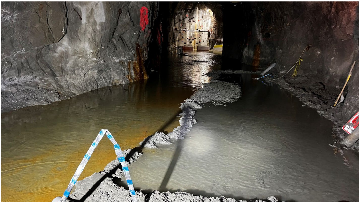
Photo 2: Ponding water at the 9080 Bulkhead
