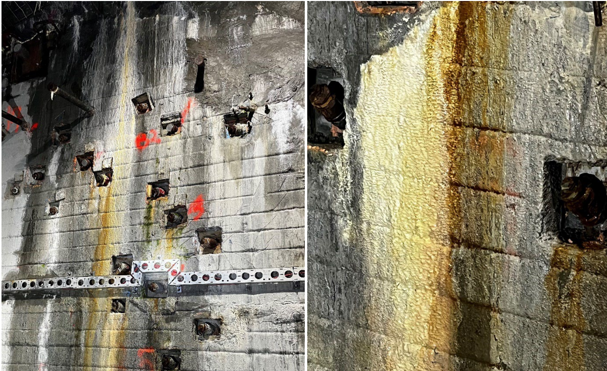
Photo 5: Precipitate on Face of 9080 Bulkhead (left). Close up of precipitate originating from fracture in bulkhead face (right).
