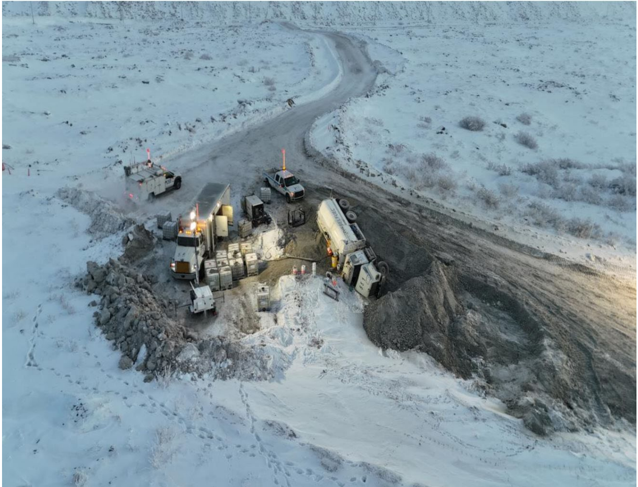
Figure 4: Aerial image of fuel pump-off operations and decanted totes of fuel.
