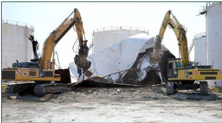
Demolition, landfill and hazardous waste removal
