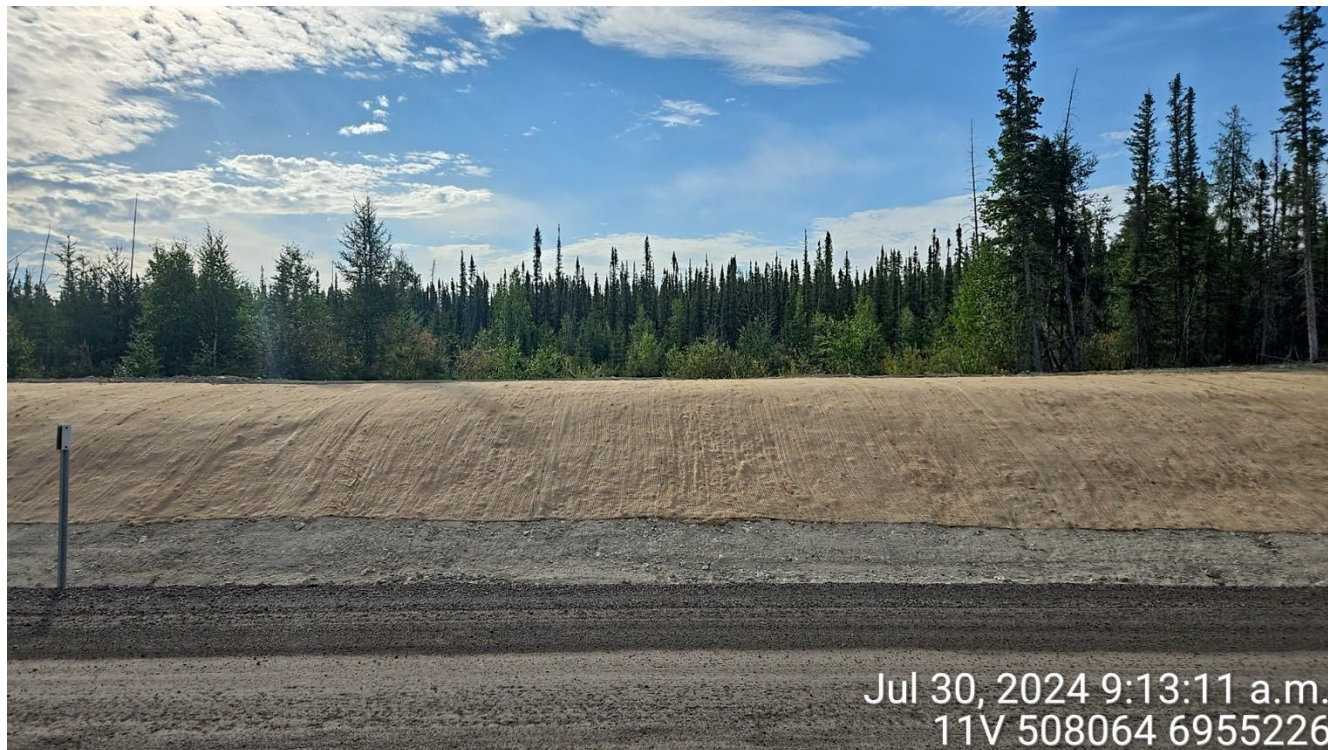
Figure 4-2: Looking east at the erosion control matting installation on the east side south approach at ~Sta40+078.
