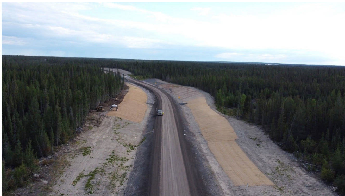
Figure 4-3: Drone image looking north at the progression of erosion control matting installation on the, south approach to Duport River.
