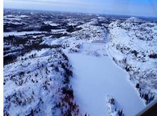
Photo #14: Overview of Mill Lake, the CDF, and the Mill Lake water treatment facility.
