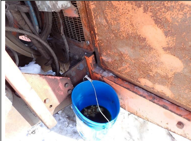
Photo #11: Oily water stored behind the drill that will need to be appropriately disposed of.
