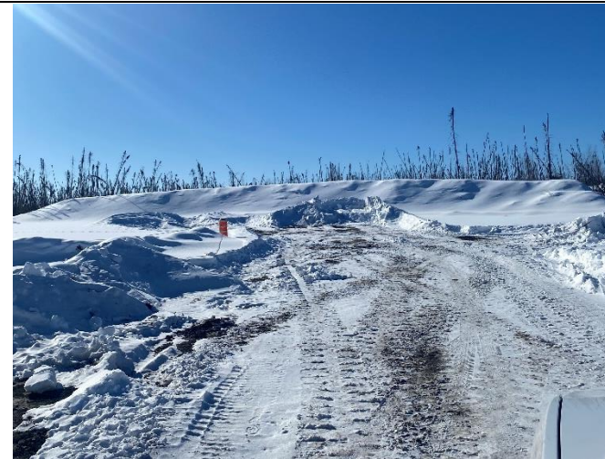
Photo #15: Drill removed from site. Photo provided by Sanexen.
