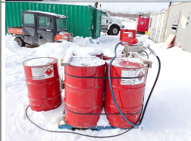
Photo #8: Fuel drums near the camp facilities not stored in proper secondary containment.
