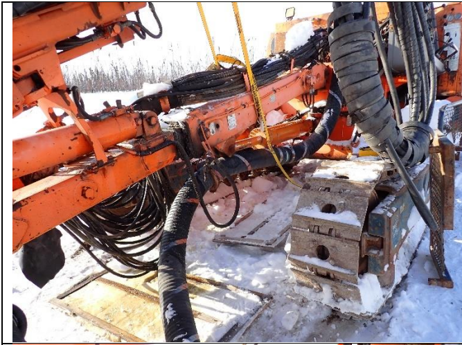
Photo #9: A saturated drip tray under drilling machinery that needs to be replaced.
