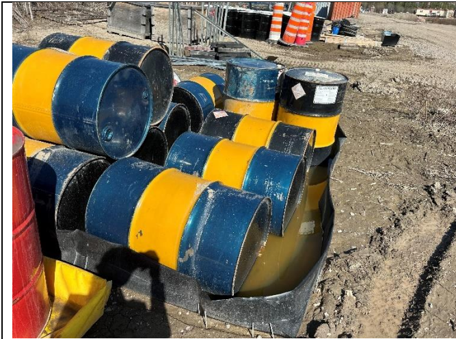
Photo #13: Water in the secondary containment berms needs to be drained and appropriately disposed of for the berms to effectively function as secondary containment.
