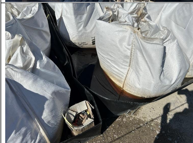
Photo #12: Water in a secondary containment berm containing the megabag waste bags. This water will need to be drained and appropriately disposed to ensure the secondary containment can effectively function.
