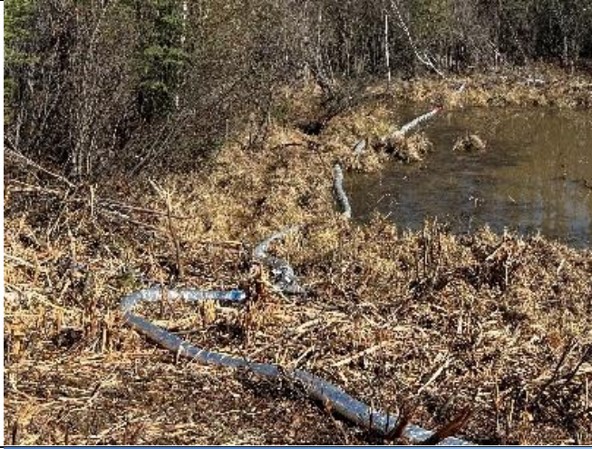
Photo #5: Portion of the camp wastewater discharge line that continues into the trees to a discharge field.
