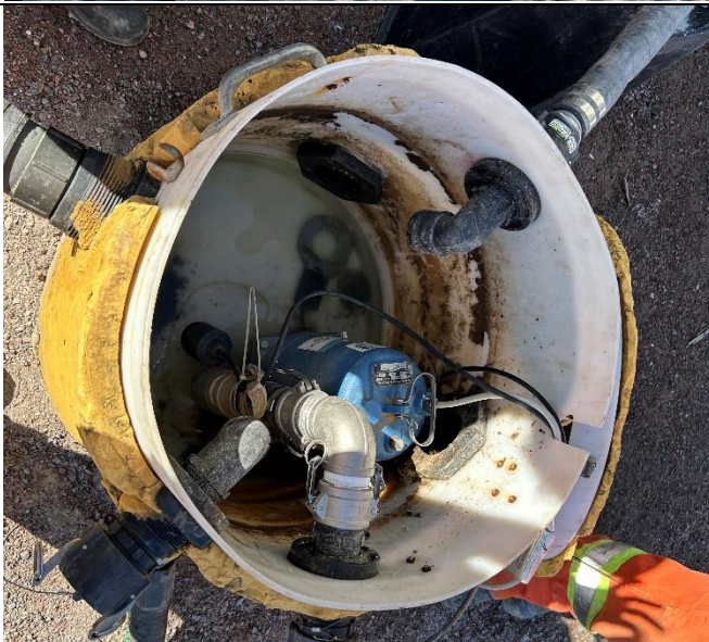
Photo #8: Water pump associated with the camp wastewater treatment plant. A curious bear has been removing the cover.
