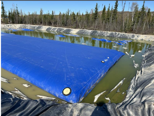
Photo #7: One of the blue bladder tanks on site within the wastewater containment structure. Water will need to be treated before being discharge this summer.
