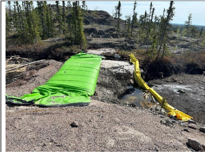
Photo #17: Aqua-dam and silt curtains adjacent to Mill Lake. Water levels are low, and these are not currently needed to hold back water from draining into Sherman Lake.
