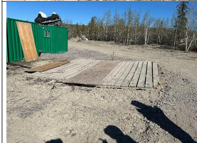
Photo #3: Grey water sump from the winter camp with boards covering it to prevent wildlife interaction.
