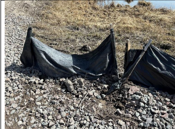
Photo #18: A silt fence near the water withdrawal point that requires repositioning.
