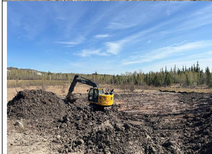
Photo #2: A tailings cover area being prepared for remediation capping near Beta Lake.
