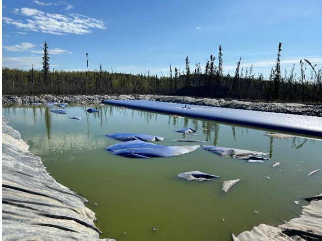
Photo #6: Overview of the wastewater containment structure, holding free water and two blue bladder tanks.
