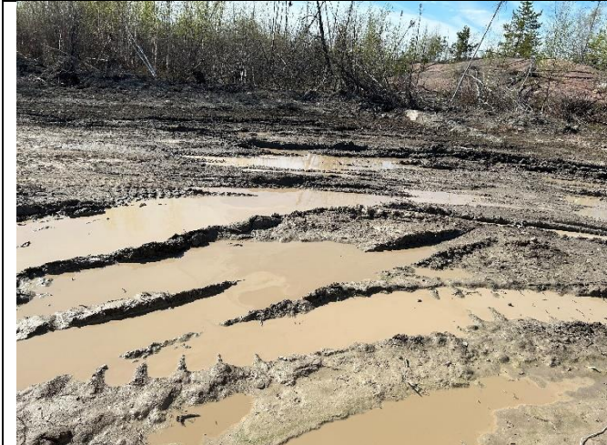
Photo #14: Minor rutting and standing water at a low-lying spot at camp.
