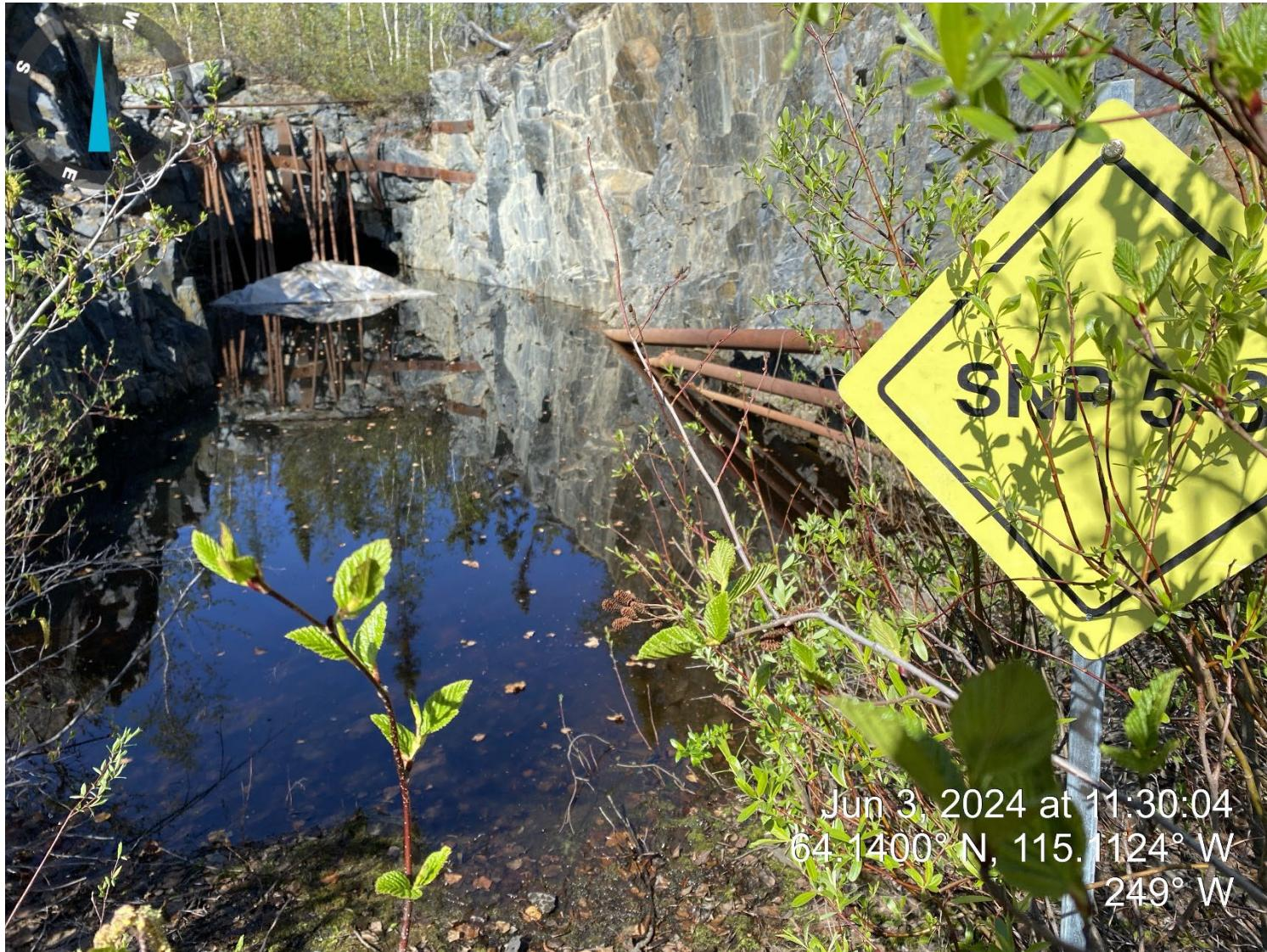
Photograph A-5: SNP 5-8, Damoti Lake Site Decline Ramp (Minewater Pooled at Entrance of Adit). Photo Orientation: West.
