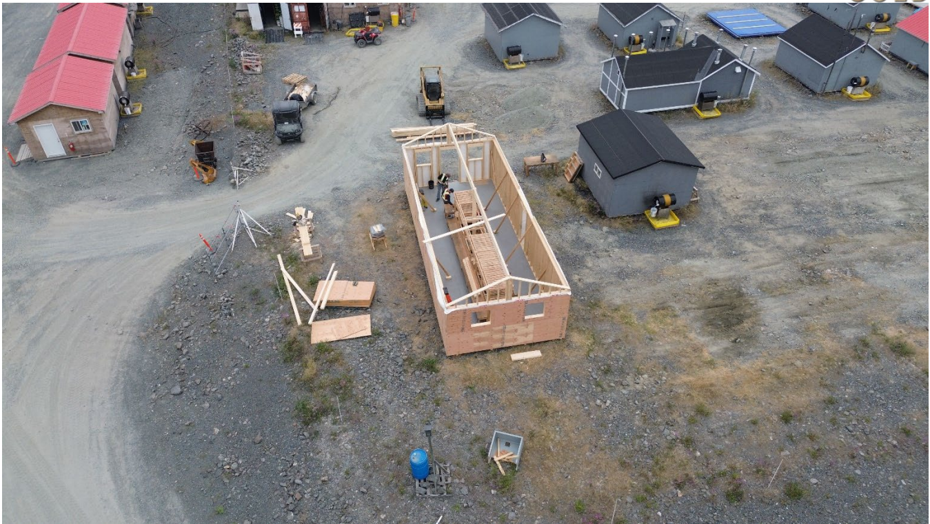
Figure 40: Aerial view of the ongoing construction of the new drillers dry (2023).
