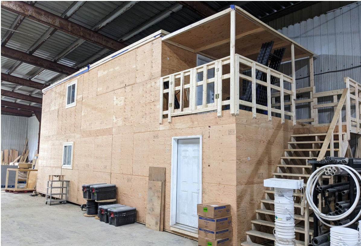
Figure 37: Two story storage building within “Big Blue” (2023).
