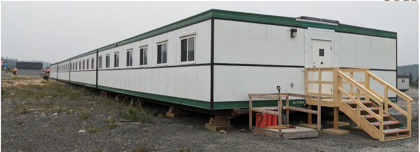
Figure 20: Outside view of dormitory trailers northern back entrance, with fire fighting equipment by the stairs (2023).
