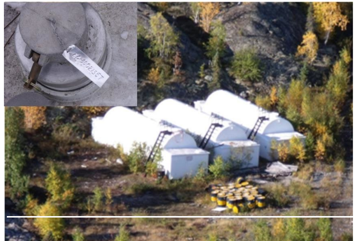
Figure 45: Aerial view of three double, 75,000 litre, bulk tanks at ramp area near Damoti camp. Inset shows metal tag with Environment Canada ID number EC-00021357.
