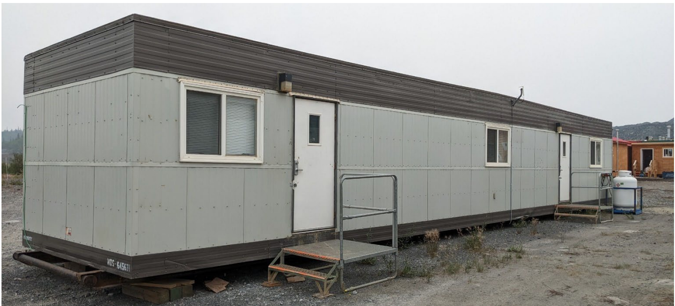
Figure 29: Outside of environmental and engineering skid mounted office trailer (2023).
