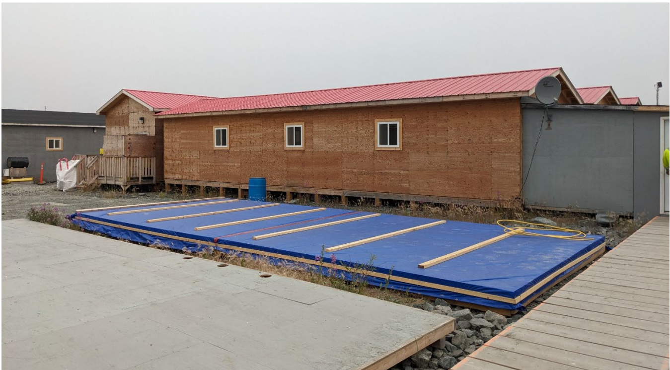
Figure 41: Photo of platform that has been insulated and wrapped up for use as a building platform in 2024 (2023).
