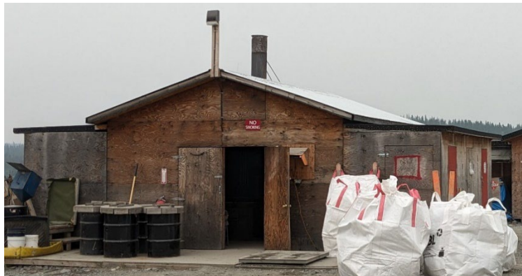
Figure 14: Outside of incinerator shack, with mega bags in front ready to be weighed before being flown out of camp (2023).
