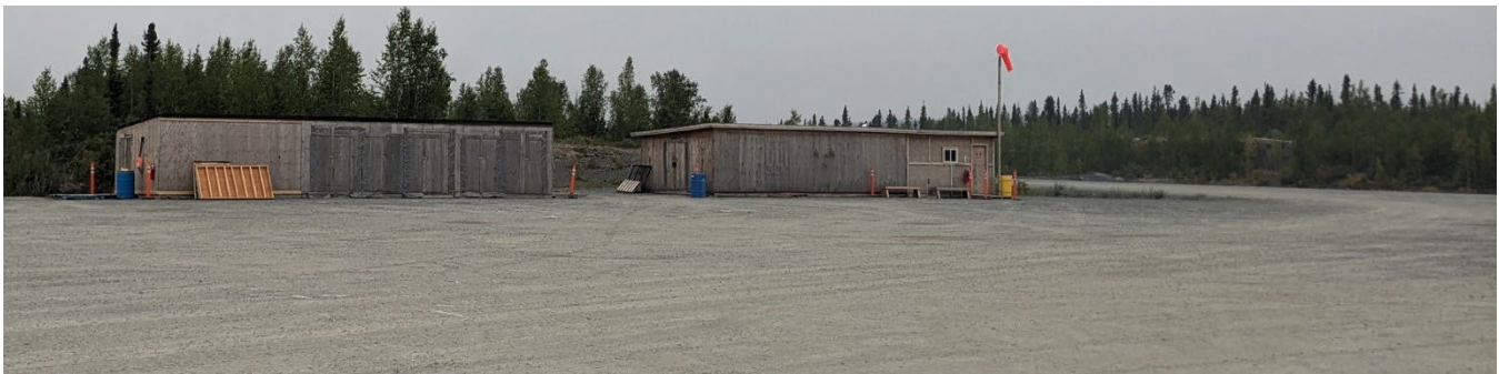
Figure 16: Colomac apron storage buildings, with Major Drilling's storage building on the left and general storage and waiting room on the right side with a windsock. Further to the right the airstrip and entrance to the apron is visible (2023).
