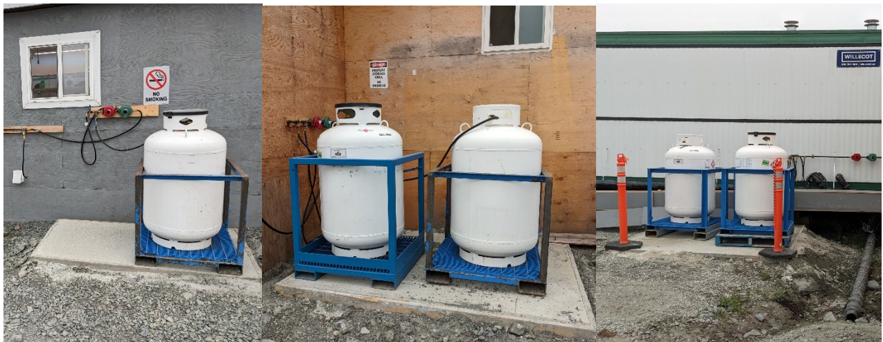
Figure 33: Concrete pads with propane pigs for the new bathhouse, the kitchen, and for the new dormitory trailer from left to right respectively (2023).
