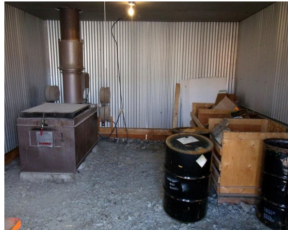
Figure 59: Incinerator building (interior) at Colomac camp. Inciner8, Model A600(sec) Incinerator on the left and bins on the right are for partitioning different types of waste based on burn rate (2014).
