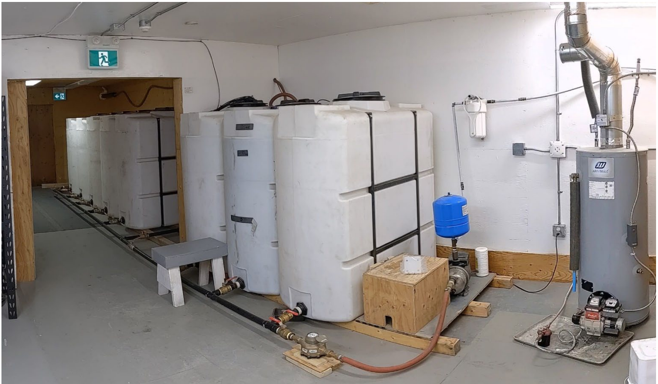
Figure 31: Inside water tank house at the back of the new washhouse (2023).
