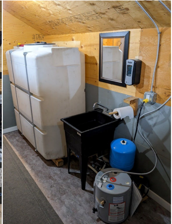
Figure 39: New sink and water tank in the old toilet facility (2023).
