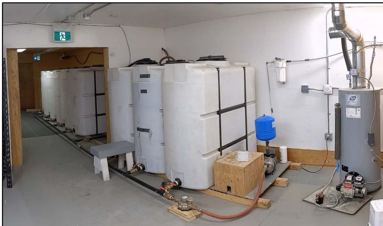
Figure 11: Main washhouse and kitchen water tanks and hot water tank (2023).
