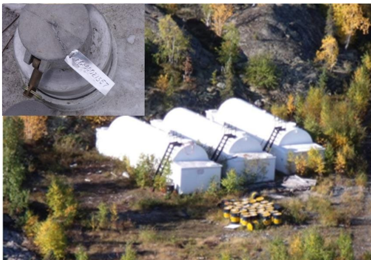
Figure 31: Aerial view of three double, 75,000 litre, bulk tanks at ramp area near Damoti camp. Inset shows metal tag with Environment Canada ID number EC-00021357.
