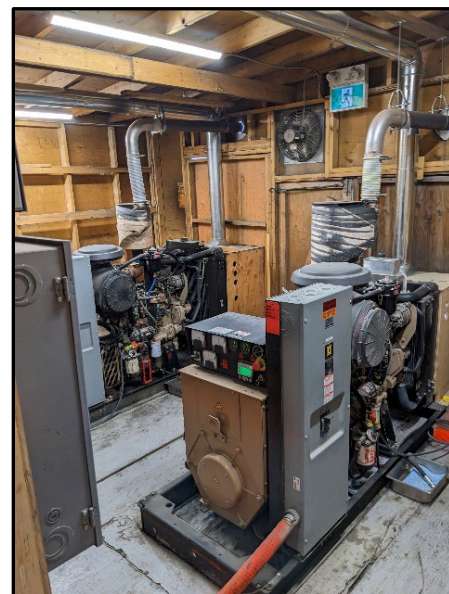
Figure 12: 75Kw and 100 Kw John Deere diesel generators (2023).
