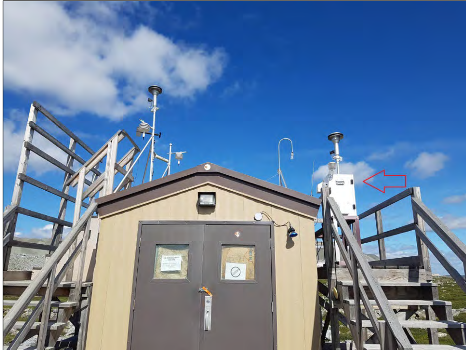
Photo 3.1-1 Continuous air monitoring building (CAMB)
