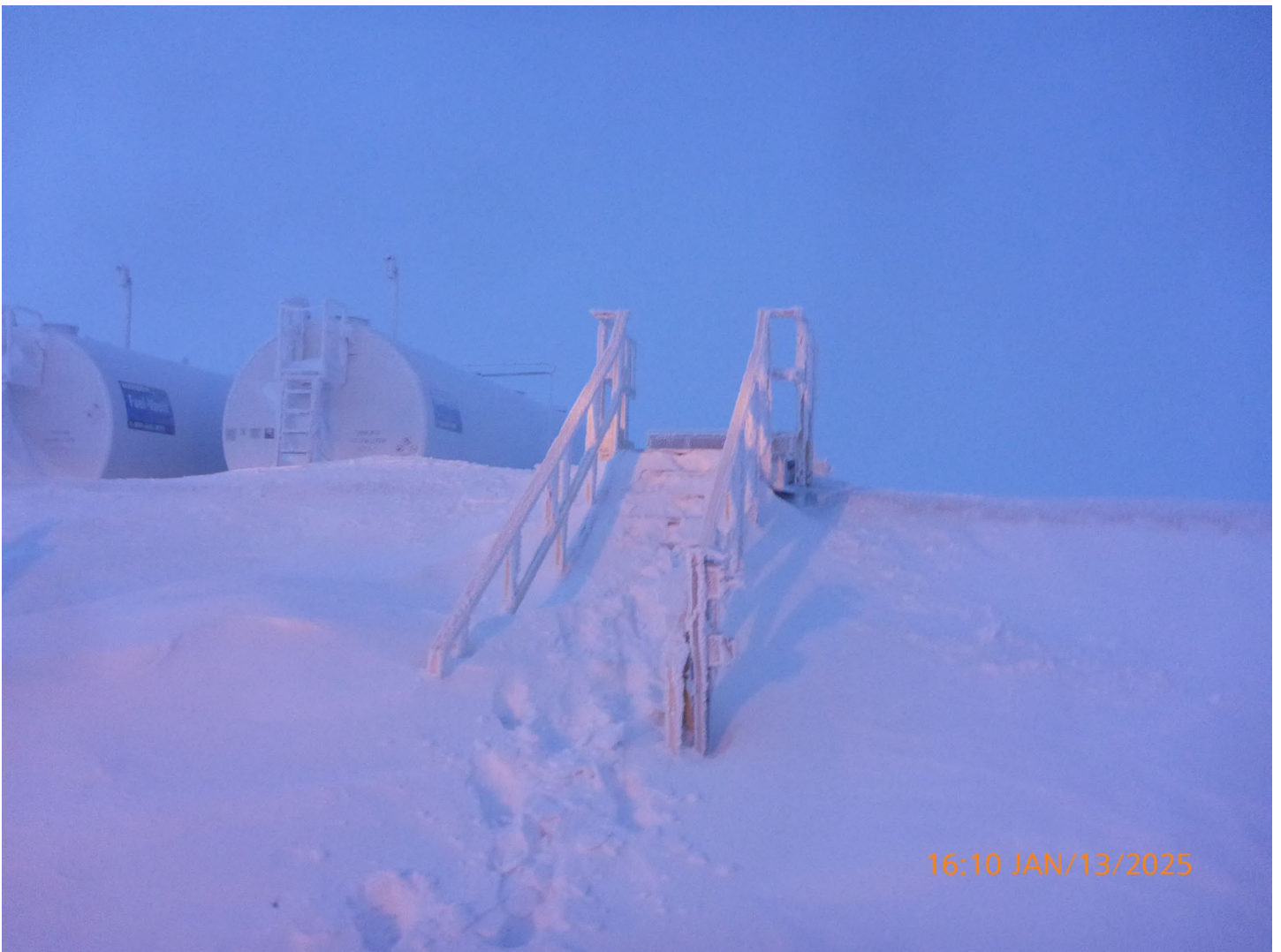
Photo 14 – Aviation Fuel Storage – The tank farm appears to be inspected regularly. The Inspector recommends that access to the tank farm be maintained to facilitate regular inspections.
