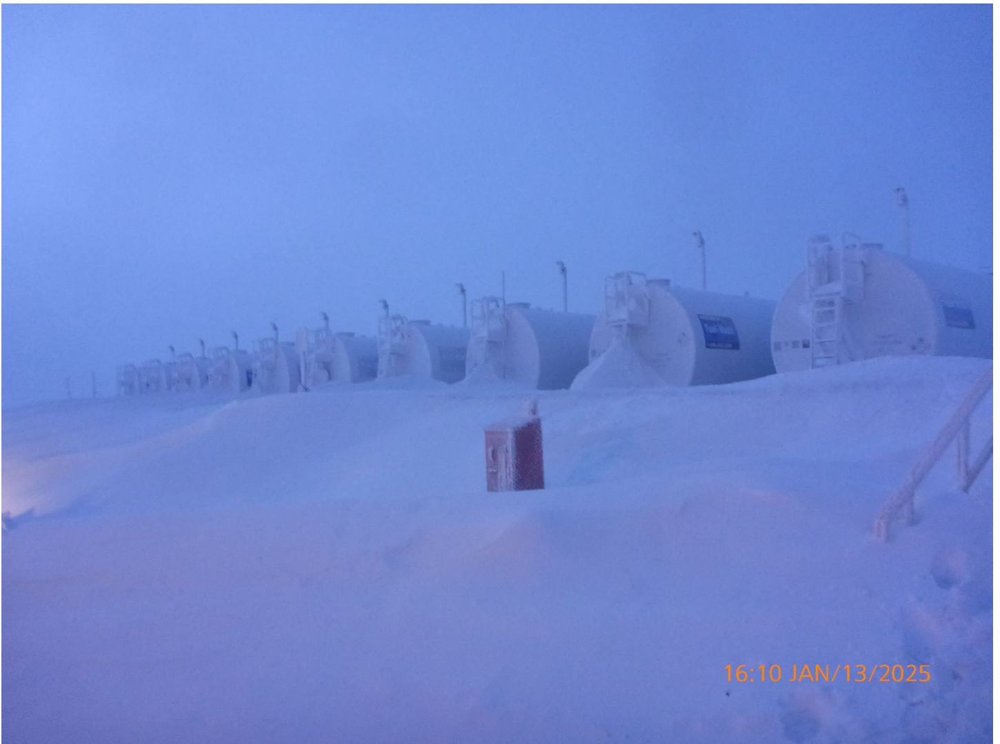
Photo 13 – Aviation Fuel Storage – Aviation fuel is stored in a 1 million litre tank farm located by the Drill Core Logging Facility. Jet A aviation fuel is transported on the winter road. The tank farm is located within a lined containment berm.
