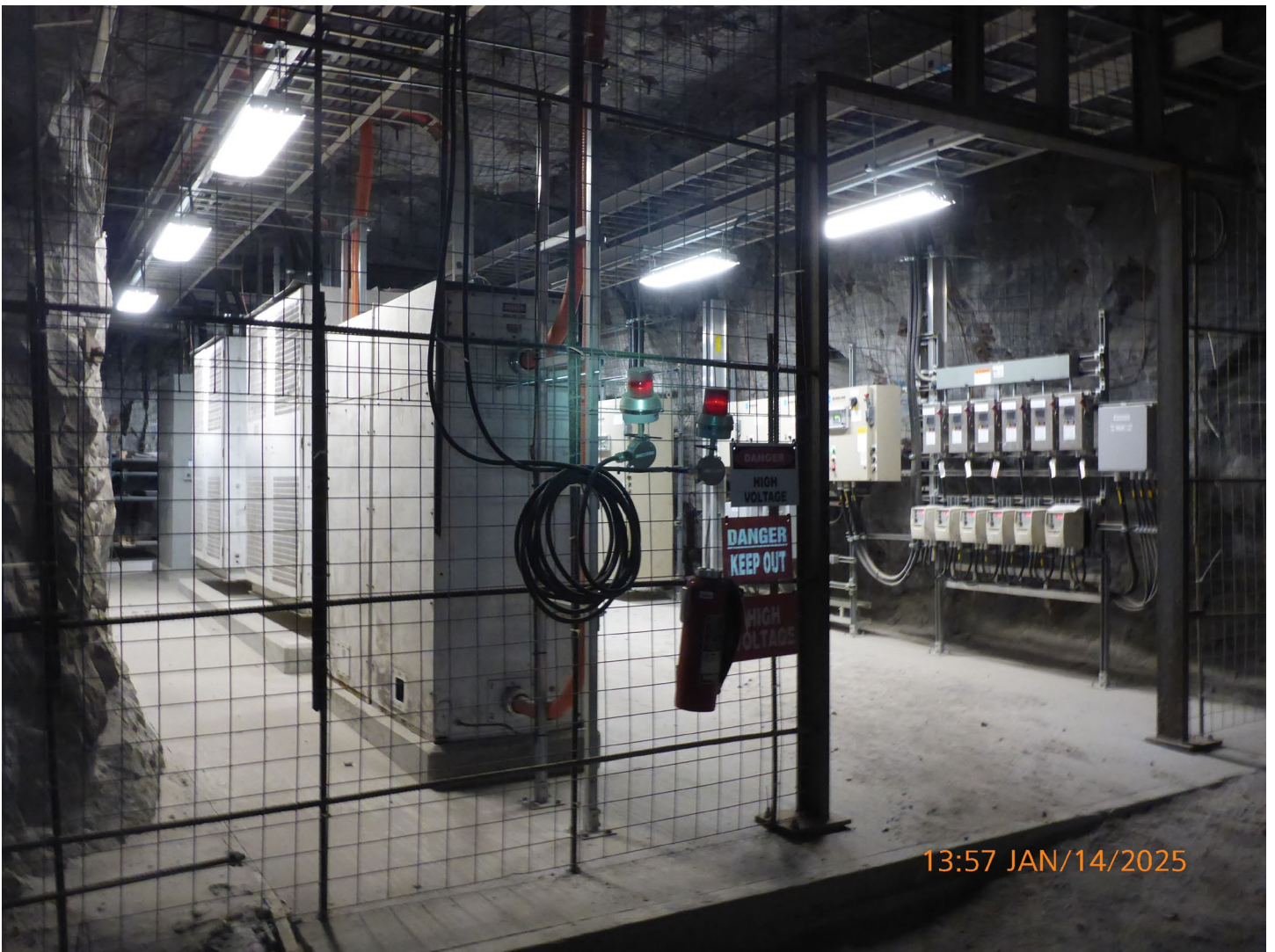
Photo 24 – Misery Underground – The underground electrical substation contains transformers and switch gear used to operate underground fans and pumps.
