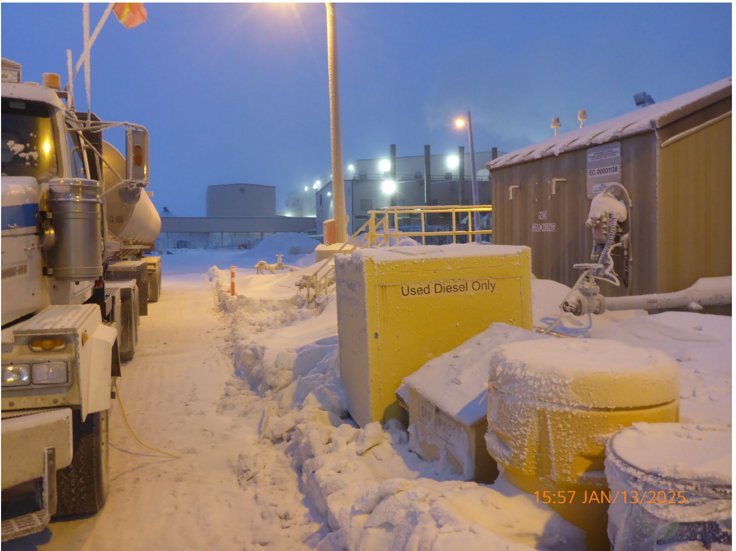
Photo 3 – Main Tank Farm Transfer Area – Spill response equipment was snowed in and not easily accessible. The spill response equipment needs to be dug out to allow for easy access.
