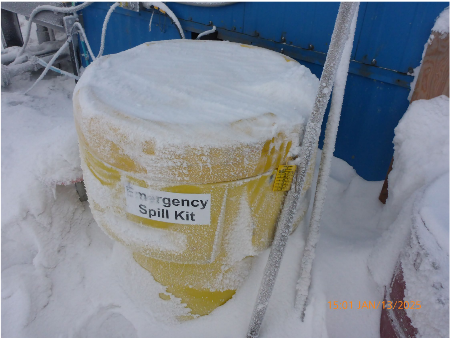
Photo 9 – Sable Refuelling – The spill kit was fully stocked, but buried in snow. The spill kit needs to be dug out to ensure easy access for spill response.
