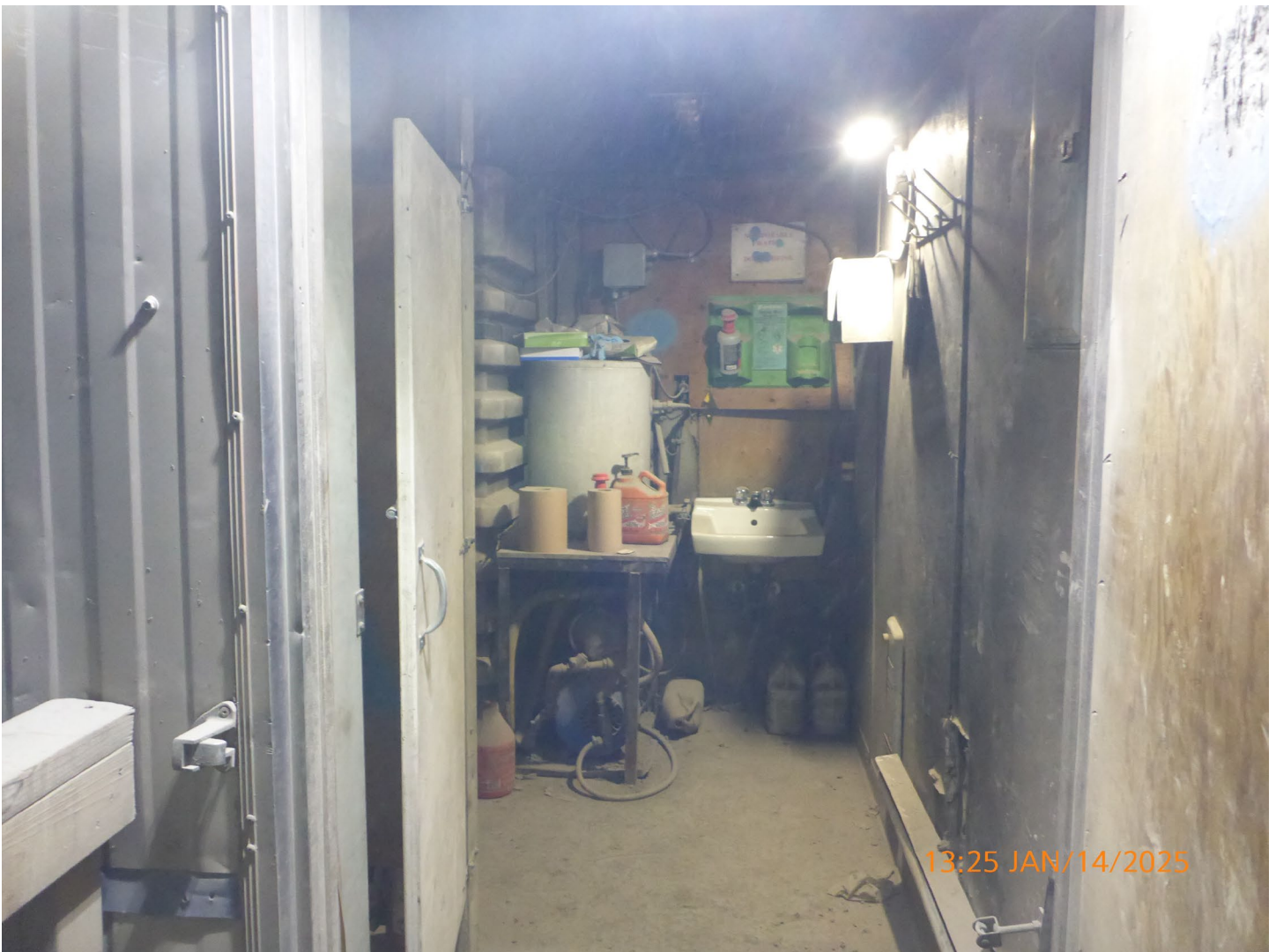
Photo 18 – Misery Underground – A washroom facility is located on the 2050 level of the mine. Waste is contained in a holding tank and transported to the Sewage Treatment Plant.
