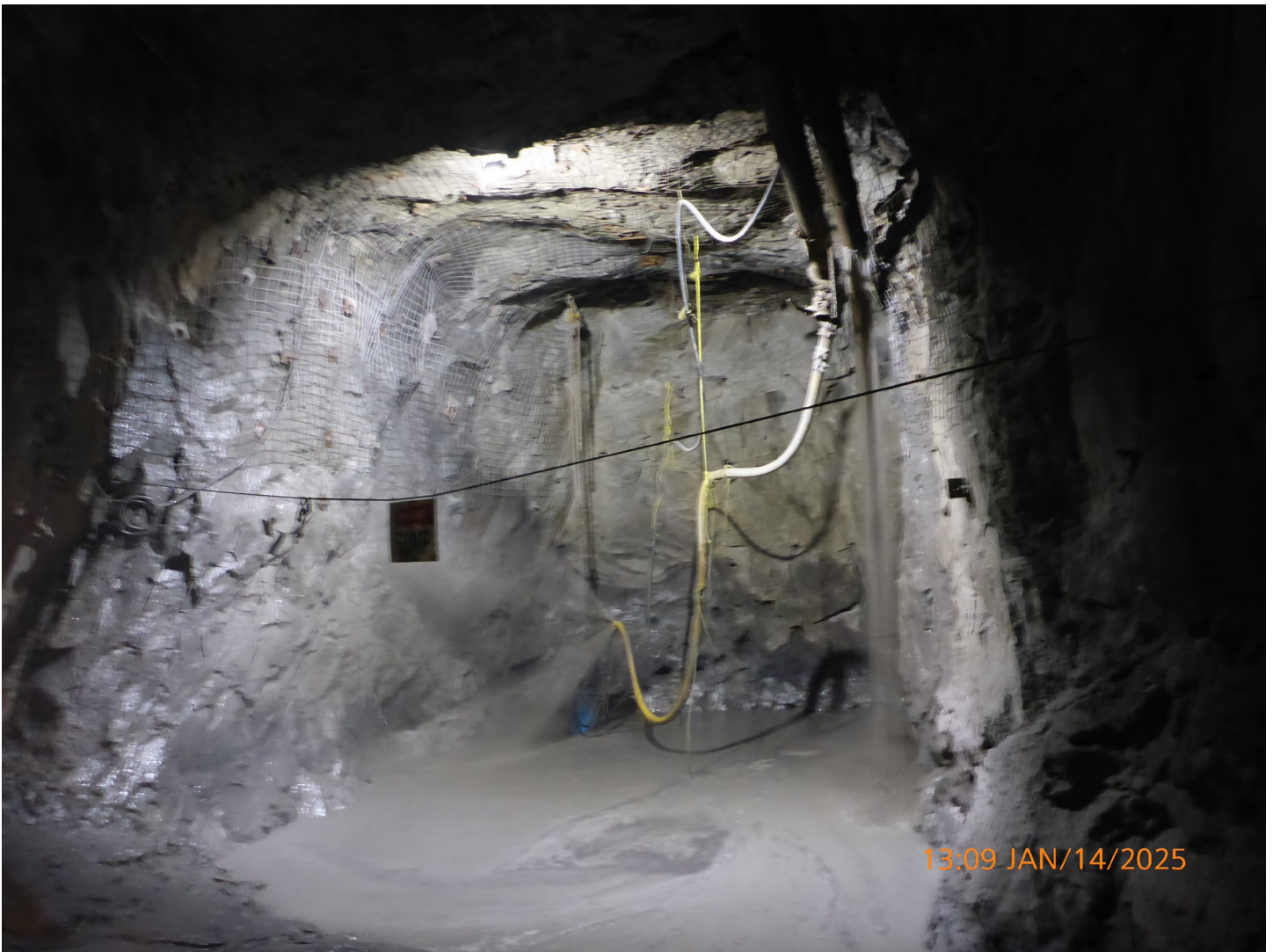
Photo 21 – Misery Underground – Water is collected in sumps on each level. Water is then pumped into the water collection system that reports to the Mud Wizard, and eventually to surface.
