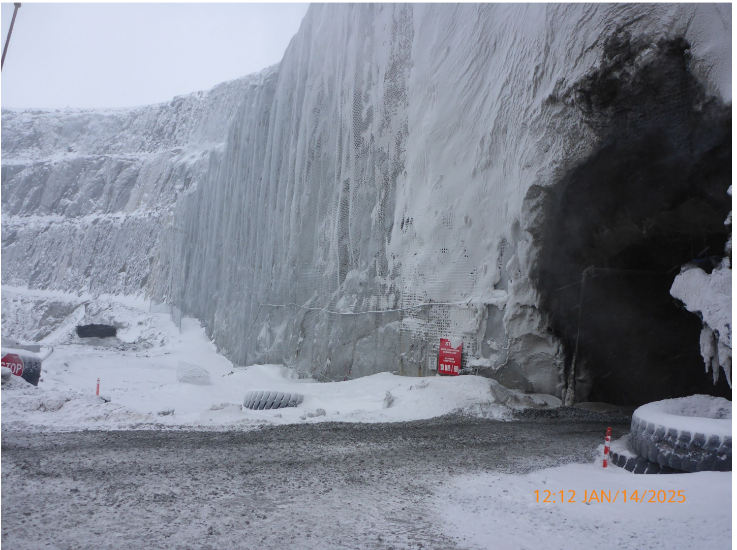
Photo 15 – Misery Underground – The opening of the Misery Underground portal is on the ramp of the Misery Pit. Ore is transported out of the mine and placed outside the portal, then transported to the Process Plant.
