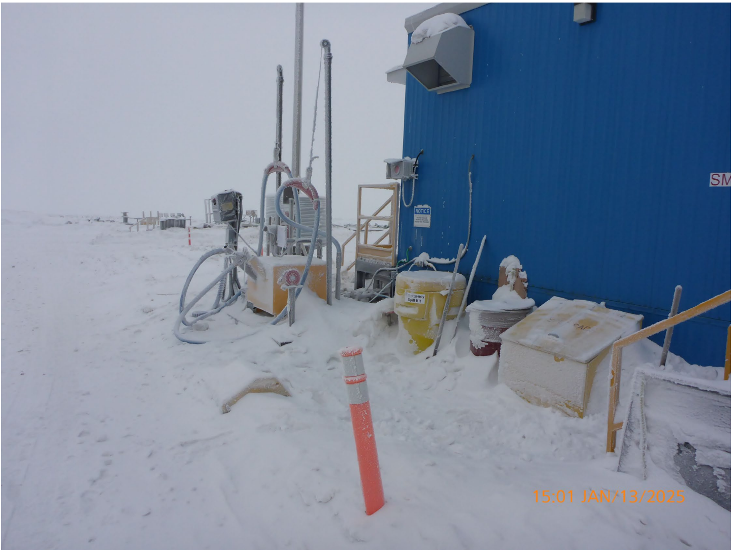
Photo 7 – Sable Refuelling – The Sable refuelling area was clean and well maintained with no indication of any hydrocarbon leaks or spills. Spill response equipment was fully stocked and easily accessible.
