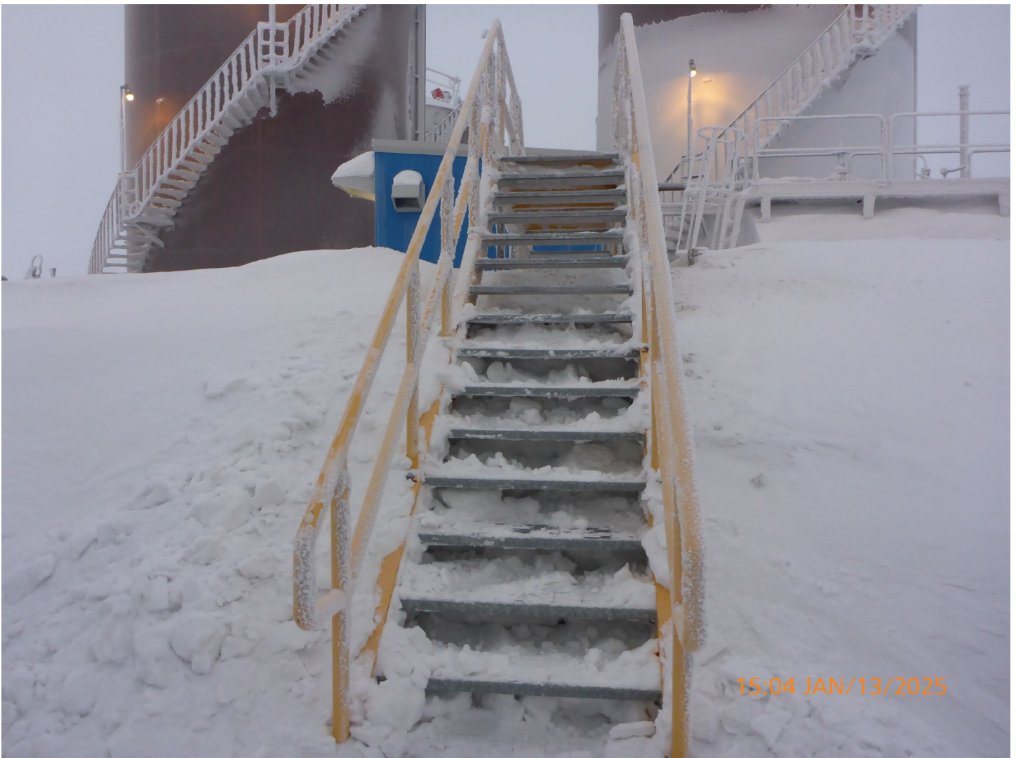
Photo 6 – Sable Tank Farm – Access to the Tank Farm is being maintained to facilitate regular inspections.
