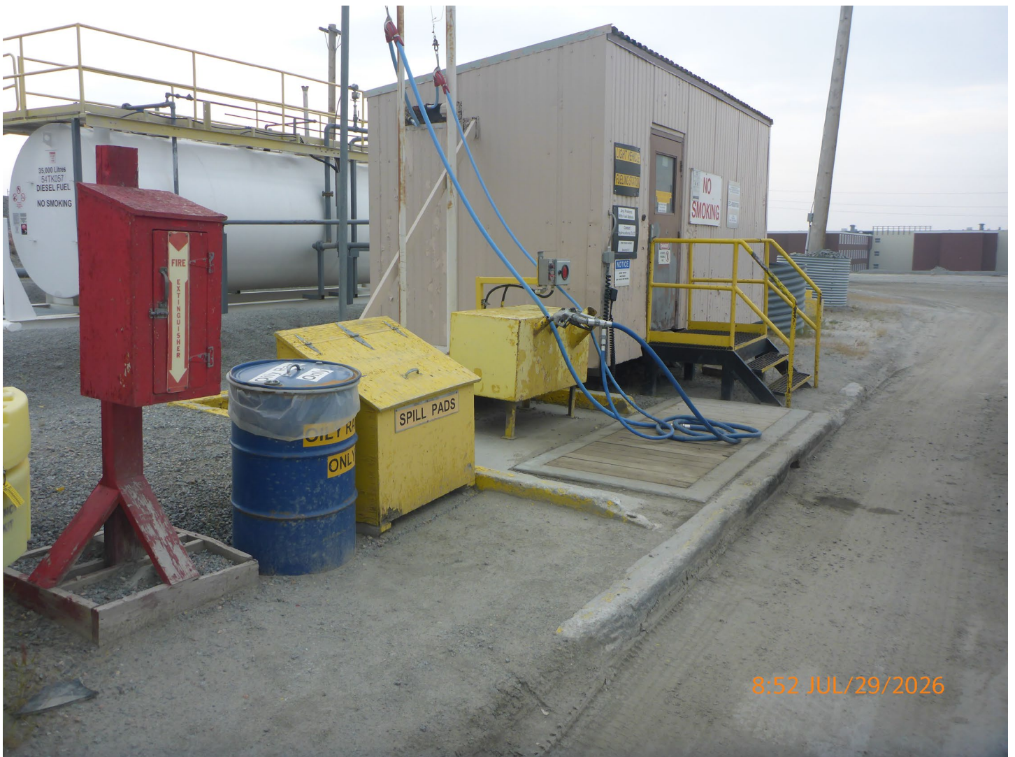
Photo 13 – Main Camp Refuelling – The Main Camp Refuelling station was clean and well maintained. Spill response equipment was fully stocked and easily accessible.
