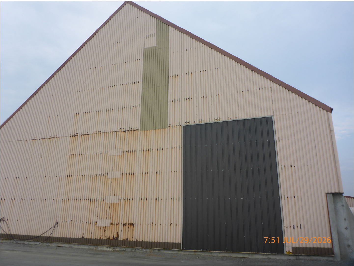
Photo 1 – Ammonium Nitrate Building – Repairs to the exterior siding of the AN Building are complete.
