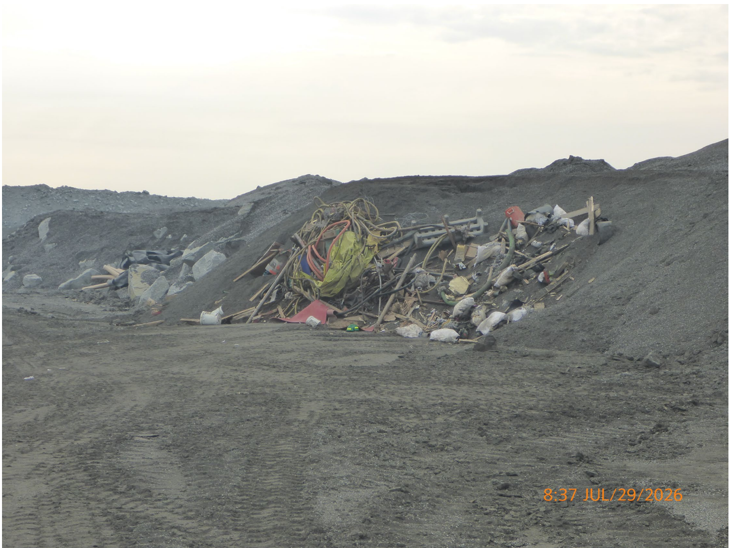
Photo 11 – Landfill – The Landfill has been recently covered with Coarse Kimberlite Rejects from the Process Plant.
