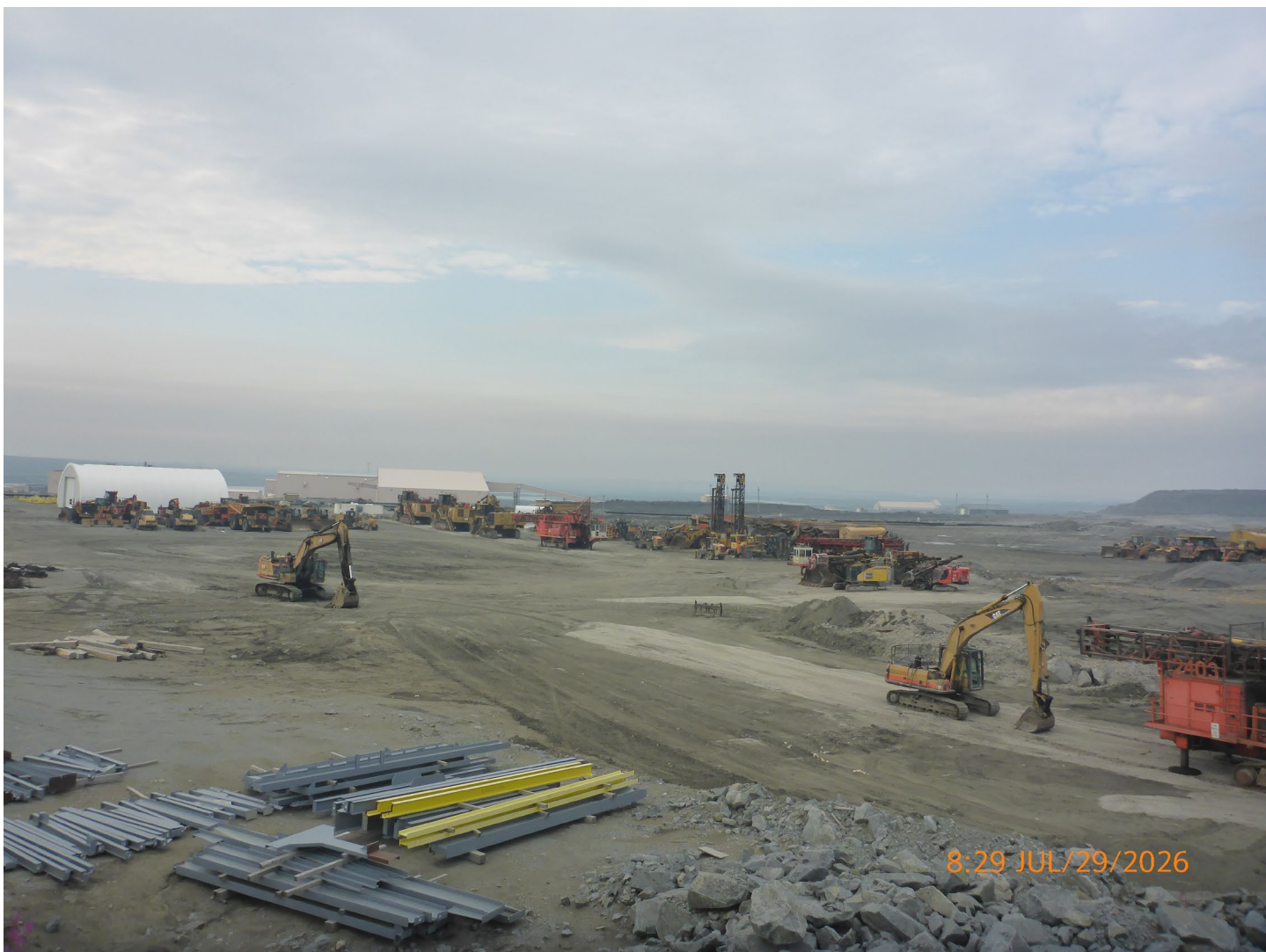
Photo 7 – Zone 12 – Several units from the mobile equipment fleet are being stored in Zone 12 of the Panda/Koala Waste Rock Pile during care and maintenance.
