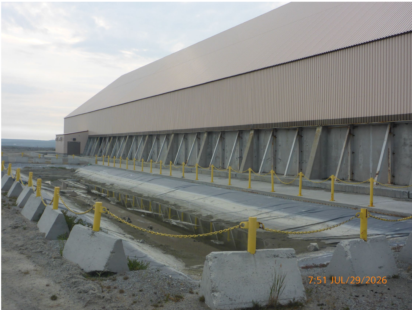
Photo 4 – Ammonium Nitrate Building – The area around the AN Building is graded toward lined sumps that are designed to contain any contaminated runoff. The sumps were empty and have plenty of capacity.
