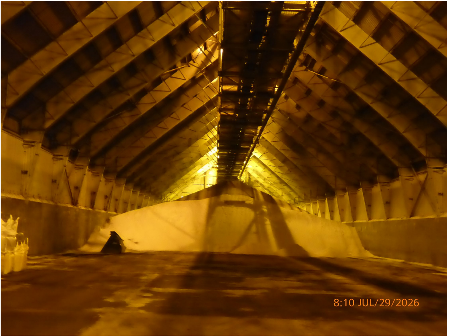
Photo 6– Ammonium Nitrate Building – Approximately 4.6 million kilograms of Ammonium Nitrate is currently stored in the Building.
