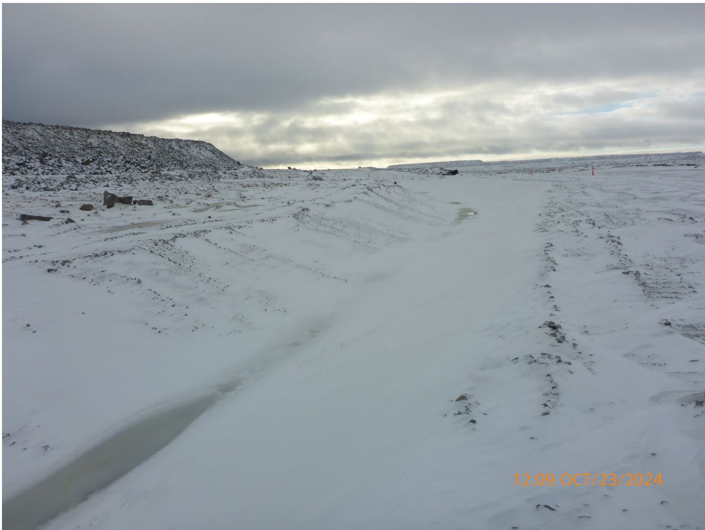
Photo 2 – Point Lake Project – WRSA Perimeter trench construction is continuing. The trench is lined and graded toward a collection sump.
