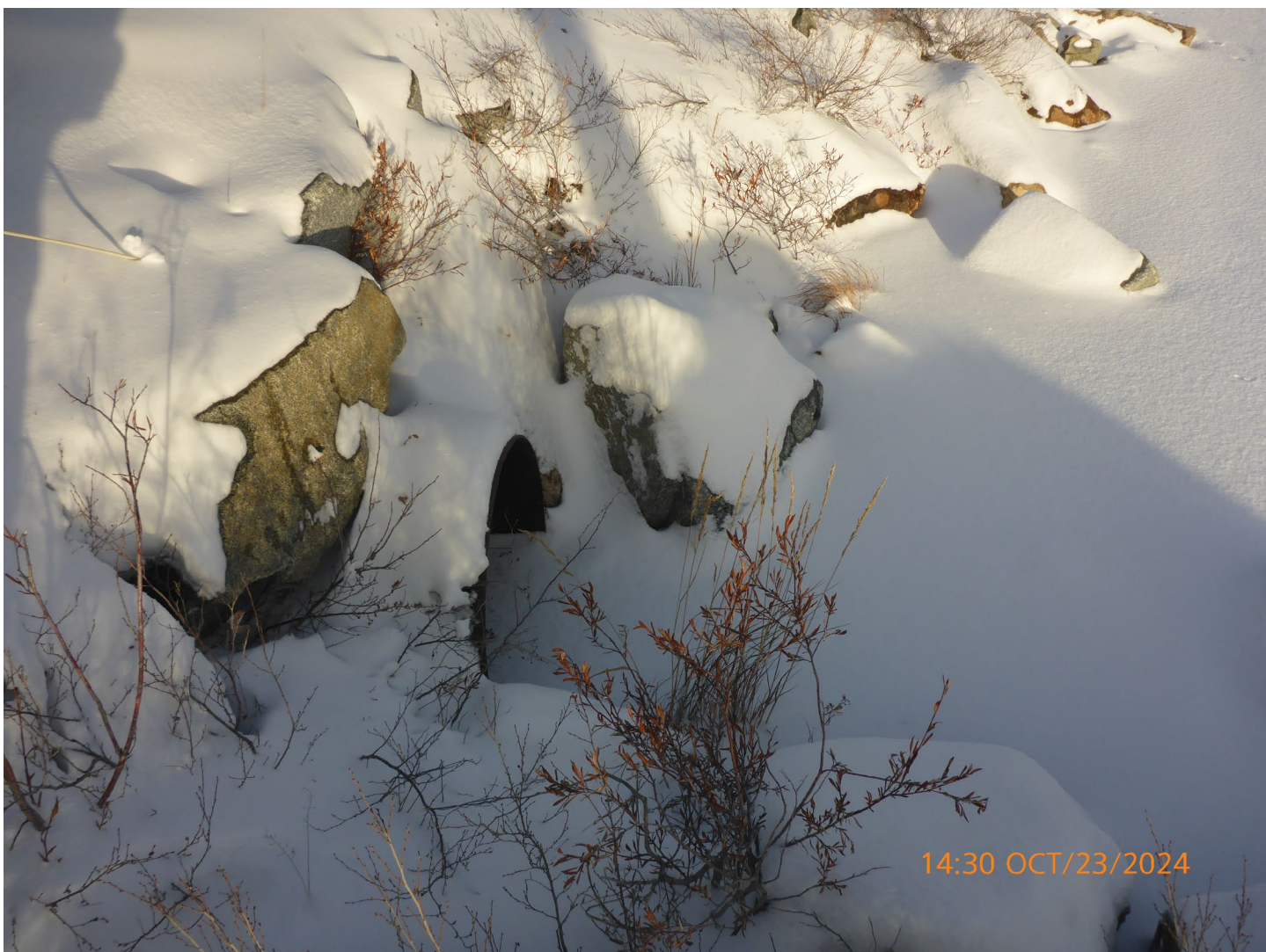
Photo 26 – PDC Culverts – The culverts along the PDC are beginning to fill in with snow. Normally Ekati staff will cover these culverts to prevent them from becoming packed with snow. A packed culvert will potentially create a flooding situation in the spring. Culverts along the PDC and the Airstrip are of particular concern. Arctic should cover these culverts as soon as possible.
