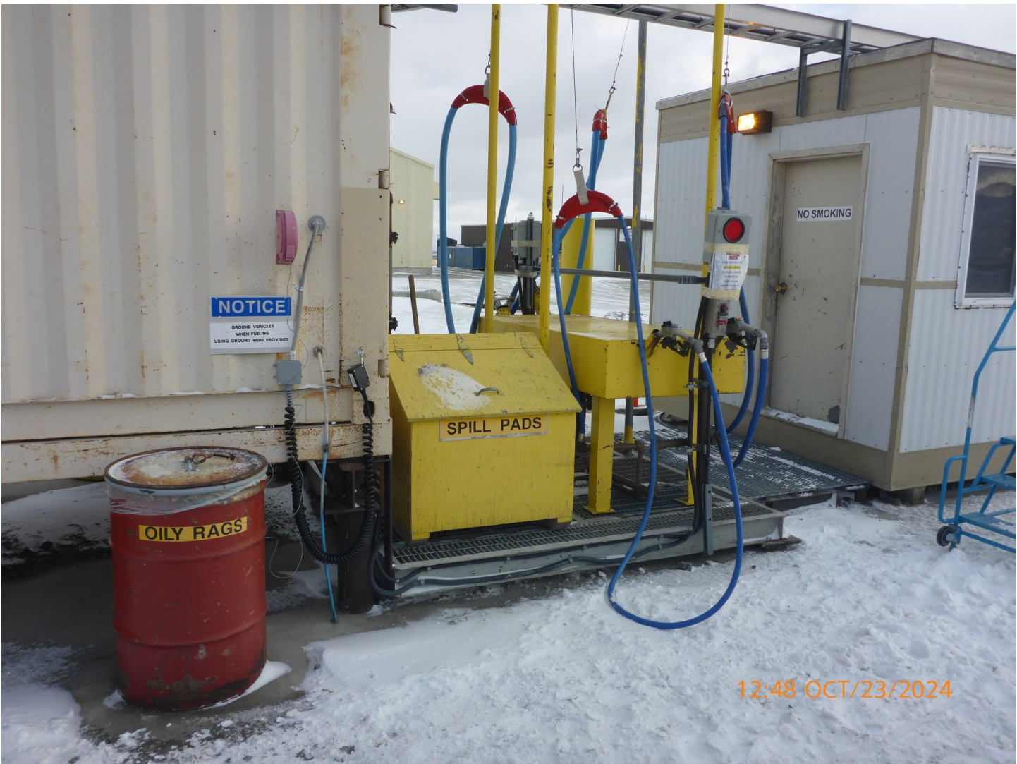
Photo 7 – Misery Refuelling Station – The refuelling station was clean and well organized with no indication of any leaks or spills. Spill response equipment was fully stocked and easily accessible.
