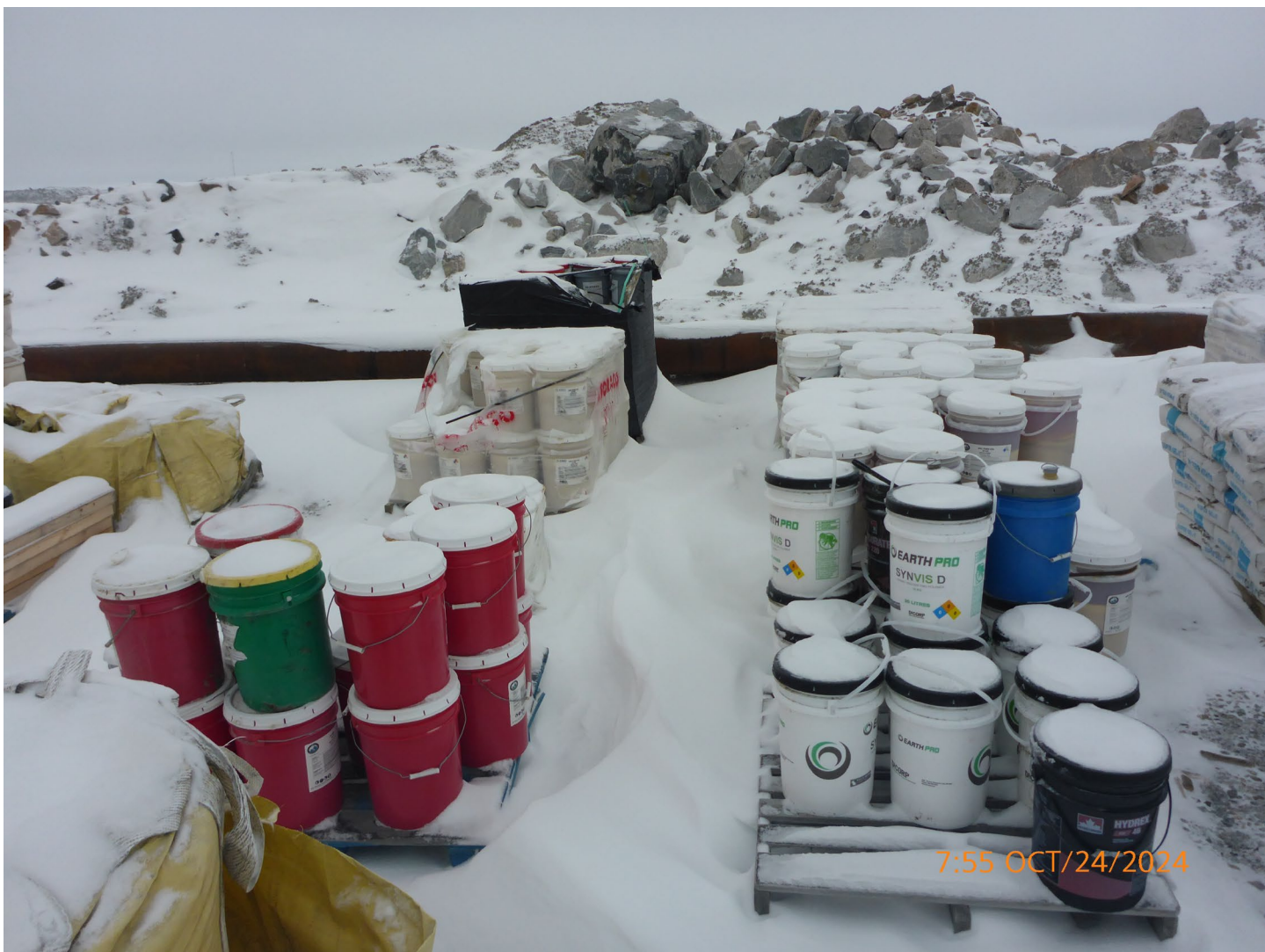
Photo 33 – Sable Drilling – Drilling additives are stored out of the way on pallets to prevent breakage and spills.
