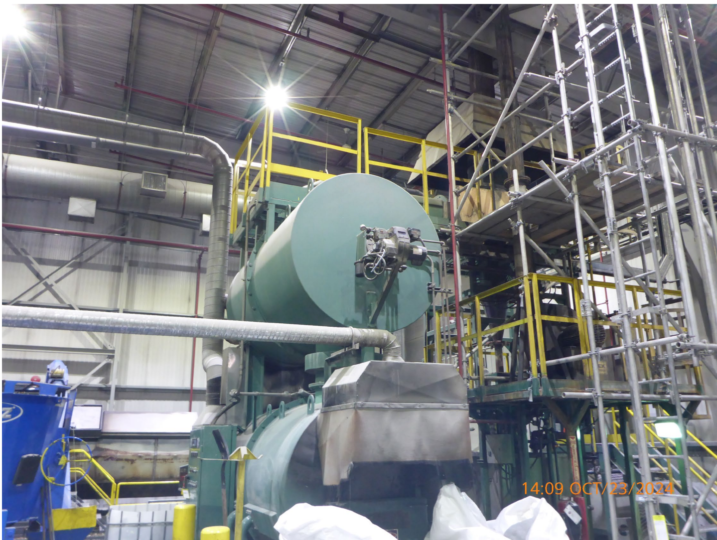
Photo 22 – Incinerator Building – Ekati is equipped with two dual chambered incinerators. The incinerators were scheduled for tuning and stack testing in the summer of 2024; however the testing was not able to proceed.
