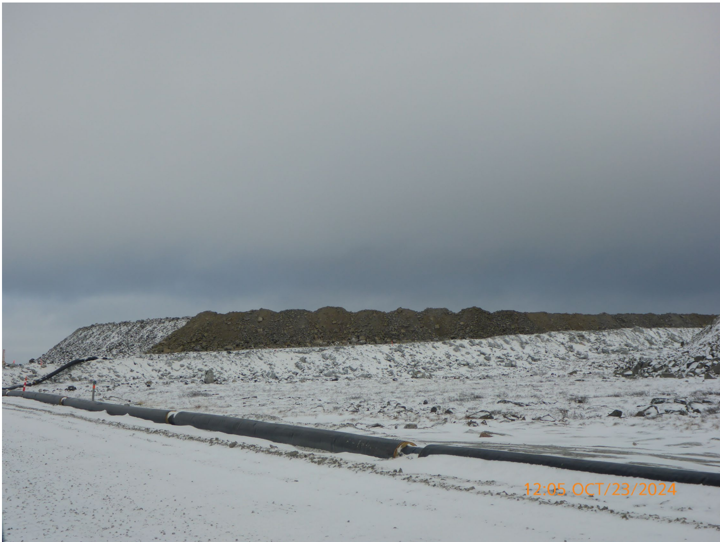
Photo 1 – Point Lake Project – Waste rock is being placed in the Point Lake WRSA
