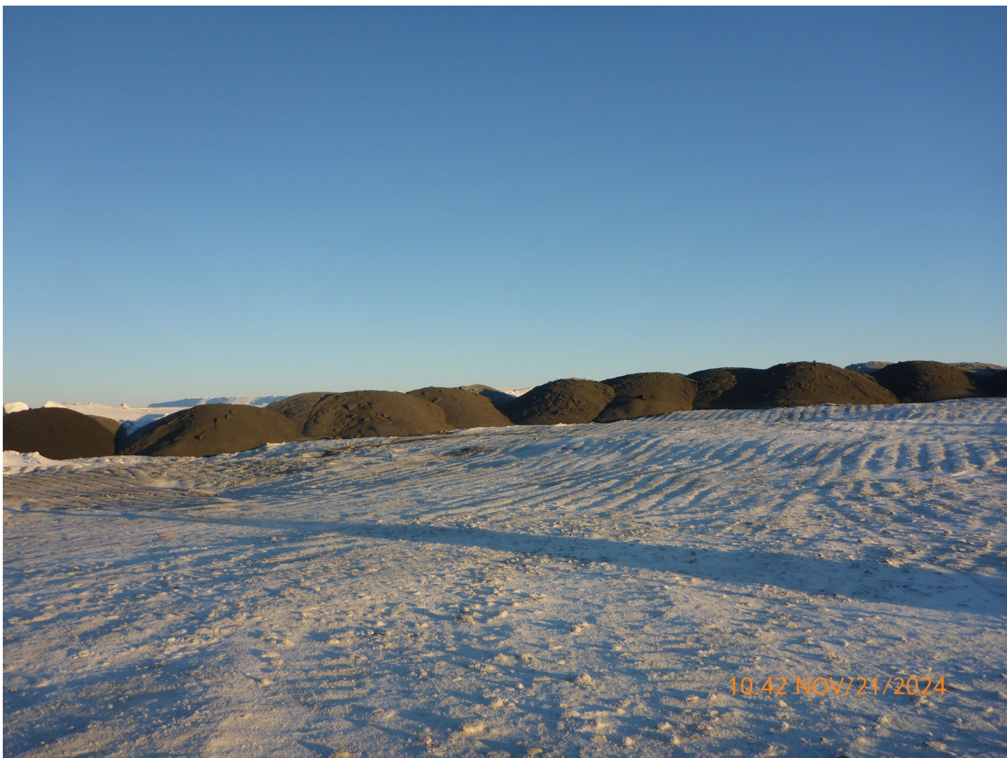
Photo 21 – Coarse Processed Kimberlite Dump – The coarse processed kimberlite disposal area is being placed as per the Wastewater Processed Kimberlite Management Plan. Coarse Kimberlite is also used to cap the landfill in between lifts.
