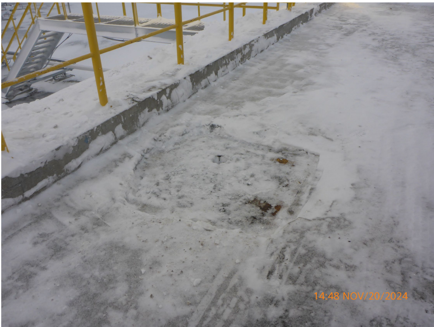
Photo 9 – Misery Refuelling Station – The containment sump at the Misery Refuelling station has been chipped out and is free of ice. The sump is functional and should contain any future spills.
