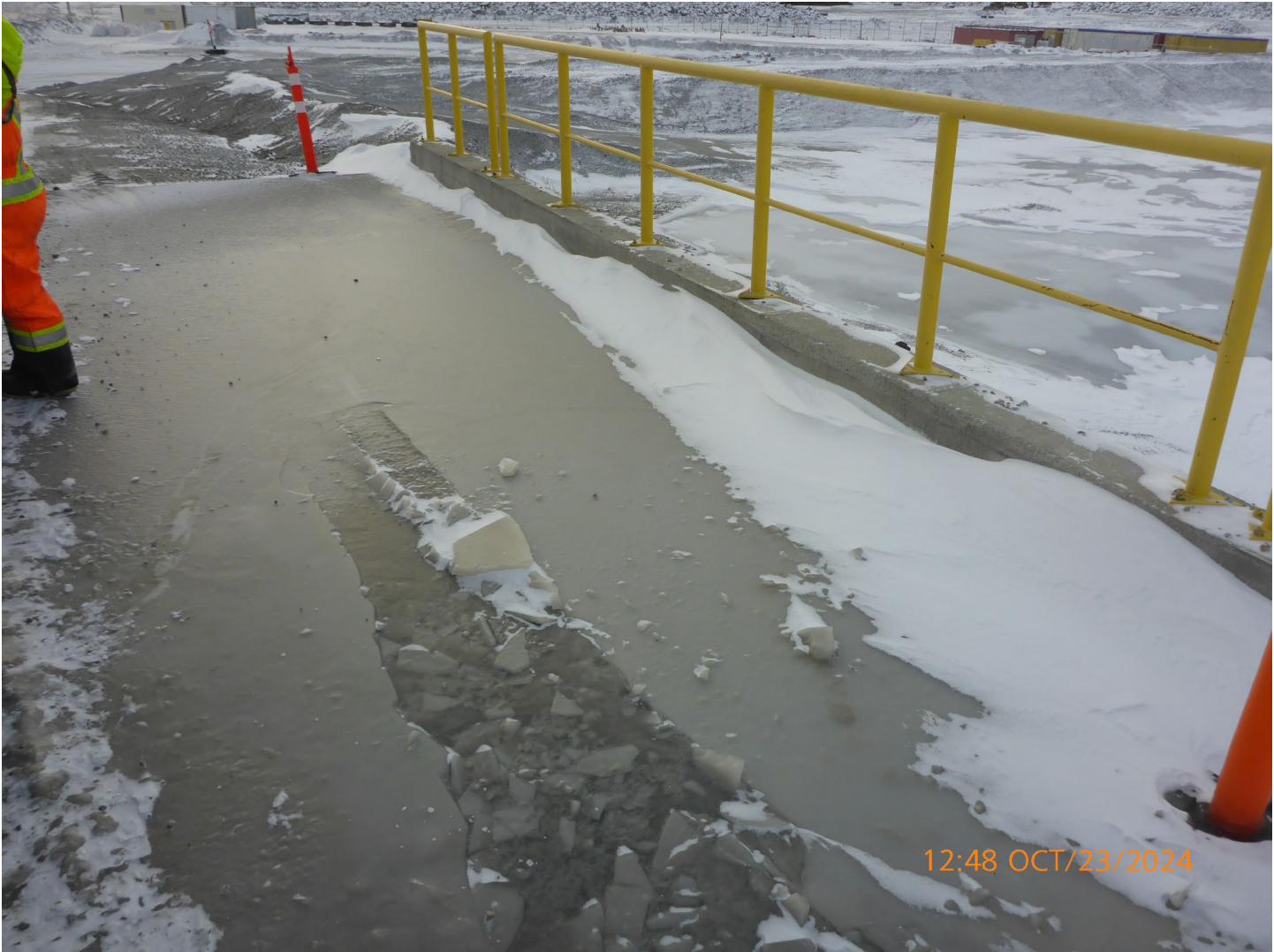
Photo 8 – Misery Refuelling Station – The containment sump at the Misery refuelling station was iced over. This will need to be cleaned out in order to provide spill containment capacity.
