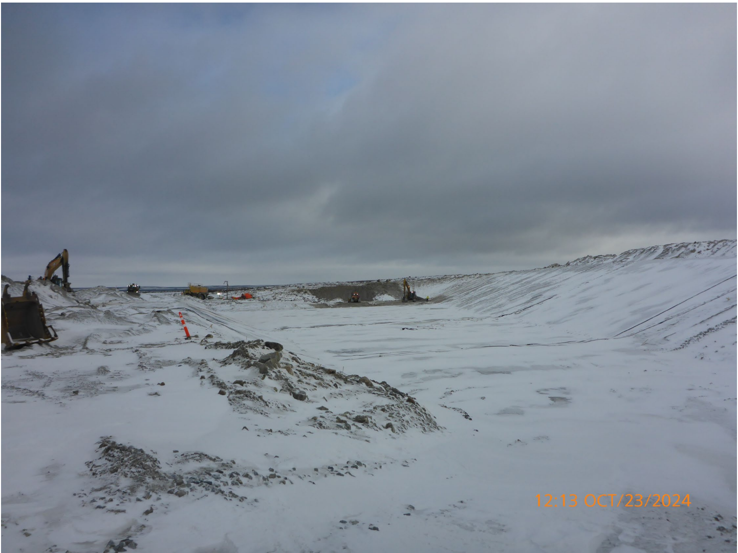
Photo 3 – Point Lake Project – Collection sump is designed to catch any runoff from the Point Lake WRSA. Water is then intended to be pumped into King Pond or the Lynx Pit.
