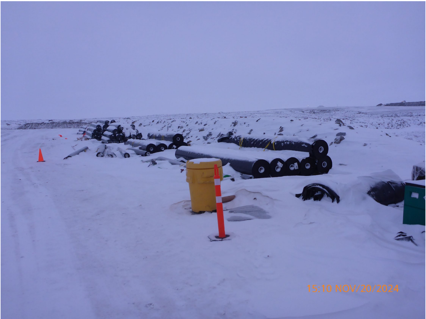
Photo 4 – Point Lake Project – Liner material is being staged along the Point Lake road.
