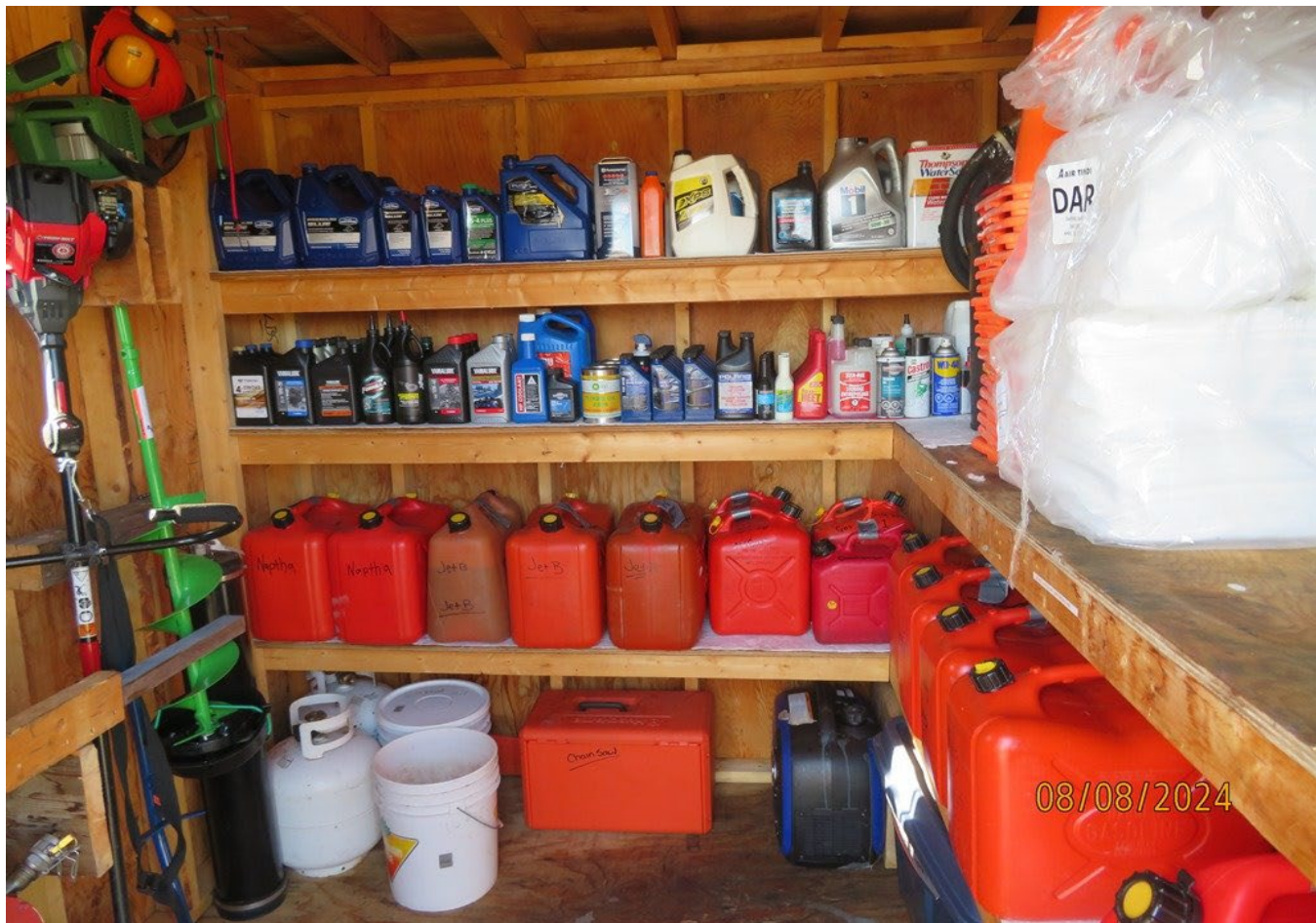
Figure 10 Absorbent pads and secondary containment are used where a possibility of leak is present.
