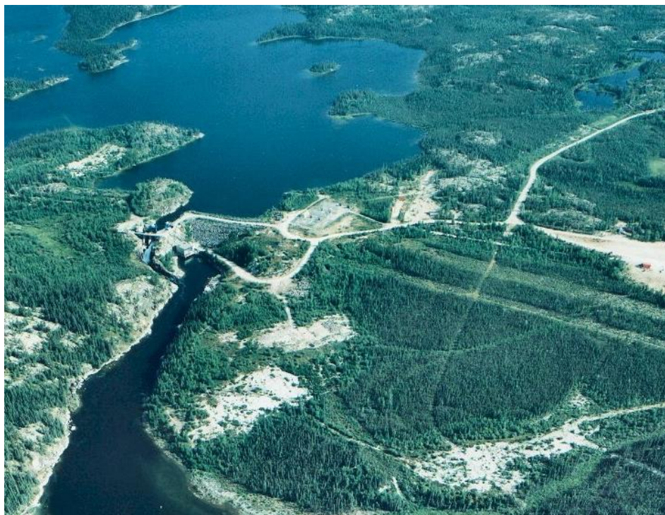
Figure 3: Snare Falls Generating Station, showing all core infrastructure within 200 m radius and dam above an existing waterfall; 15.5 km downstream of Snare Rapids.
