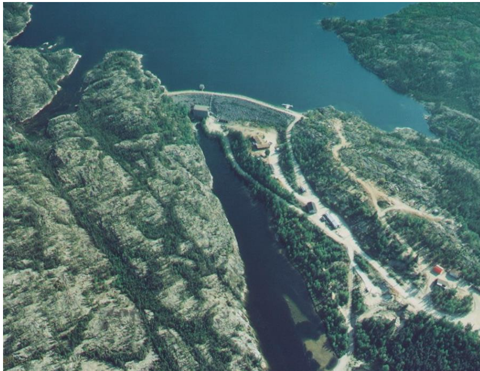
Figure 2: Snare Rapids Generating Station; Bigspruce Reservoir in background; Spillway 5b not shown.
