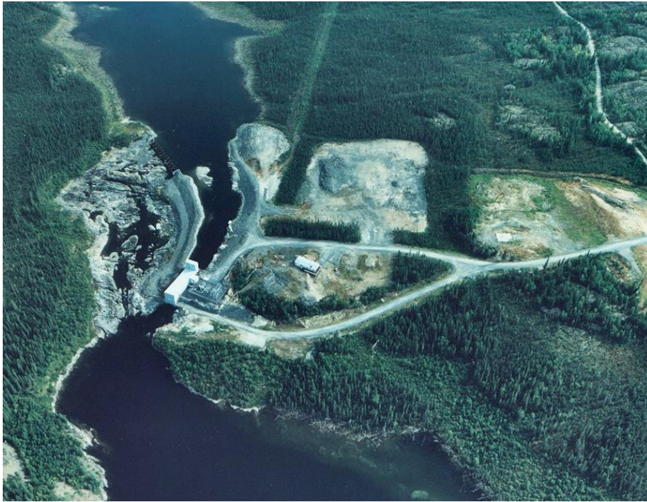
Figure 4: Snare Cascades Generating Station, natural channel adjacent to dam serves as spillway; dam built above a steep chute or series of rapids, 3 km downstream from Snare Falls.
